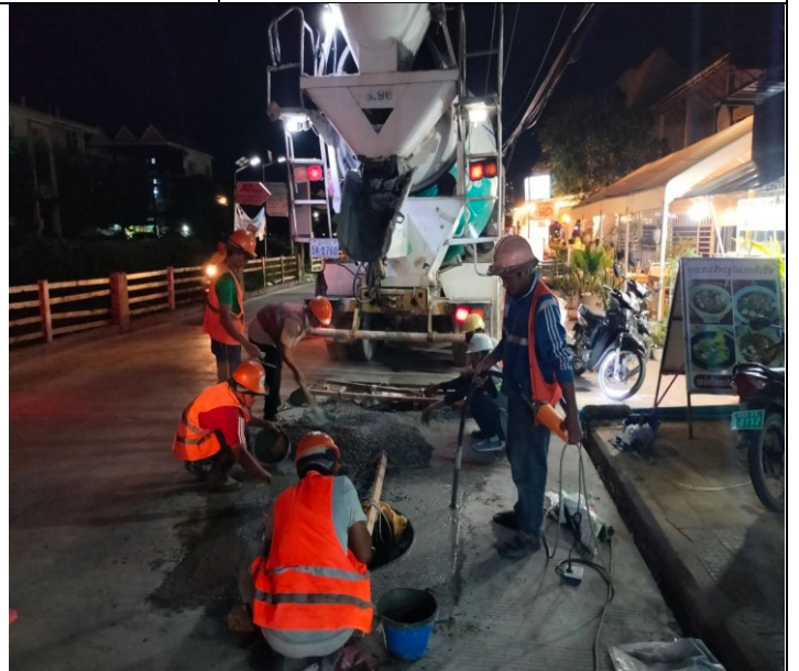
Photo: 06 Manhole Cover Instalation activity
