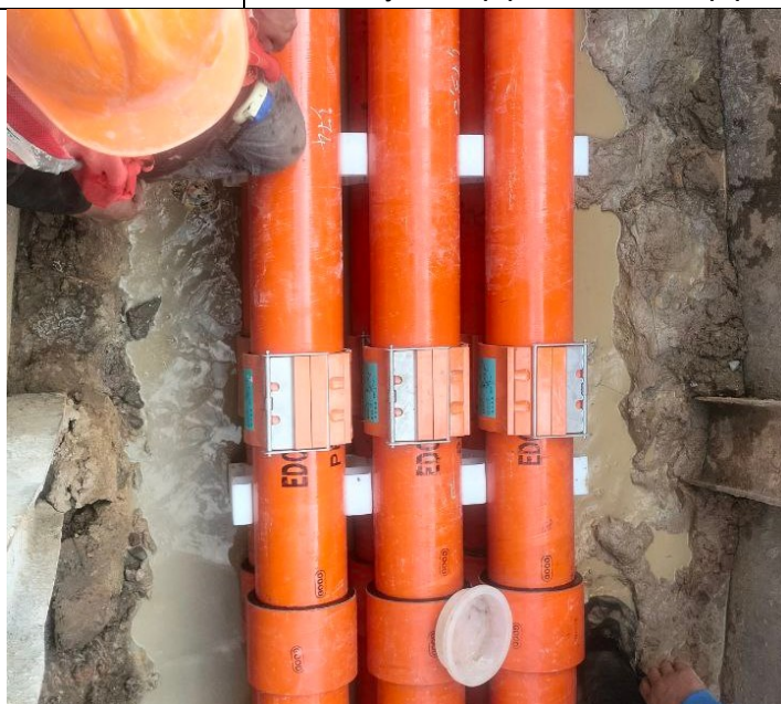
Photo: 24 Assembly PFP pipes and OFC pipe
