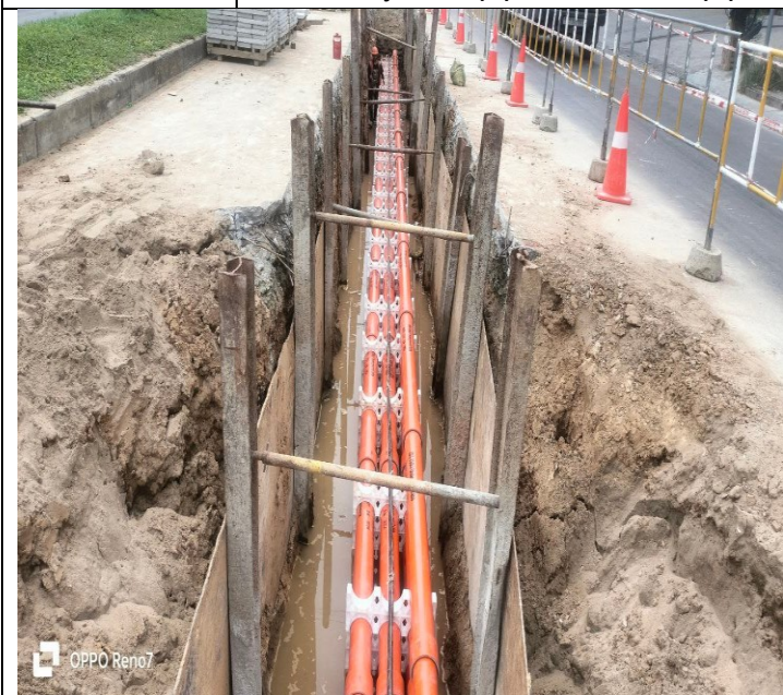
Photo: 23 Assembly PFP pipes and OFC pipe
