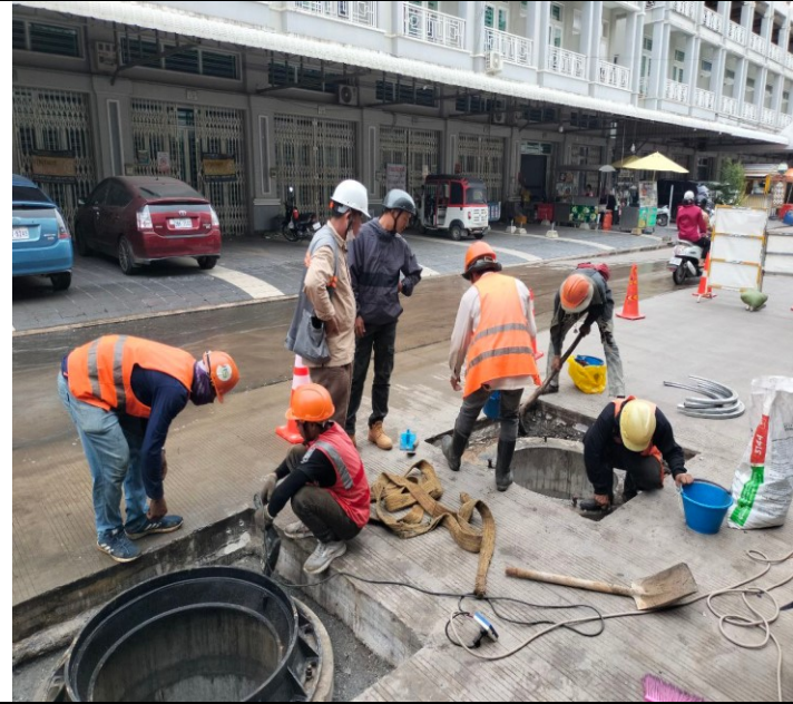
Photo: 01 Manhole Cover Instalation activity
