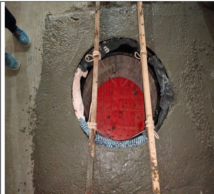
Photo: 07 Manhole Cover Installation activity
