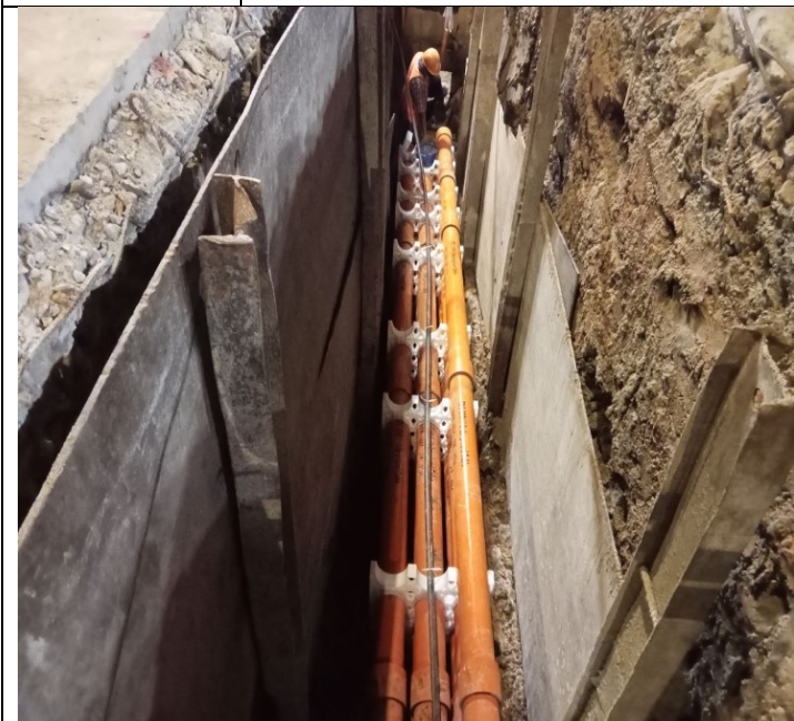
Photo: 09 Assembly PFP pipes and OFC pipe
