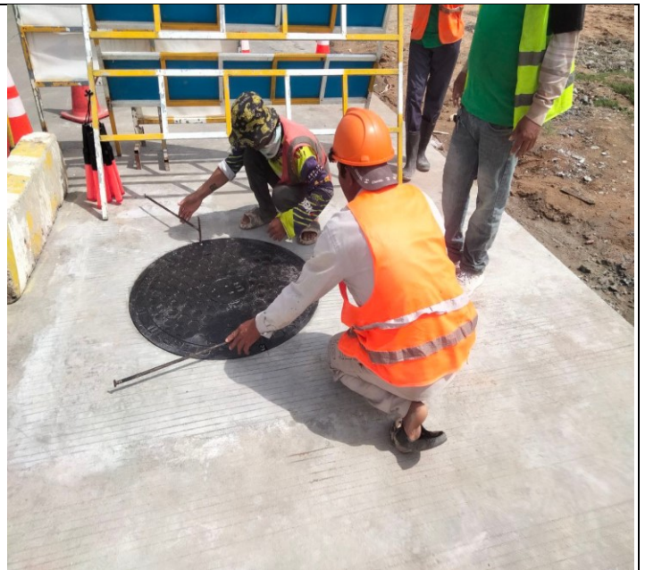
Photo: 14 Manhole Cover Installation activity
