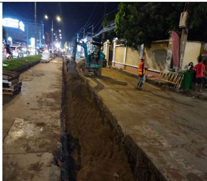
Base course backfilling and compaction
