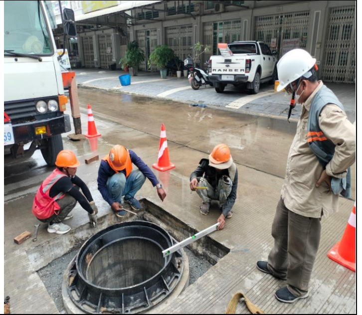
Photo: 02 Manhole Cover Instalation activity
