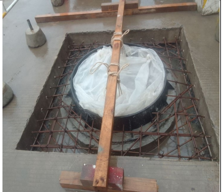
Photo: 04 Manhole Cover Instalation activity
