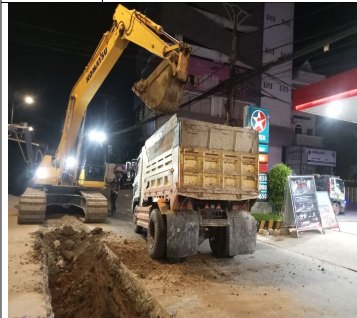
Photo: 15 Soil excavation and concrete road
