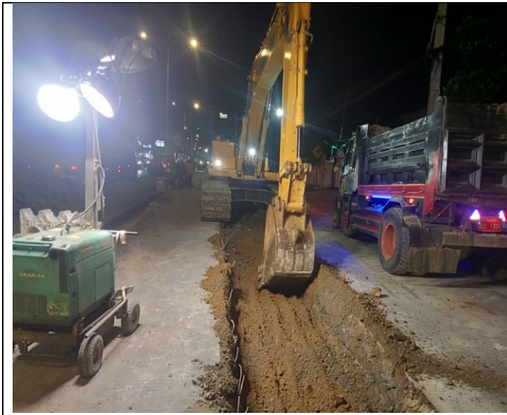
Soil excavation and concrete road
