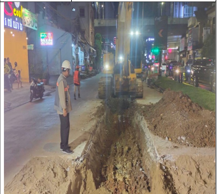
Soil excavation and concrete road
