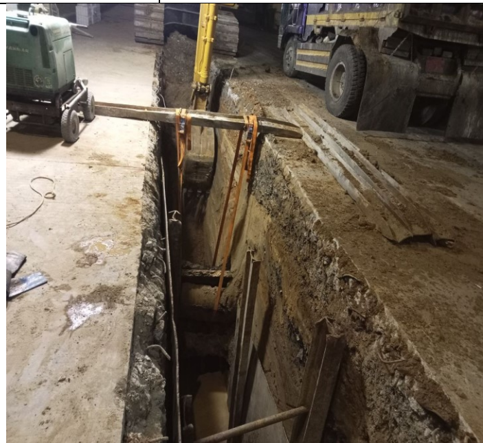
Photo: 16 Soil excavation and concrete road
