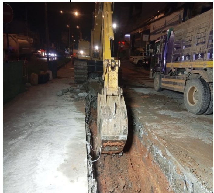
Photo: 10 Soil excavation and concrete road
