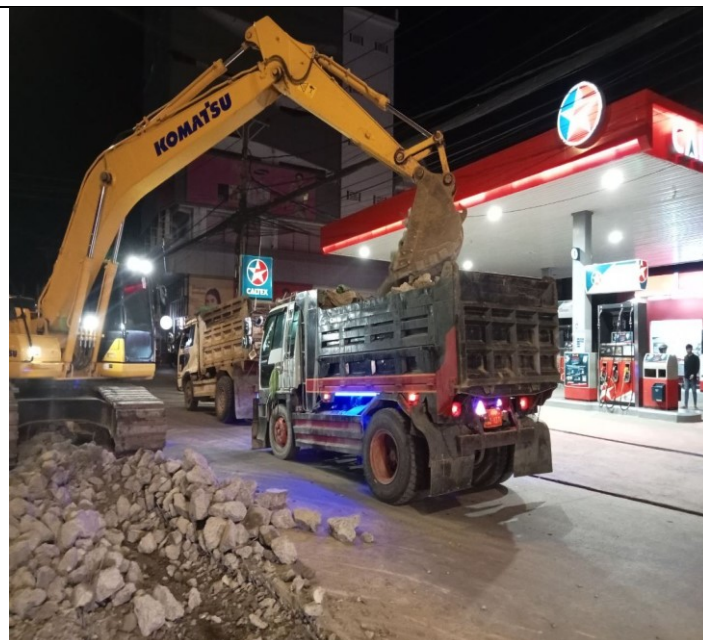
Photo: 14 Soil excavation and concrete road
