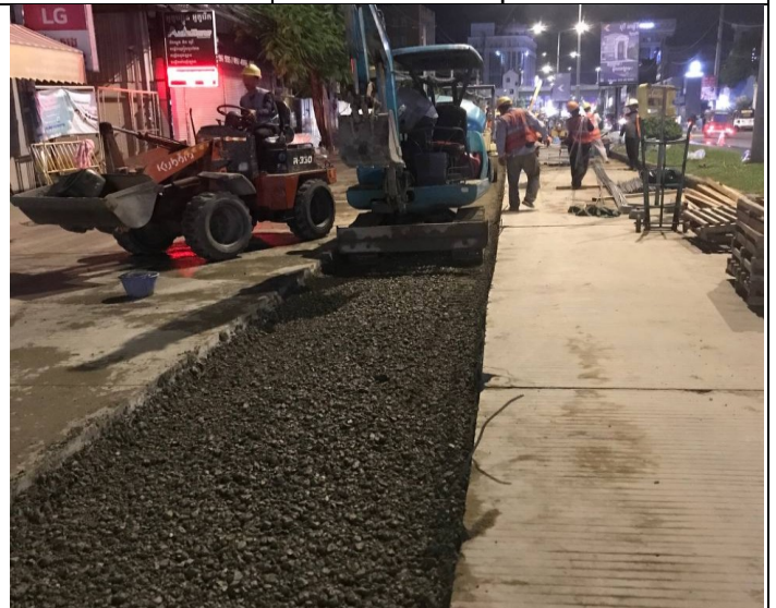
Base course backfilling and compaction
