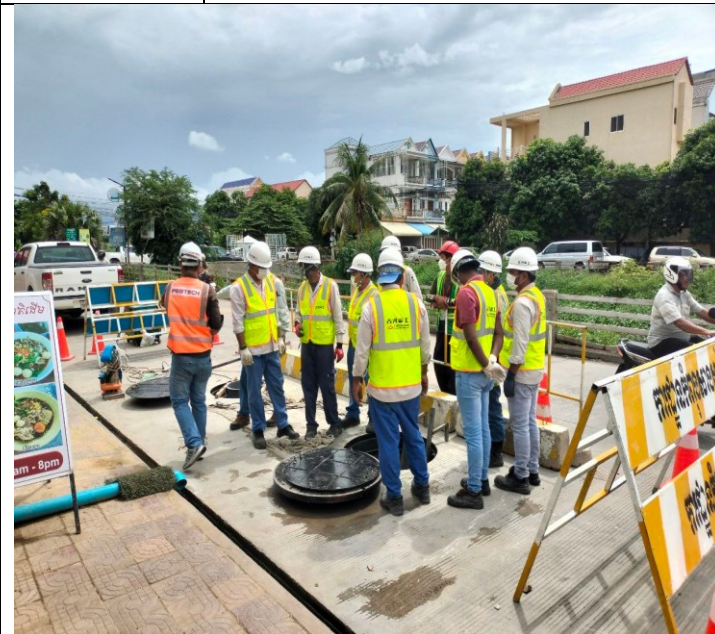
Photo: 17 Manhole Cover Installation activity
