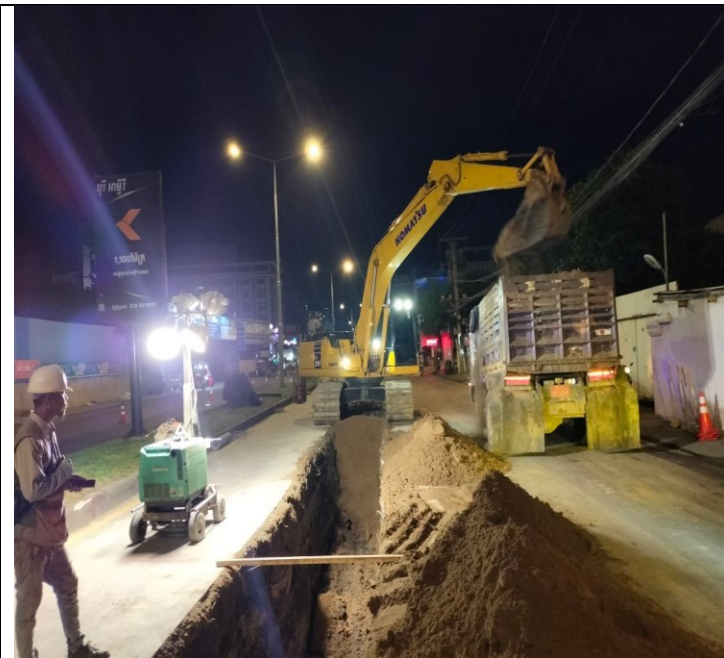
Photo: 07 Soil excavation and concrete road
