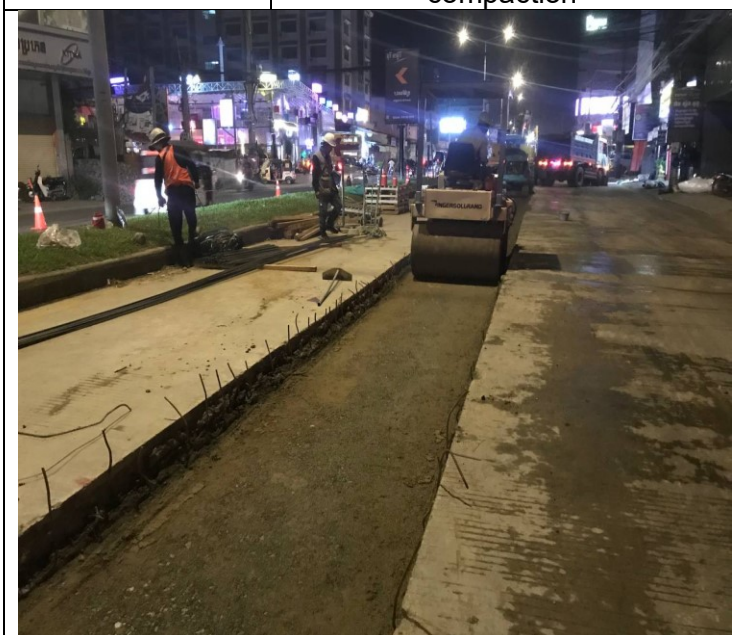
Base course backfilling and compaction
