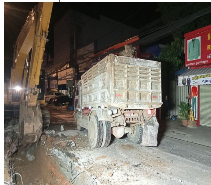
Photo: 11 Soil excavation and concrete road
