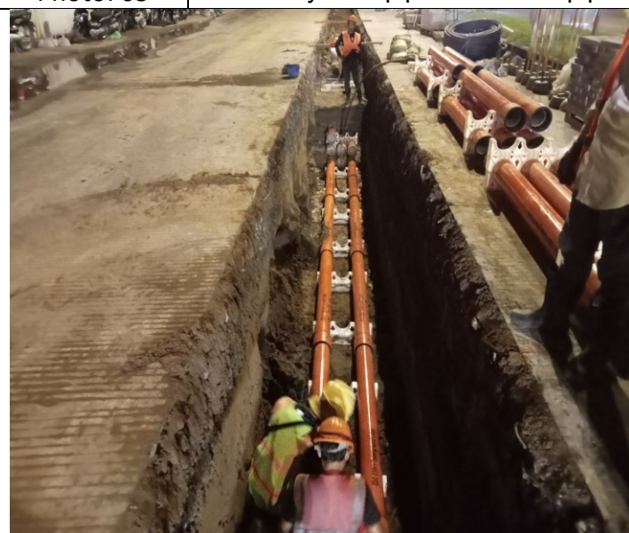
Photo: 05 Assembly PFP pipes and OFC pipe
