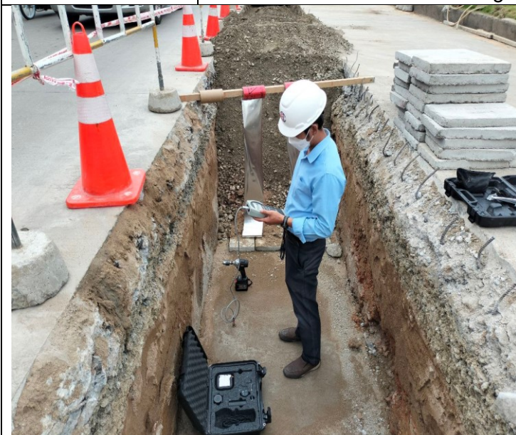
Photo: 03 Thermal test of Sand backfilling
