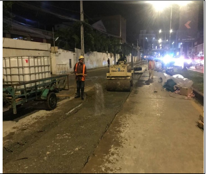
Base course backfilling and compaction
