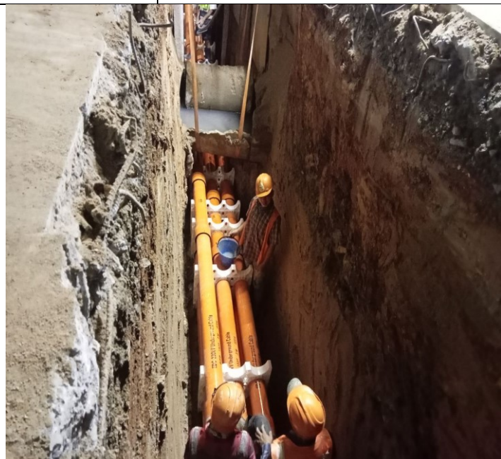
Photo: 10 Assembly PFP pipes and OFC pipe
