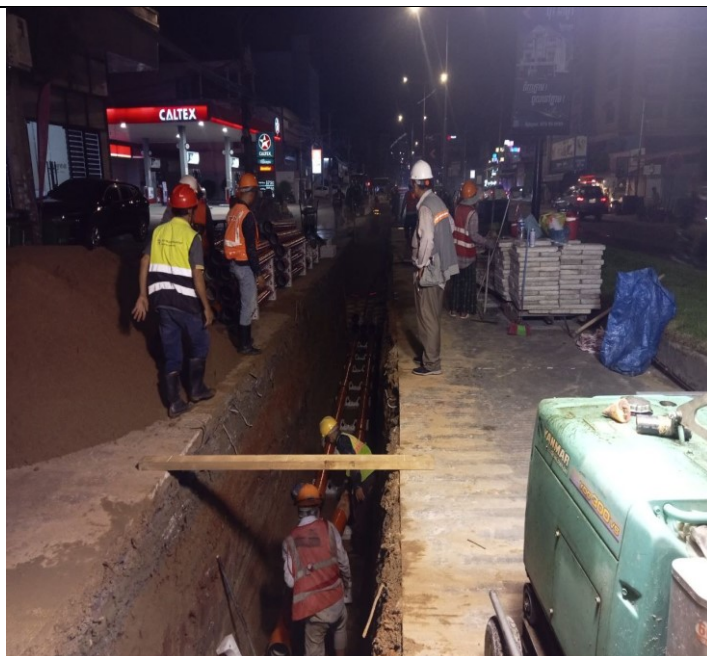
Photo: 14 Assembly PFP pipes and OFC pipe
