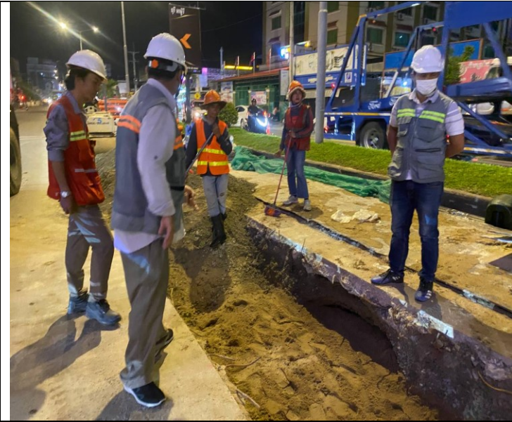
Base course backfilling and compaction
