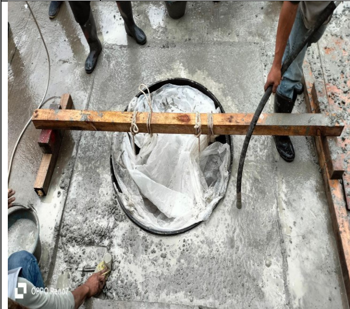
Photo: 09 Manhole Cover Installation activity
