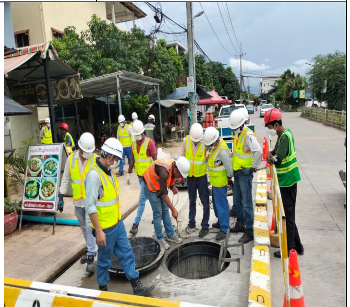
Photo: 18 Manhole Cover Installation activity
