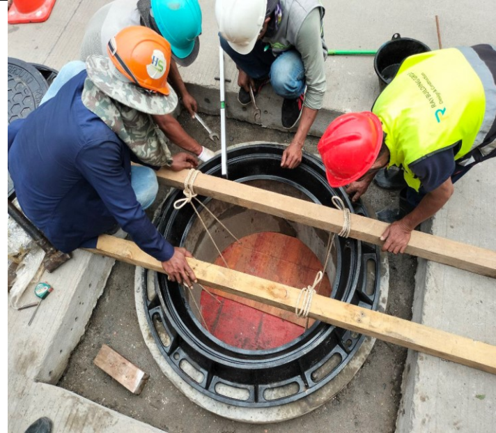
Photo: 03 Manhole Cover Instalation activity
