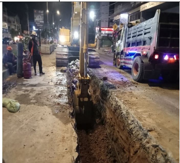
Photo: 12 Soil excavation and concrete road
