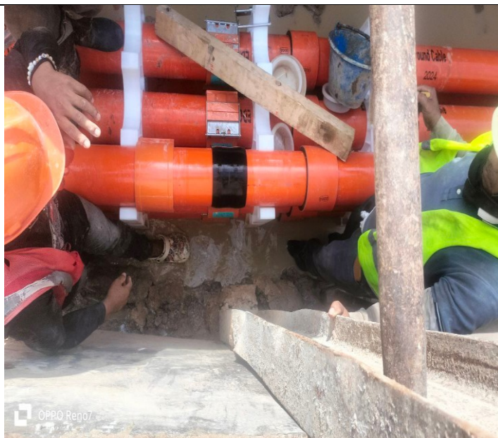
Photo: 20 Assembly PFP pipes and OFC pipe
