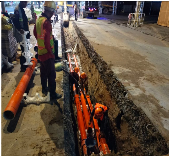
Photo: 16 Assembly PFP pipes and OFC pipe
