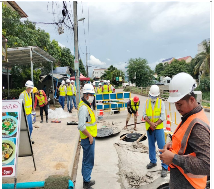
Photo: 16 Manhole Cover Installation activity
