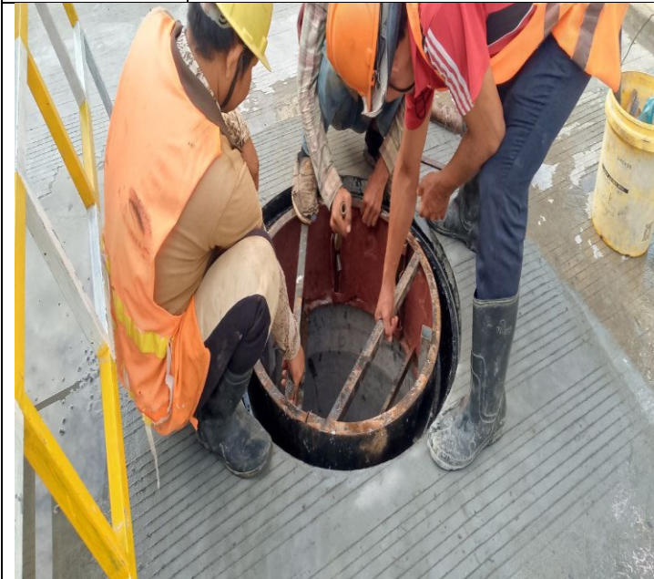
Photo: 11 Manhole Cover Installation activity
