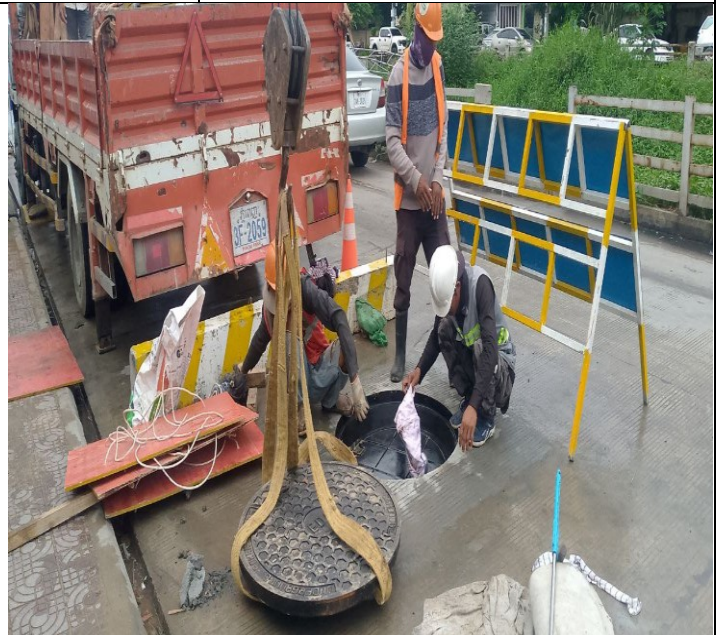
Photo: 12 Manhole Cover Installation activity
