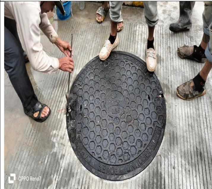
Photo: 15 Manhole Cover Installation activity
