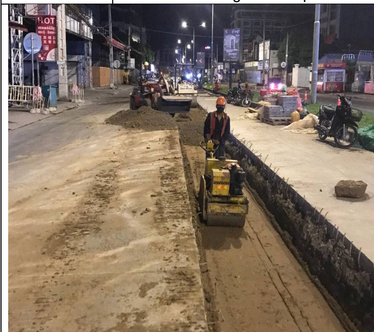
Photo: 11 Sand backfilling and compaction
