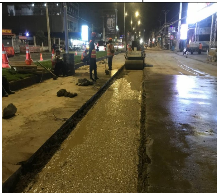
Base course backfilling and compaction
