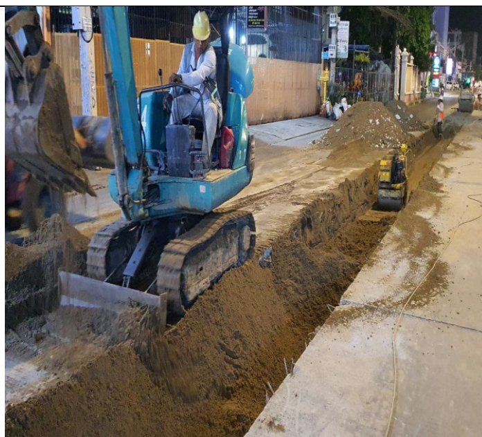
Photo: 08 Sand backfilling and compaction
