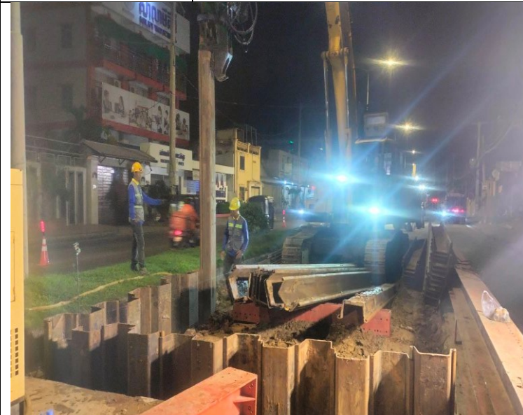
Sheet Pile Installation activity
