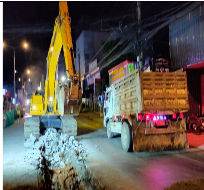
Photo: 08 Soil excavation and concrete road
