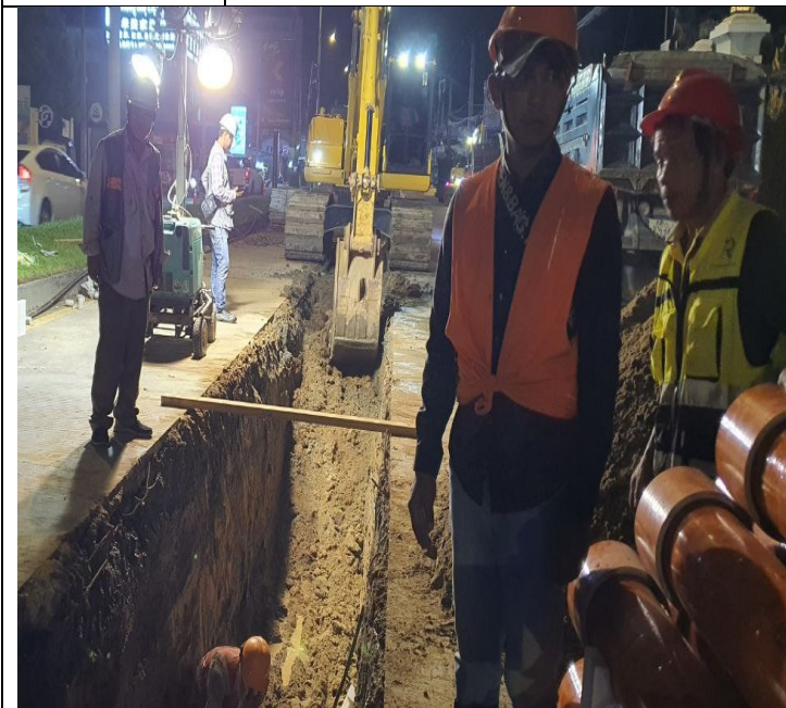
Photo: 17 Soil excavation and concrete road
