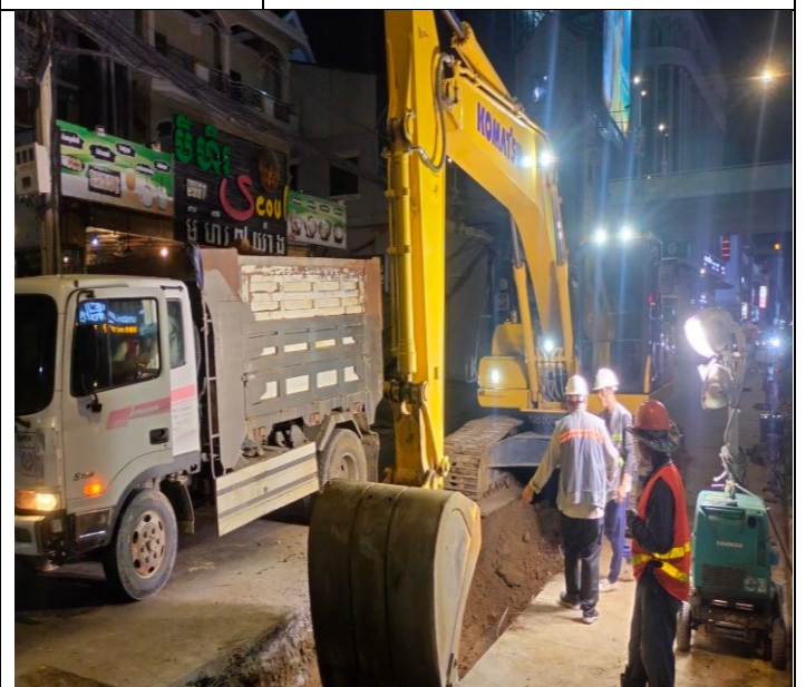
Soil excavation and concrete road
