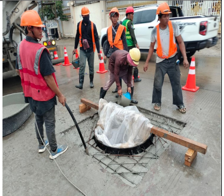
Photo: 10 Manhole Cover Installation activity
