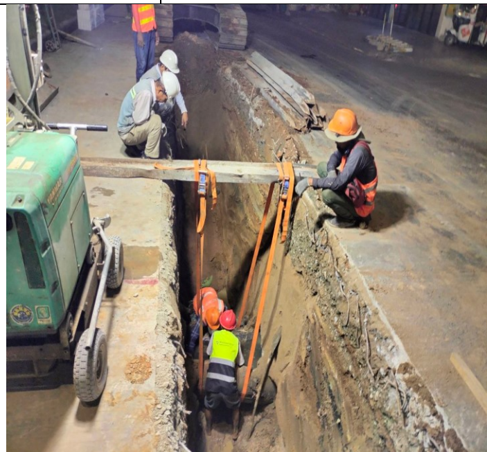
Photo: 18 Soil excavation and concrete road
