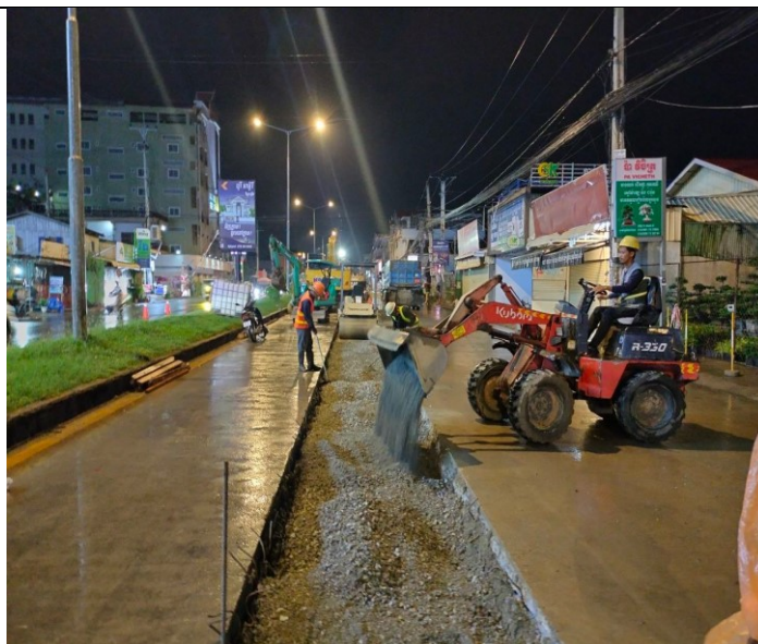
Base course backfilling and compaction
