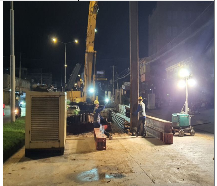
Sheet Pile Installation activity
