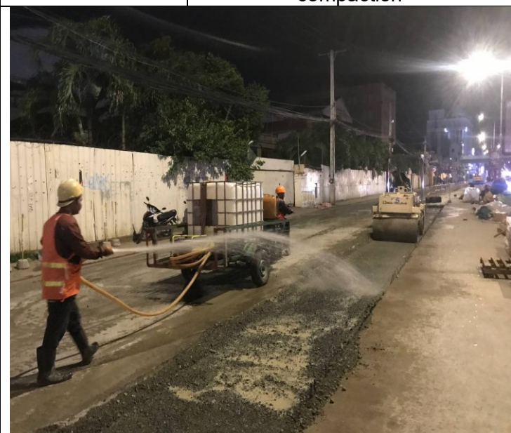
Base course backfilling and compaction
