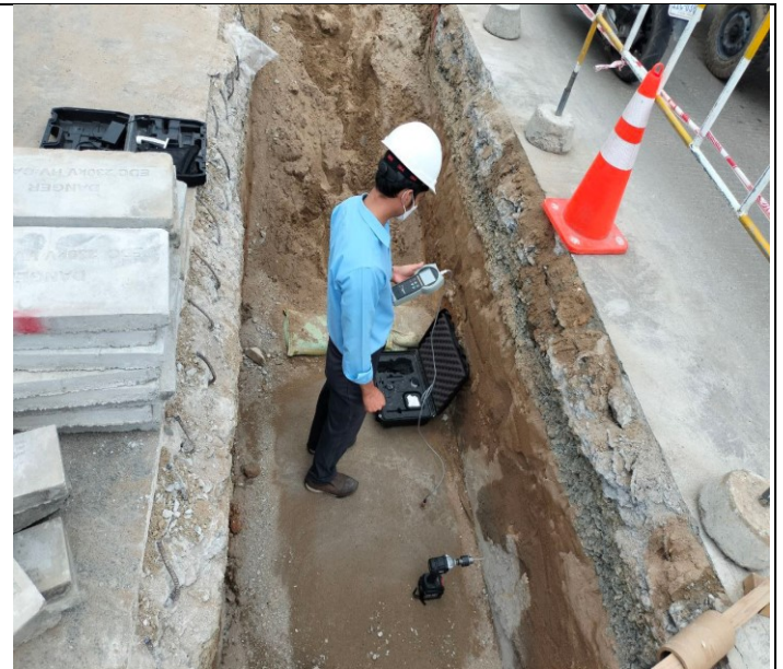
Photo: 02 Thermal test of Sand backfilling
