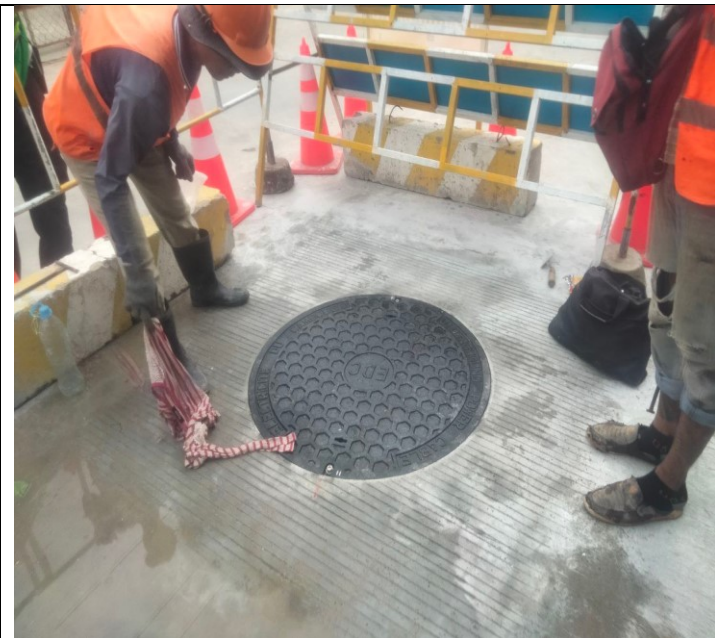
Photo: 13 Manhole Cover Installation activity
