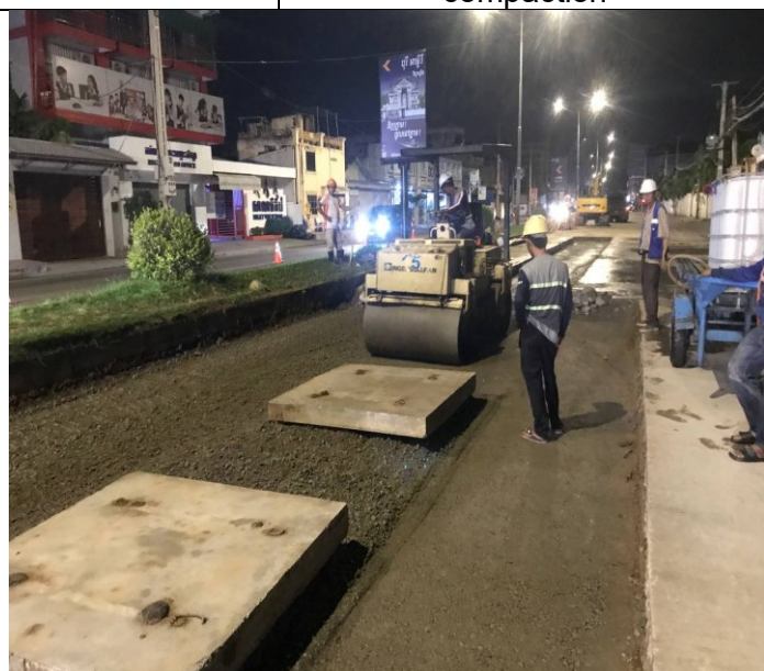
Base course backfilling and compaction
