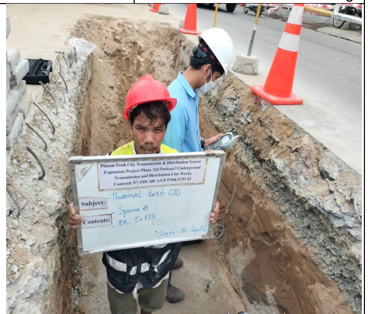
Photo: 04 Thermal test of Sand backfilling
