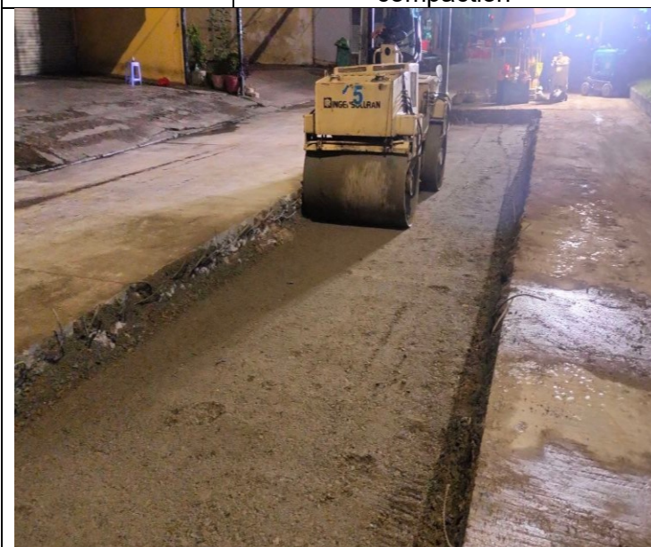
Base course backfilling and compaction
