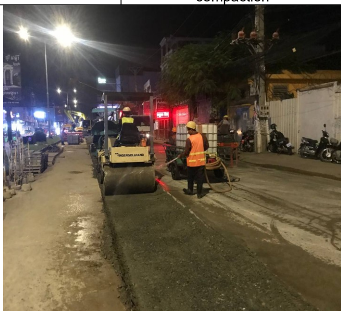
Base course backfilling and compaction
