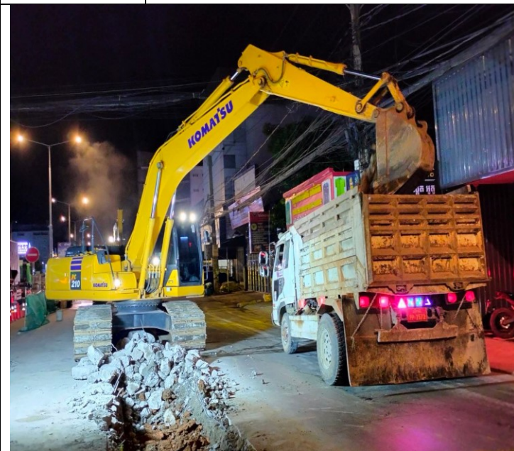
Photo: 09 Soil excavation and concrete road
