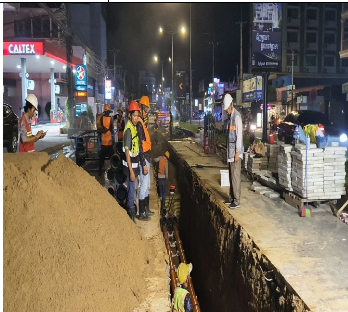
Photo: 18 Assembly PFP pipes and OFC pipe
