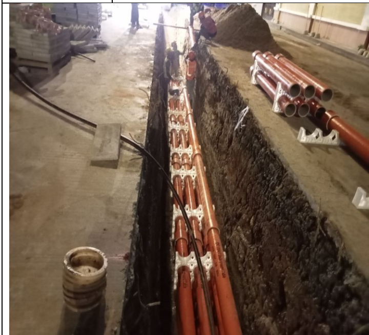
Photo: 15 Assembly PFP pipes and OFC pipe
