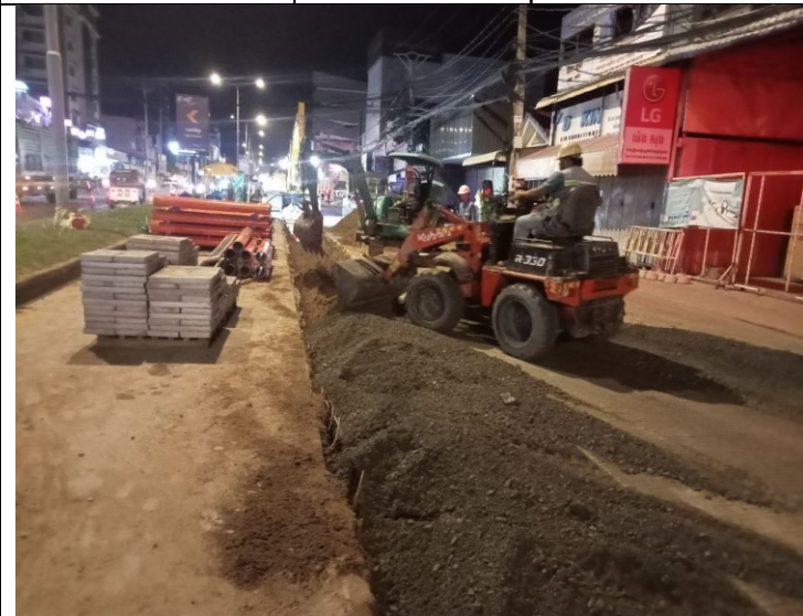
Base course backfilling and compaction
