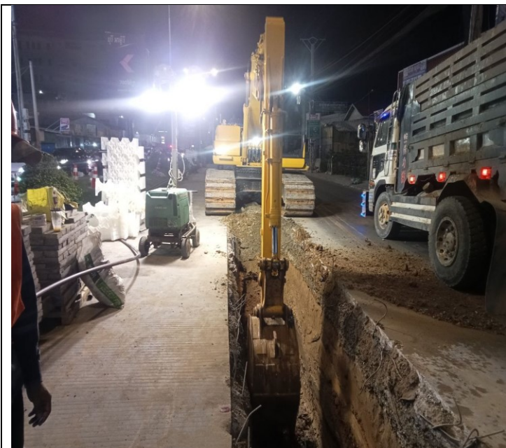
Photo: 13 Soil excavation and concrete road
