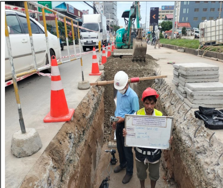
Photo: 01 Thermal test of Sand backfilling
