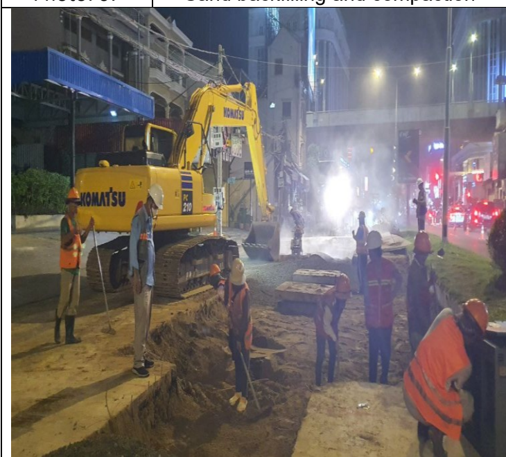
Photo: 09 Sand backfilling and compaction
