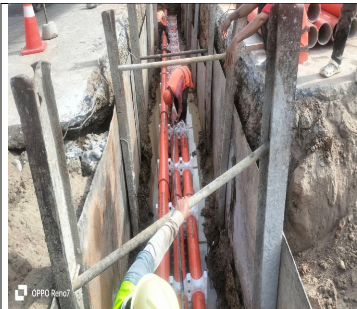
Photo: 19 Assembly PFP pipes and OFC pipe
