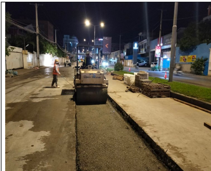
Base course backfilling and compaction
