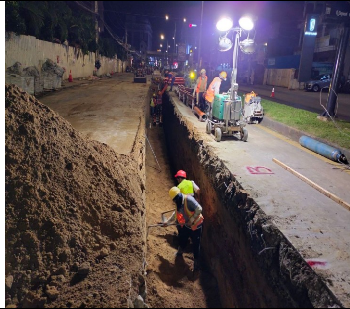
Photo: 01 Assembly PFP pipes and OFC pipe
