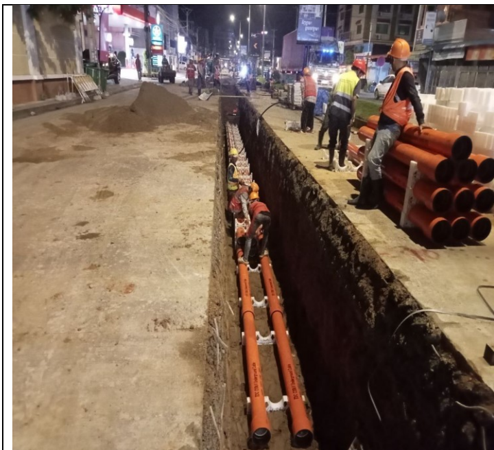
Photo: 13 Assembly PFP pipes and OFC pipe
