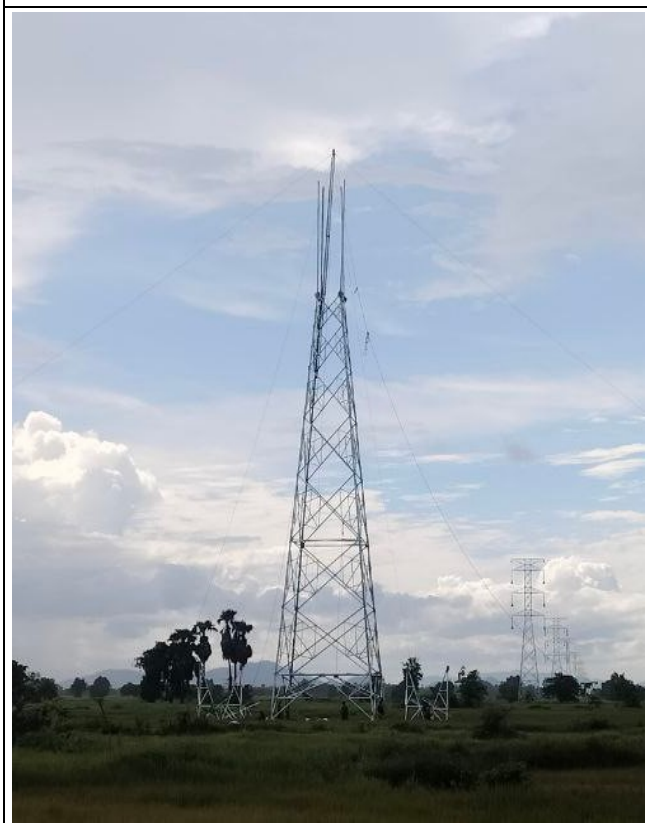
T-A086 Tower erection.
