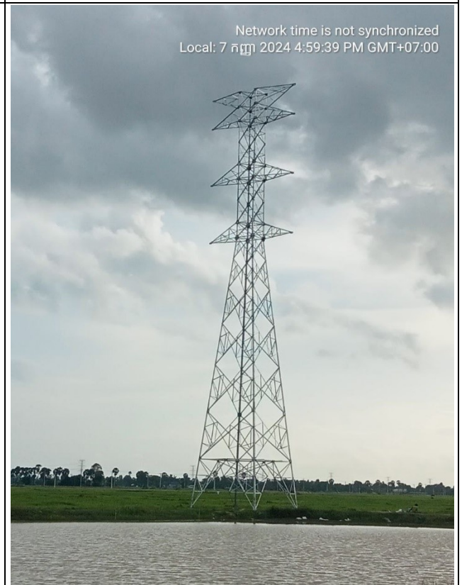
T-A007 Erection completd.
