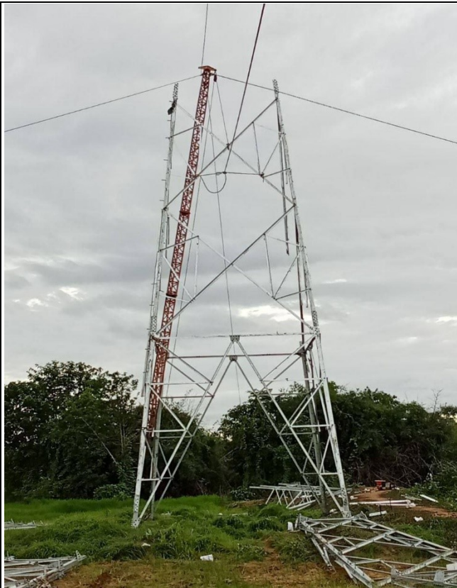
T-A105 Tower erection.
