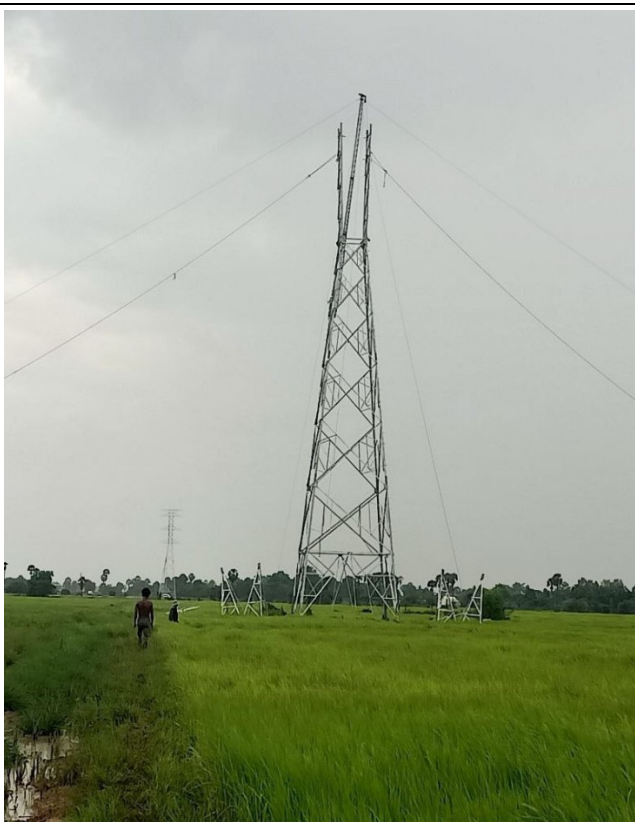
T-A009 Tower erection .
