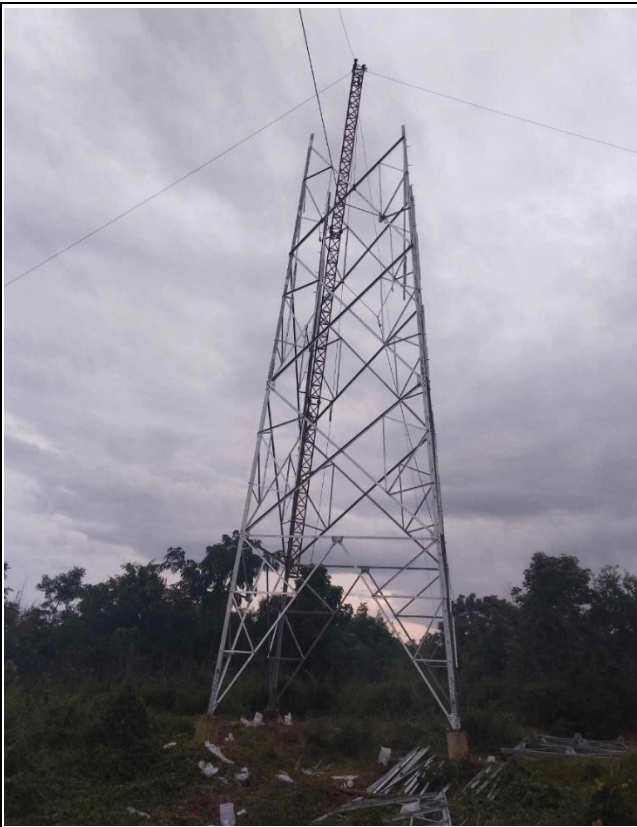
T-A174 Tower erection .
