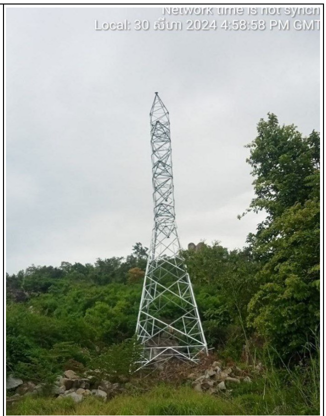
T-A159 Erection completed.
