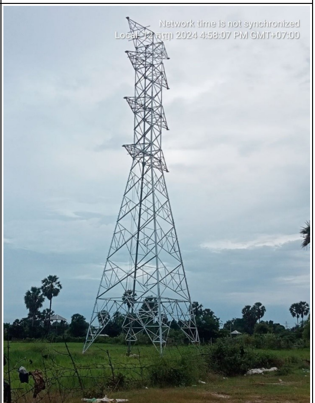
T-A005 Erection completd.
