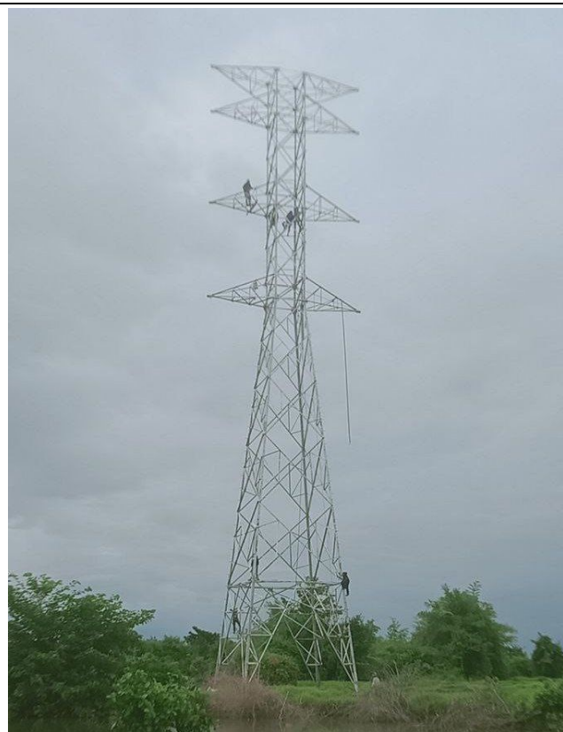
T-A103 Erection completd.
