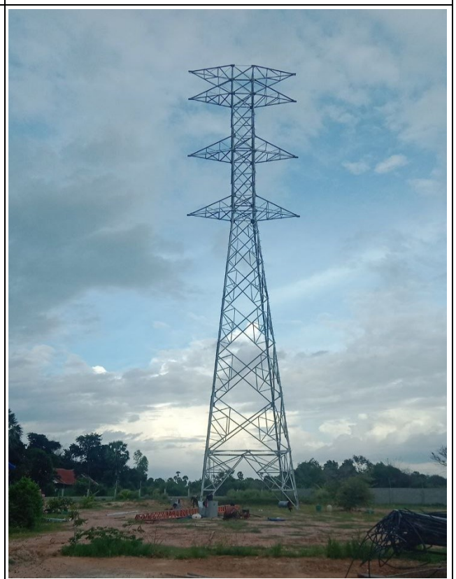
T-A014 Erection completd.
