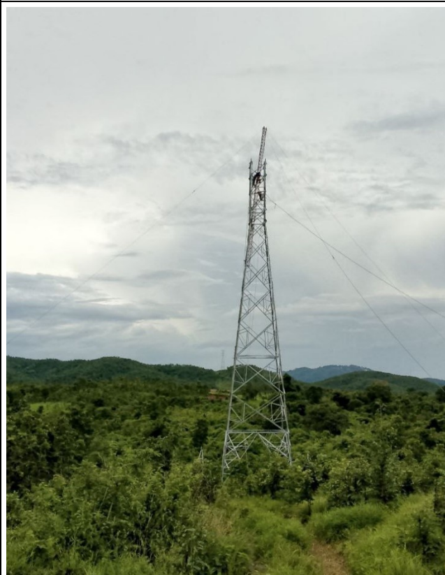
T-A185 Tower erection .
