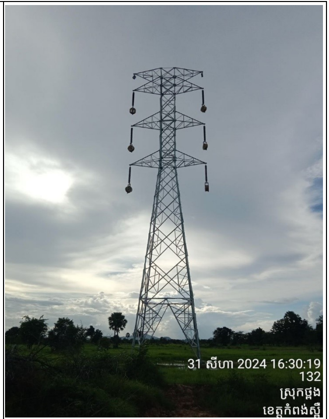
Hang insulator disk and roller.
