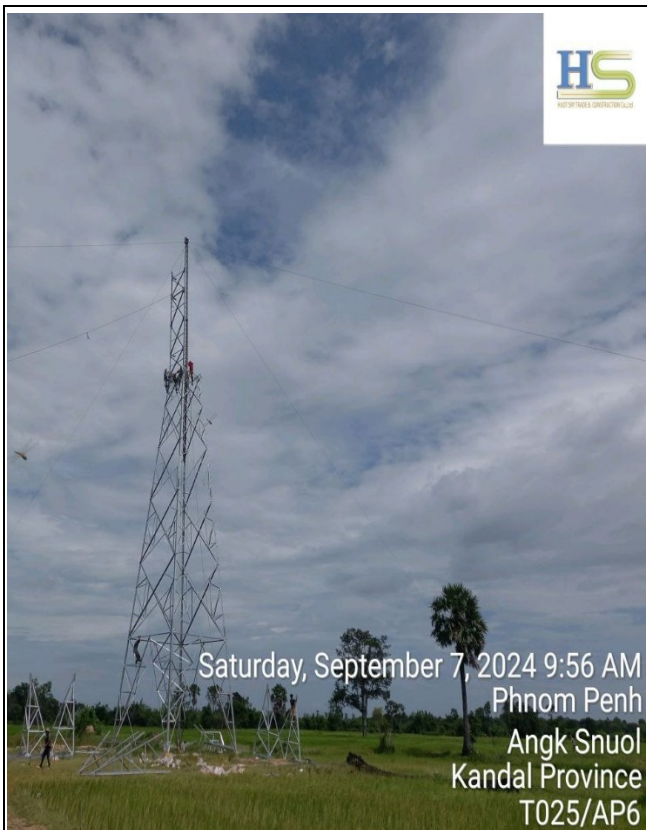
T-A013 Tower erection .
