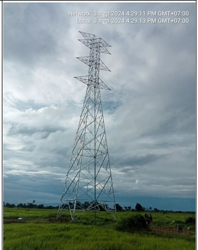
T-A081 Erection completed.
