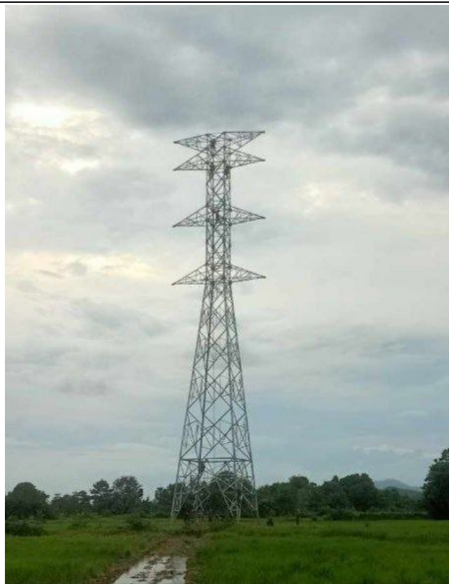
T-A119 Erection completed.
