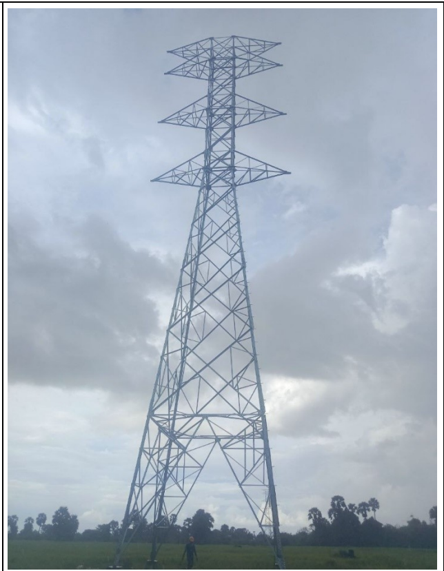
T-A015 Erection completed.
