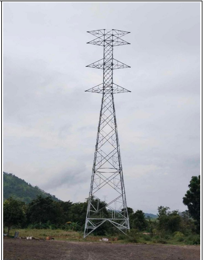
T-A153 Erection completed.
