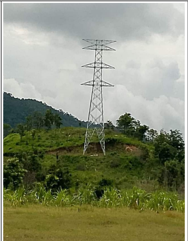
T-A150 Erection completed.
