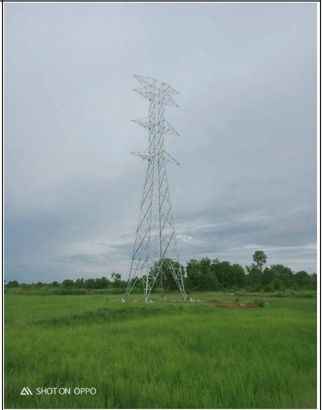
T-A120 Erection completd.
