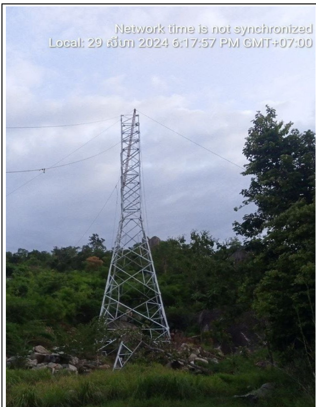
T-A159 Tower erection.
