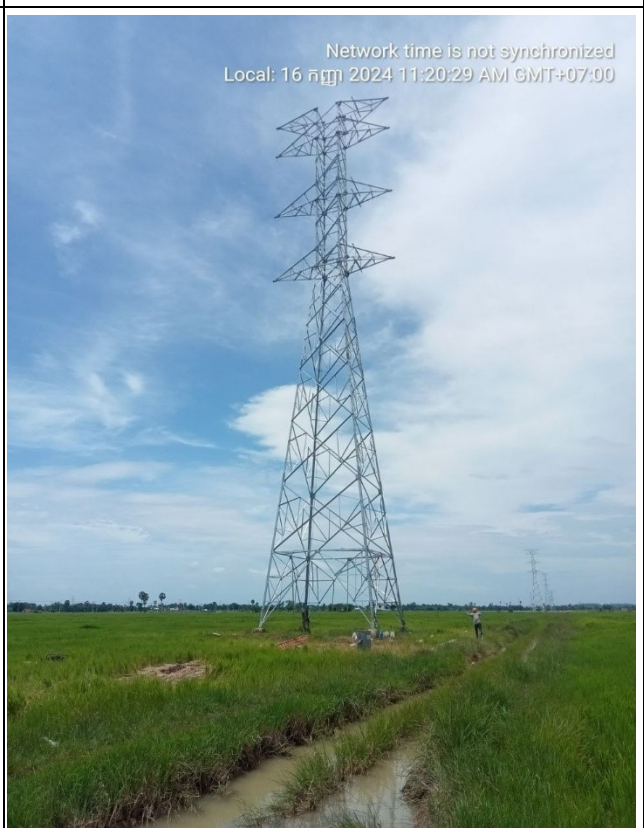
T-A008 Erection completd.
