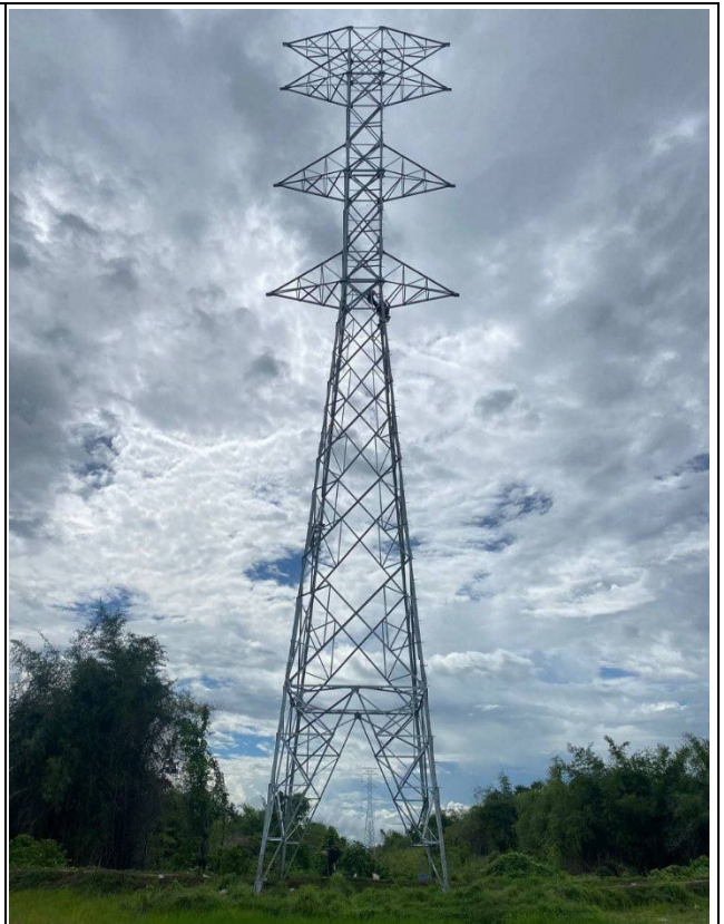
T-A105 Erection completed.
