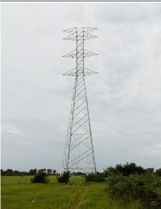
T-A017 Erection completd.
