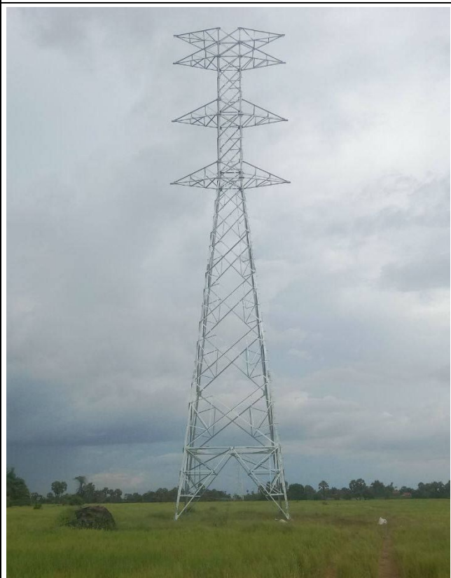
T-A016 Erection completed .
