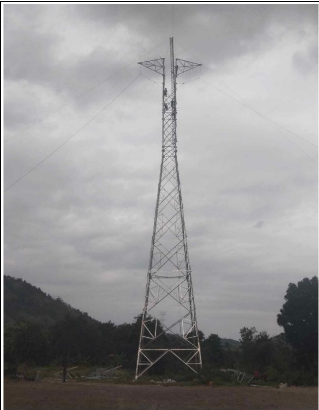
T-A153 Erection completed.
