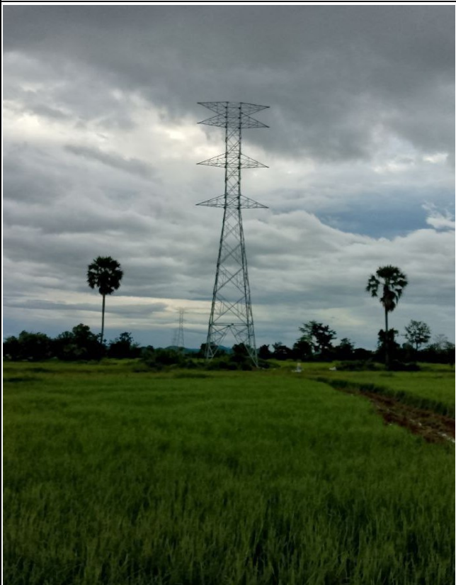
T-A114 Erection completd.
