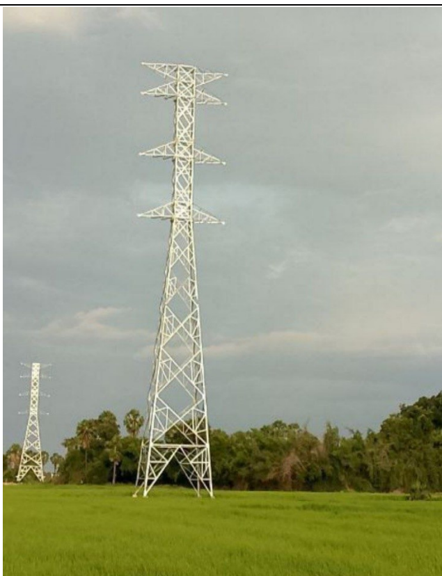
T-A006 Erection completed .
