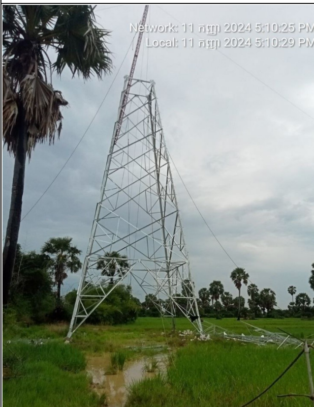
T-A005 Tower erection .
