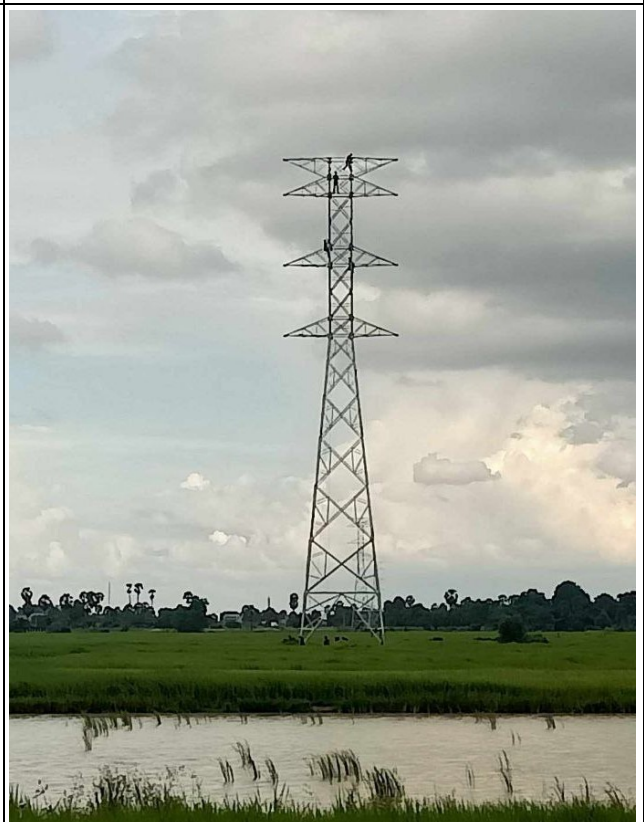
T-A009 Erection completd.
