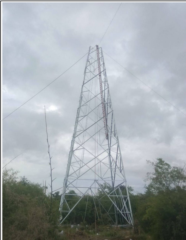
T-A018 Tower erection .
