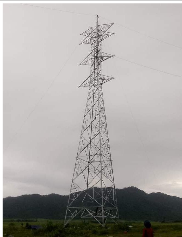
T-A148 Tower erection .
