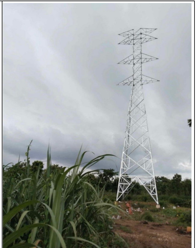
T-A174 Erection completed.
