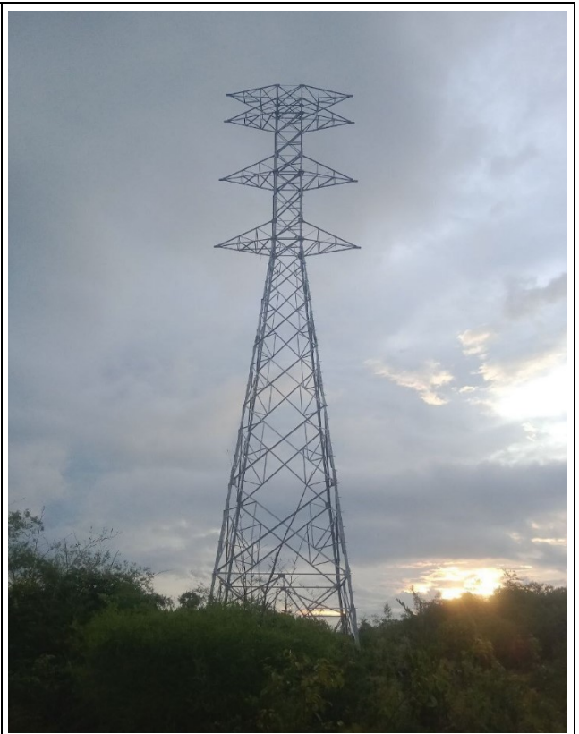
T-A018 Erection completed.
