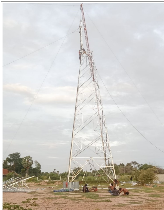
T-A014 Tower erection .
