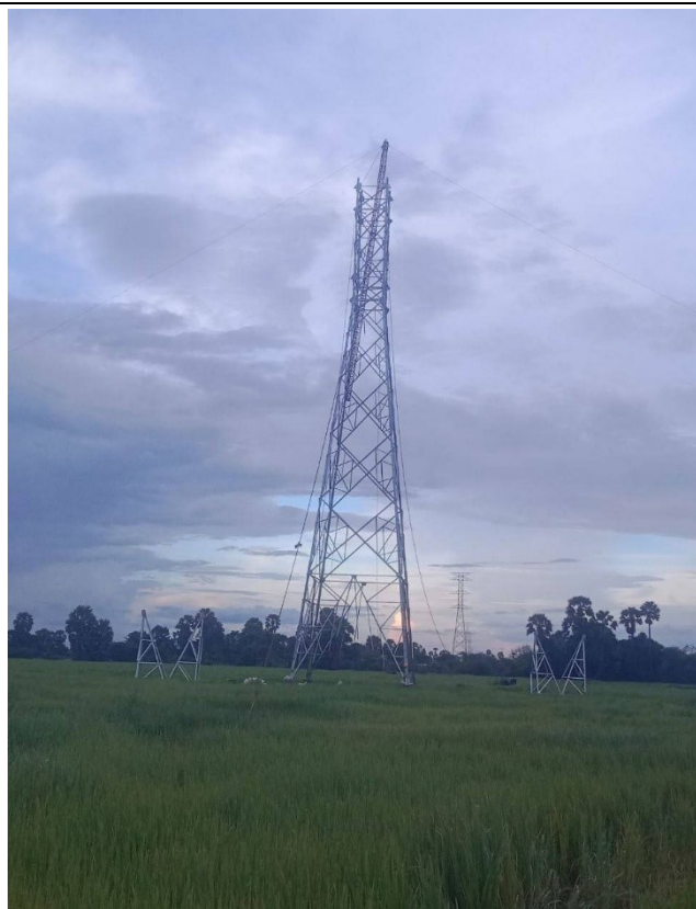
T-A015 Tower erection .
