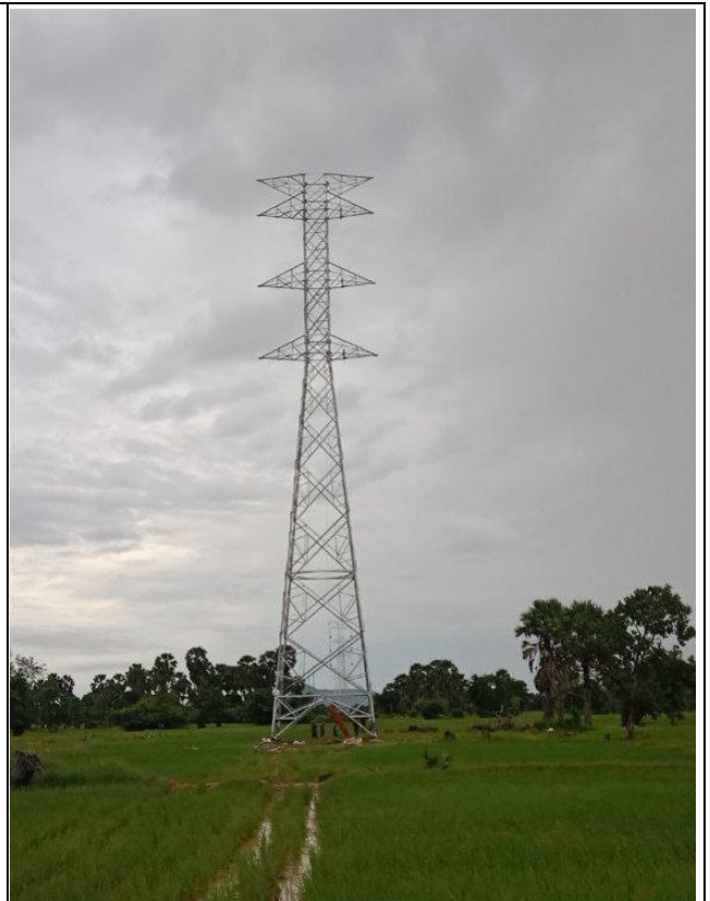
T-A071 Erection completed.
