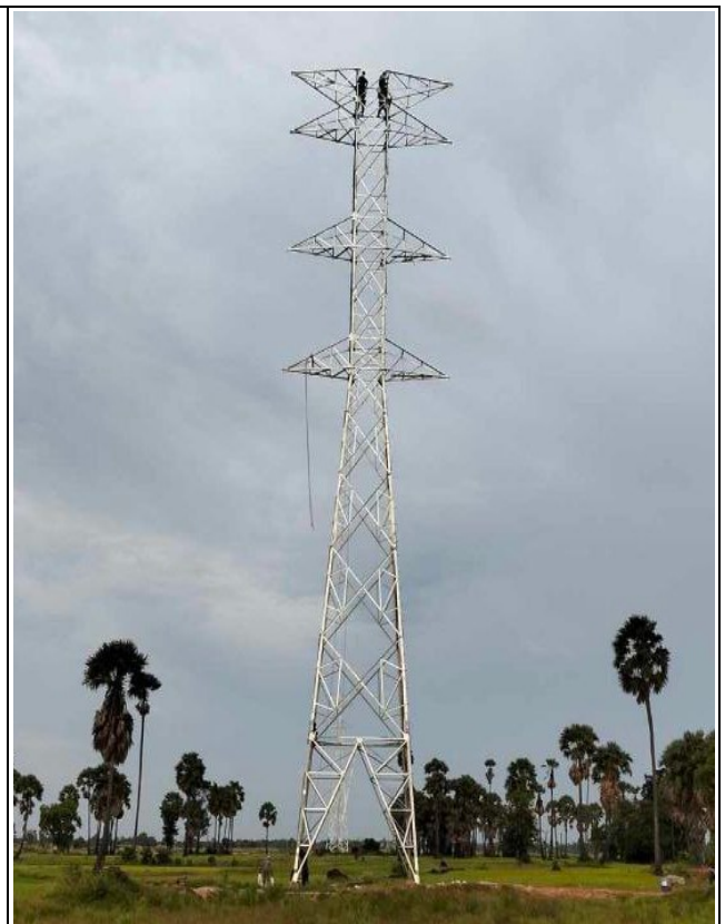
T-A013 Erection completed.
