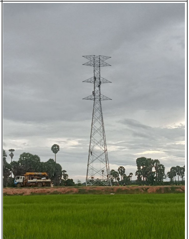
T-A012 Erection completd.
