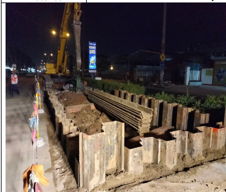
Photo: 05 Sheet Pile Installation activity
