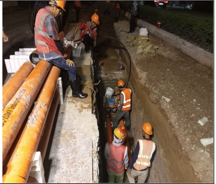
Photo: 02 Assembly PFP pipes and OFC pipe
