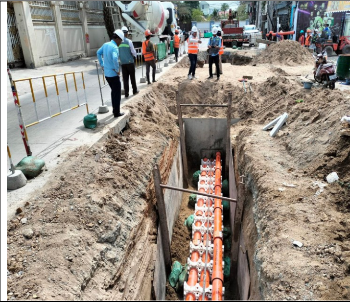
Photo: 01 Assembly PFP pipes and OFC pipe
