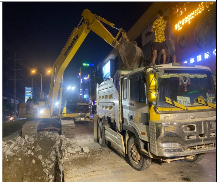
Photo: 04 Soil excavation and concrete road
