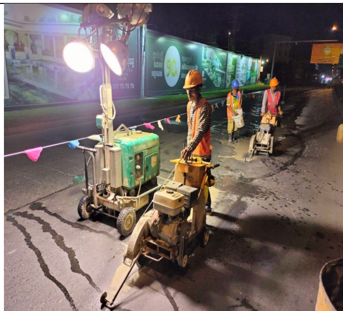
Photo: 04 Saw cutting of concrete road
