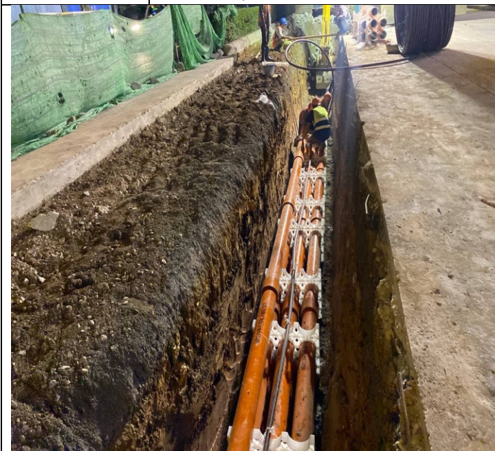
Photo: 11 Assembly PFP pipes and OFC pipe
