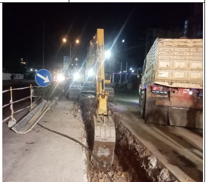
Photo: 06 Soil excavation and concrete road
