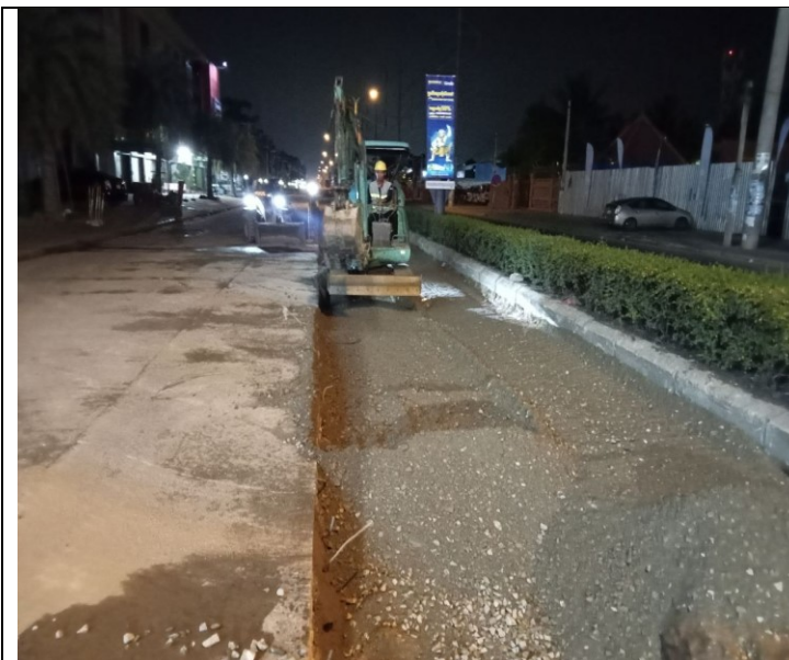
Base course backfilling and compaction
