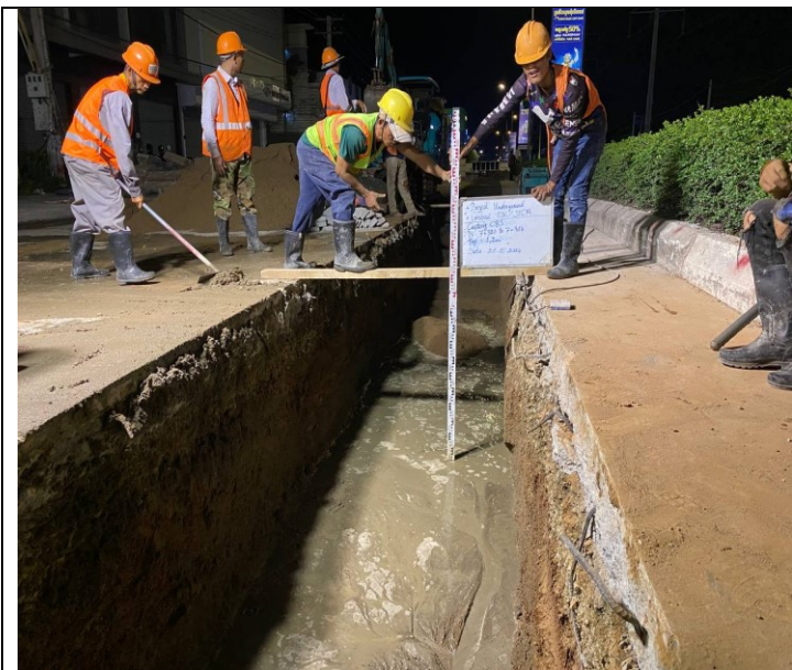
Photo: 19 Assembly PFP pipes and OFC pipe
