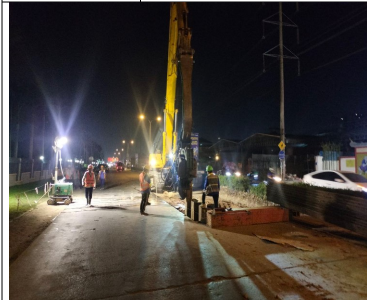
Photo: 03 Sheet Pile Installation activity
