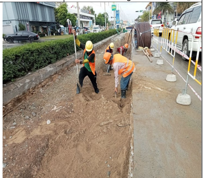
Photo: 06 Sand backfilling and compaction
