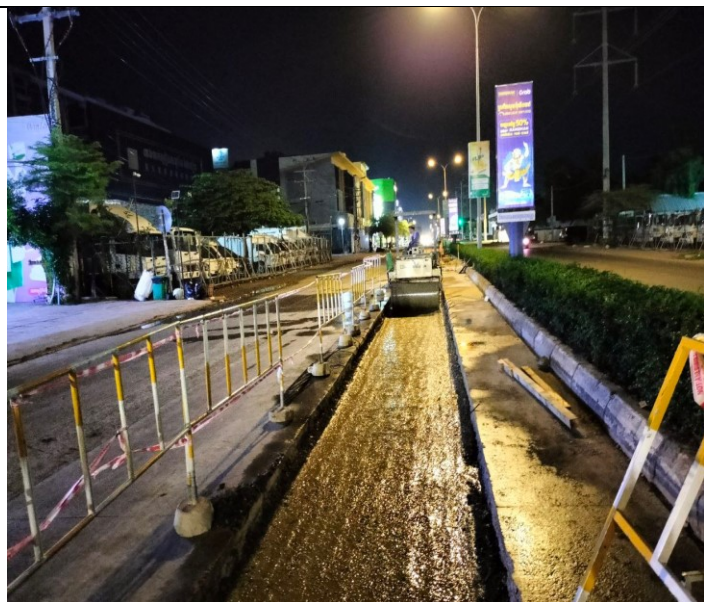
Base course backfilling and compaction
