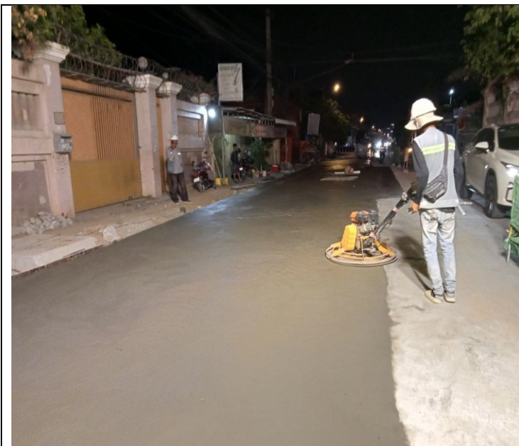
Photo: 07 Manhole of concrete road activity
