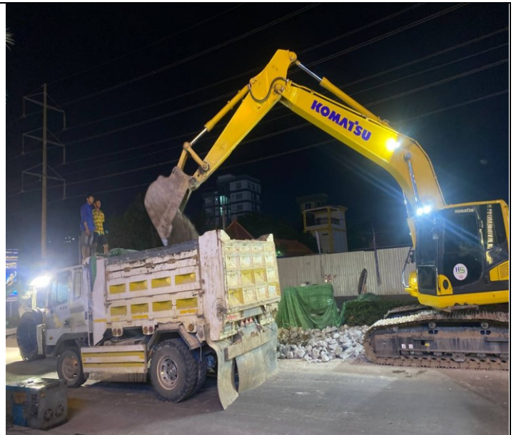
Photo: 02 Soil excavation and concrete road
