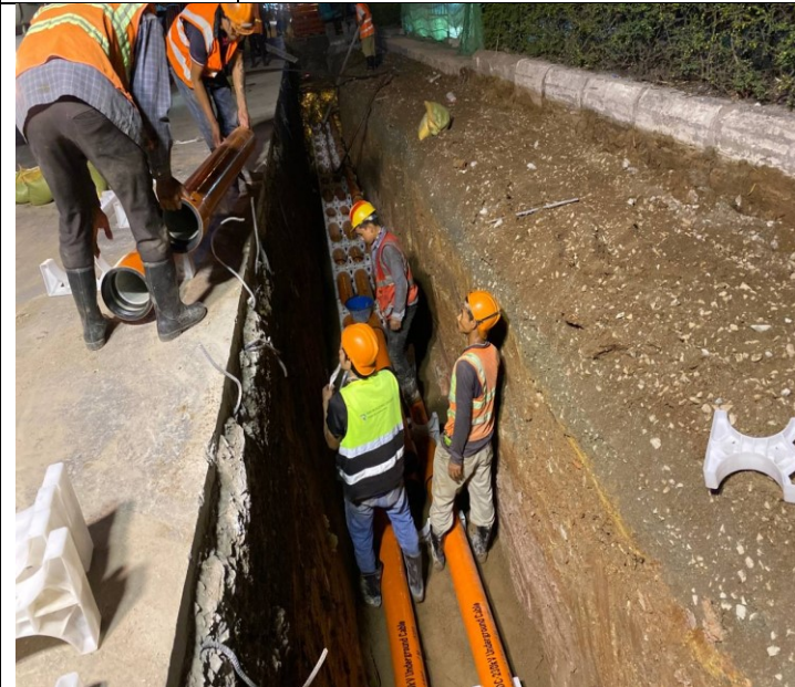
Photo: 15 Assembly PFP pipes and OFC pipe
