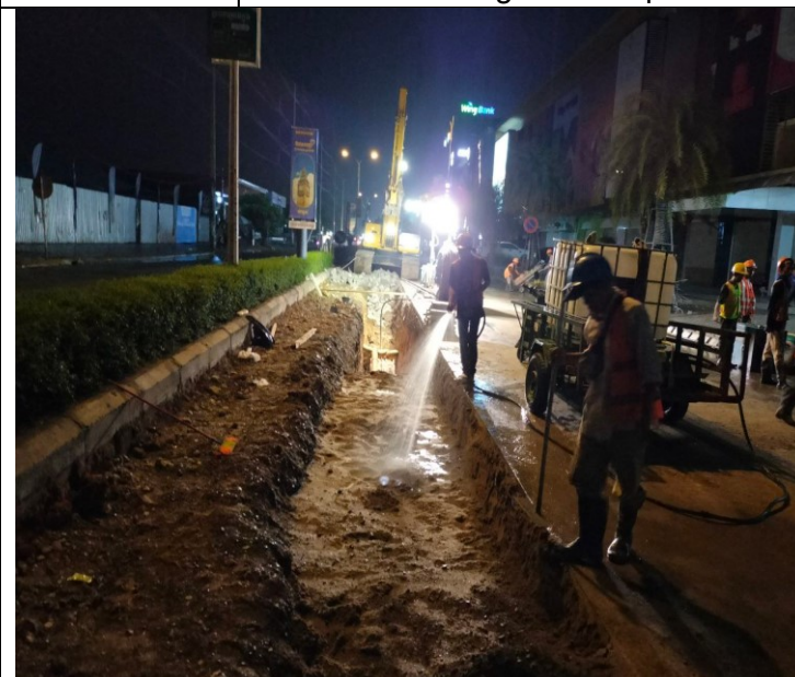
Photo: 05 Sand backfilling and compaction
