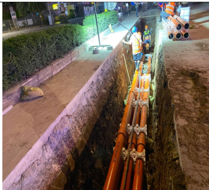
Photo: 26 Assembly PFP pipes and OFC pipe
