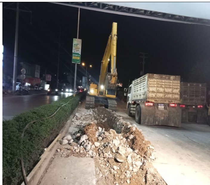
Photo: 08 Soil excavation and concrete road
