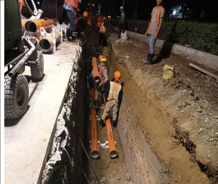
Photo: 03 Assembly PFP pipes and OFC pipe
