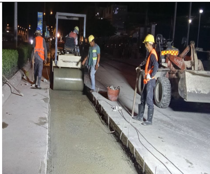
Base course backfilling and compaction
