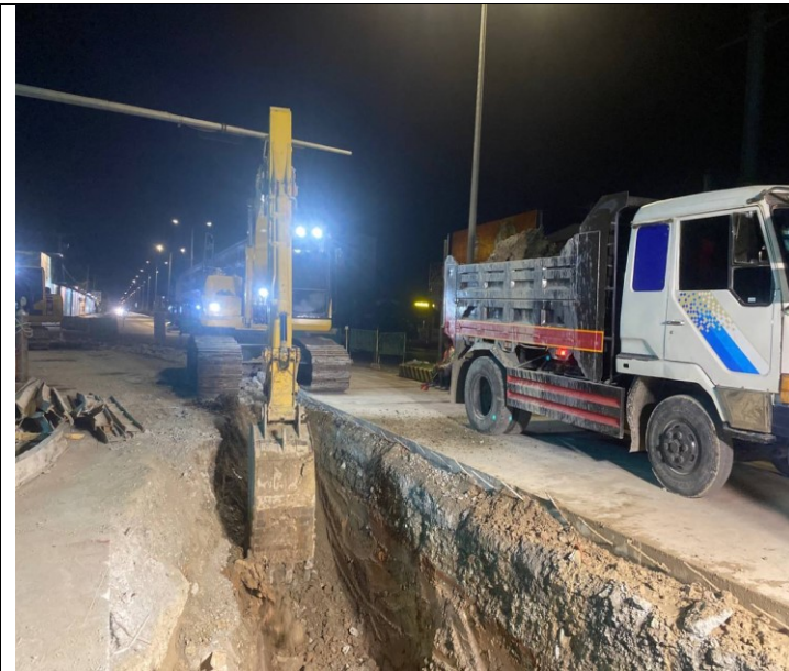
Photo: 01 Soil excavation and concrete road
