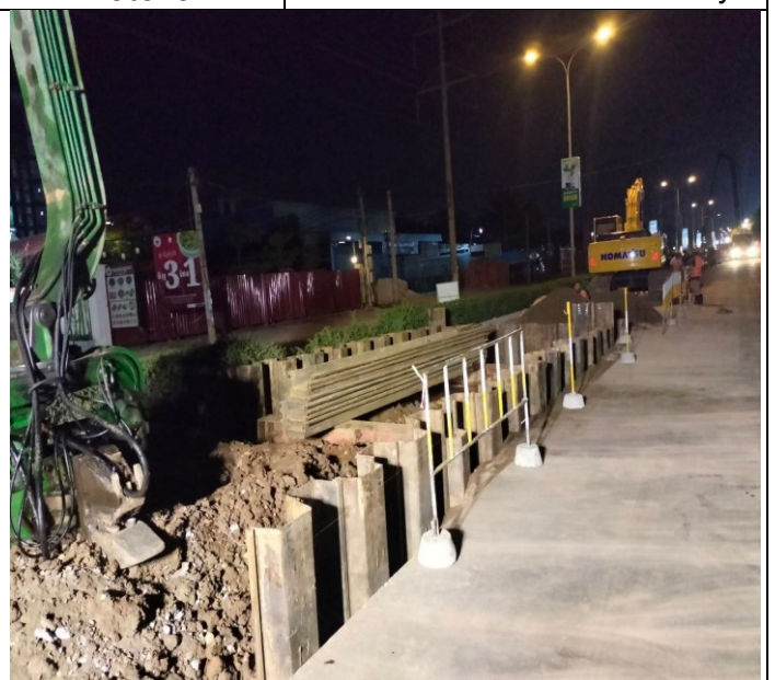
Photo: 06 Sheet Pile Installation activity
