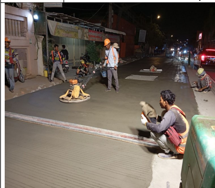
Photo: 09 Manhole of concrete road activity
