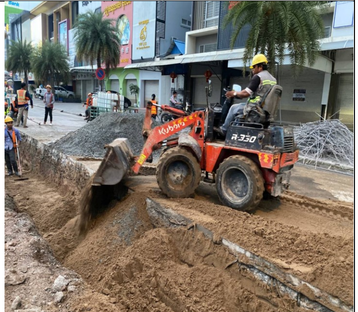
Photo: 04 Sand backfilling and compaction
