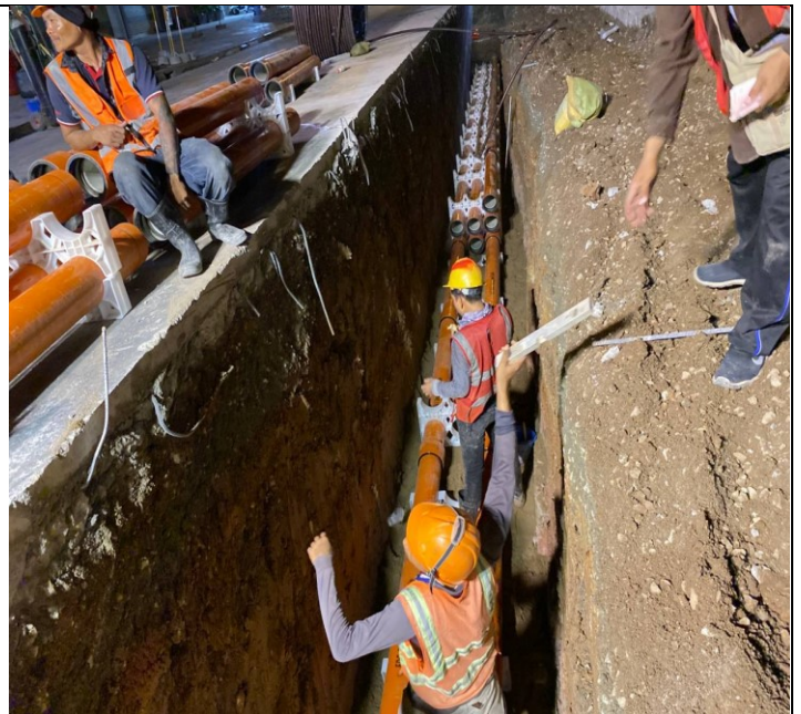
Photo: 14 Assembly PFP pipes and OFC pipe
