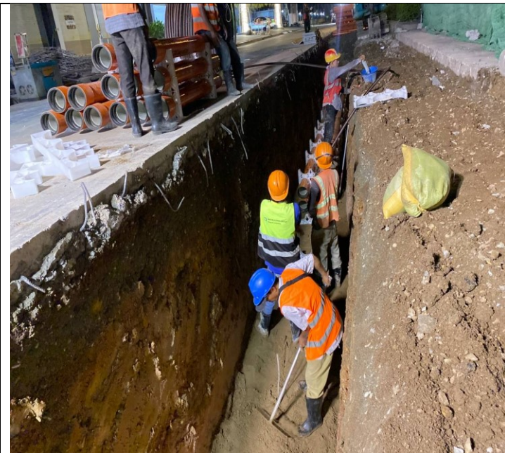
Photo: 13 Assembly PFP pipes and OFC pipe
