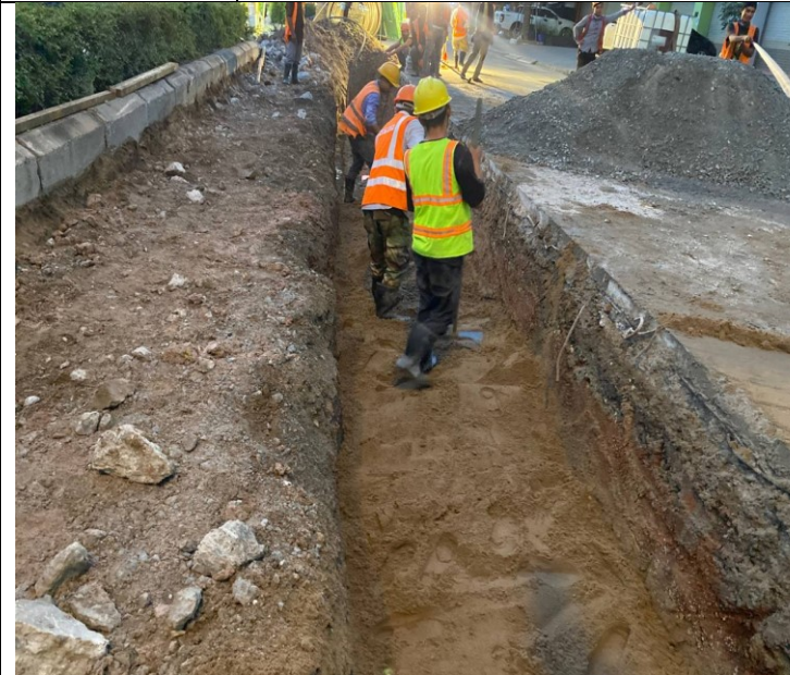
Photo: 03 Sand backfilling and compaction
