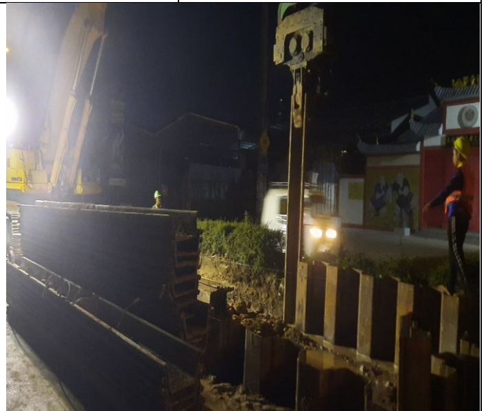
Photo: 04 Sheet Pile Installation activity
