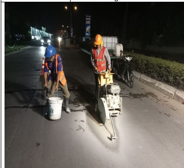
Photo: 07 Saw cutting of concrete road
