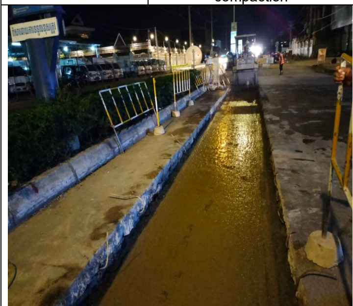
Base course backfilling and compaction
