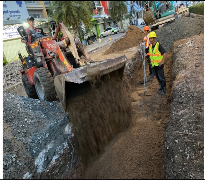
Photo: 02 Sand backfilling and compaction
