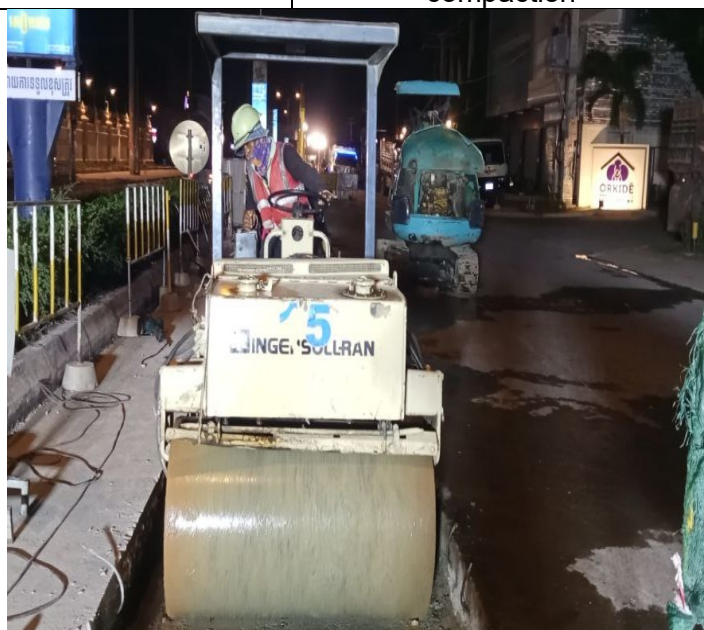
Base course backfilling and compaction
