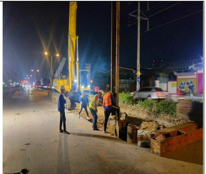
Photo: 02 Sheet Pile Installation activity
