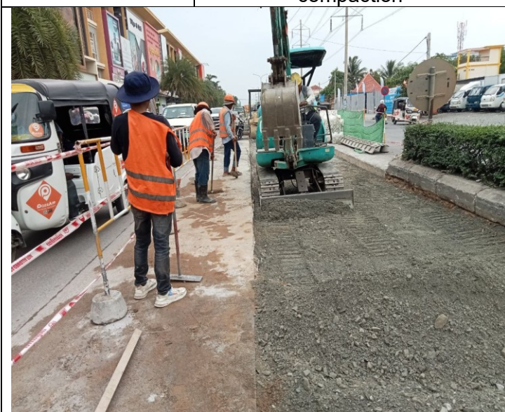
Base course backfilling and compaction
