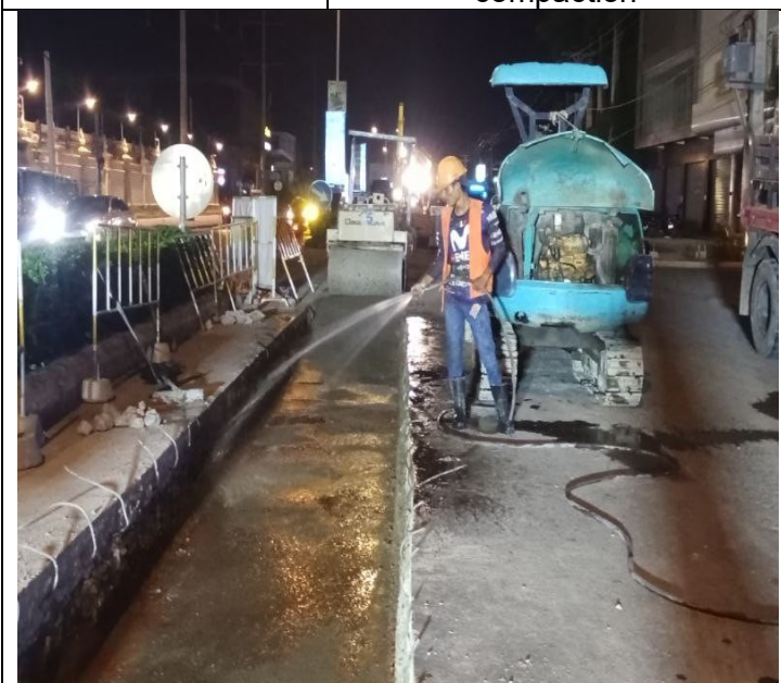
Base course backfilling and compaction
