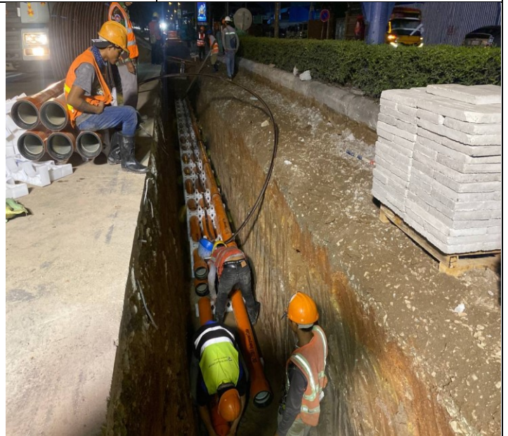
Photo: 16 Assembly PFP pipes and OFC pipe
