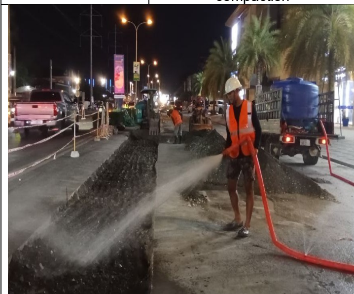
Base course backfilling and compaction
