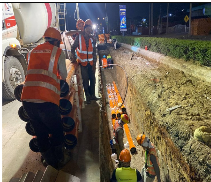
Photo: 08 Assembly PFP pipes and OFC pipe
