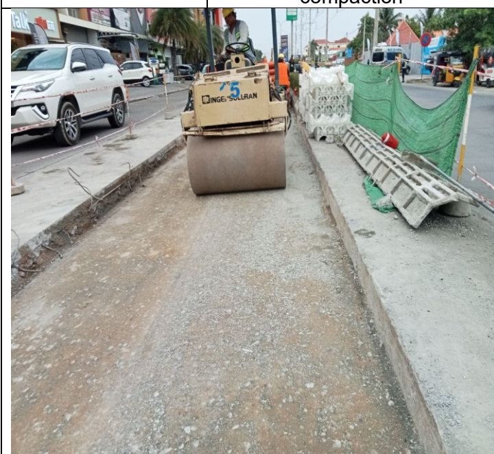
Base course backfilling and compaction
