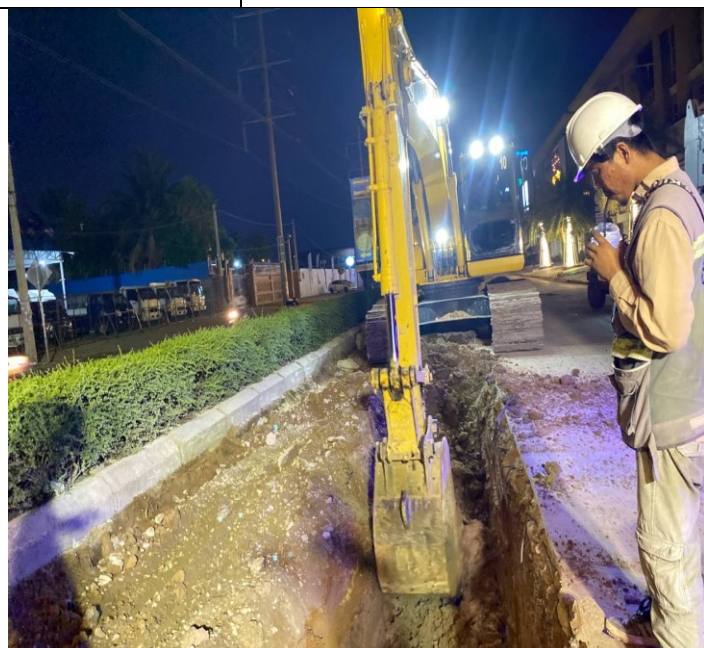
Photo: 10 Soil excavation and concrete road
