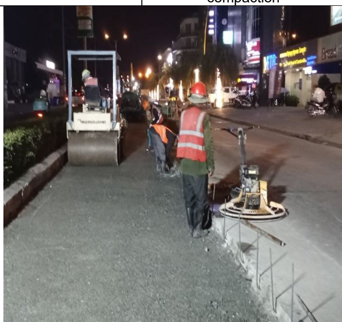
Base course backfilling and compaction
