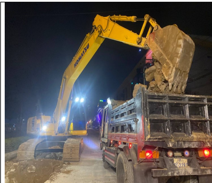
Photo: 07 Soil excavation and concrete road
