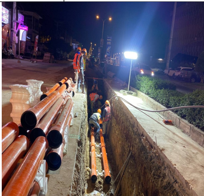
Photo: 24 Assembly PFP pipes and OFC pipe
