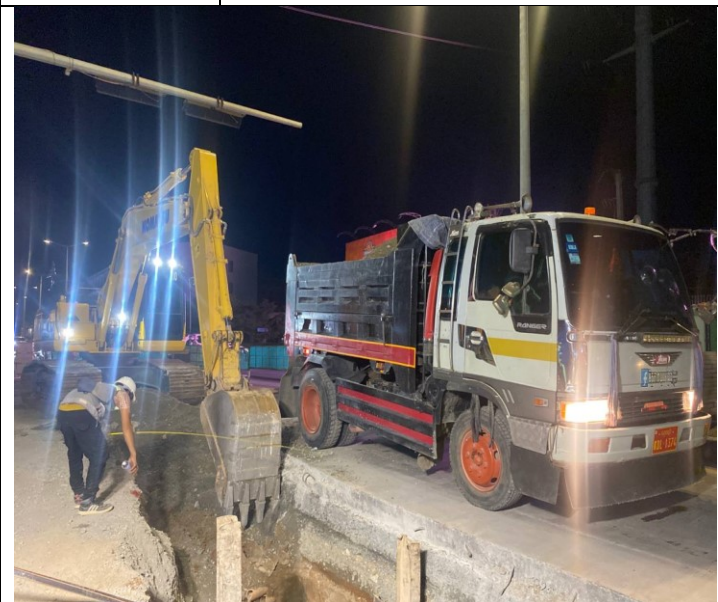
Photo: 03 Soil excavation and concrete road
