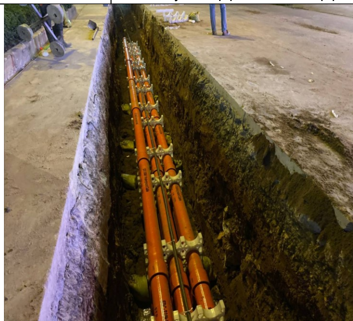
Photo: 28 Assembly PFP pipes and OFC pipe
