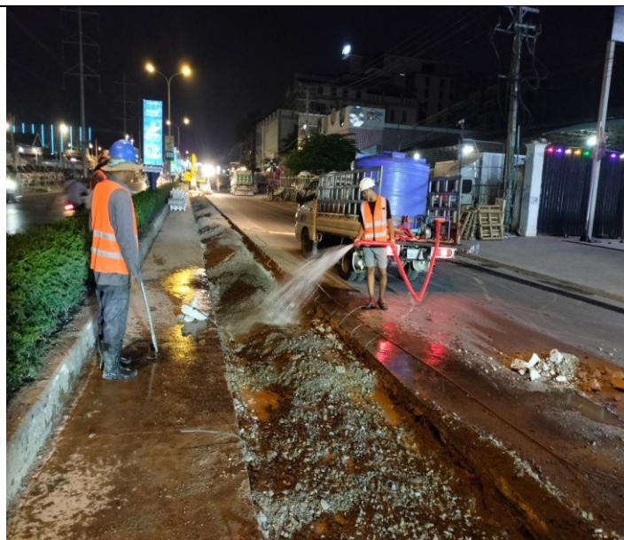
Base course backfilling and compaction
