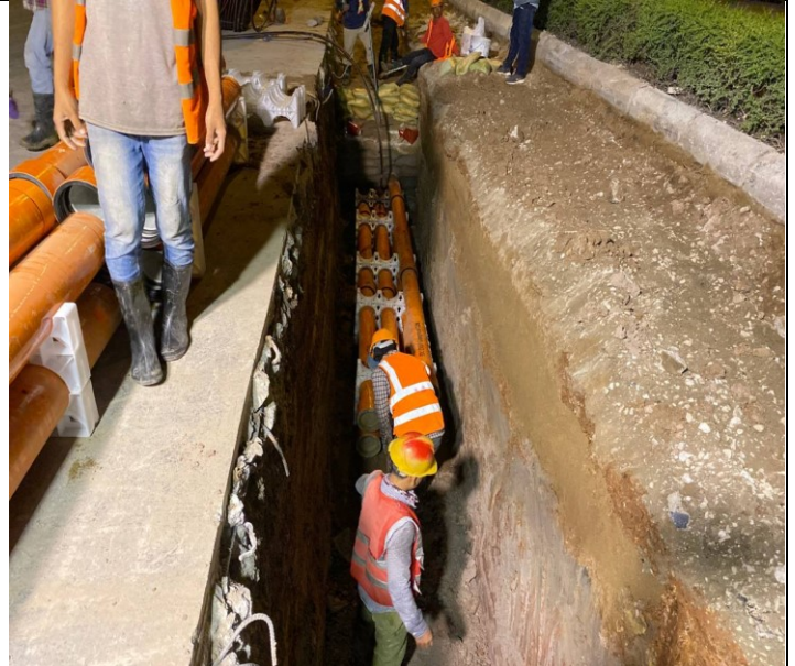
Photo: 04 Assembly PFP pipes and OFC pipe
