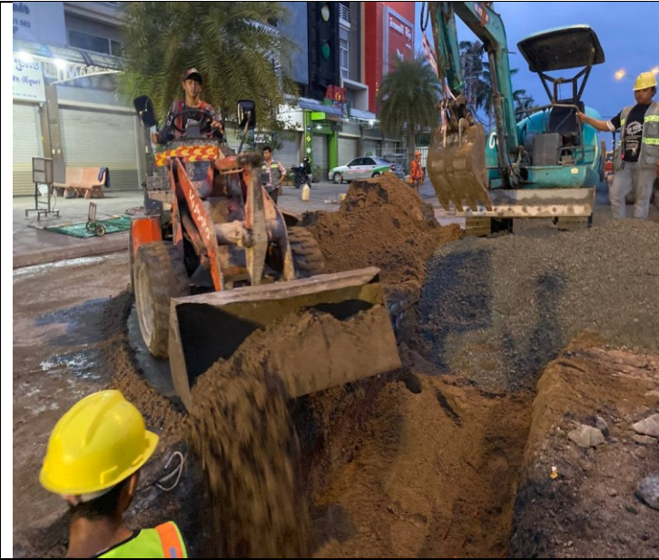
Photo: 01 Sand backfilling and compaction
