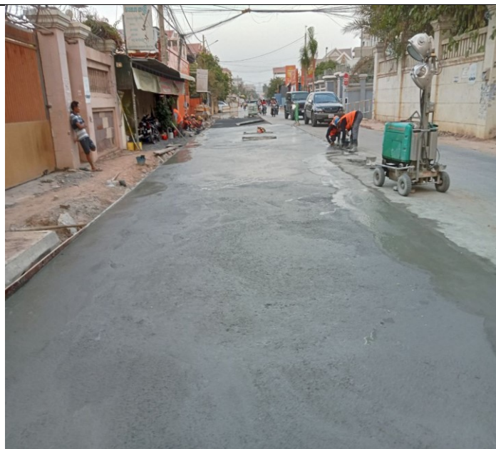
Photo: 08 Manhole of concrete road activity
