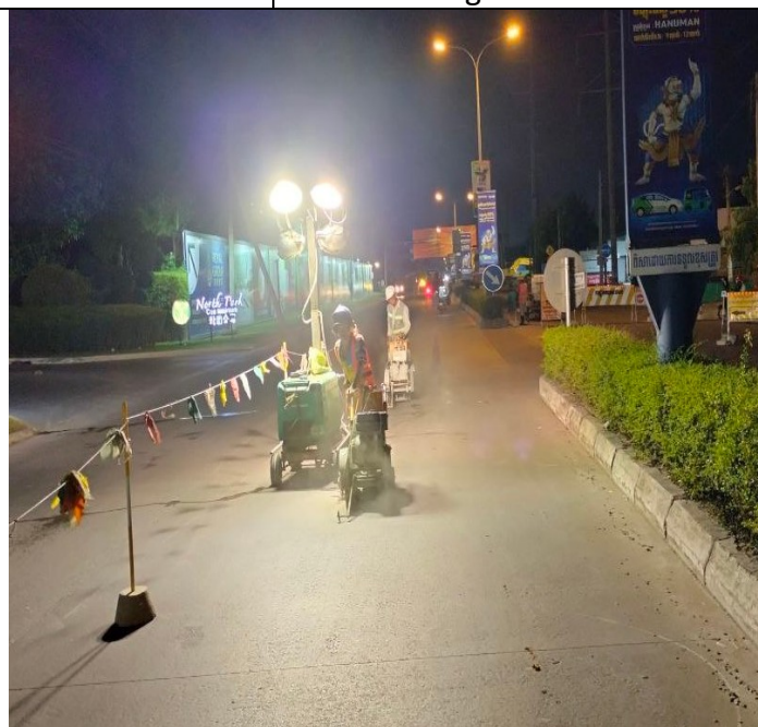
Photo: 08 Saw cutting of concrete road
