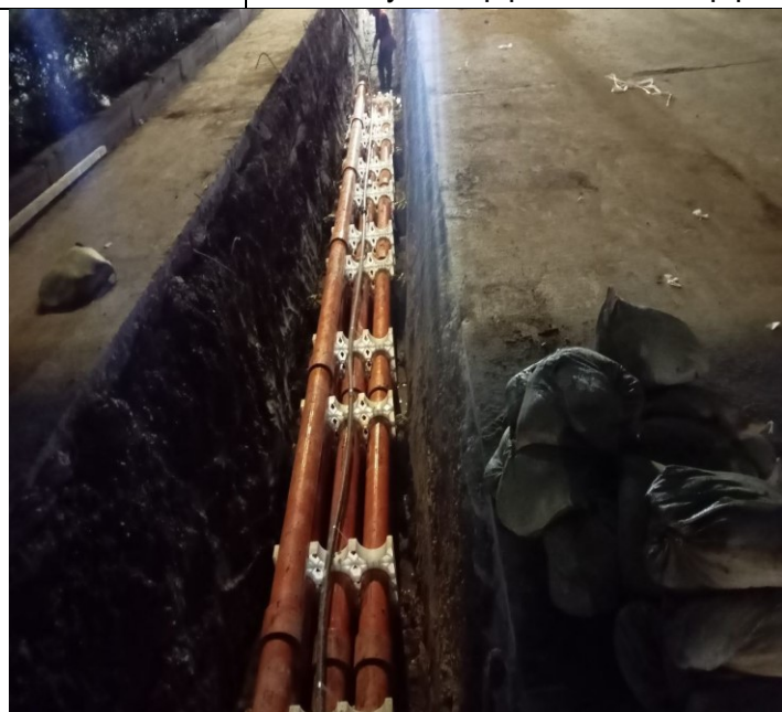
Photo: 30 Assembly PFP pipes and OFC pipe
