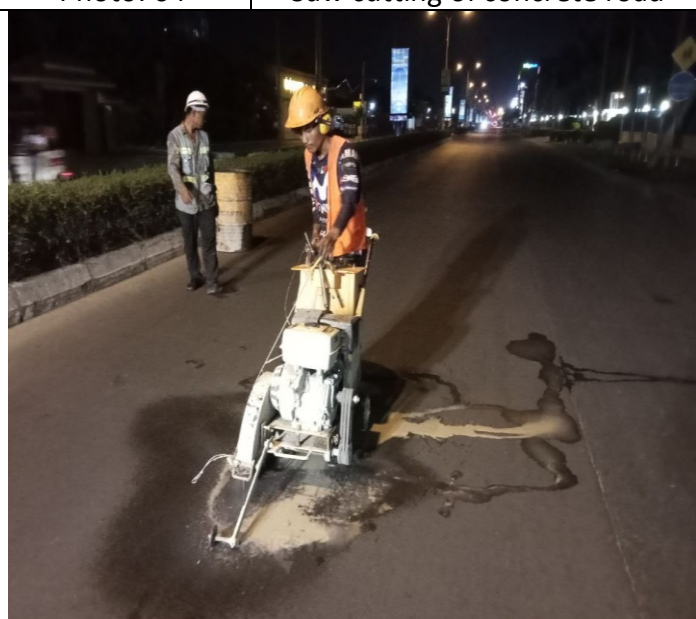
Photo: 06 Saw cutting of concrete road
