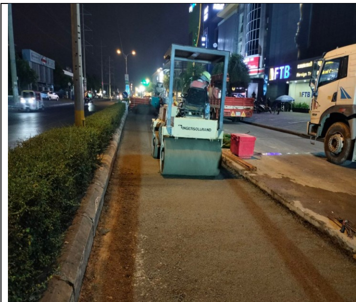
Base course backfilling and compaction
