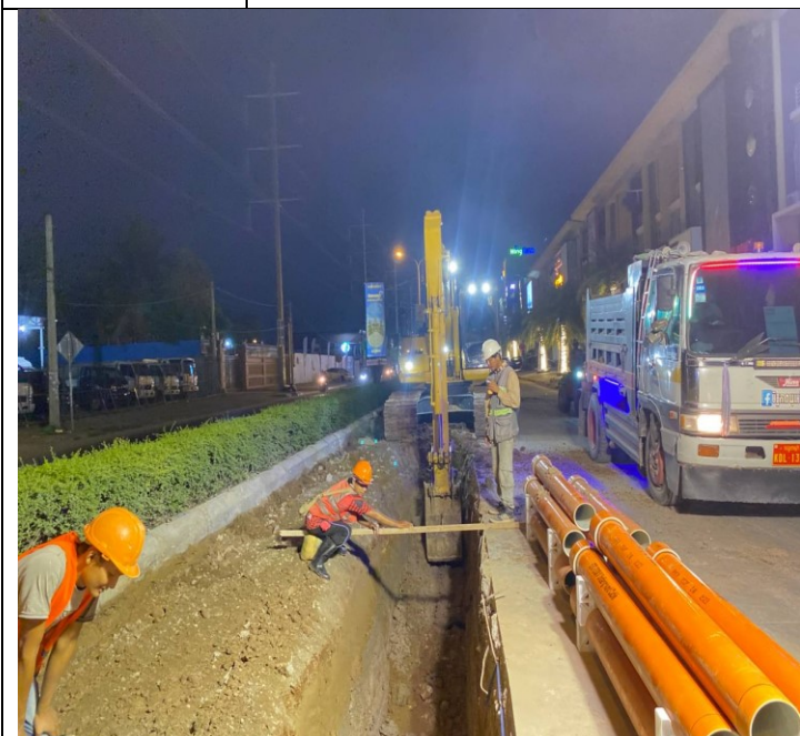
Photo: 11 Soil excavation and concrete road
