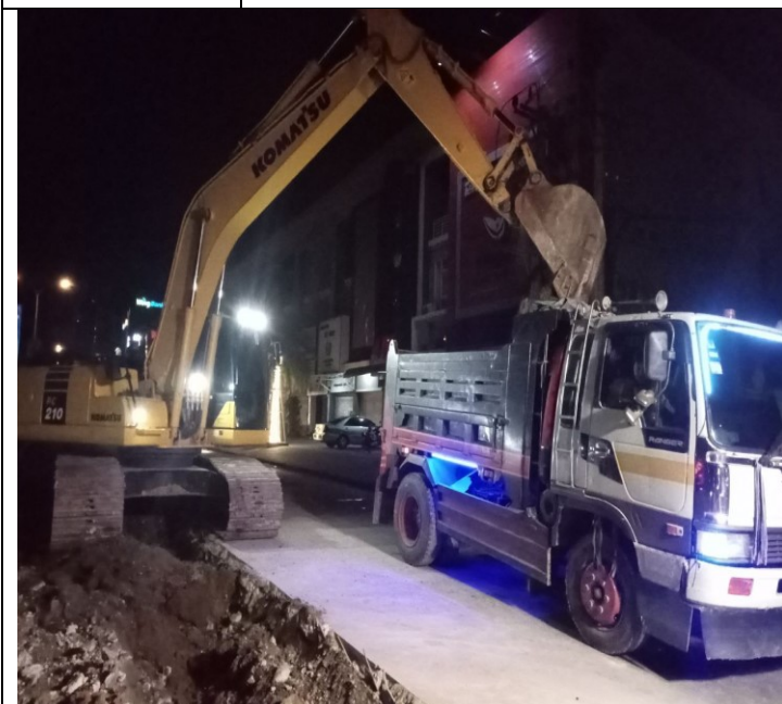
Photo: 09 Soil excavation and concrete road
