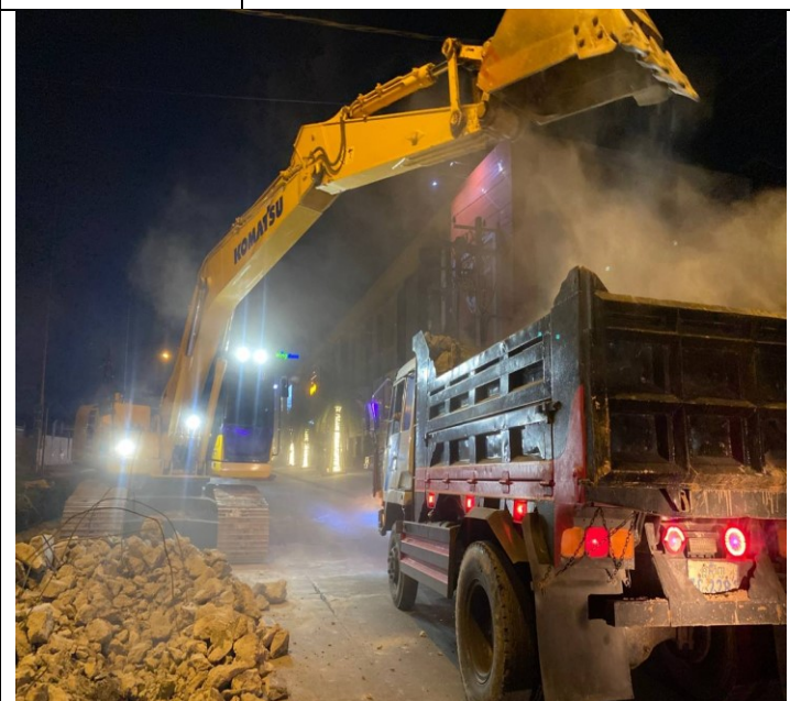
Photo: 05 Soil excavation and concrete road
