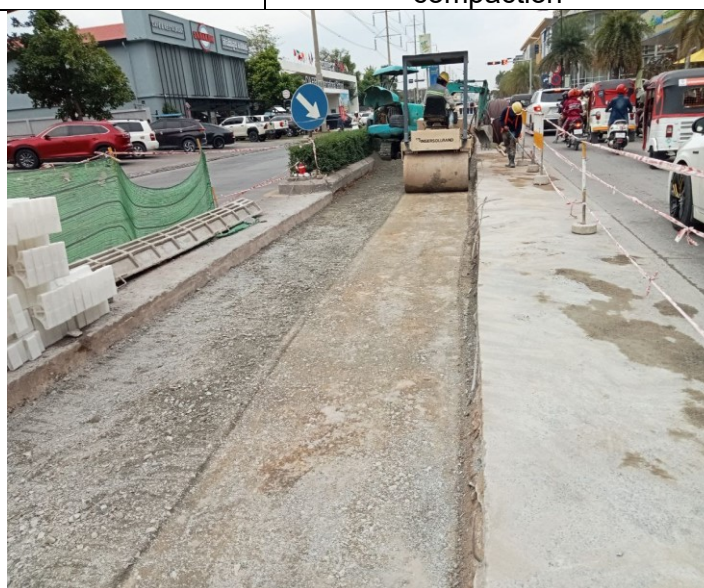
Base course backfilling and compaction
