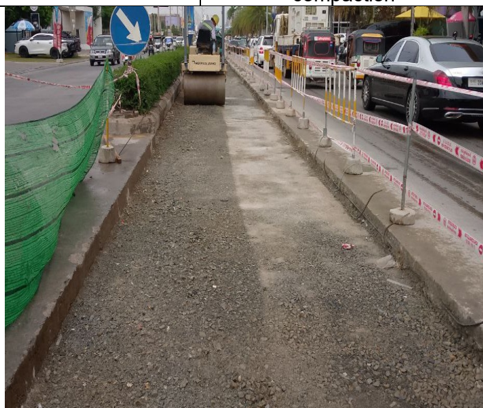
Base course backfilling and compaction
