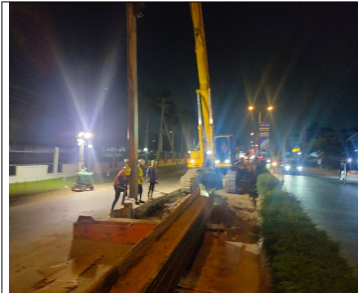
Photo: 01 Sheet Pile Installation activity
