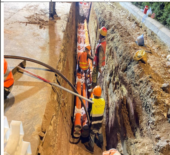
Photo: 09 Assembly PFP pipes and OFC pipe
