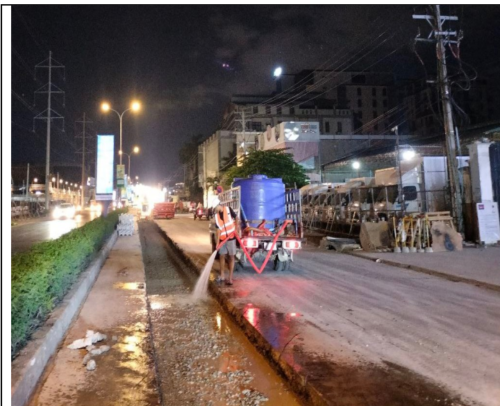
Base course backfilling and compaction
