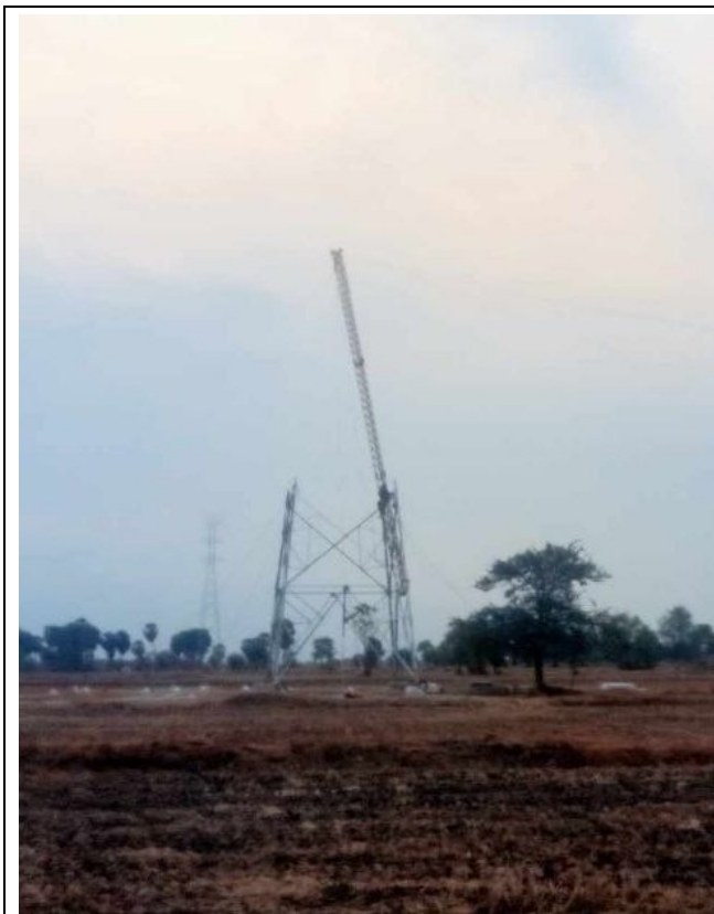
TA070 Tower erection .
