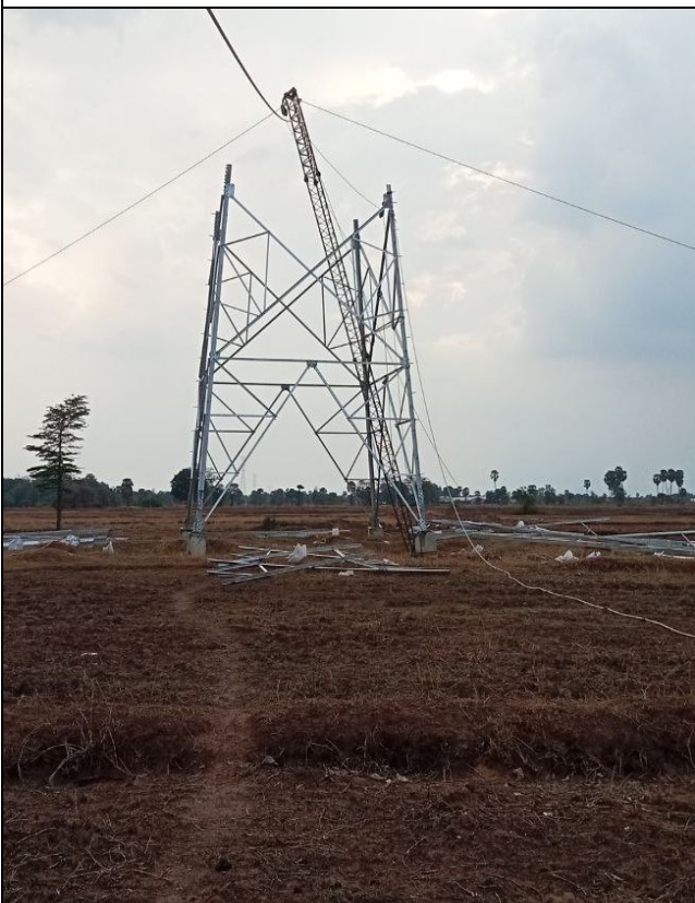
TA066 Tower erection .
