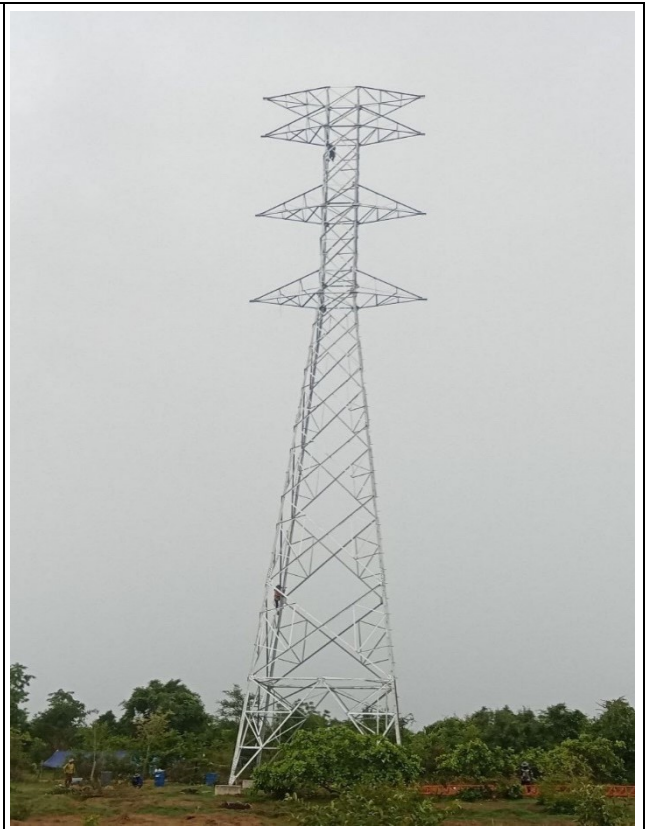
TA112 Tower erection completed .
