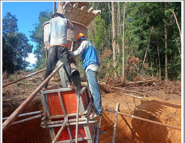
Casting concrete chimney
