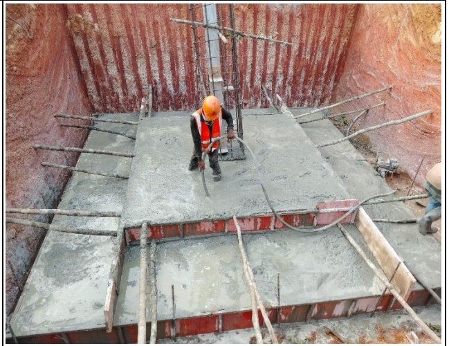
Concrete vibration
