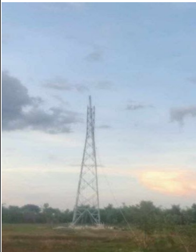
TA104 Tower erection .
