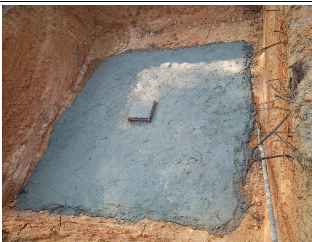
Casting concrete lean.
