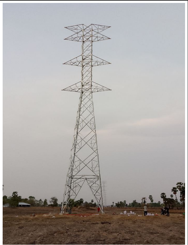
TA040 Erection completd.
