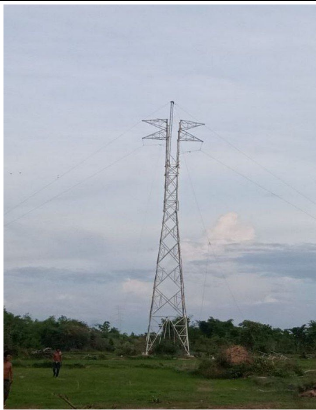
TA098 Tower erection .
