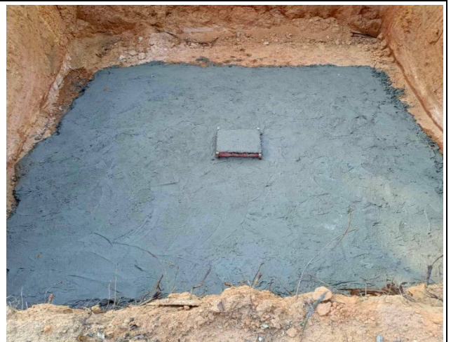
Casting concrete lean.
