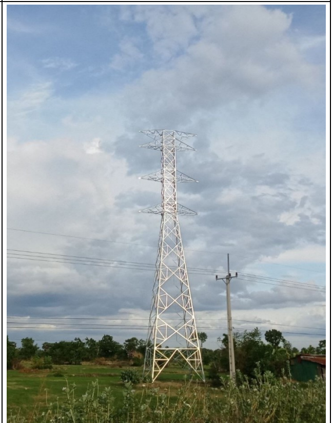
TA116 Tower erection completed .
