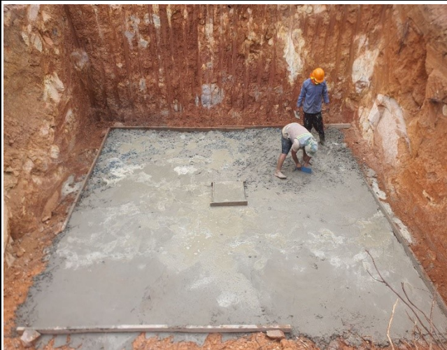
Casting concrete lean
