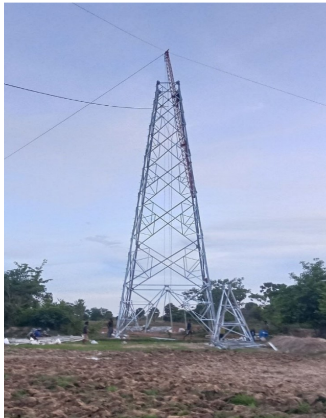
TA108 Tower erection .
