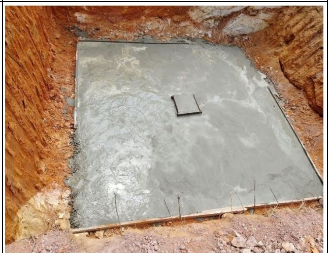
Casting concrete lean
