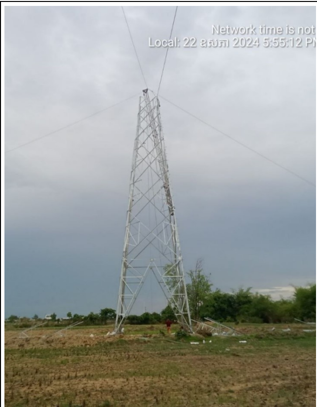
TA095 Tower erection .
