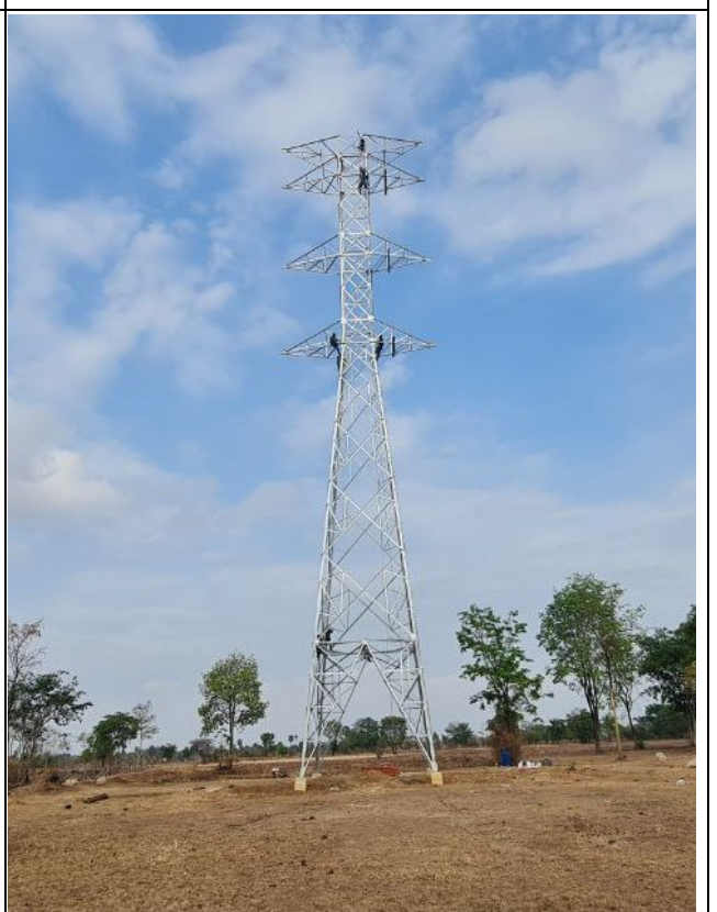
TA064 Tower erection completed.
