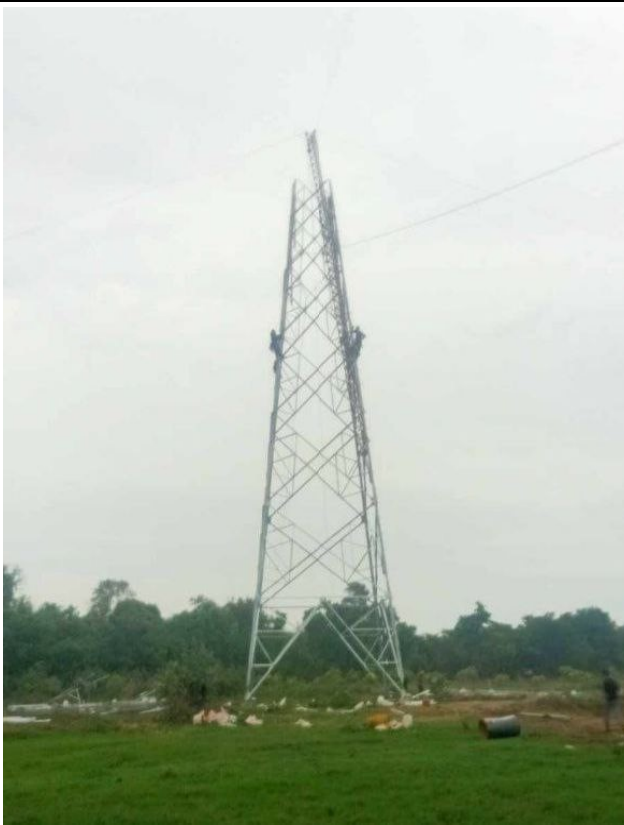
TA123 Tower erection .
