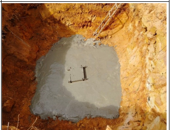
Casting concrete lean
