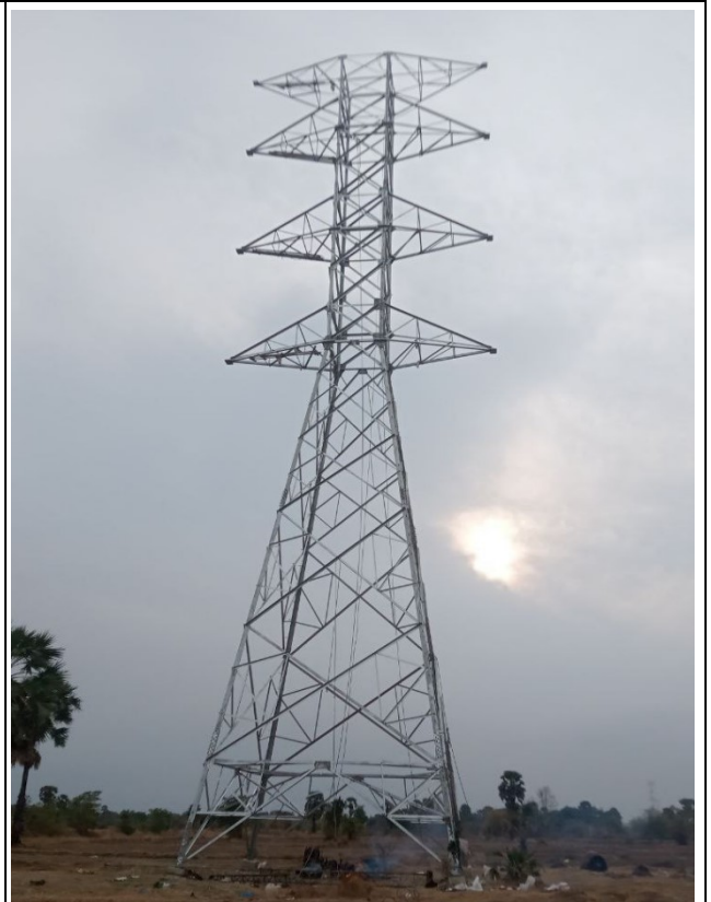
TA048 Tower erection completed.
