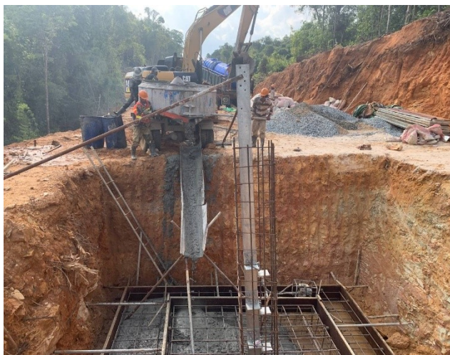
Casting concrete base .
