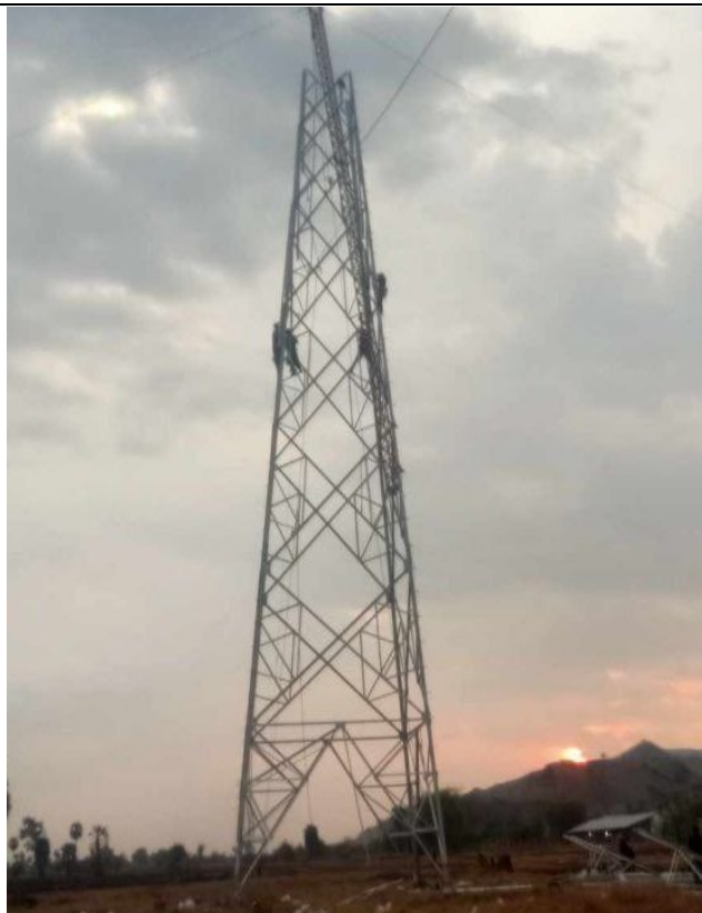
TA039 Tower erection
