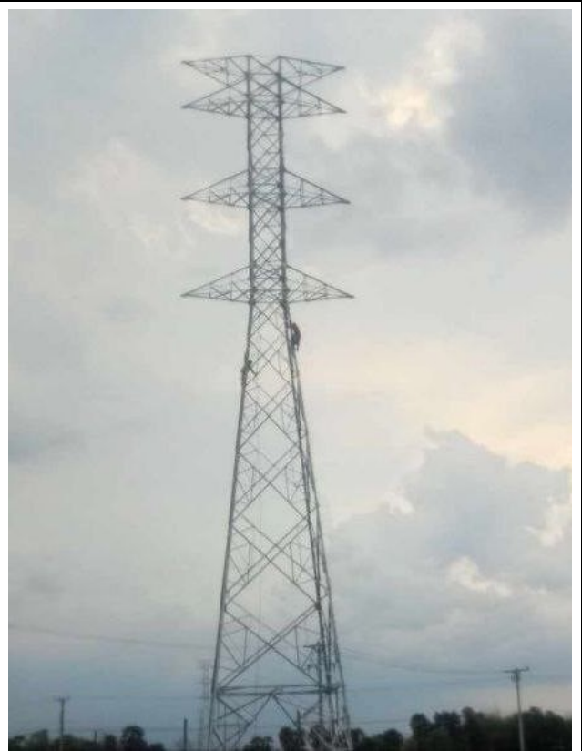
TA023 Erection completed.
