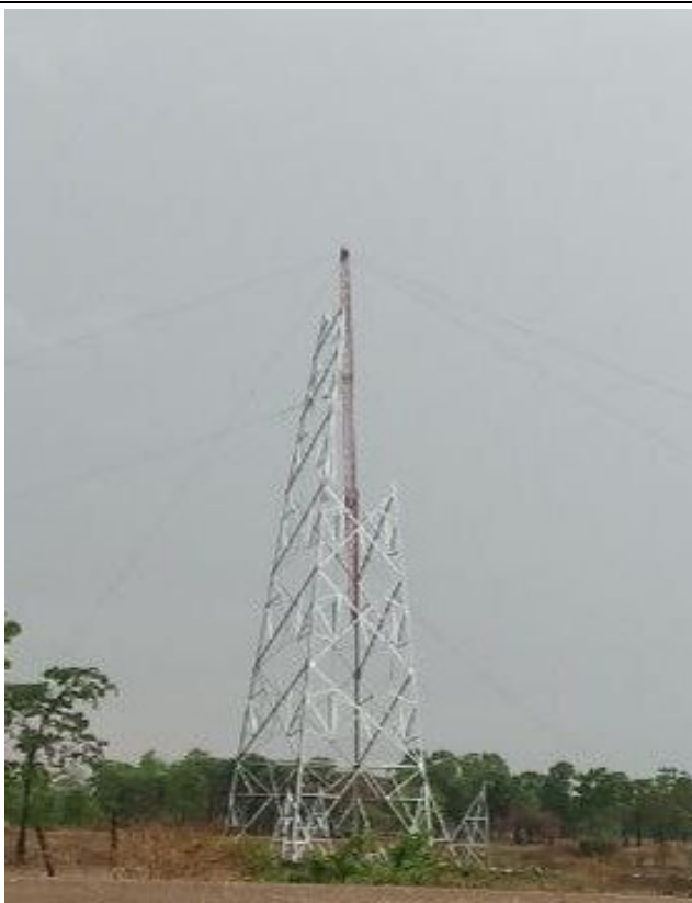
TA080 Tower erection .
