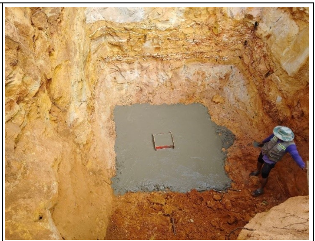
Casting concrete lean
