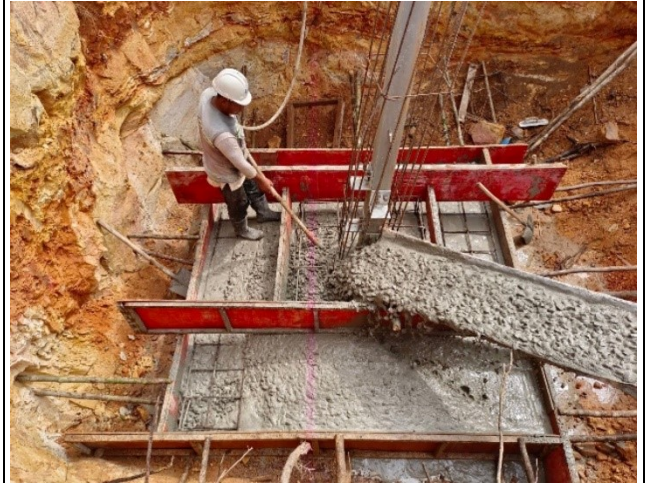
Casting concrete base & Vibration
