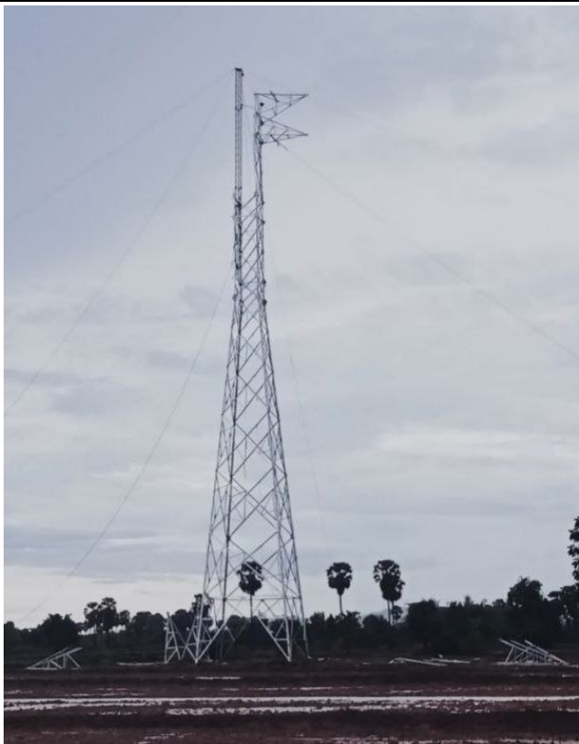
TA106 Tower erection .
