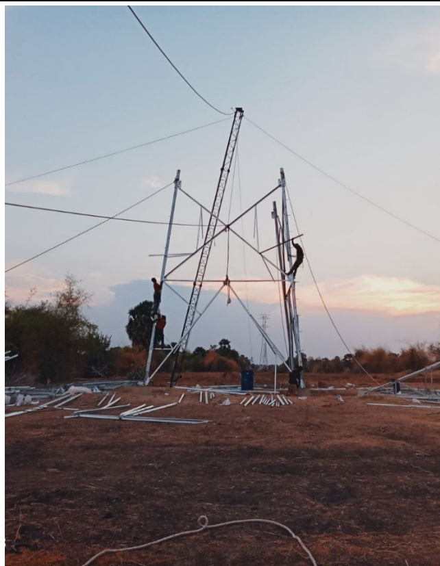
TA046 Tower erection .
