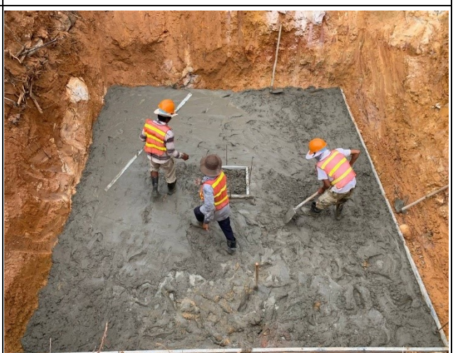
Casting concrete lean.
