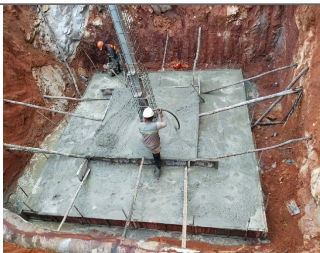
Casting concrete & Concrete vibration
