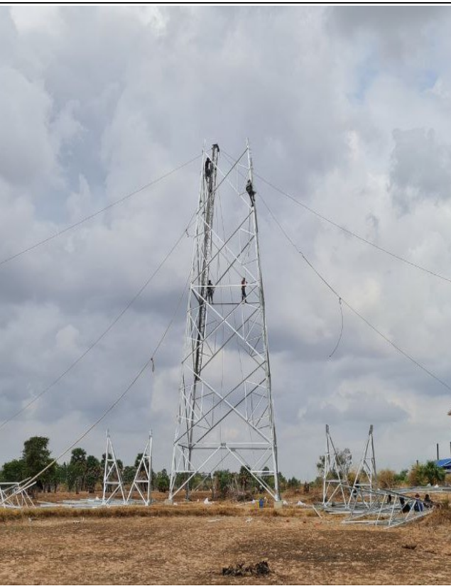
TA045 Tower erection .
