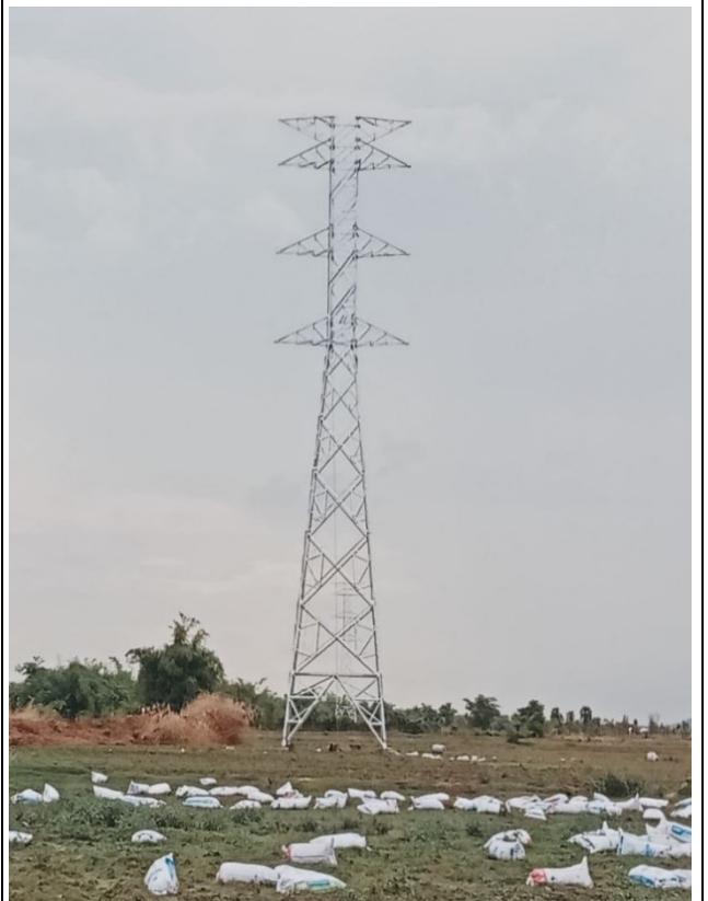
TA094 Tower erection completed .
