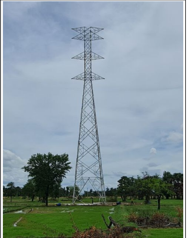
TA068 Tower erection completed.
