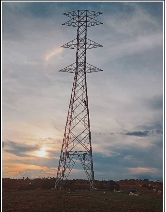
TA093 Tower erection completed .
