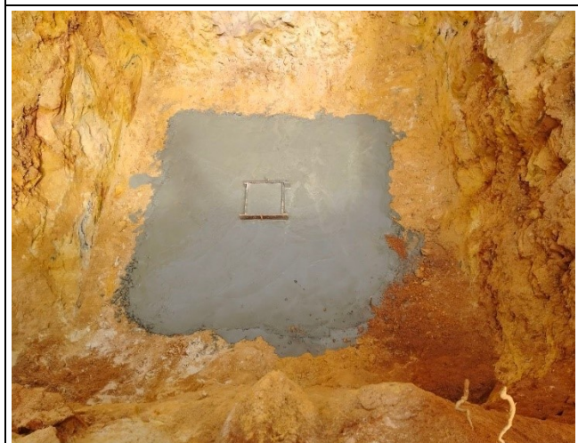
Casting concrete lean
