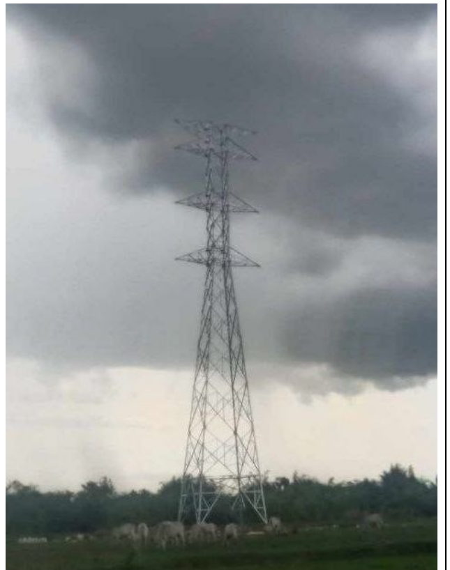
TA104 Tower erection completed .
