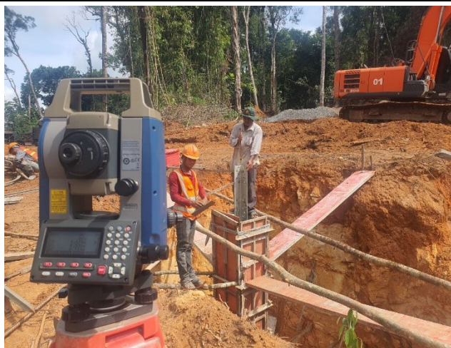
Casting concrete chimney
