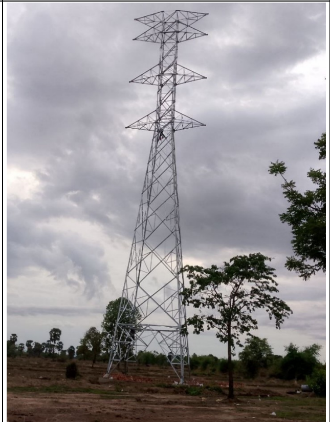
TA080 Tower erection completed .
