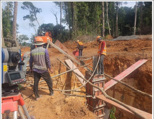
Concrete vibration
