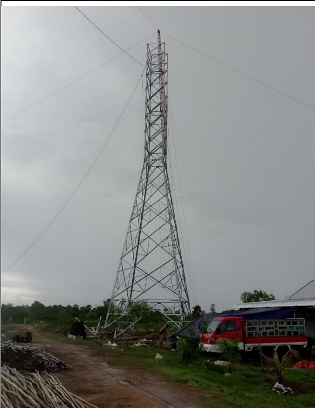
TA121 Tower erection .
