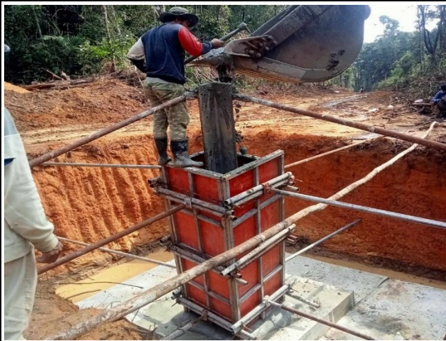
Casting concrete chimney.
