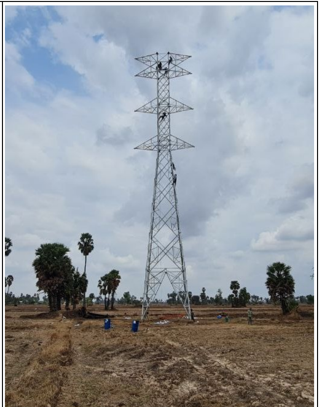
TA058 Tower erection completed
