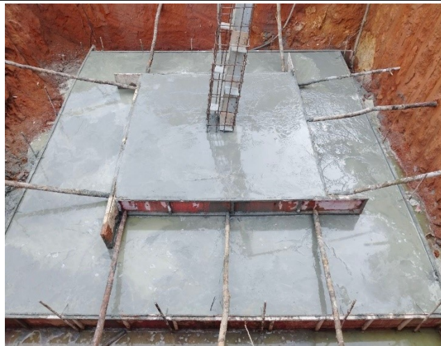
Casting concrete Base
