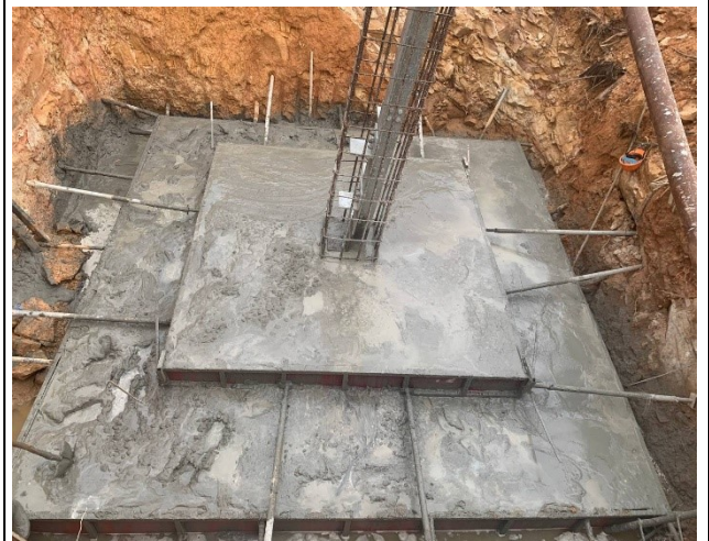
Casting concrete base .
