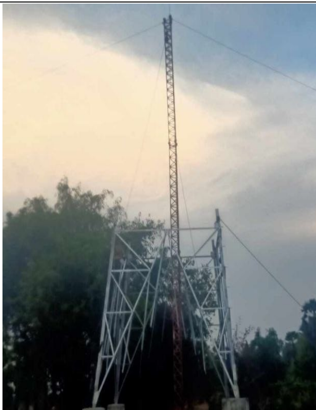
TA077 Tower erection .
