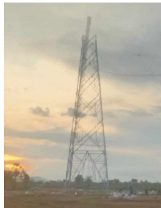
TA084 Tower erection .
