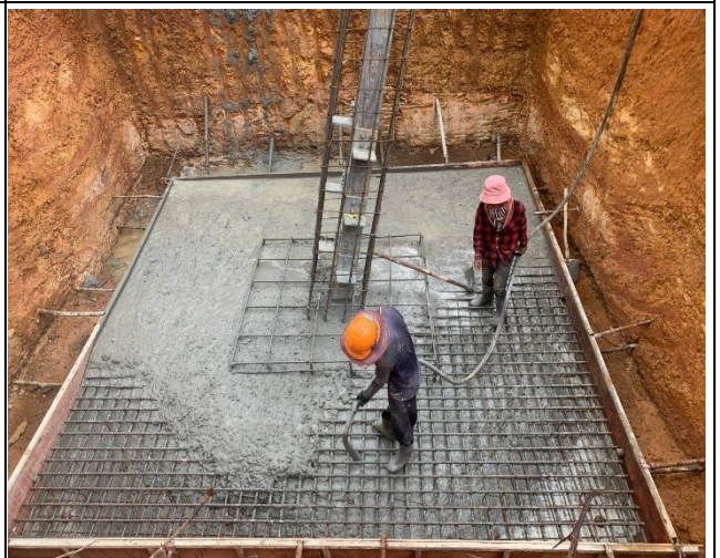
Concrete vibration
