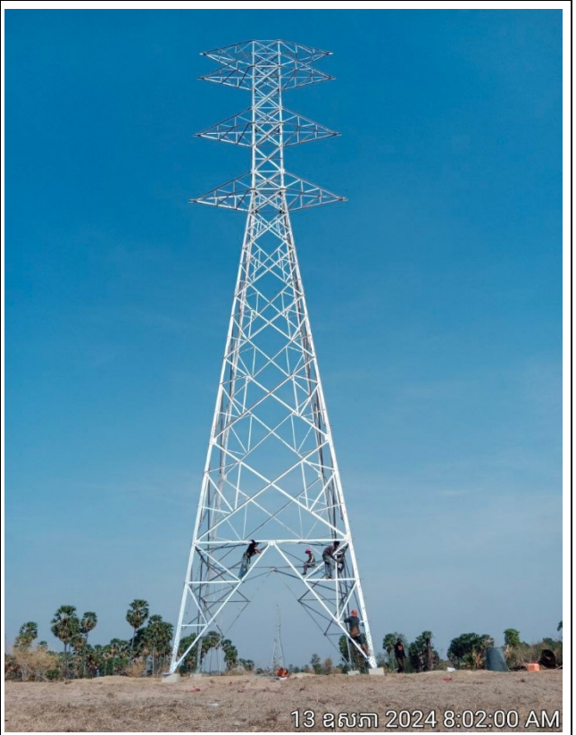
TA047 Tower erection completed.
