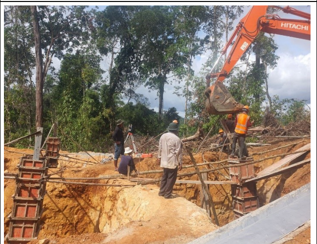
Casting concrete chimney
