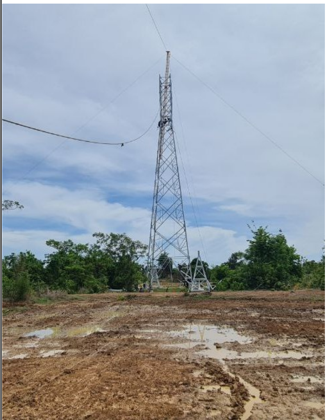
TA108 Tower erection completed .
