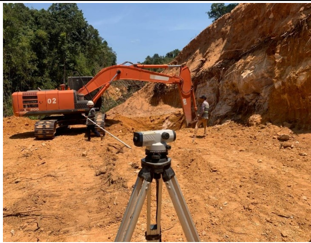
Soil excavatoin of the pit.
