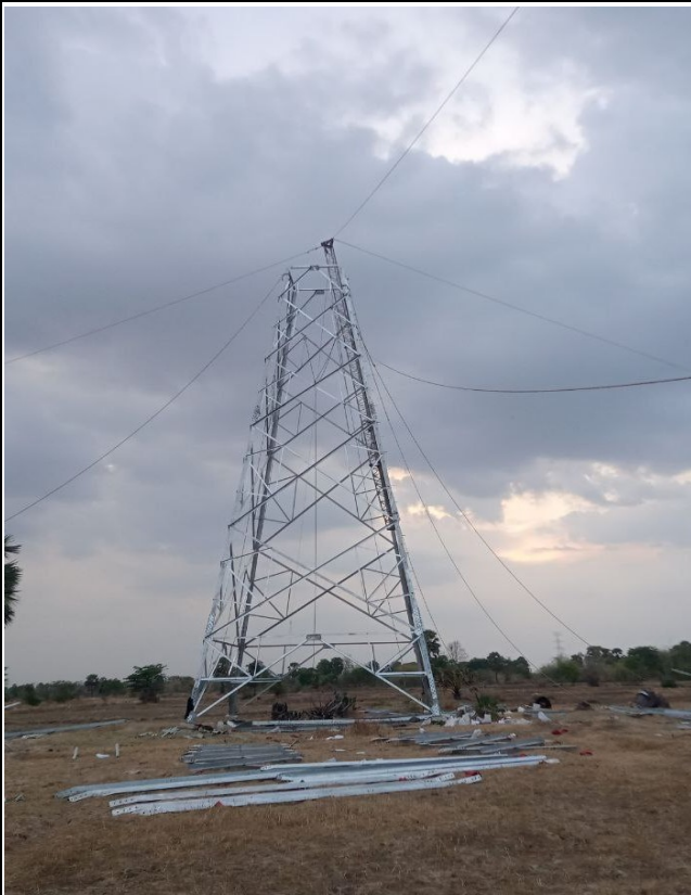
TA048 Tower erection .
