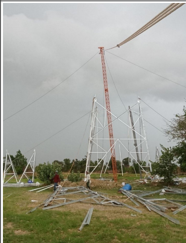
TA116 Tower erection .
