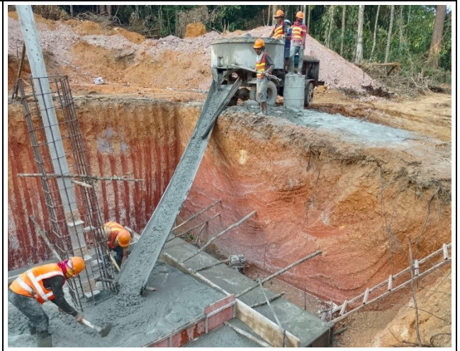
Casting concrete
