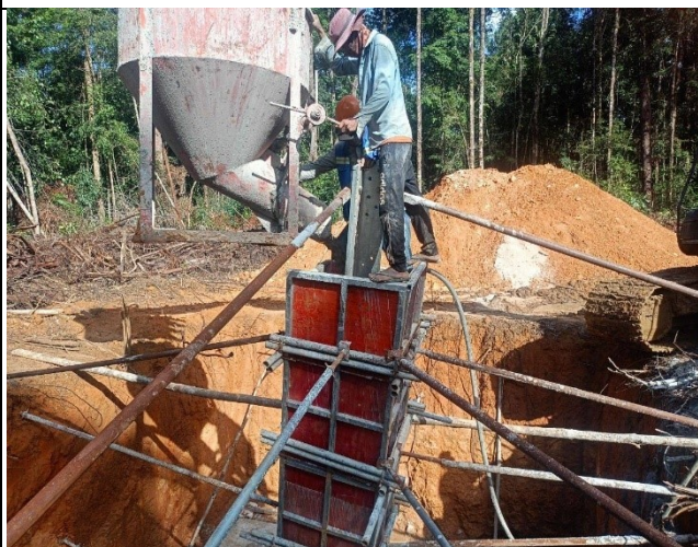
Casting concrete chimney
