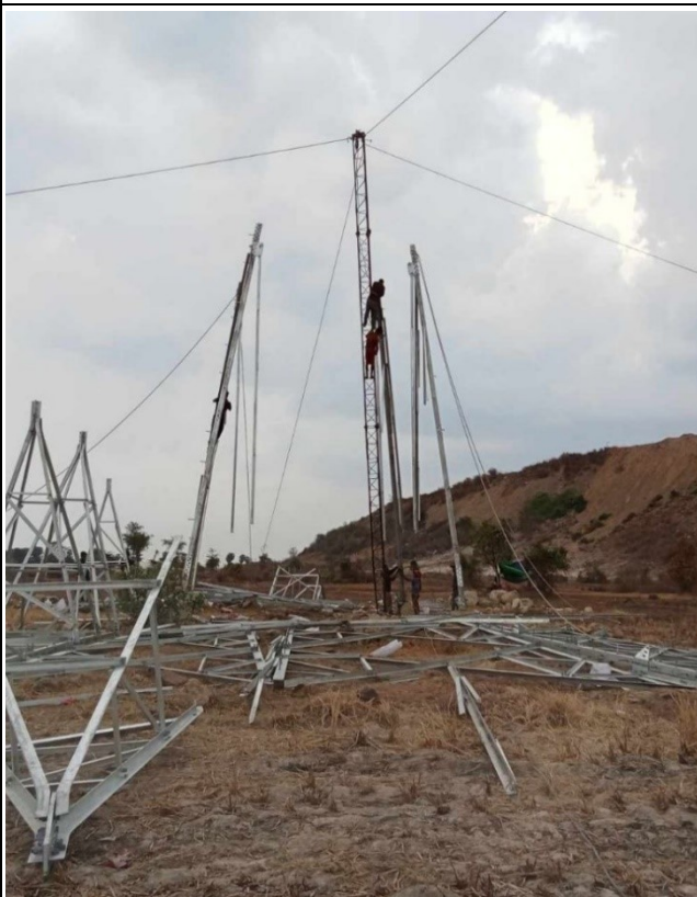
TA043 Tower erection
