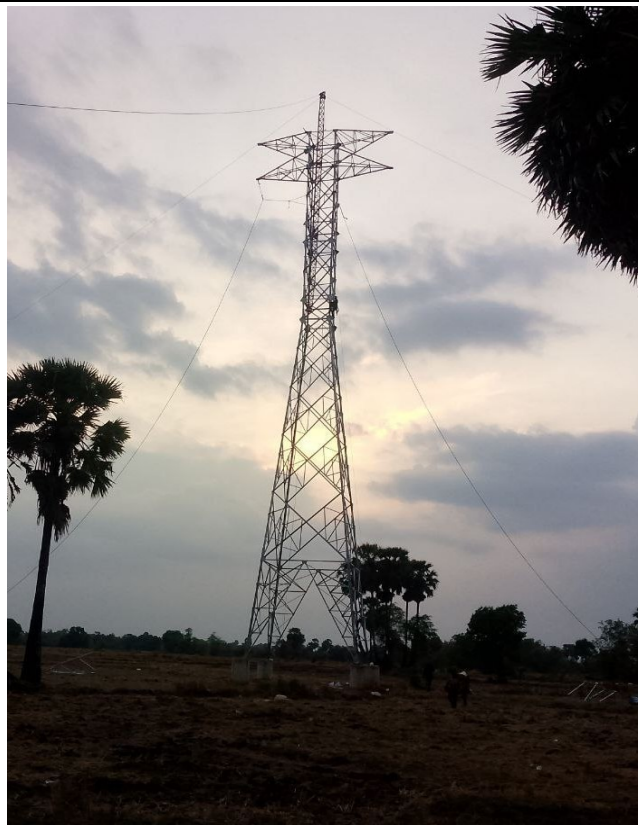
TA078 Tower erection .
