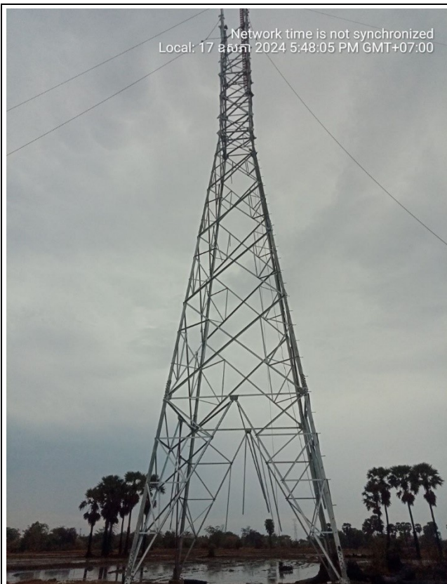
TA062 Tower erection .
