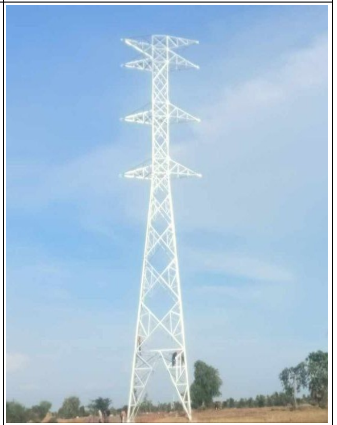
TA084 Tower erection completed .
