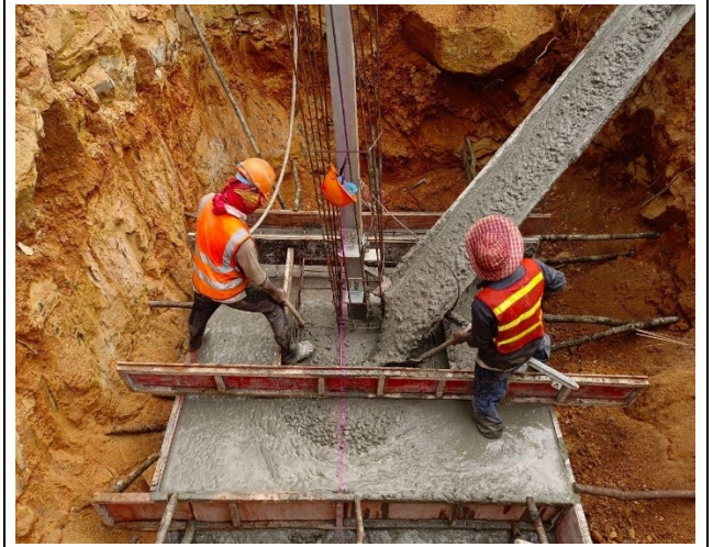
Concrete vibration
