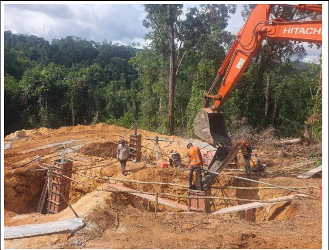
Casting concrete chimney & Vibration
