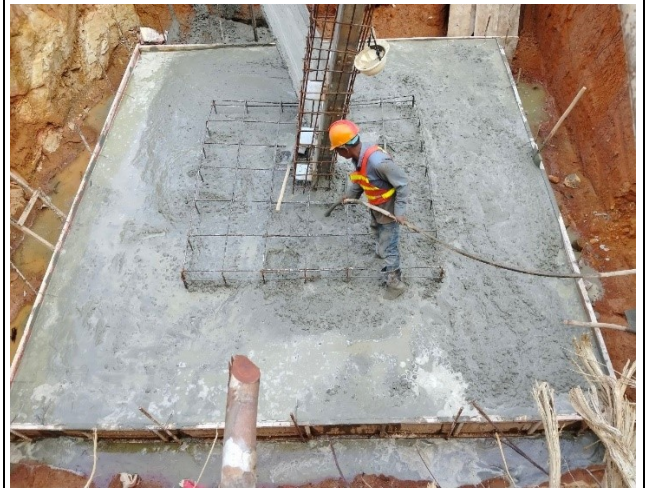
Casting concrete & Concrete vibration
