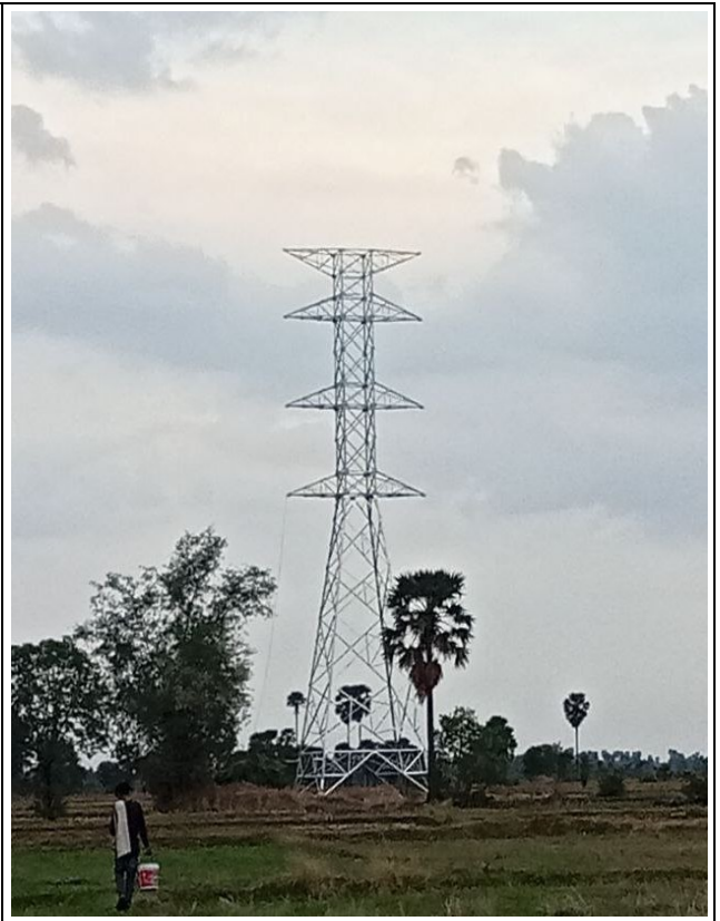
TA067 Tower erection completed.
