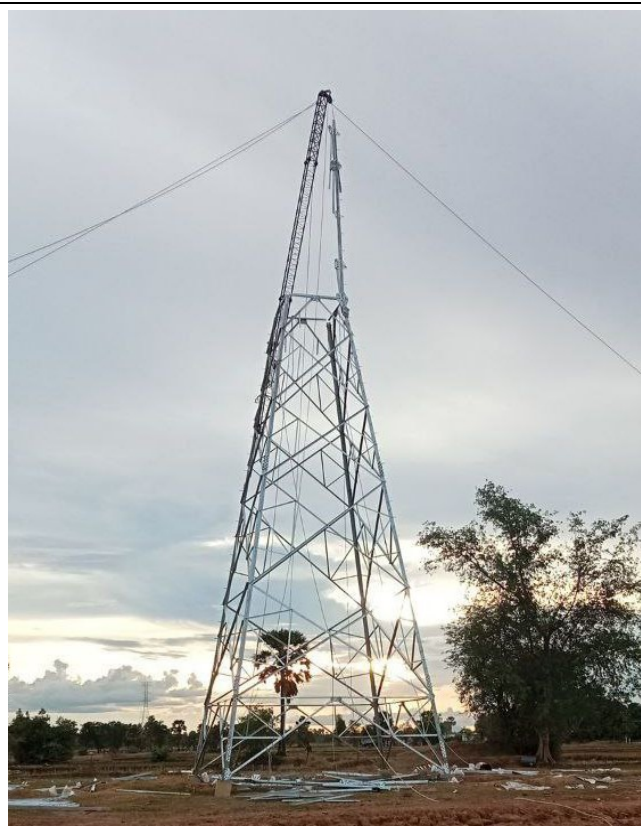
TA067 Tower erection .
