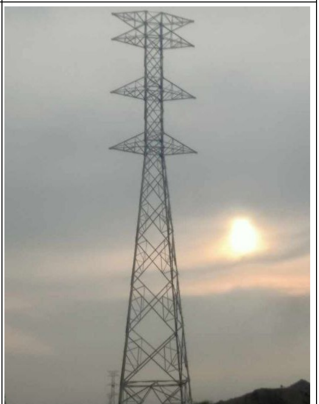
TA039 Erection completd.
