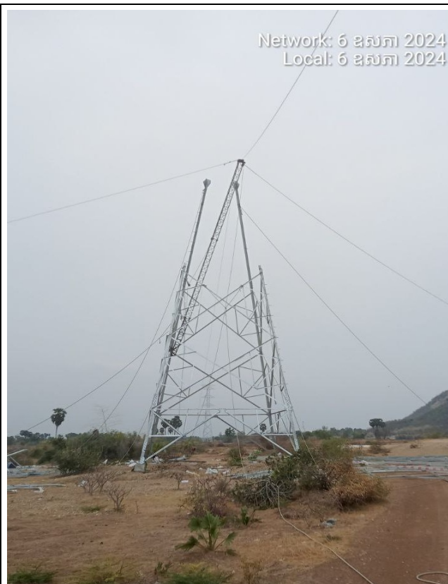
TA042 Tower erection
