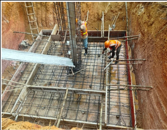
Install rebar , formwork & cleaning
