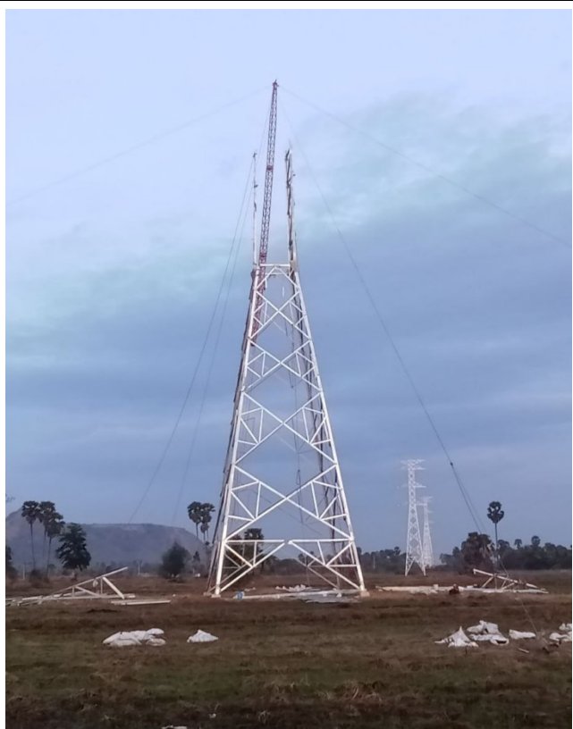
TA059 Tower erection .
