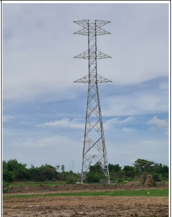
TA098 Tower erection completed .
