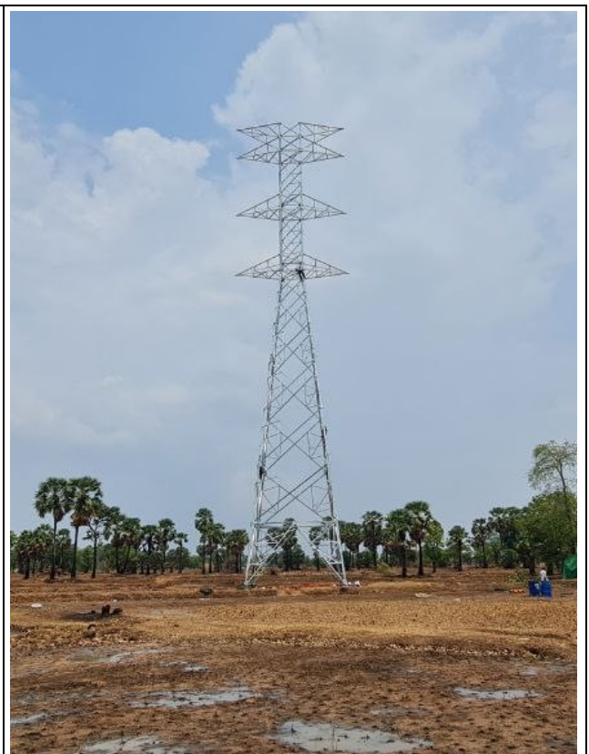
TA070 Tower erection completed .
