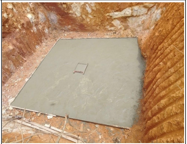
Casting concrete lean
