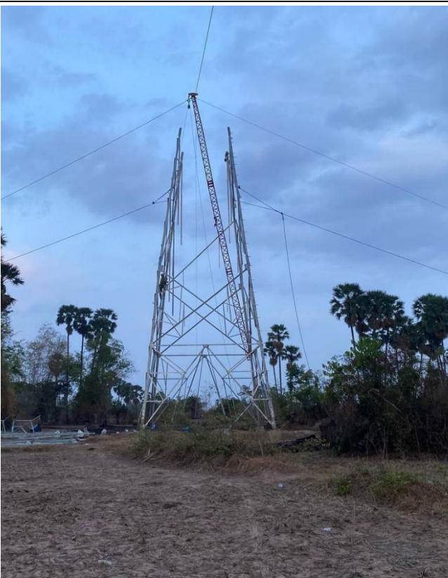
TA055 Tower erection .
