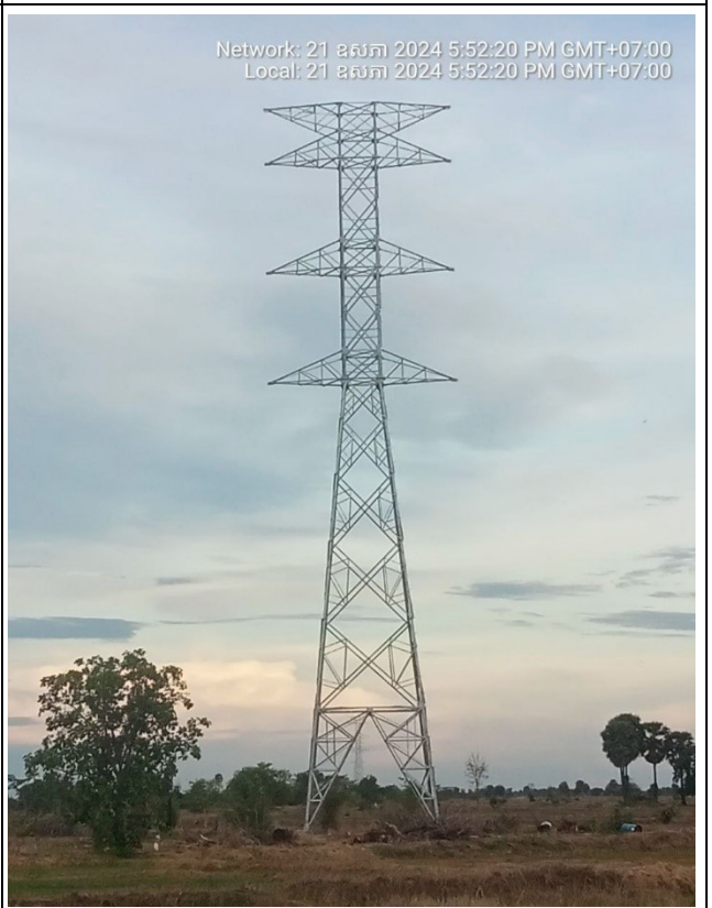
TA087 Tower erection completed .
