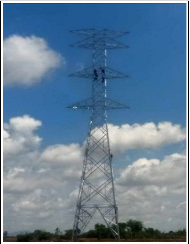
TA085 Tower erection completed .
