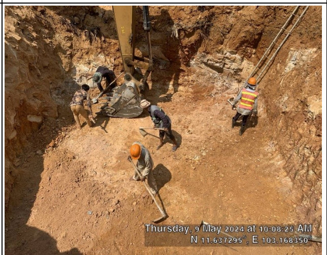
Soil cleaning of the pit .
