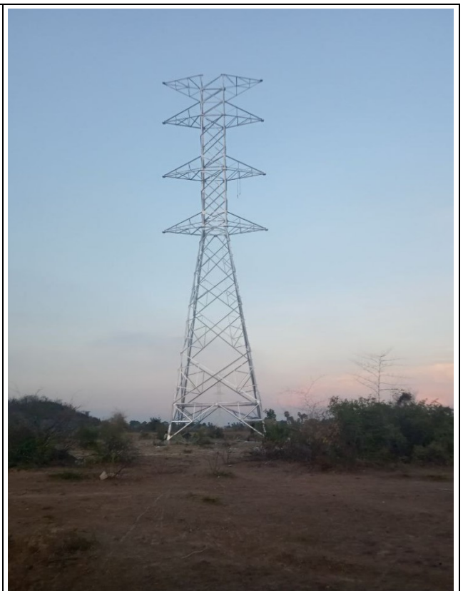
TA042 Erection completd.
