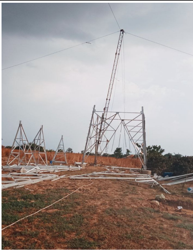
TA093 Tower erection .
