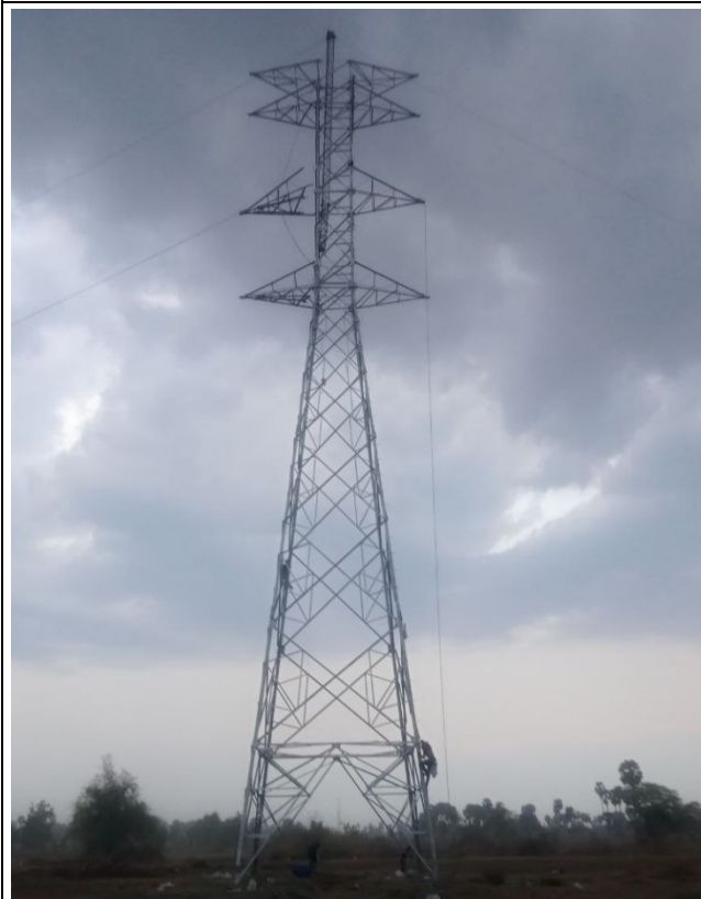
TA041 Tower erection
