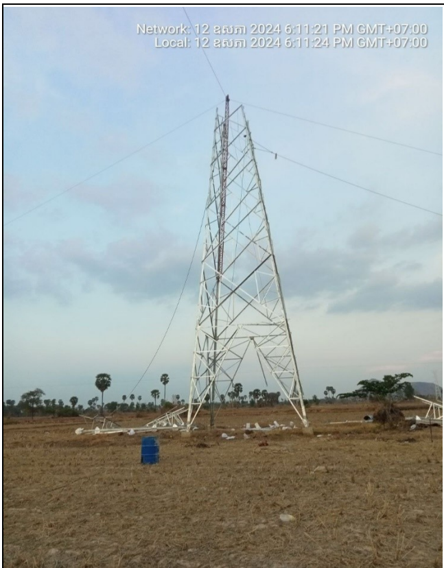
TA060 Tower erection .
