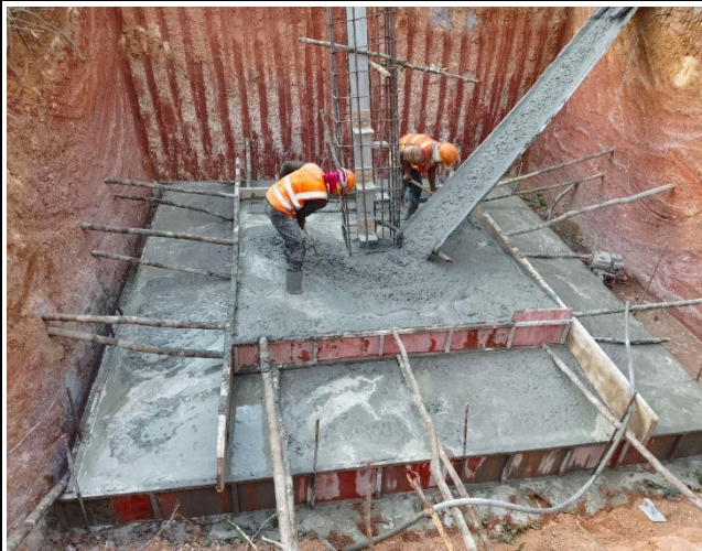
Casting concrete
