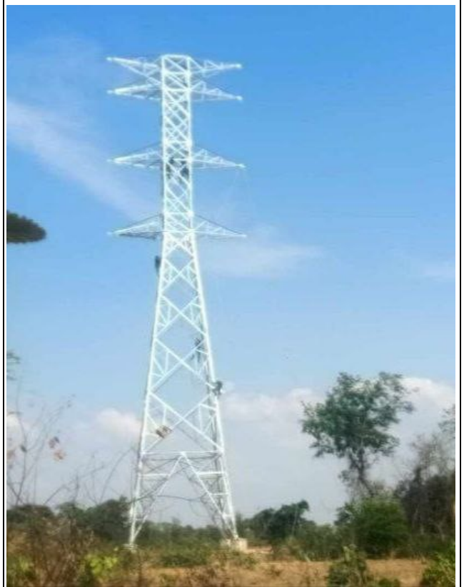
TA076 Tower erection completed .
