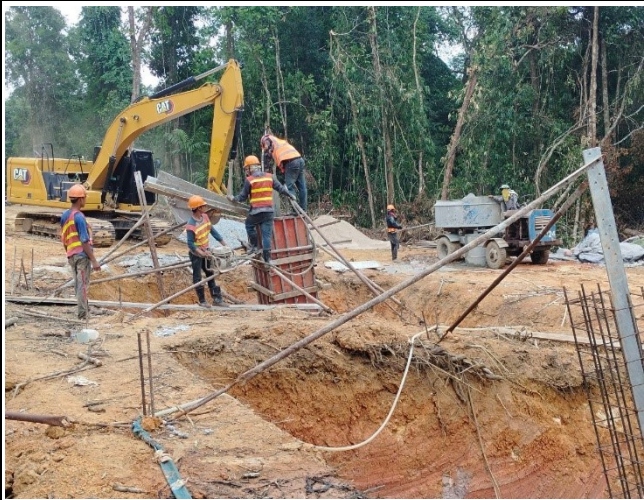
Concrete vibration
