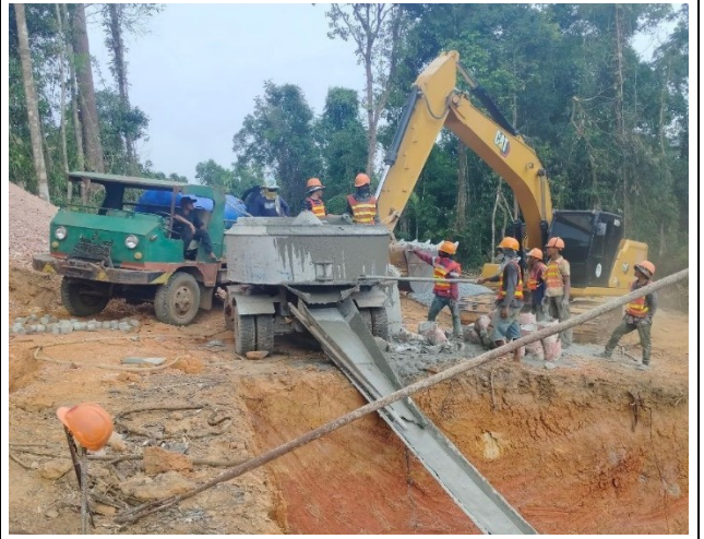
Casting concrete mixing
