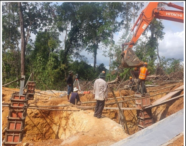
Casting concrete chimney
