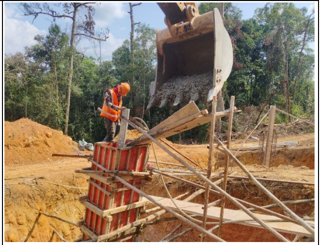
Casting concrete
