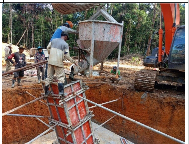
Casting concrete chimney
