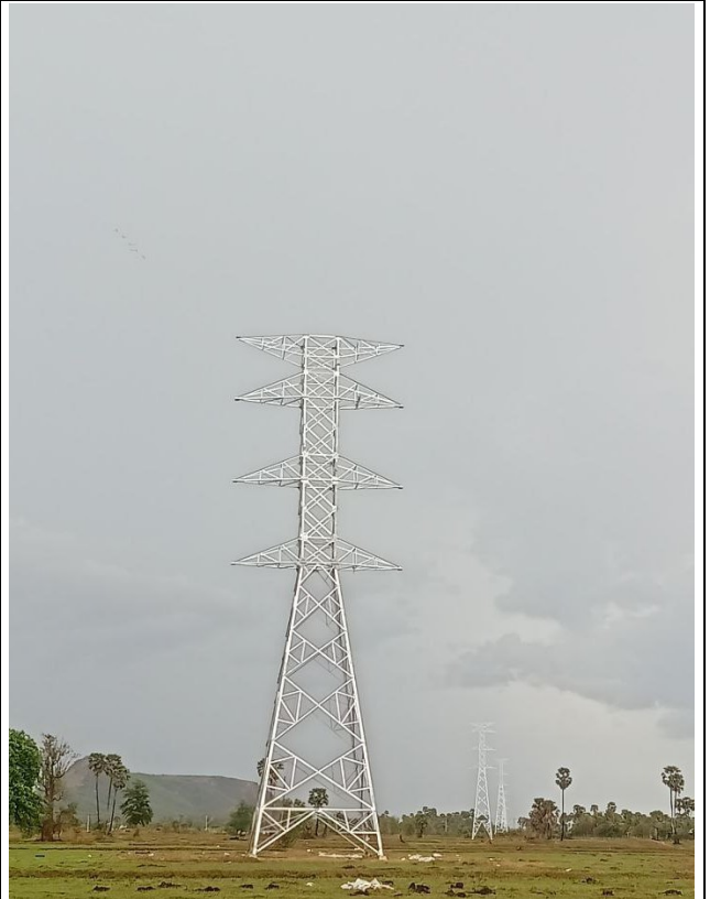
TA059 Tower erection completed
