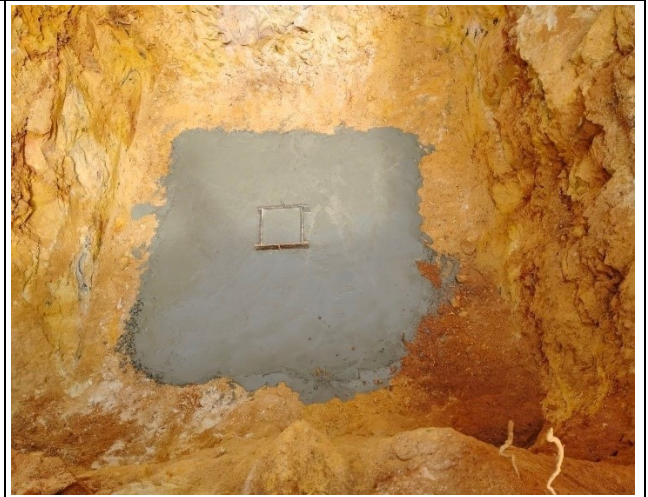
Casting concrete lean
