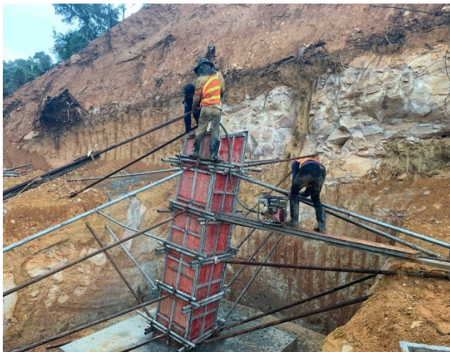
Concrete vibration.
