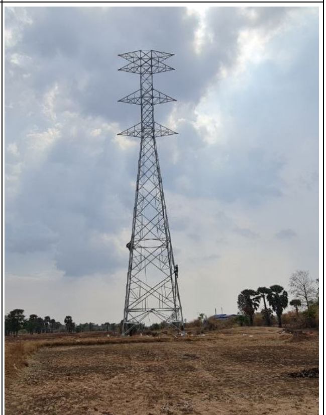
TA045 Tower erection completed .
