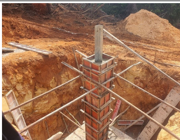
Casting concrete chimney
