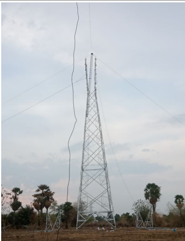
TA049 Tower erection .
