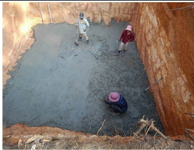
Casting concrete lean.
