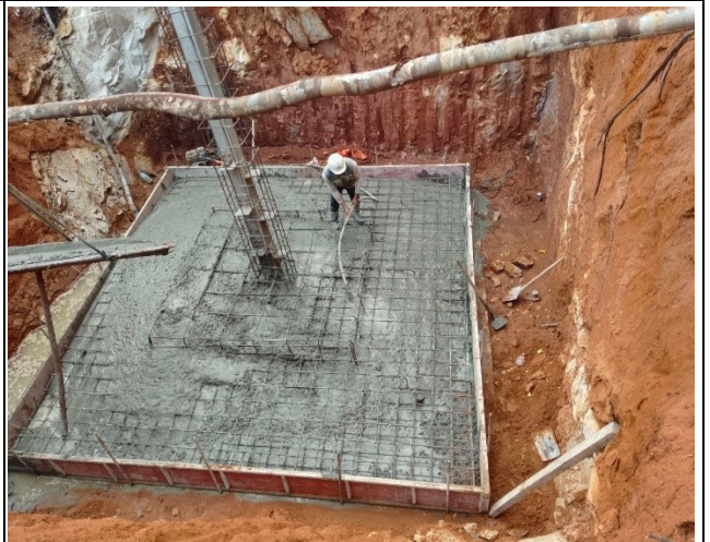
Casting concrete & Concrete vibration
