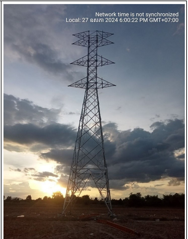
TA088 Tower erection completed .
