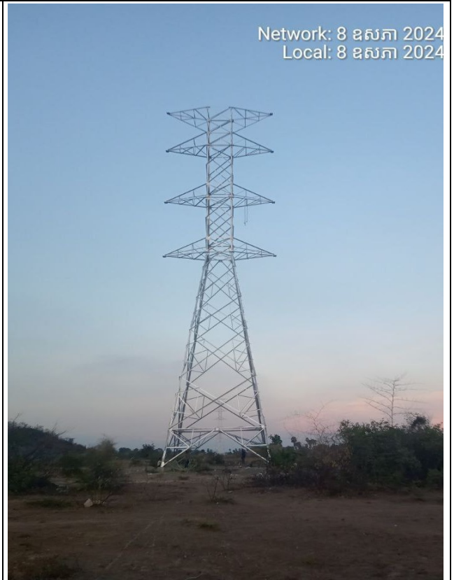
TA044 Tower erection completed .
