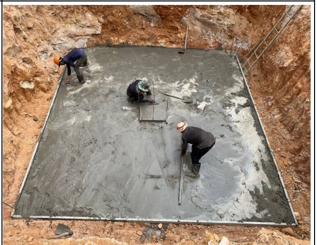
Casting concrete lean.
