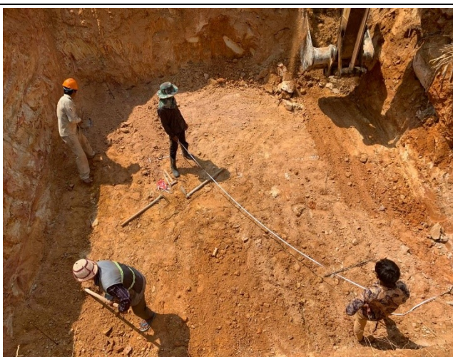
Soil cleaning of the pit .
