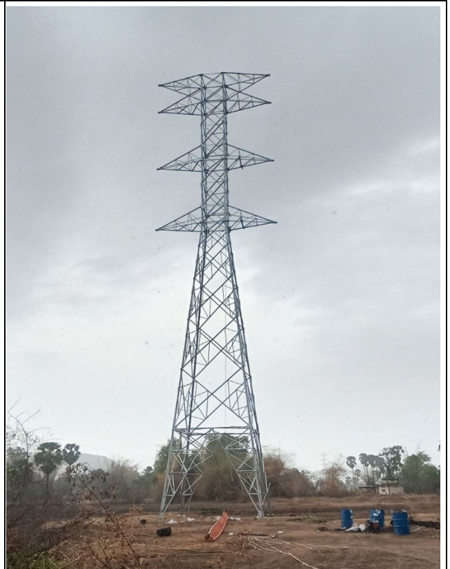
TA054 Tower erection completed.
