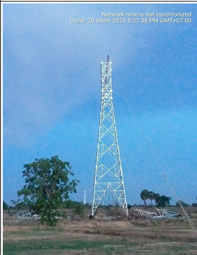
TA087 Tower erection .
