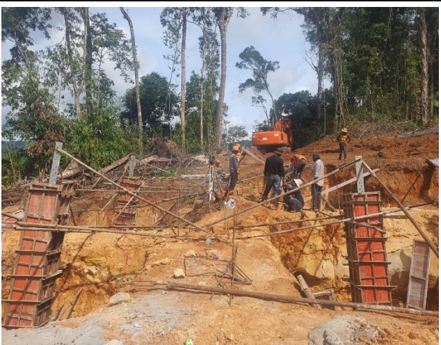
Casting concrete chimney
