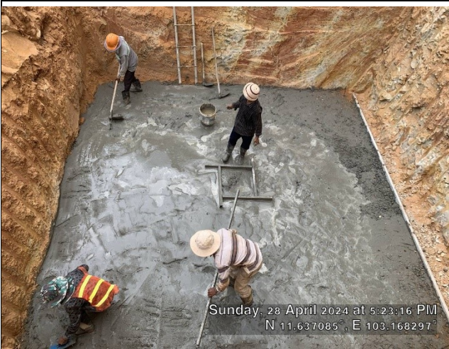
Casting concrete lean.
