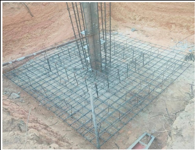
Install rebar .
