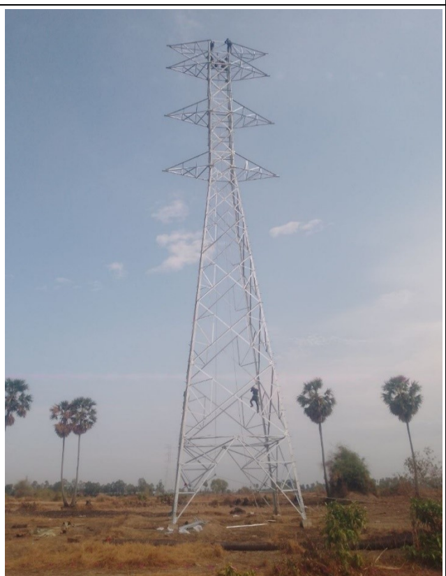
TA029 Erection completd.
