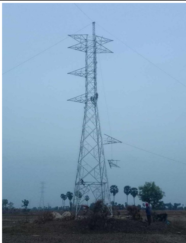
TA044 Tower erection .
