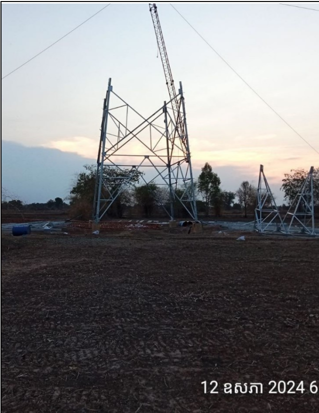
TA065 Tower erection .
