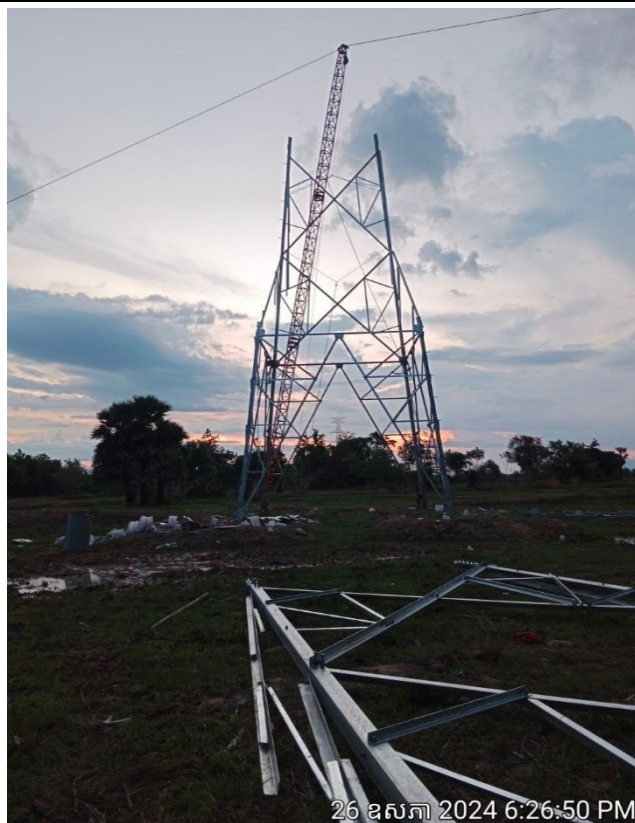
TA101 Tower erection .
