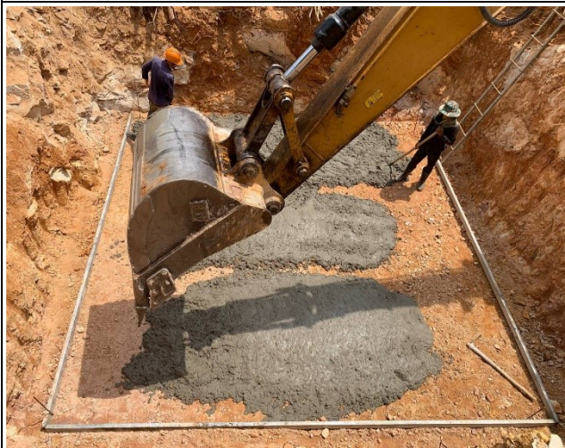
Casting concrete lean.
