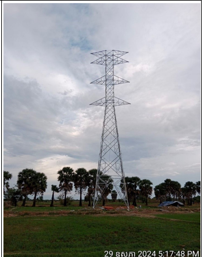
TA101 Tower erection completed .
