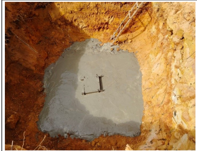
Casting concrete lean
