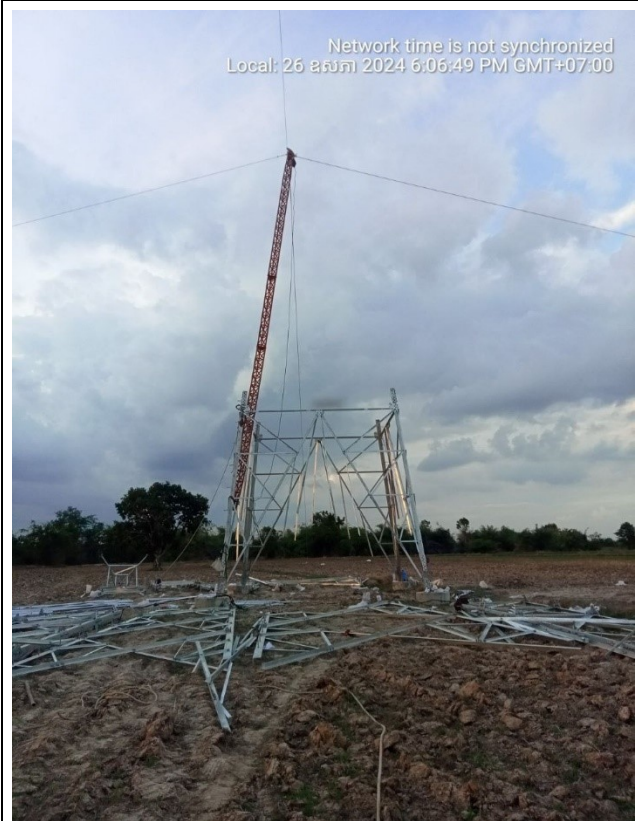
TA089 Tower erection .
