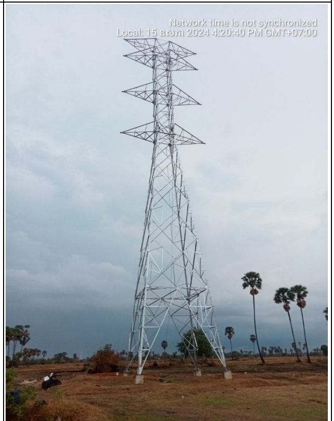
TA061 Tower erection completed.
