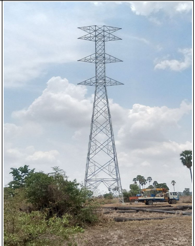
TA055 Tower erection completed.
