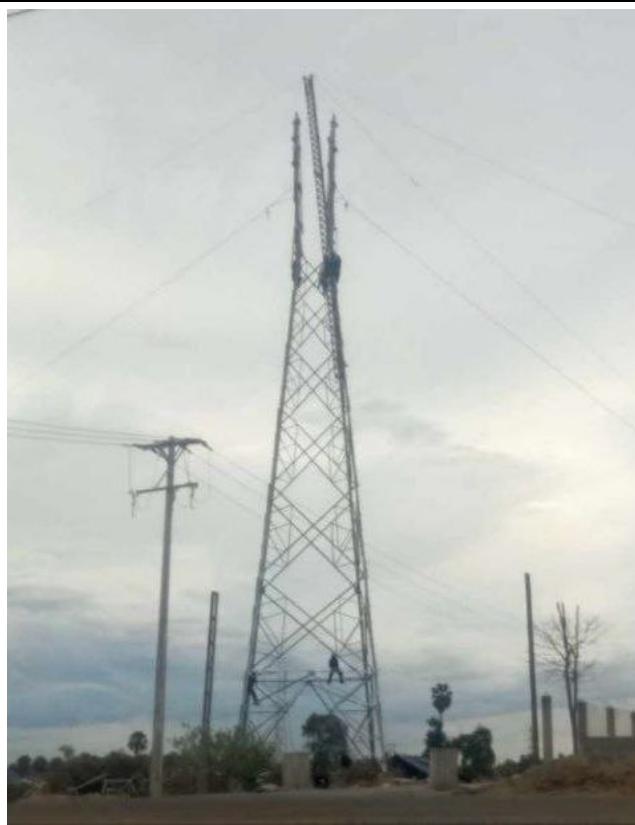
TA023 Tower erection
