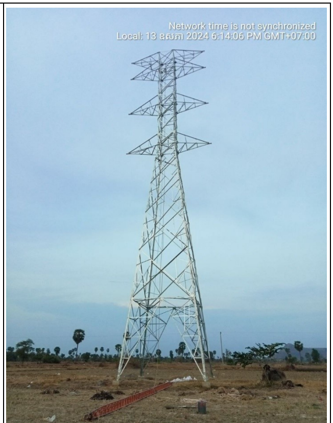
TA060 Tower erection completed.
