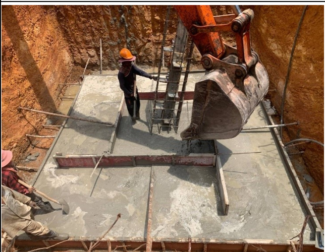
Casting concrete base.
