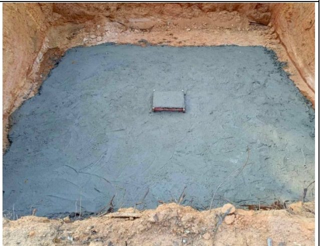
Casting concrete lean.
