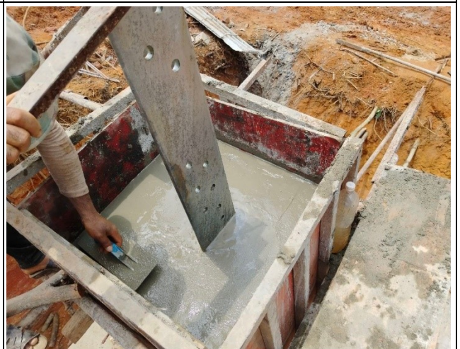
Concrete leveling
