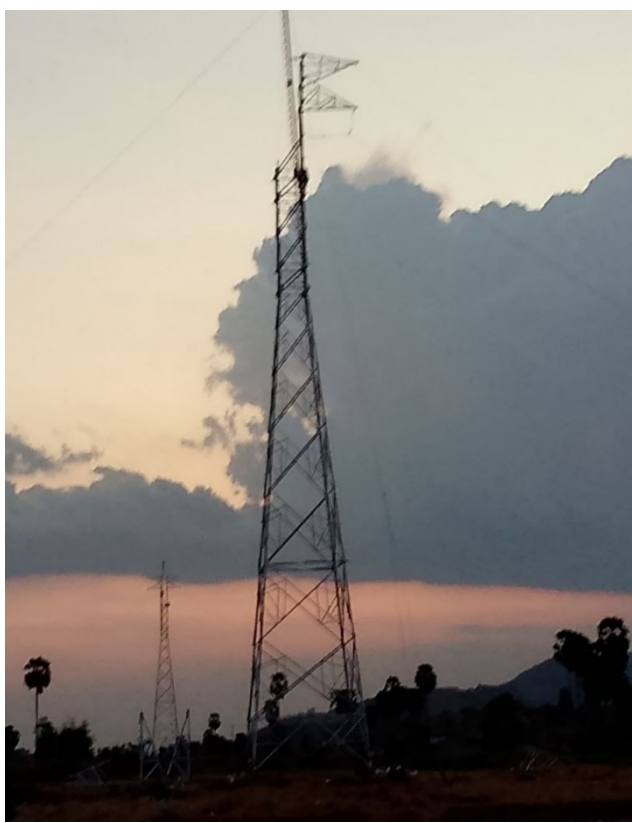
TA038 Tower erection
