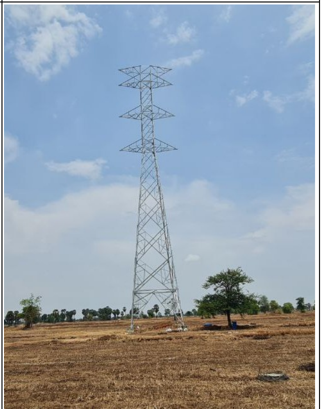
TA073 Tower erection completed.
