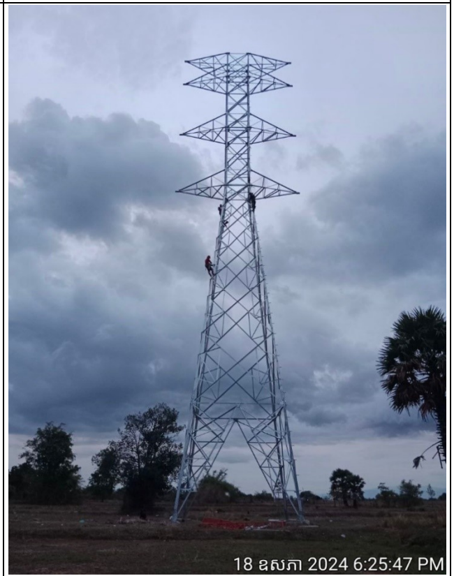
TA091 Tower erection completed .
