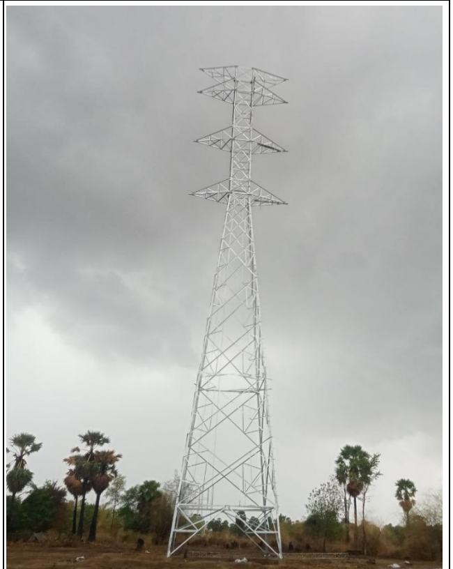
TA049 Tower erection completed.
