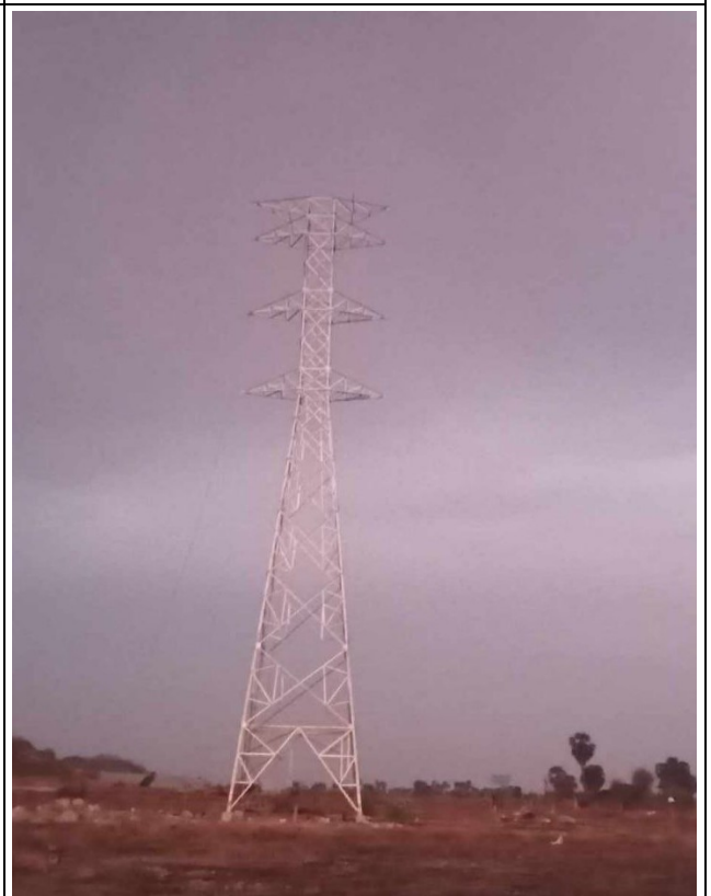
TA043 Erection completd.
