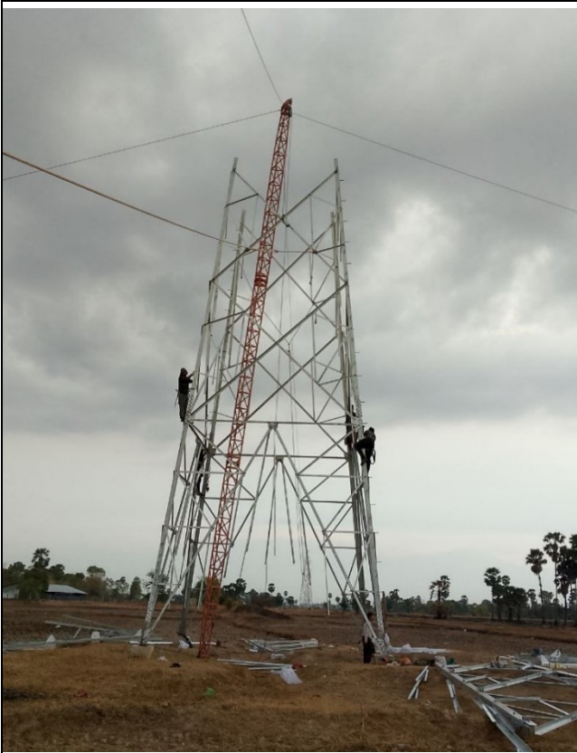
TA040 Tower erection
