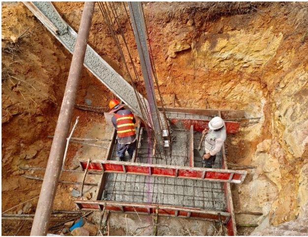
Casting concrete base
