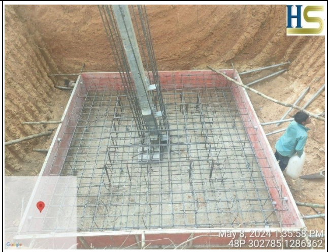
Install formworks.
