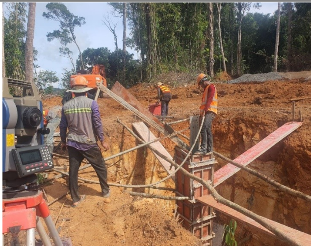
Casting concrete chimney
