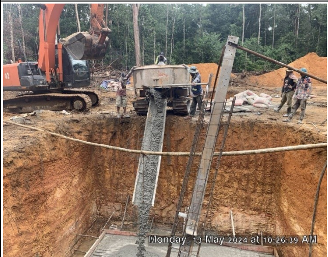
Casting concrete base
