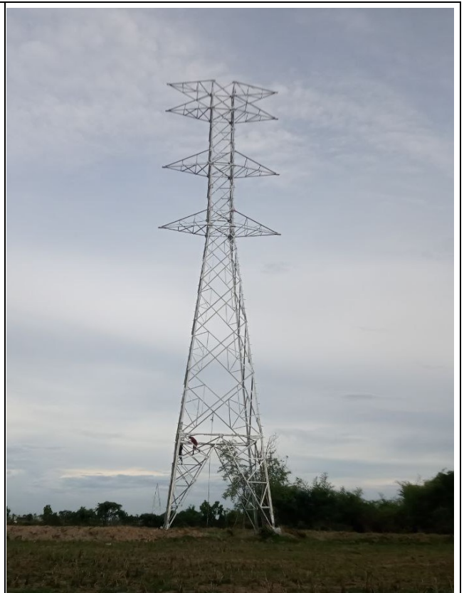
TA095 Tower erection completed .
