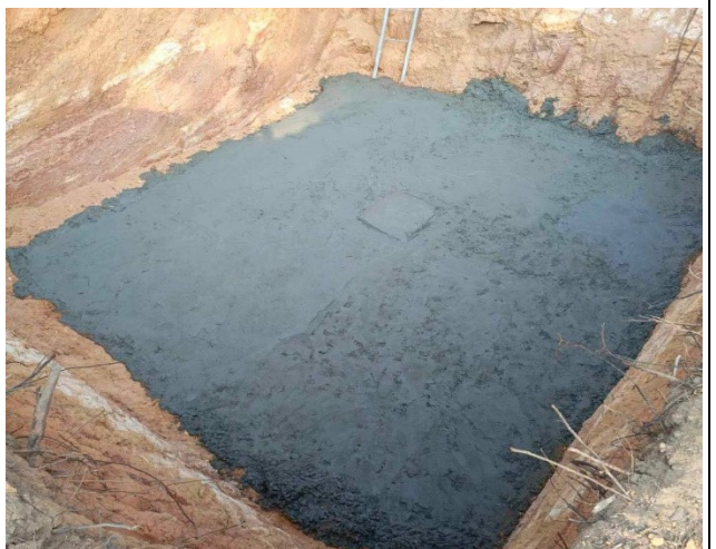
Casting concrete lean.
