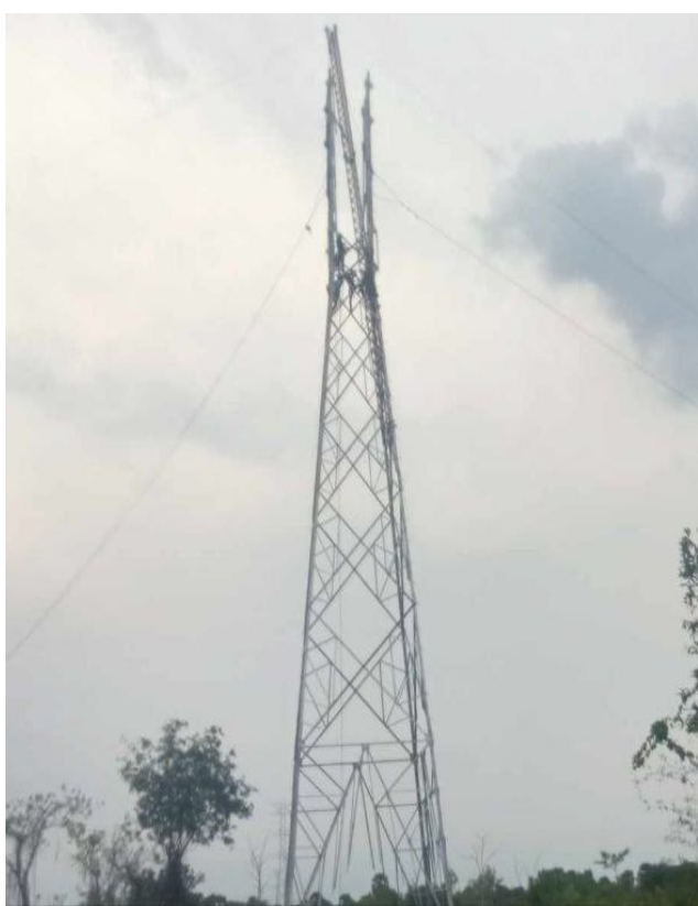
TA076 Tower erection .
