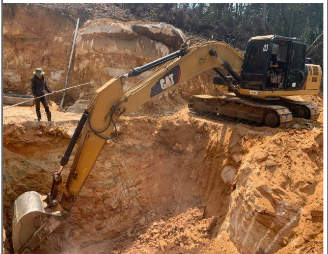
Soil excavatoin of the pit.
