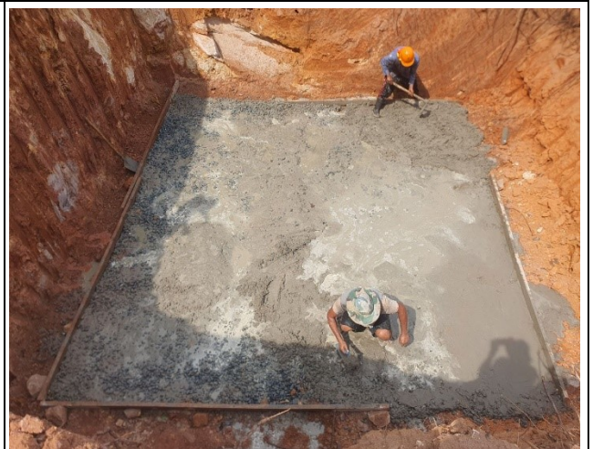
Casting concrete lean
