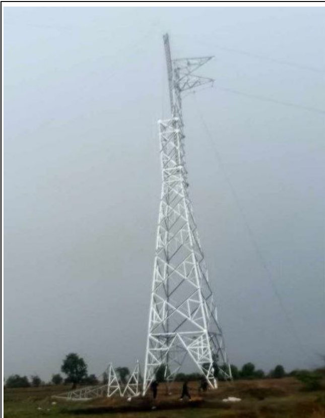
TA085 Tower erection .
