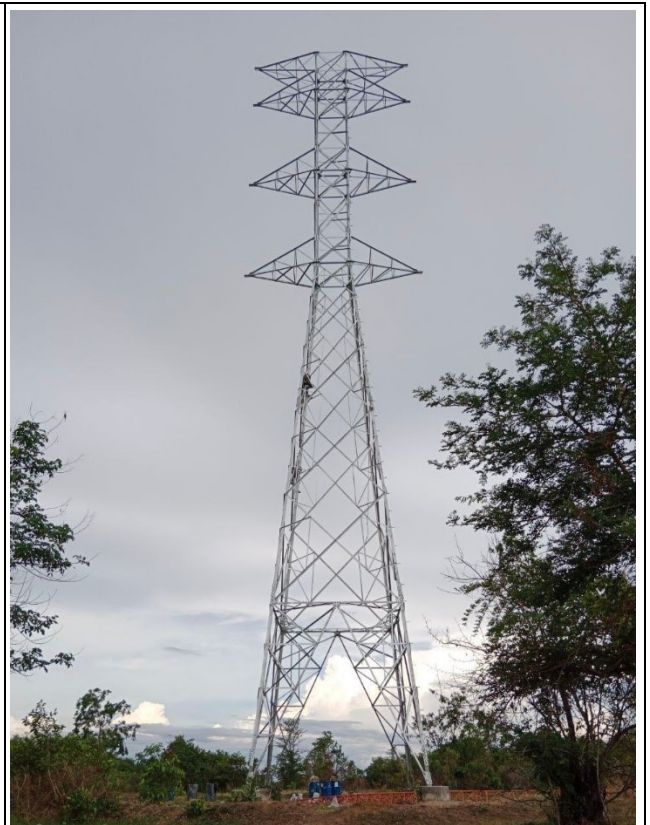
TA090 Tower erection completed .
