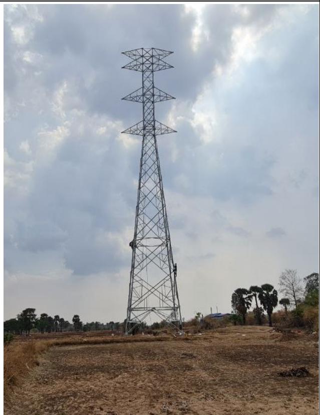
TA041 Erection completd.
