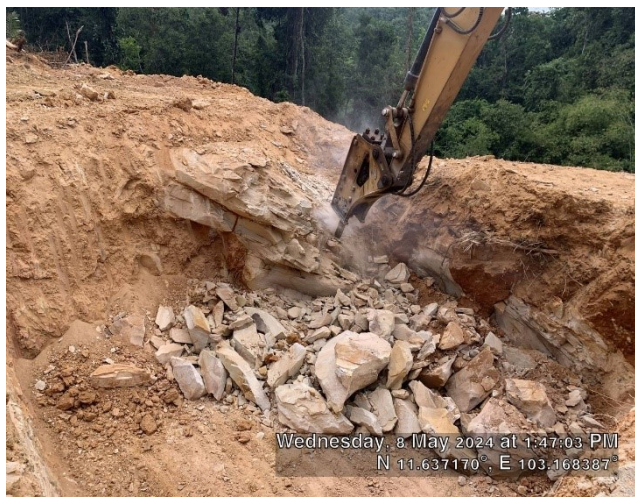
Breaking stone of the pit.
