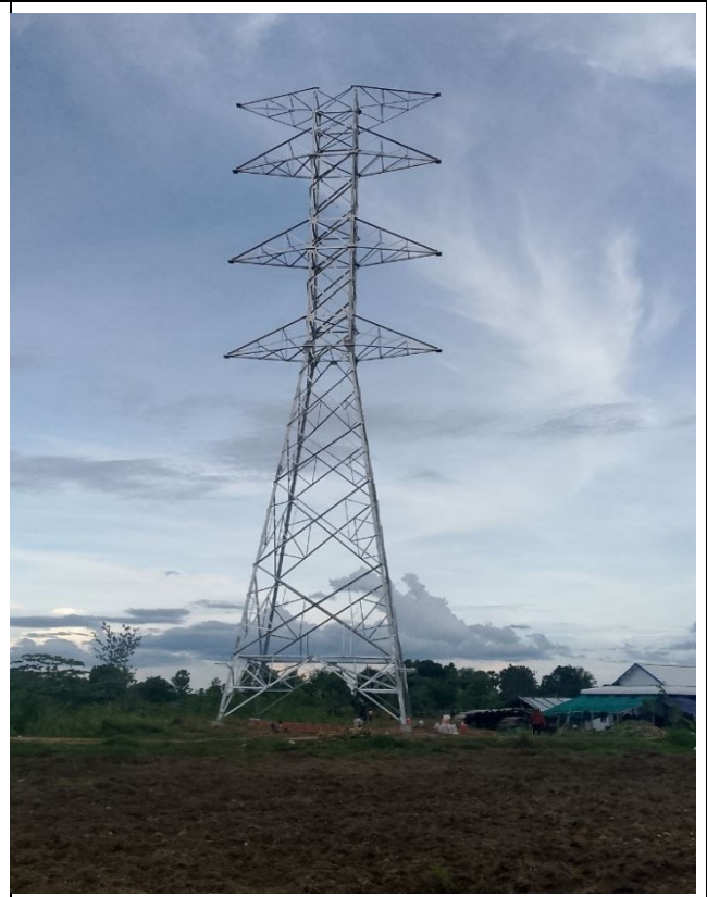
TA121 Tower erection completed .
