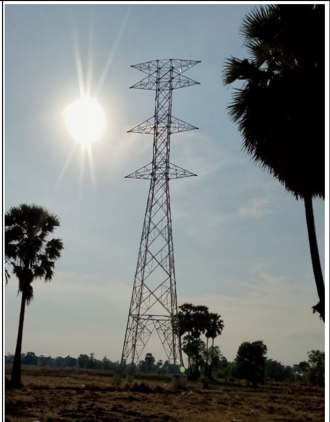
TA078 Tower erection completed .
