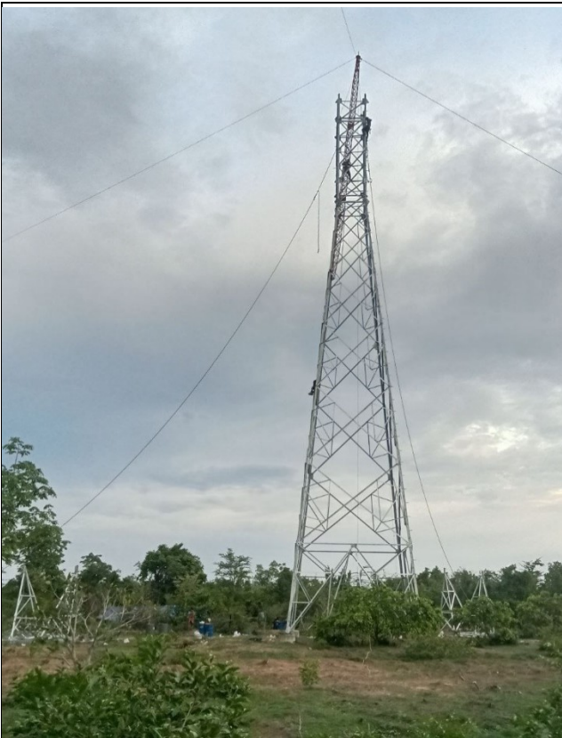
TA112 Tower erection .
