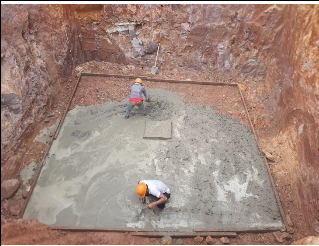
Casting concrete lean
