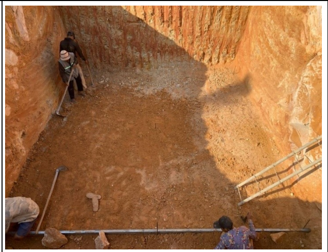
Soil excavatoin of the pit.
