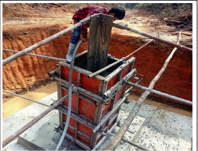
Concrete vibration.
