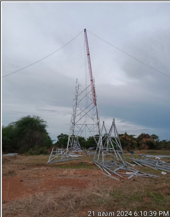
TA090 Tower erection .
