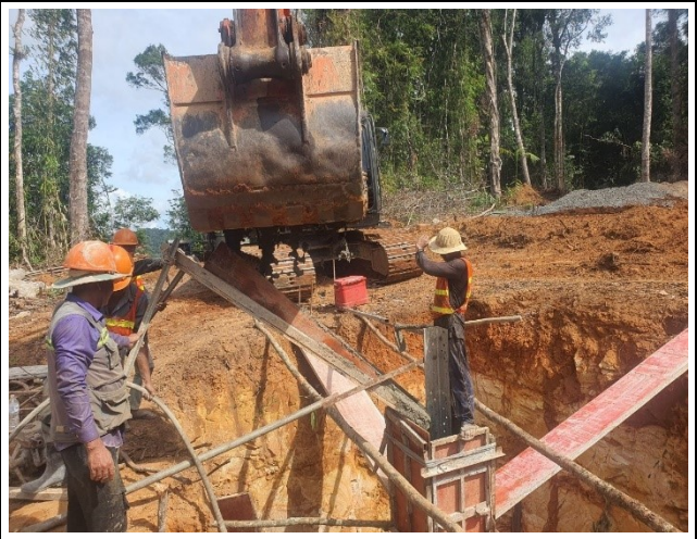
Casting concrete chimney
