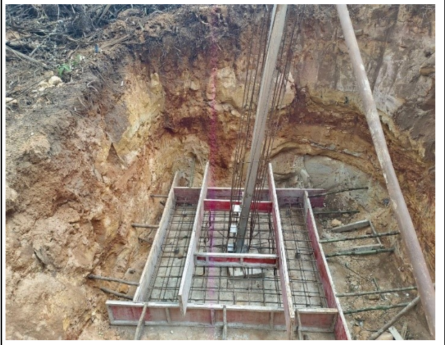
Install formworks
