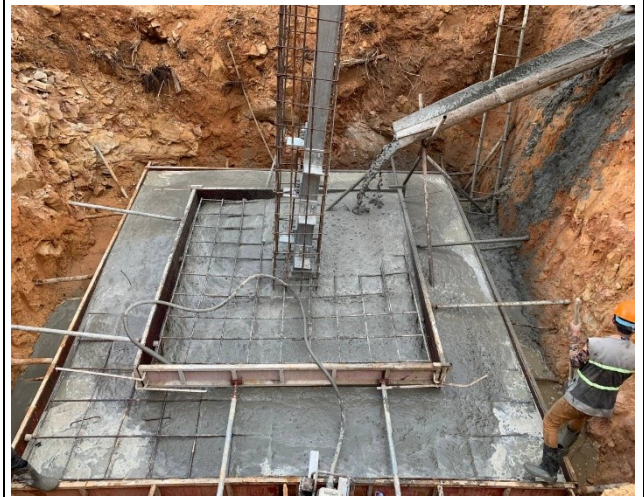
Casting concrete base .
