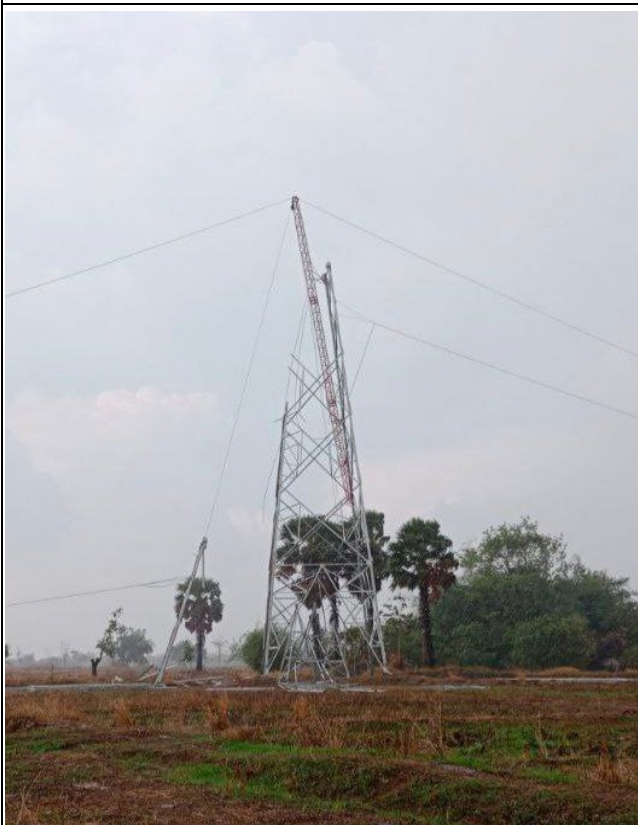
TA091 Tower erection .
