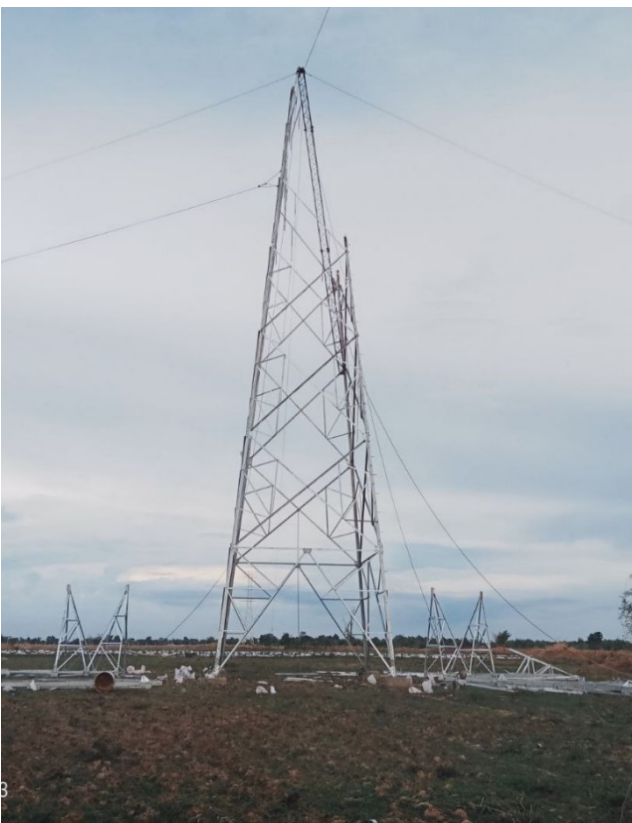
TA094 Tower erection .
