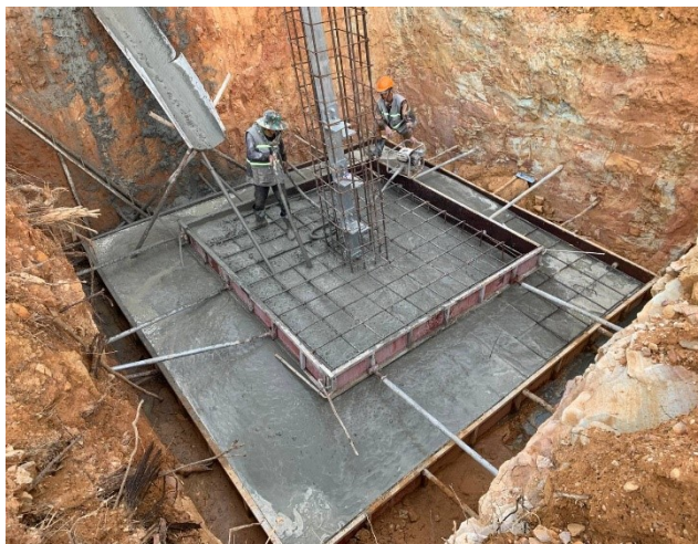
Concrete vibration of the base
