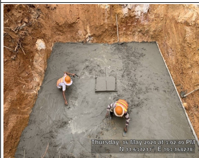
Casting concrete lean.
