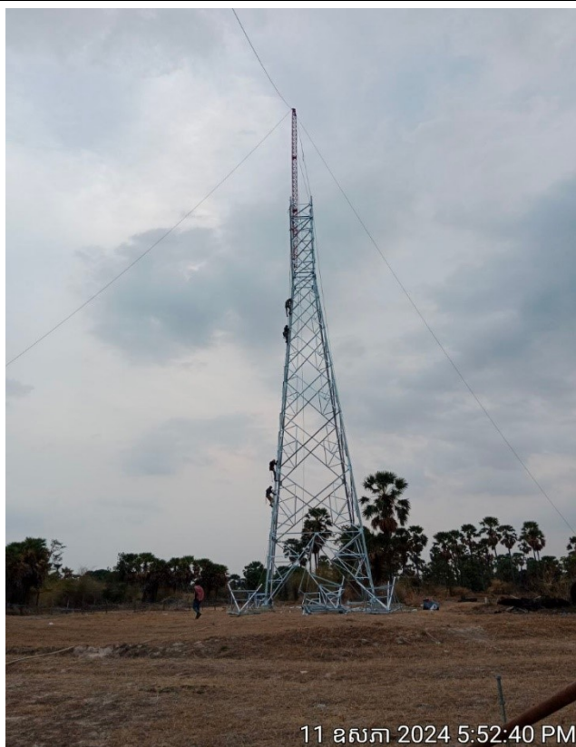
TA047 Tower erection .
