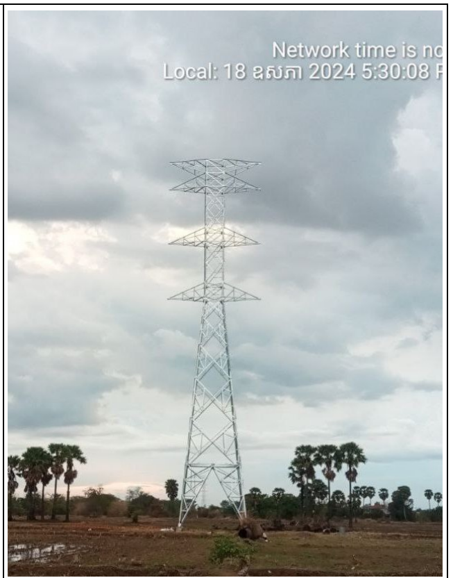
TA062 Tower erection completed.
