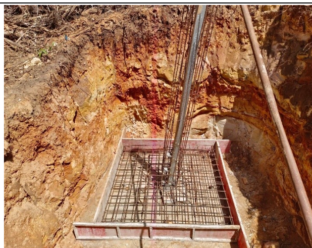
Install formworks
