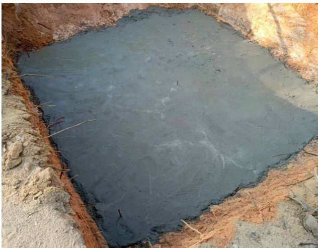
Casting concrete lean.
