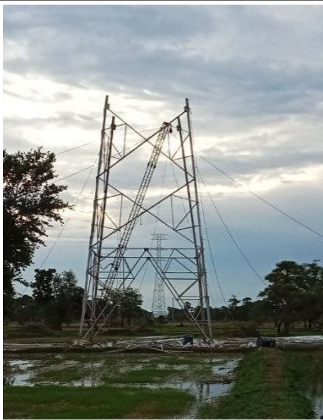
TA068 Tower erection .
