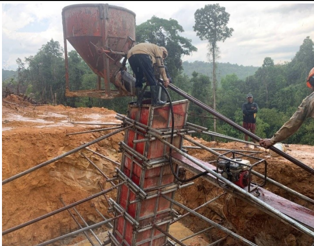
Concrete vibration.
