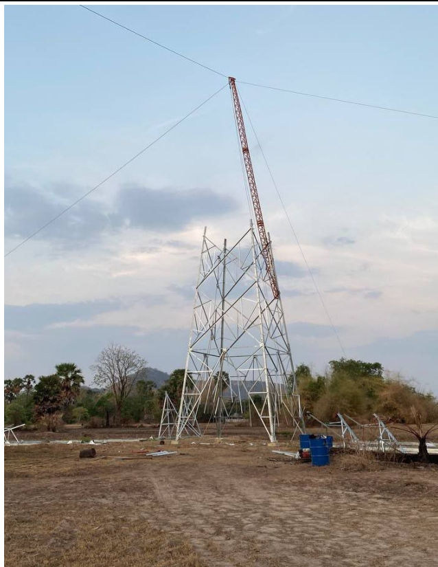
TA054 Tower erection .
