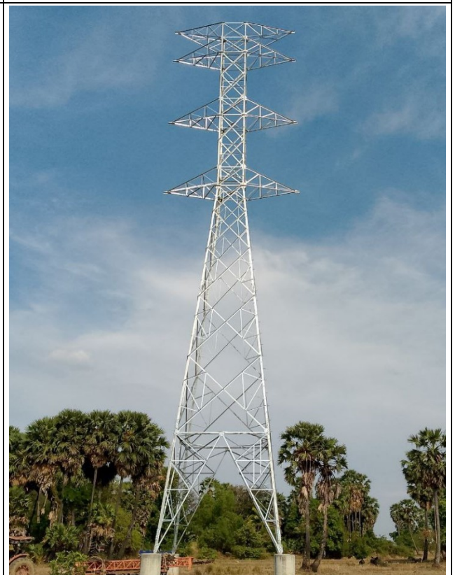
TA077 Tower erection completed .
