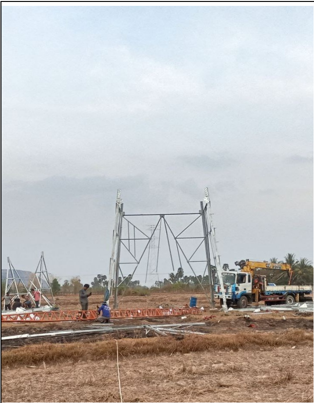
TA058 Tower erection .
