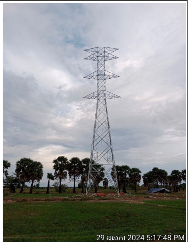
TA102 Tower erection completed .
