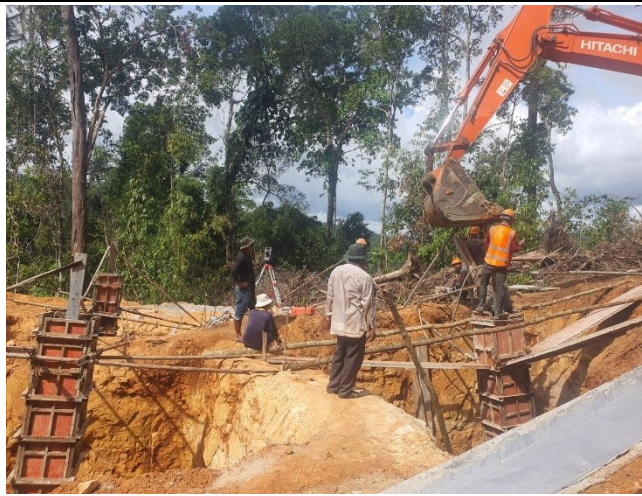
Casting concrete chimney
