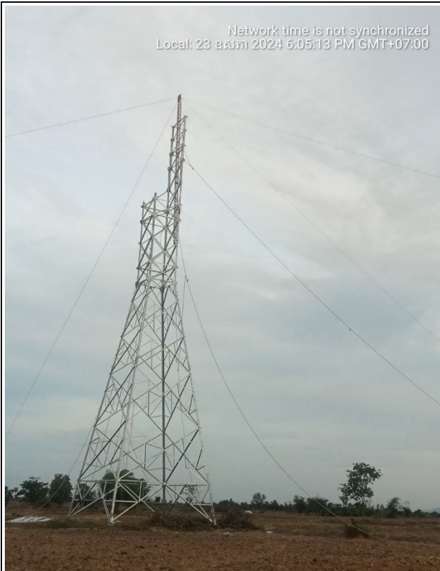
TA088 Tower erection .
