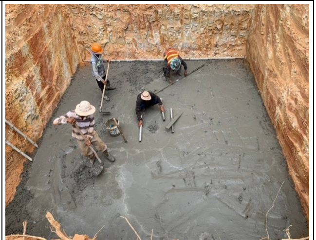
Casting concrete lean.
