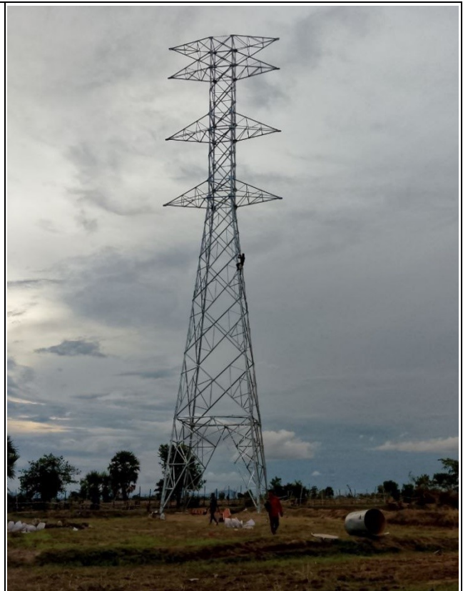
TA082 Tower erection completed .
