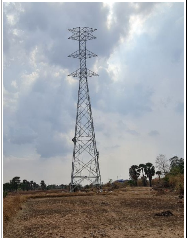
TA038 Erection completd.
