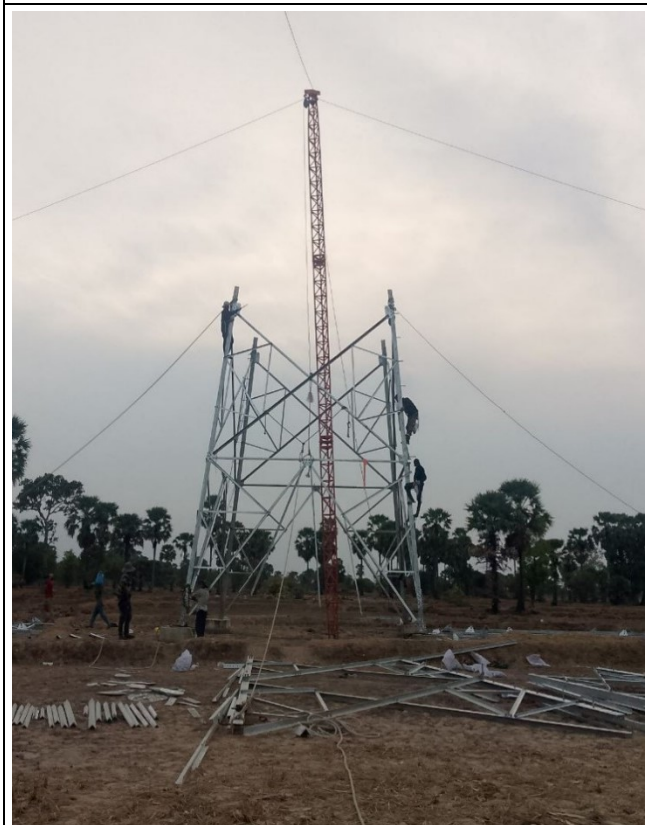
TA073 Tower erection .
