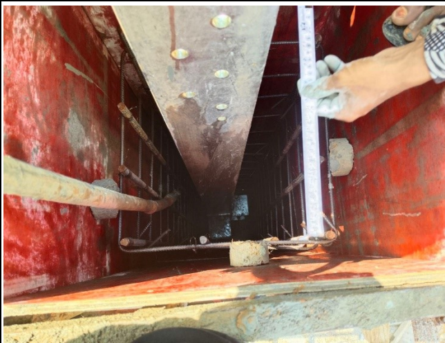
Install rebar , formwork & cleaning
