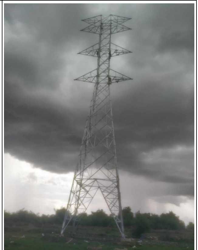
TA097 Tower erection completed .
