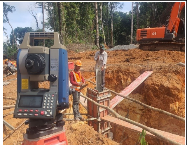
Casting concrete chimney
