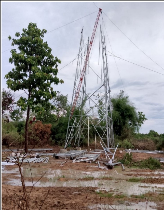
TA102 Tower erection .
