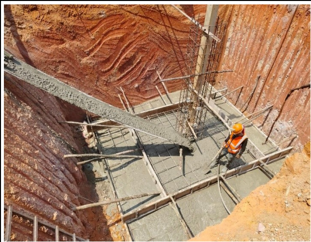
Concrete vibration
