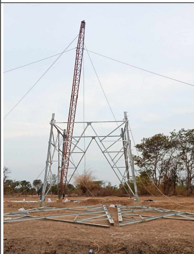
TA064 Tower erection .
