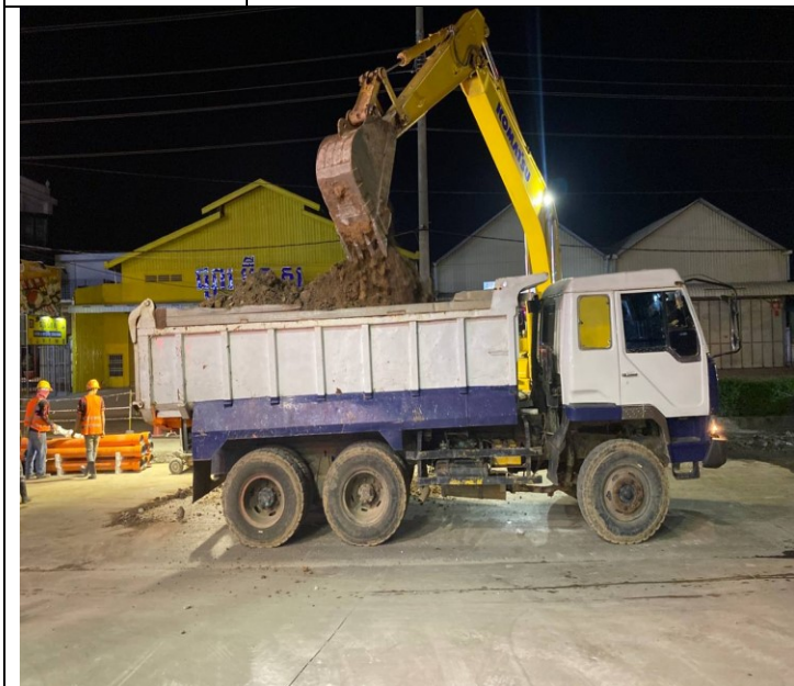
Photo: 03 Soil excavation and concrete road
