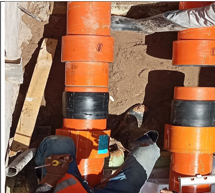
Photo: 19 Assembly PFP pipes and OFC pipe
