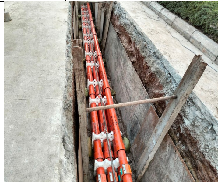
Photo: 03 Assembly PFP pipes and OFC pipe
