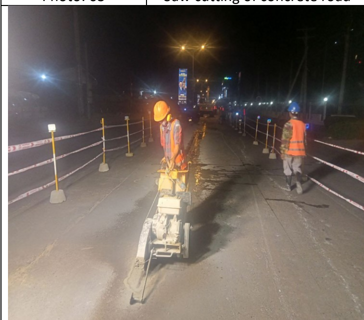
Photo: 05 Saw cutting of concrete road
