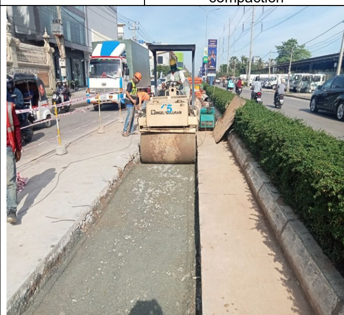
Base course backfilling and compaction
