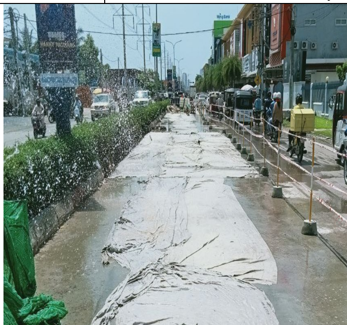
Photo: 24 Manhole of concrete road activity
