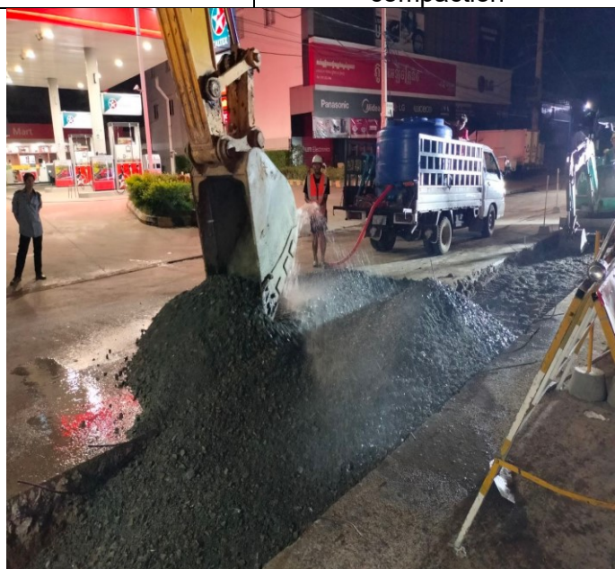
Base course backfilling and compaction
