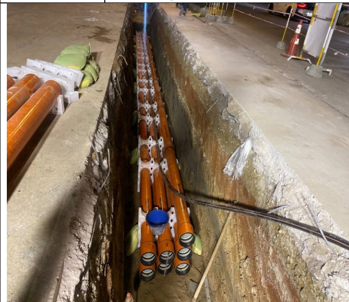
Photo: 05 Assembly PFP pipes and OFC pipe
