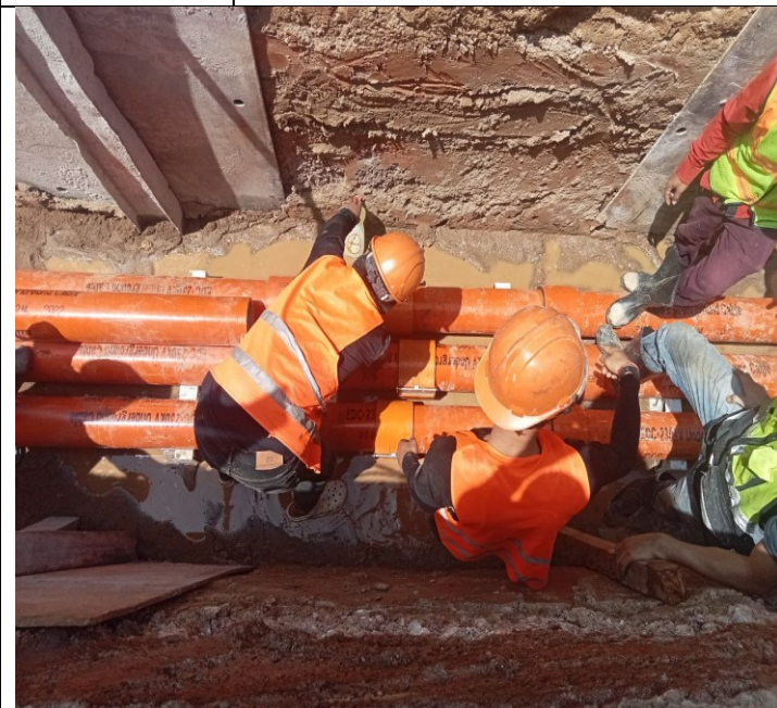
Photo: 09 Assembly PFP pipes and OFC pipe
