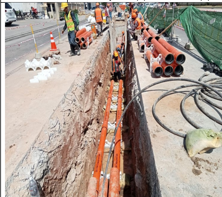
Photo: 17 Assembly PFP pipes and OFC pipe
