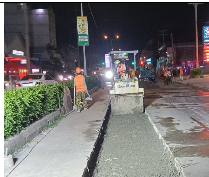
Base course backfilling and compaction
