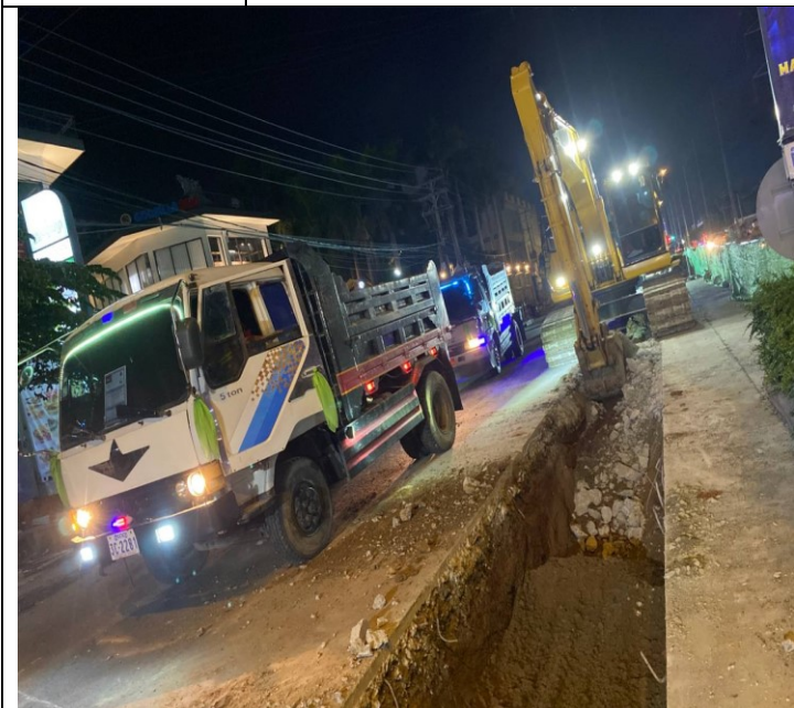
Photo: 09 Soil excavation and concrete road
