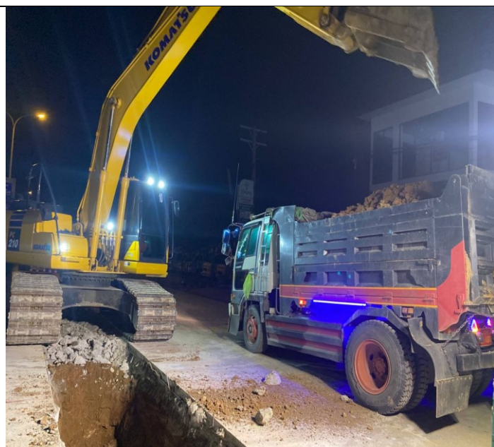
Photo: 08 Soil excavation and concrete road
