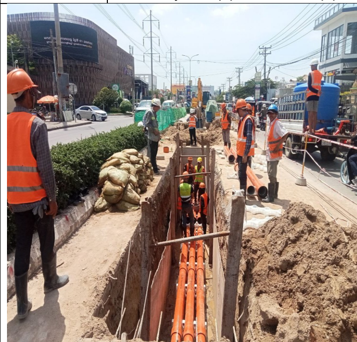
Photo: 11 Assembly PFP pipes and OFC pipe
