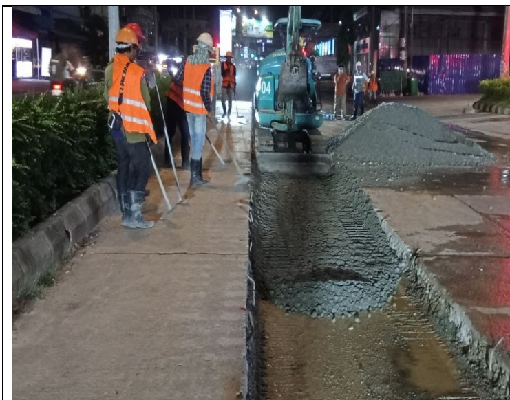
Base course backfilling and compaction
