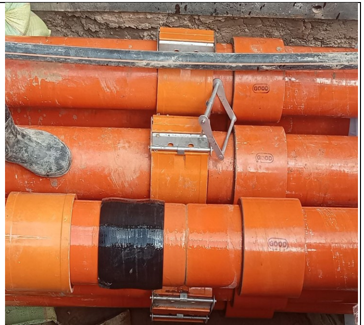
Photo: 20 Assembly PFP pipes and OFC pipe
