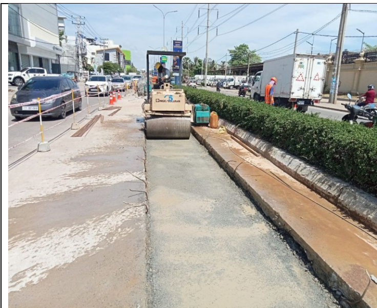
Base course backfilling and compaction
