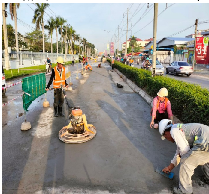
Photo: 18 Manhole of concrete road activity
