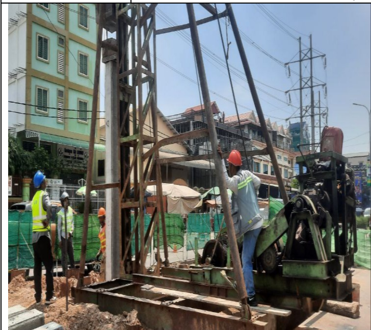
Photo: 05 Concrete Pile Installation activity
