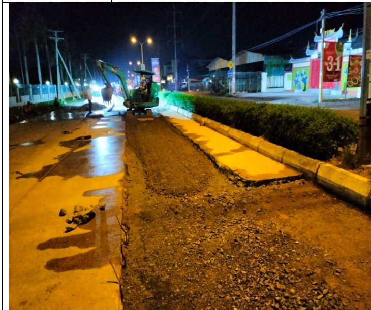
Photo: 03 Manhole of concrete road activity
