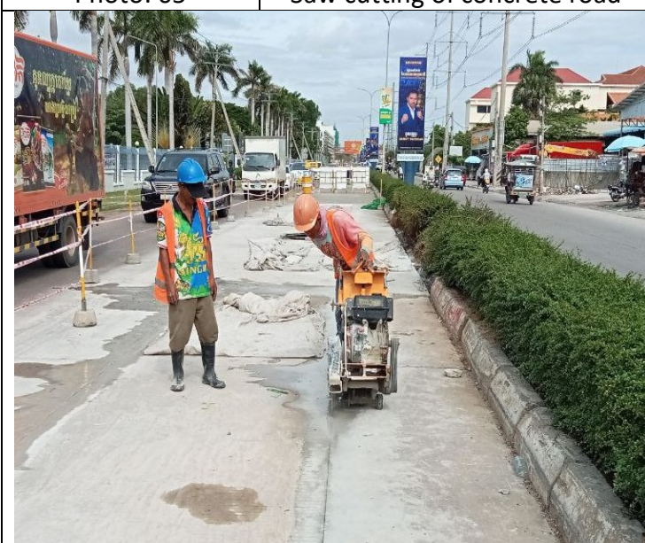
Photo: 07 Saw cutting of concrete road
