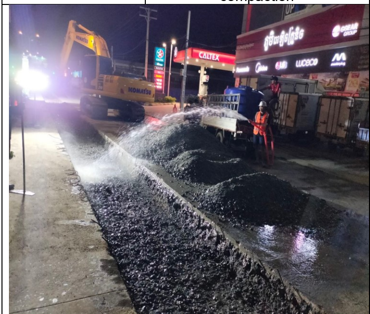
Base course backfilling and compaction
