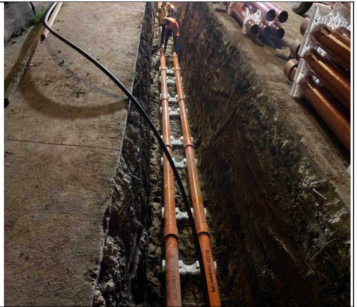
Photo: 02 Assembly PFP pipes and OFC pipe
