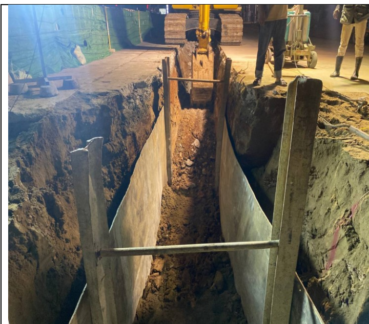
Photo: 07 Soil excavation and concrete road
