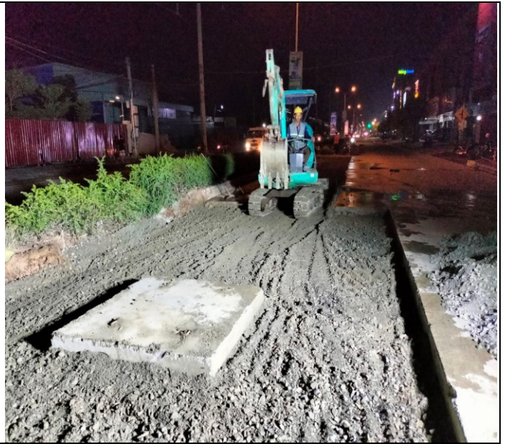
Photo: 02 Manhole of concrete road activity
