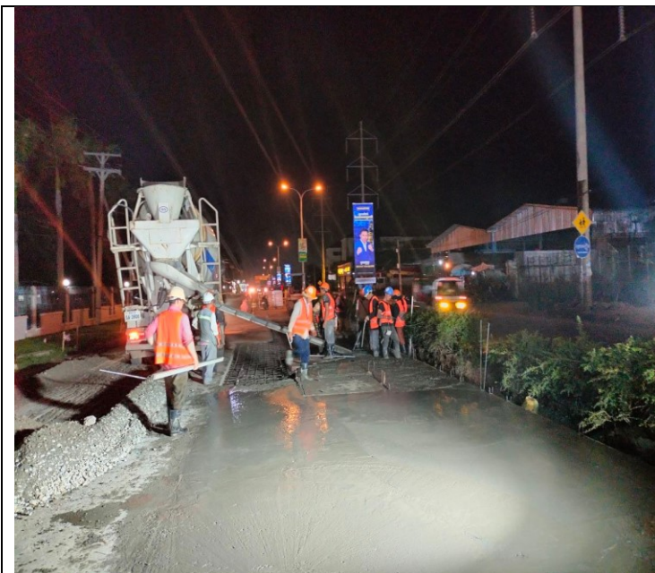
Photo: 13 Manhole of concrete road activity
