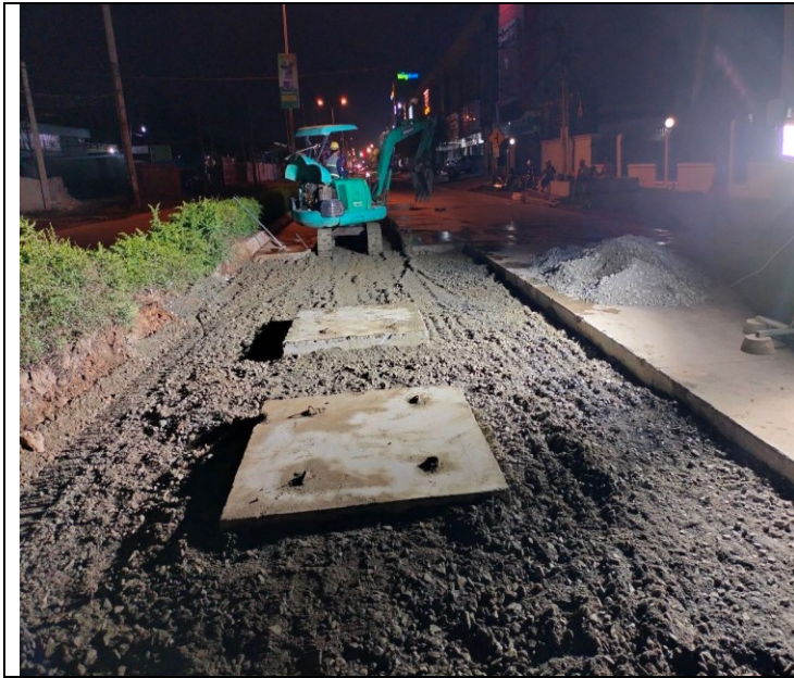
Photo: 01 Manhole of concrete road activity
