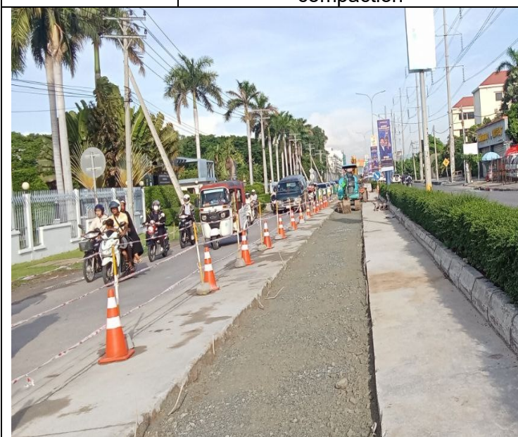
Base course backfilling and compaction
