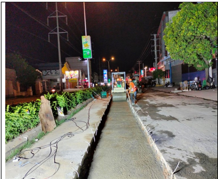
Base course backfilling and compaction
