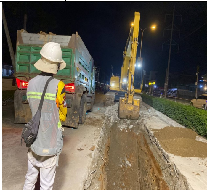
Photo: 10 Soil excavation and concrete road
