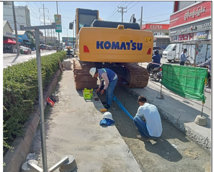
Plate test of compaction road
