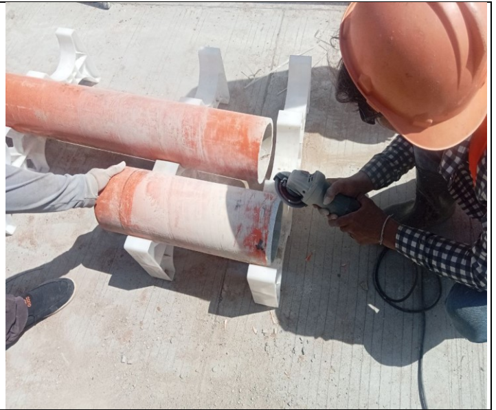
Photo: 08 Assembly PFP pipes and OFC pipe
