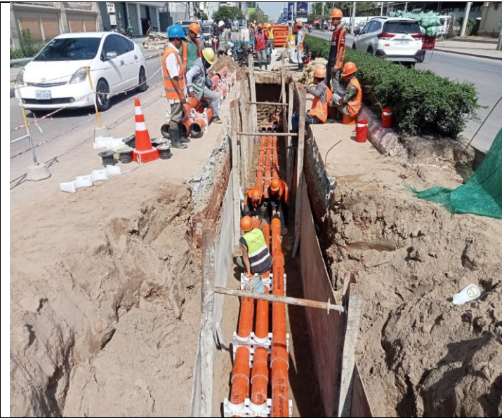
Photo: 07 Assembly PFP pipes and OFC pipe
