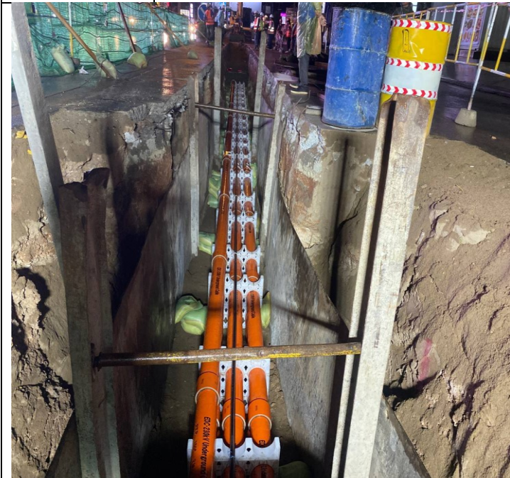
Photo: 23 Assembly PFP pipes and OFC pipe
