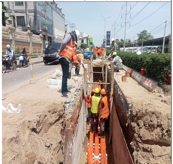
Photo: 12 Assembly PFP pipes and OFC pipe
