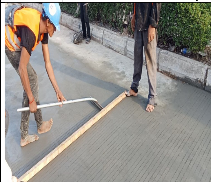
Photo: 21 Manhole of concrete road activity
