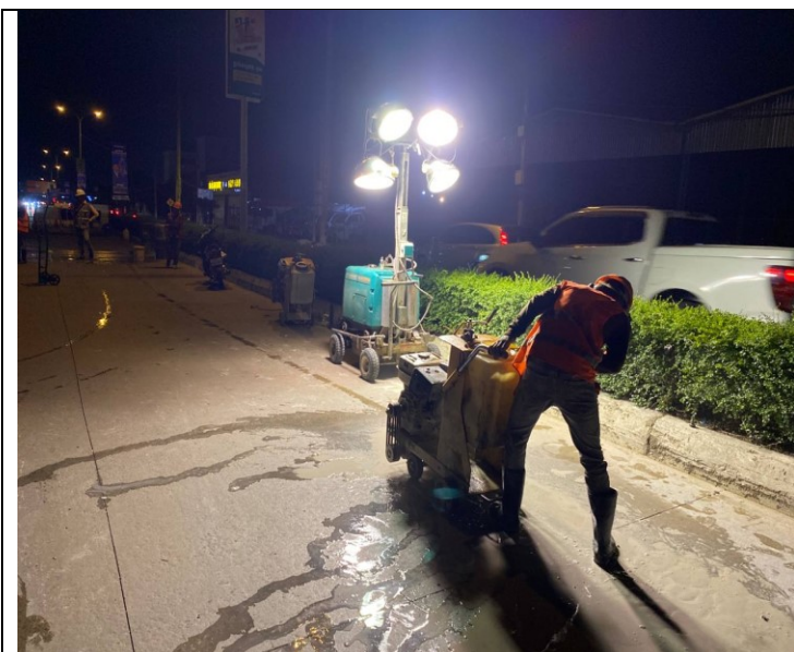
Photo: 03 Saw cutting of concrete road
