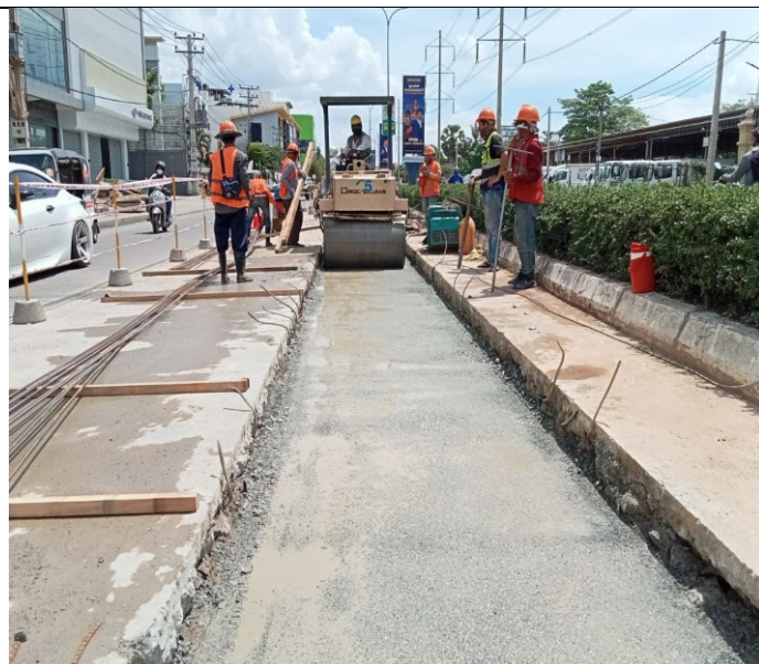
Base course backfilling and compaction
