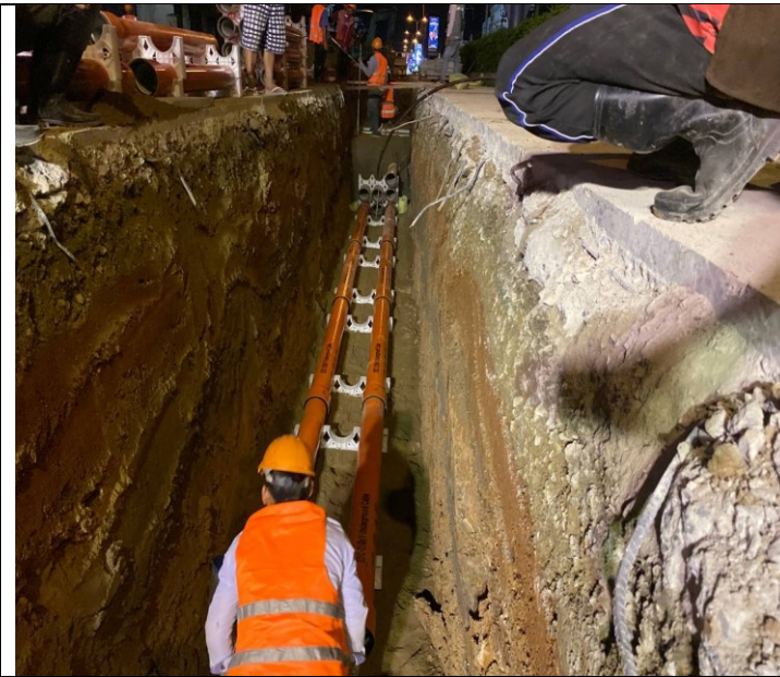
Photo: 01 Assembly PFP pipes and OFC pipe
