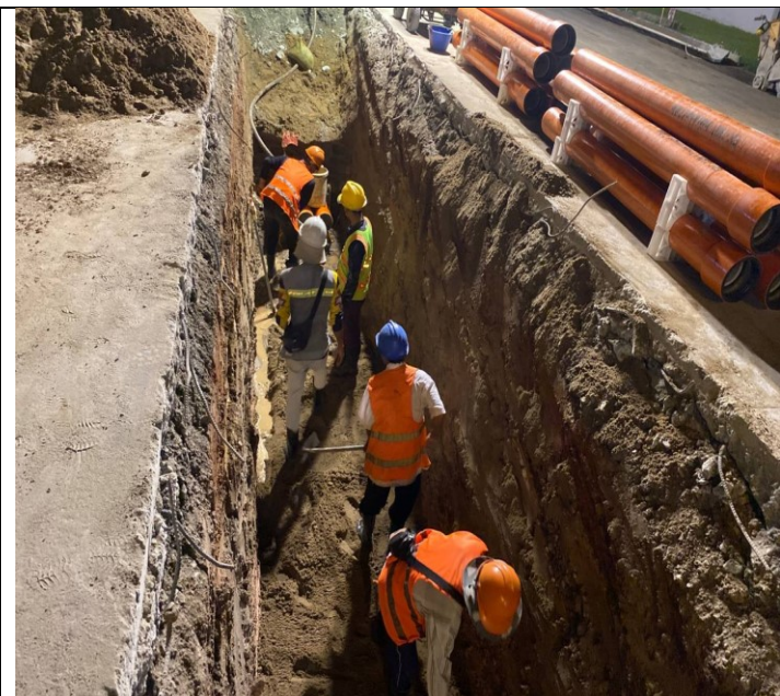
Photo: 25 Assembly PFP pipes and OFC pipe
