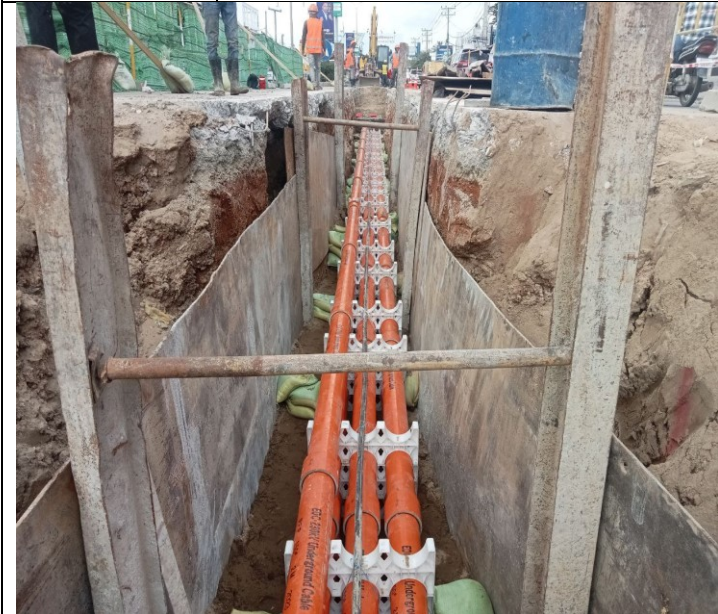
Photo: 21 Assembly PFP pipes and OFC pipe
