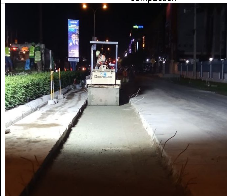
Base course backfilling and compaction
