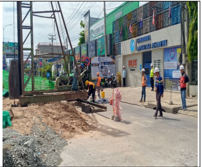
Photo: 02 Concrete Pile Installation activity
