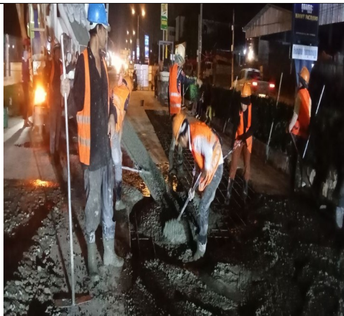
Photo: 14 Manhole of concrete road activity
