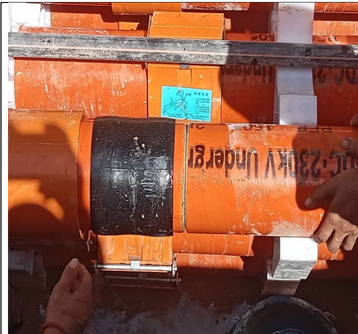
Photo: 13 Assembly PFP pipes and OFC pipe
