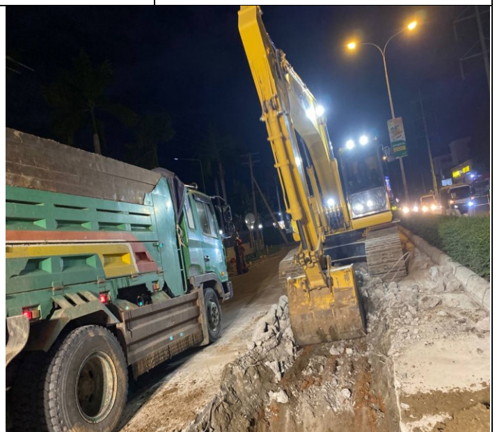
Photo: 06 Soil excavation and concrete road
