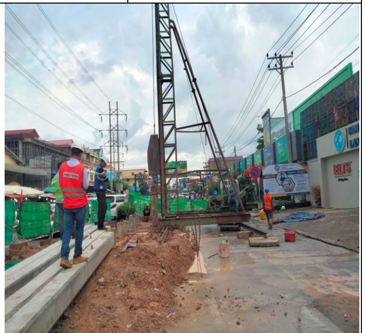
Photo: 06 Concrete Pile Installation activity
