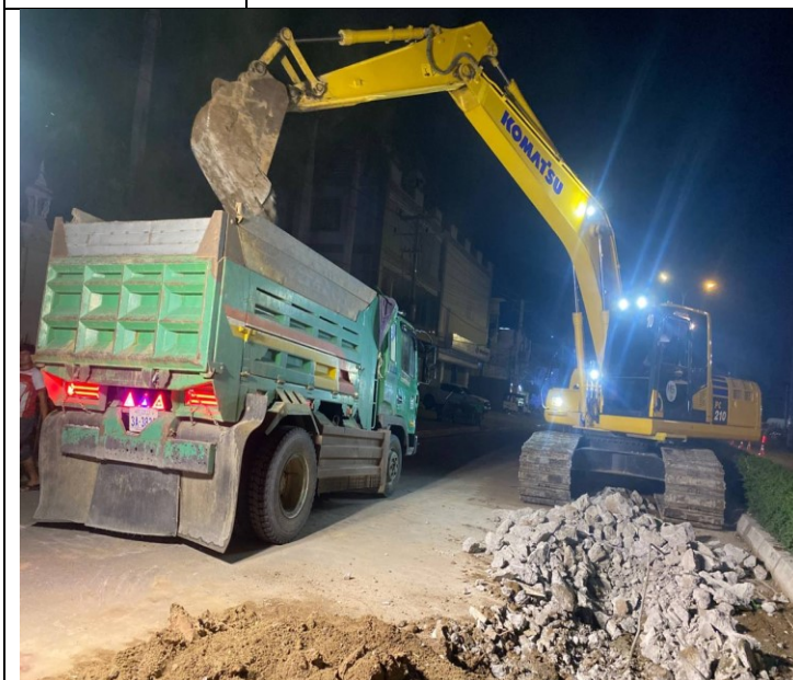
Photo: 05 Soil excavation and concrete road
