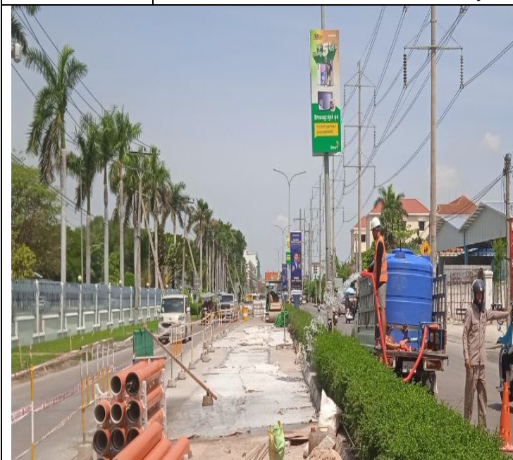
Photo: 23 Manhole of concrete road activity
