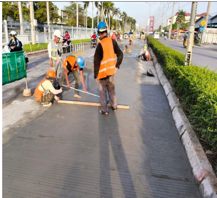
Photo: 20 Manhole of concrete road activity
