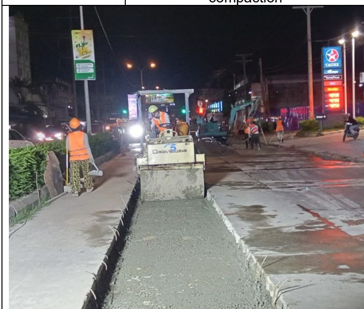
Base course backfilling and compaction
