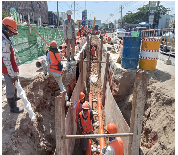
Photo: 16 Assembly PFP pipes and OFC pipe
