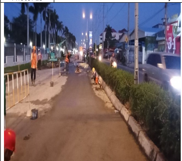
Photo: 17 Manhole of concrete road activity
