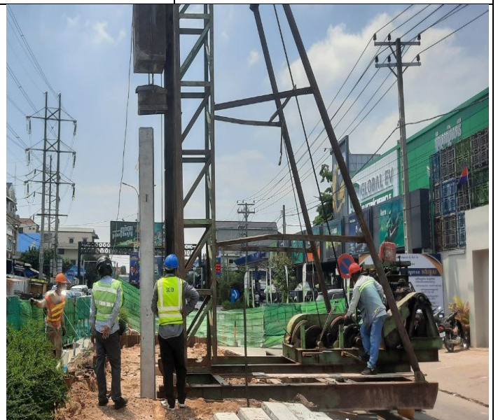
Photo: 04 Concrete Pile Installation activity
