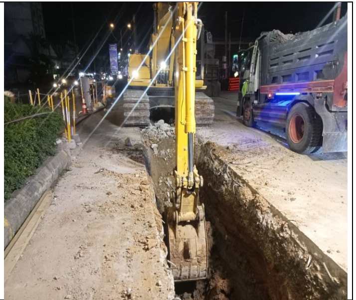
Photo: 02 Soil excavation and concrete road
