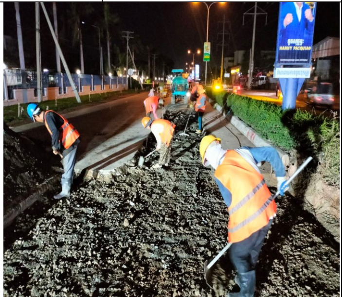
Photo: 04 Manhole of concrete road activity
