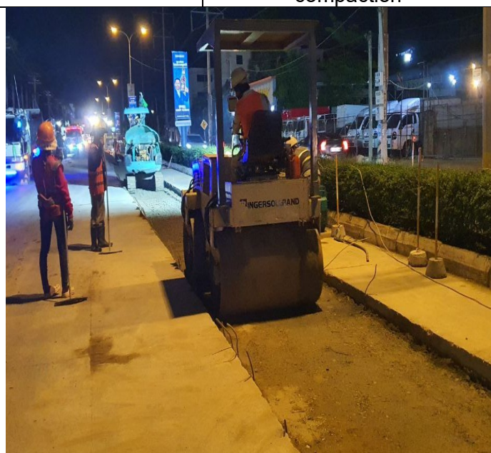
Base course backfilling and compaction
