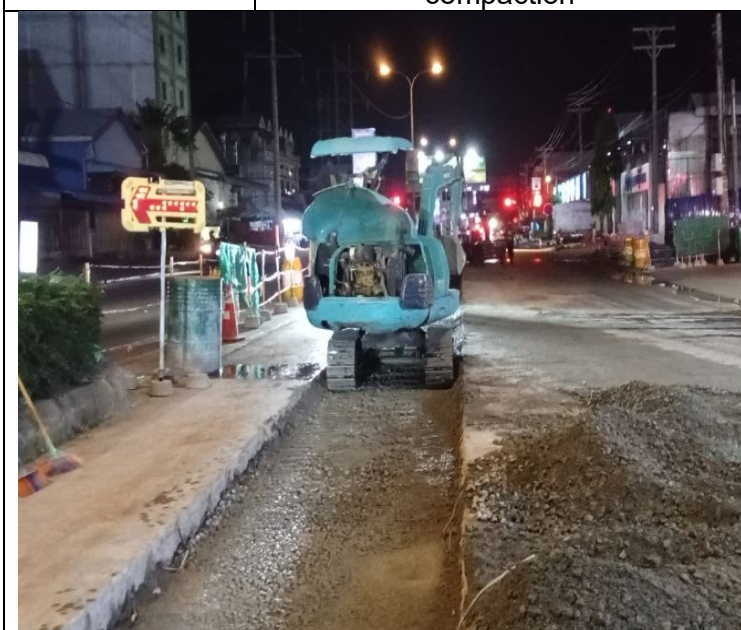
Base course backfilling and compaction
