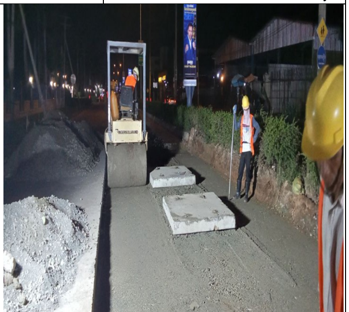
Photo: 06 Manhole of concrete road activity
