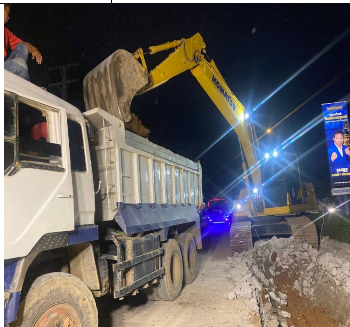
Photo: 12 Soil excavation and concrete road
