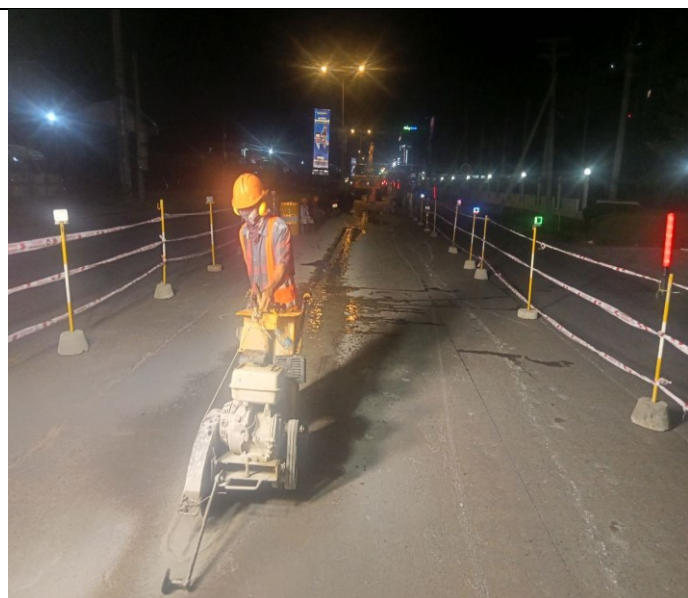
Photo: 04 Saw cutting of concrete road
