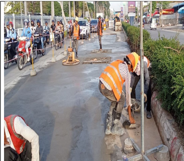
Photo: 19 Manhole of concrete road activity
