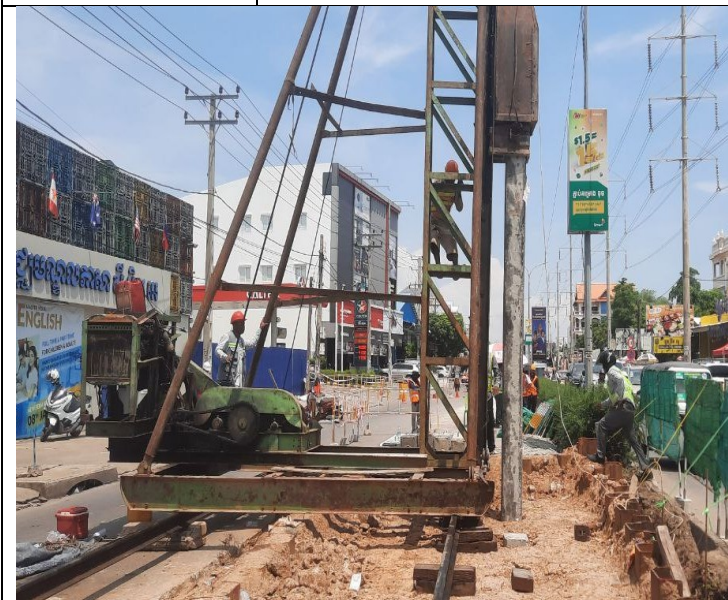
Photo: 03 Concrete Pile Installation activity
