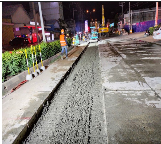
Base course backfilling and compaction
