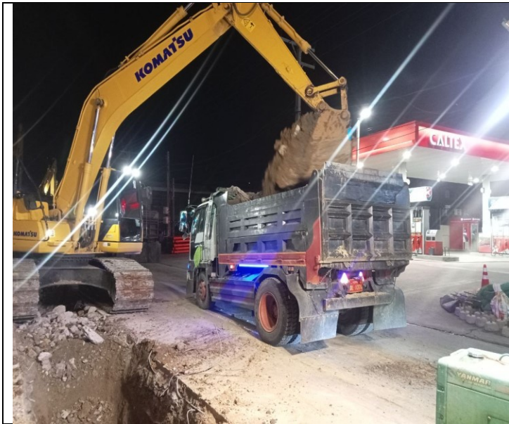
Photo: 01 Soil excavation and concrete road
