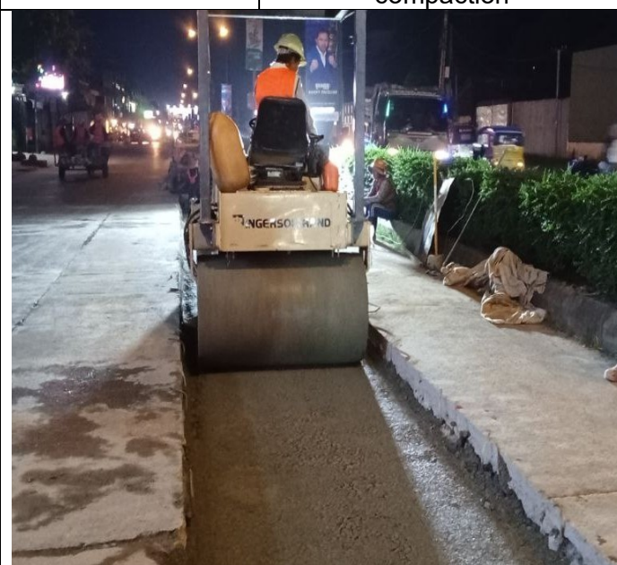
Base course backfilling and compaction
