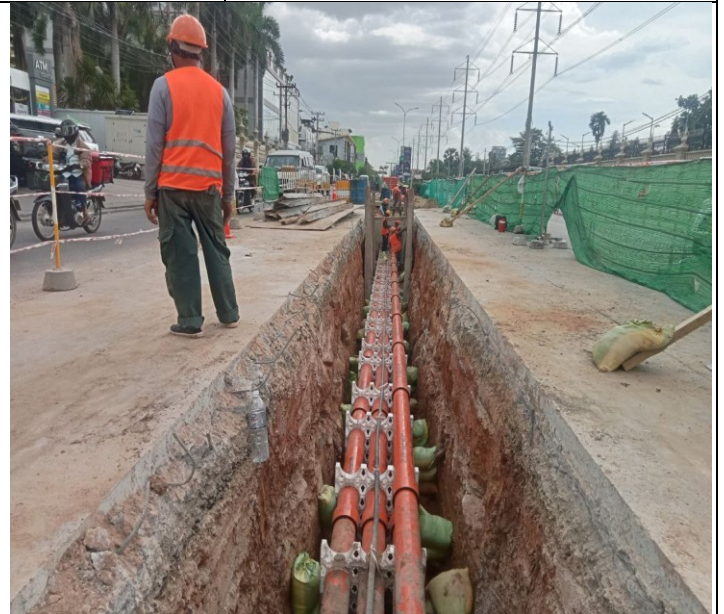
Photo: 22 Assembly PFP pipes and OFC pipe
