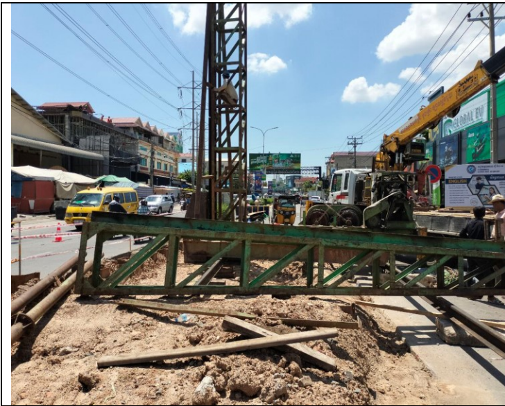
Photo: 01 Concrete Pile Installation activity
