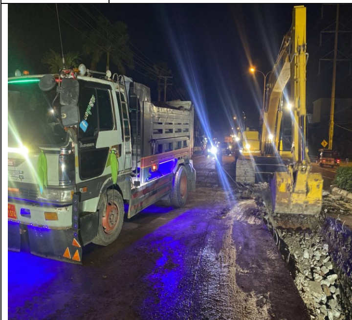
Photo: 11 Soil excavation and concrete road
