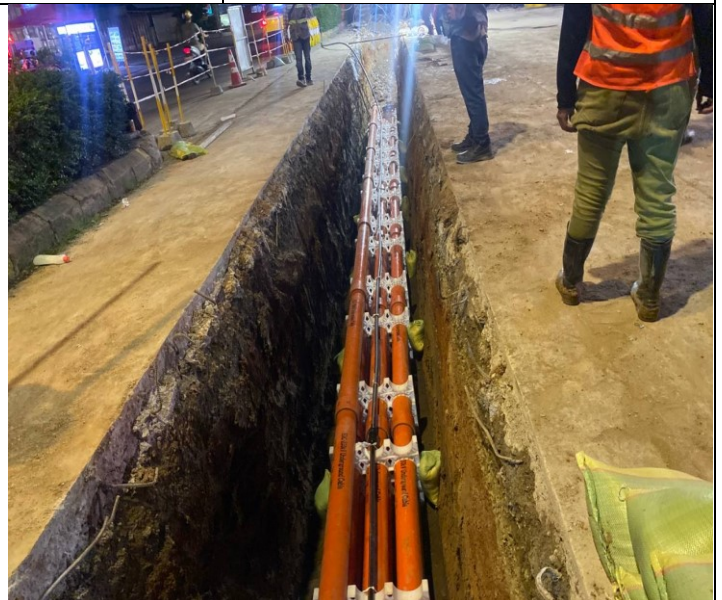
Photo: 04 Assembly PFP pipes and OFC pipe
