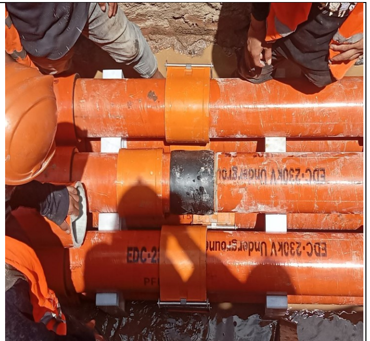
Photo: 14 Assembly PFP pipes and OFC pipe
