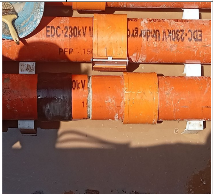
Photo: 10 Assembly PFP pipes and OFC pipe
