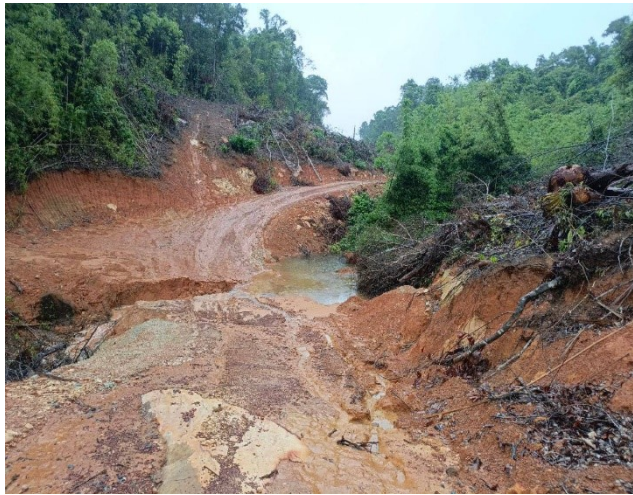
Access Road Work
