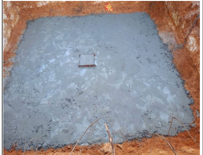
Casting concrete lean
