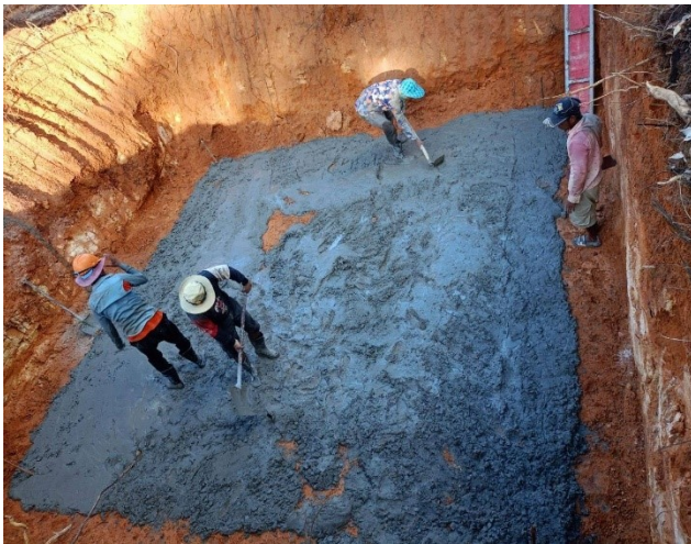
Casting concrete lean
