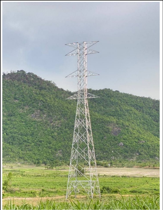
TA151 Erection completed.
