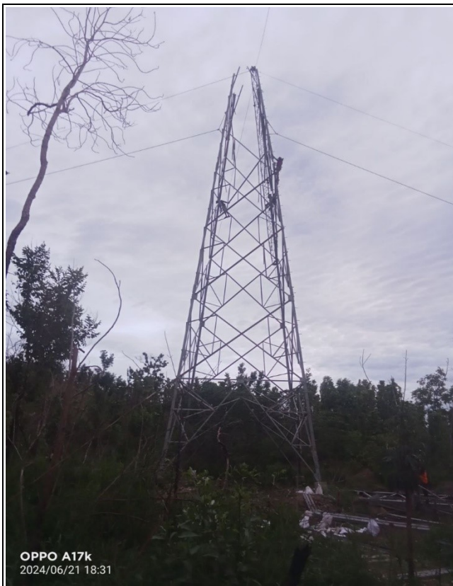
TA168 Tower erection
