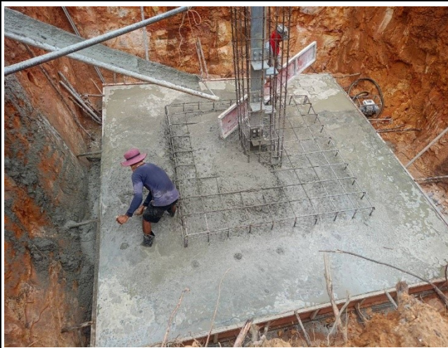
Casting concrete base .
