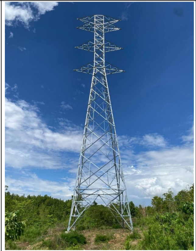
TA141 Erection completd.
