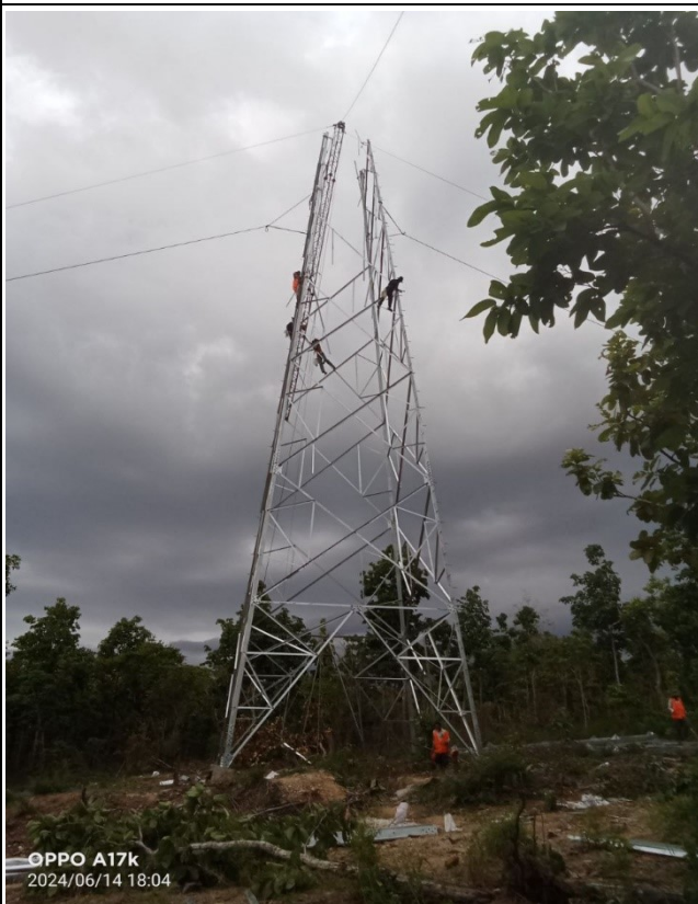
TA131 Tower erection.
