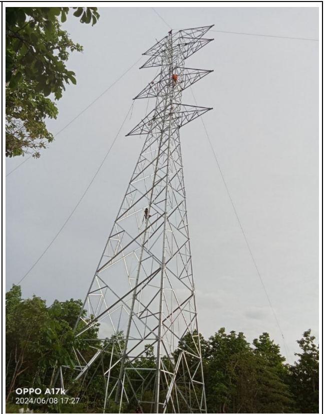
TA130 Erection completed.
