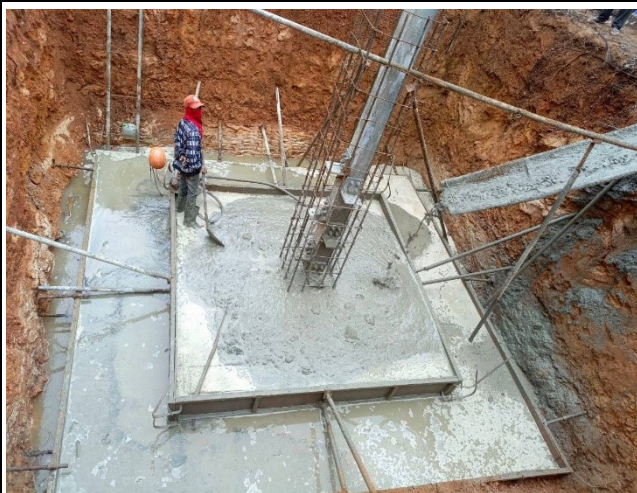
Casting concrete
