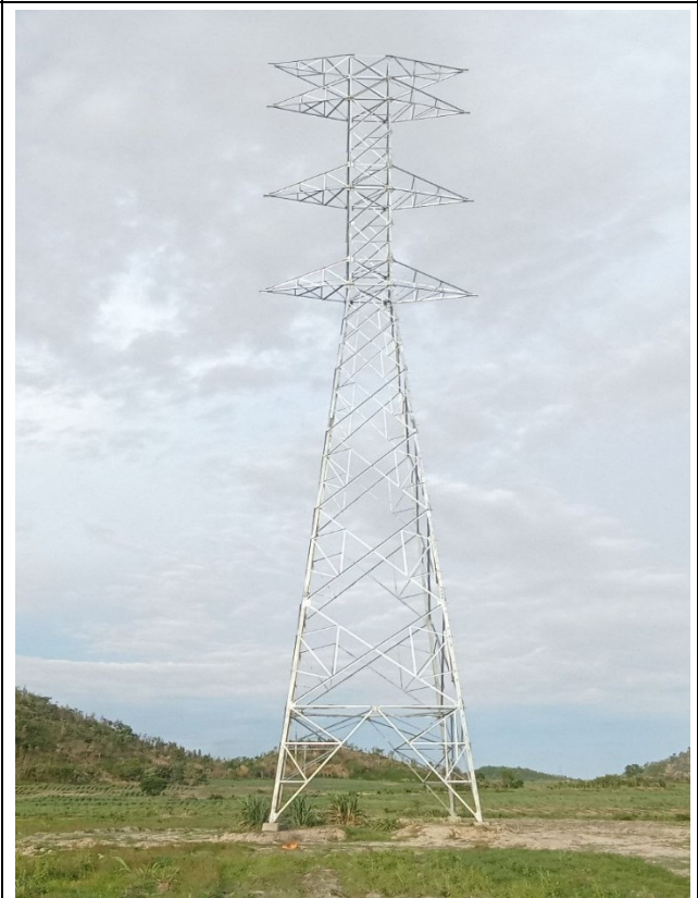
TA152 Erection completd.
