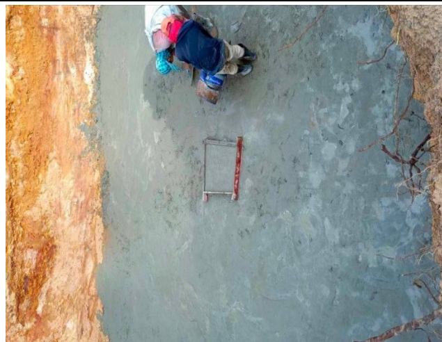
Casting concrete lean
