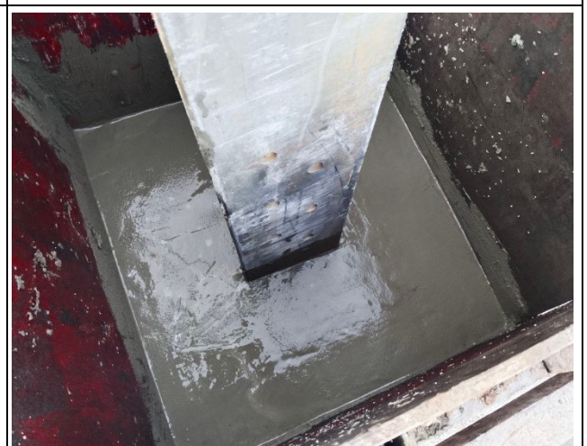
Casting concrete chimney .
