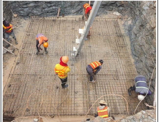
Rebar installation.
