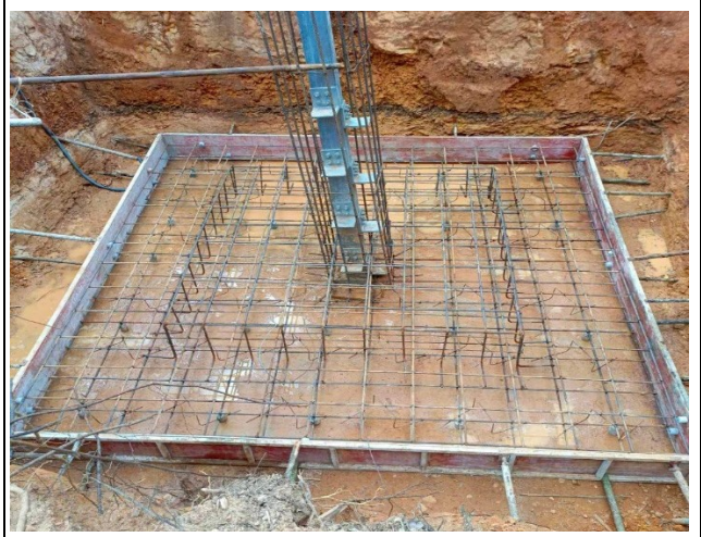
Installation rebar& formwork base.
