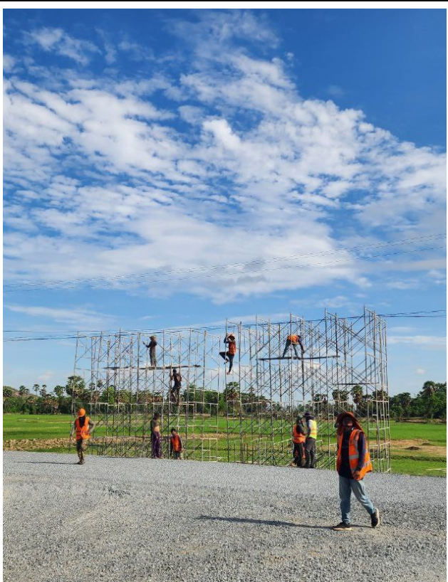
Installation scaffuding between T-A023, T-A024
