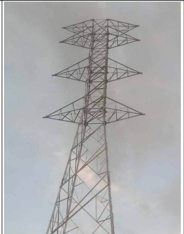
TA135 Erection completd.
