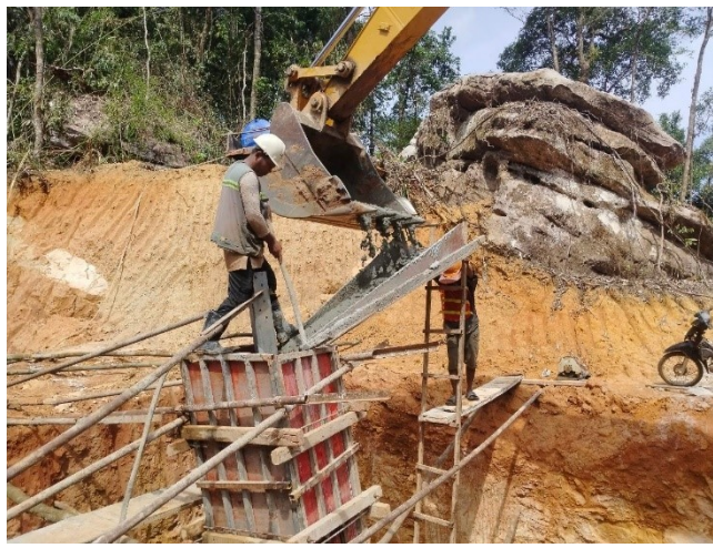
Casting concrete of the chimney.
