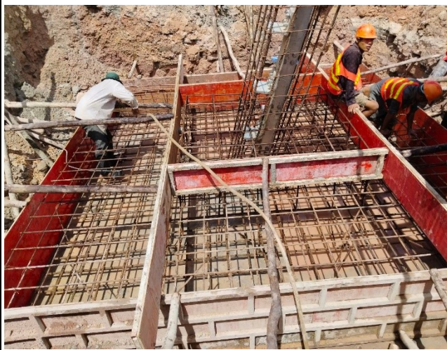
Formwork installation.
