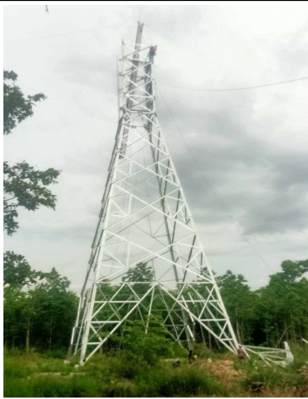
TA134 Tower erection.
