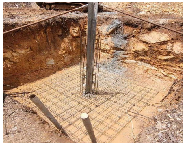
Installation rebar base .
