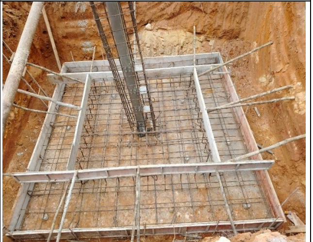
Install rebar and formworks
