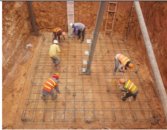
Arrengement rebar of the base .
