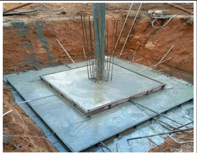
Casting concrete finish.
