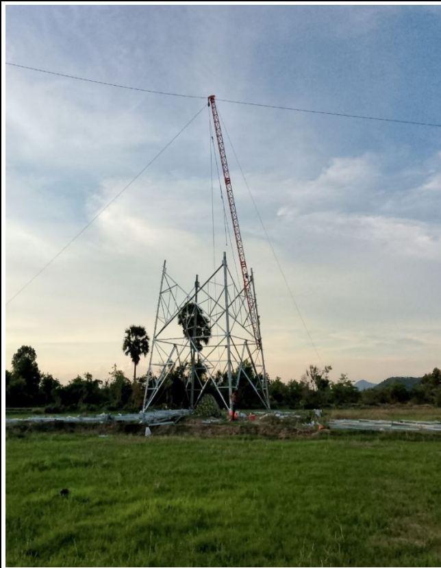
TA118 Tower erection.
