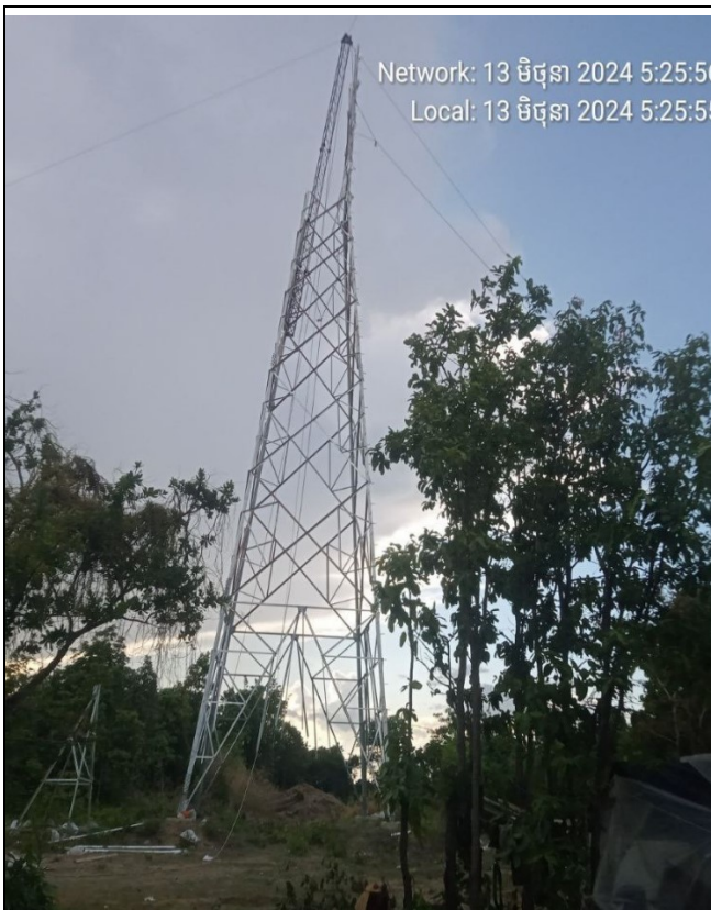
TA099 Tower erection
