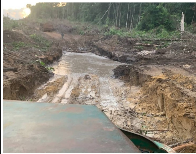
Access Road Work
