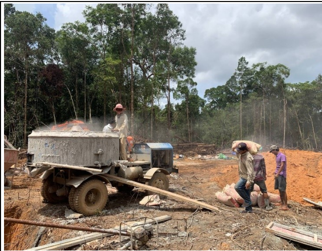
Concrete mixing for the chimney
