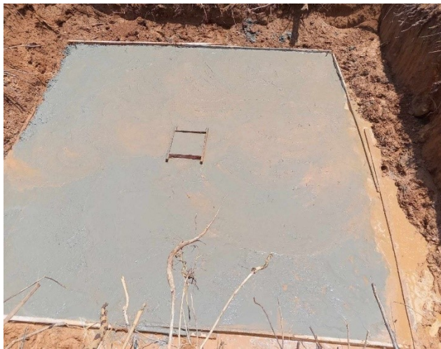
Casting concrete lean
