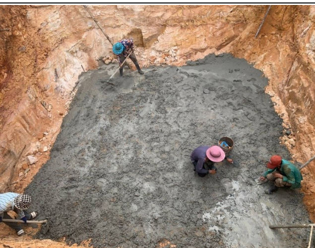
Casting concrete base.
