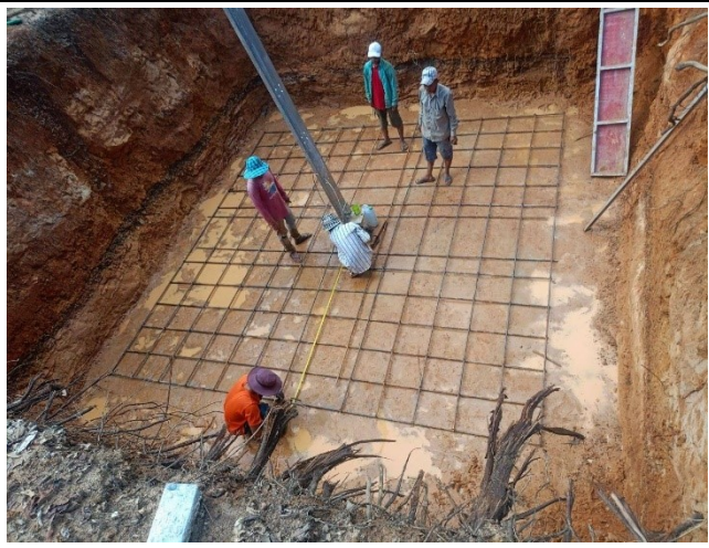
Installation rebar base .
