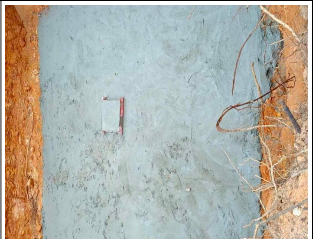
Casting concrete lean
