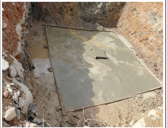
Casting concrete lean
