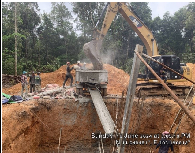
Concrete mixing .
