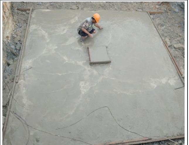
Casting concrete lean
