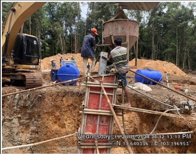
Casting concrete chimney .
