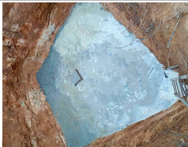
Casting concrete lean
