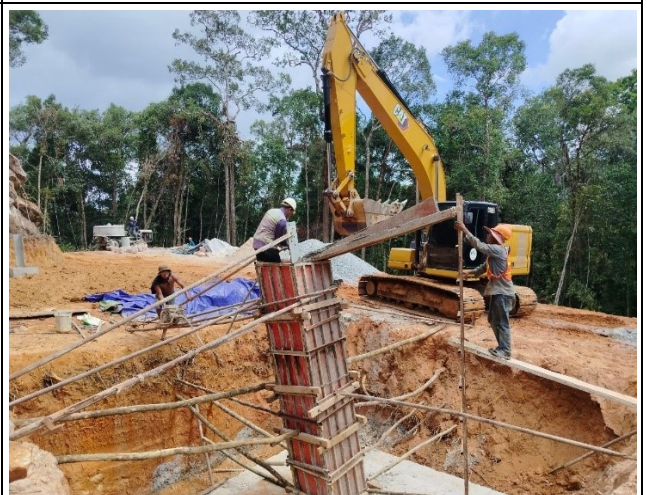
Preparation casting concrete
