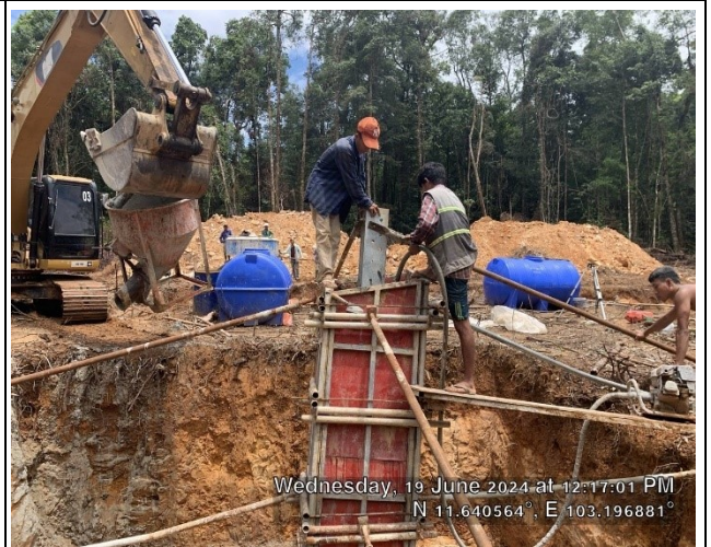
Concrete vibration.
