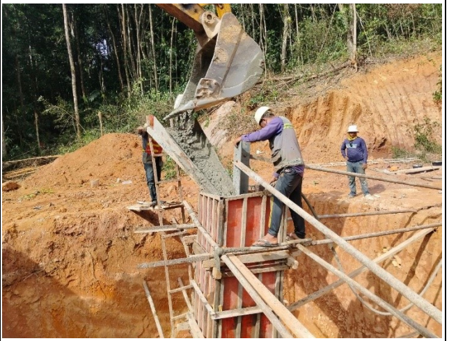
Casting concrete of the chimney.
