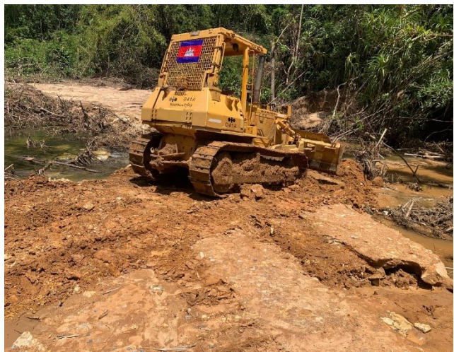
Access Road Work
