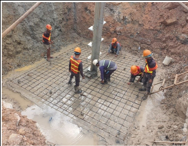
Rebar installation
