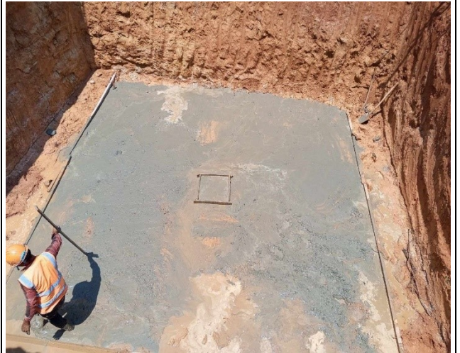
Casting concrete lean
