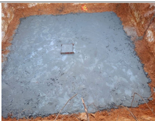
Casting concrete lean
