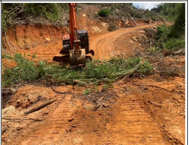
Access Road Work
