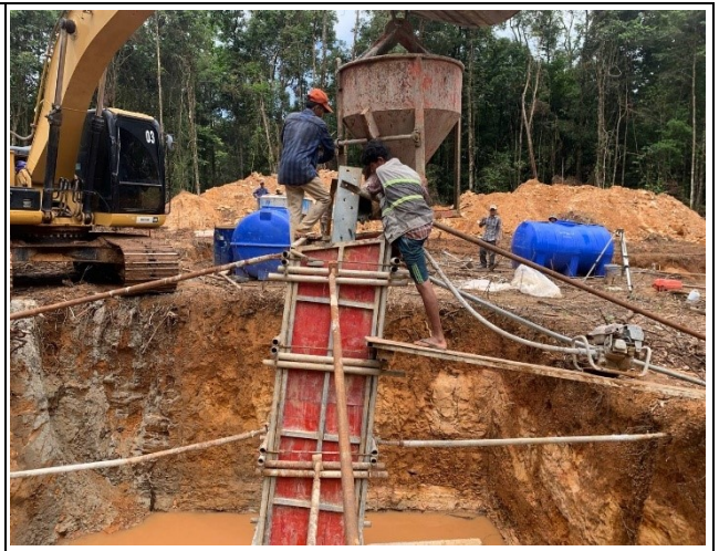
Casting concrete chimney.
