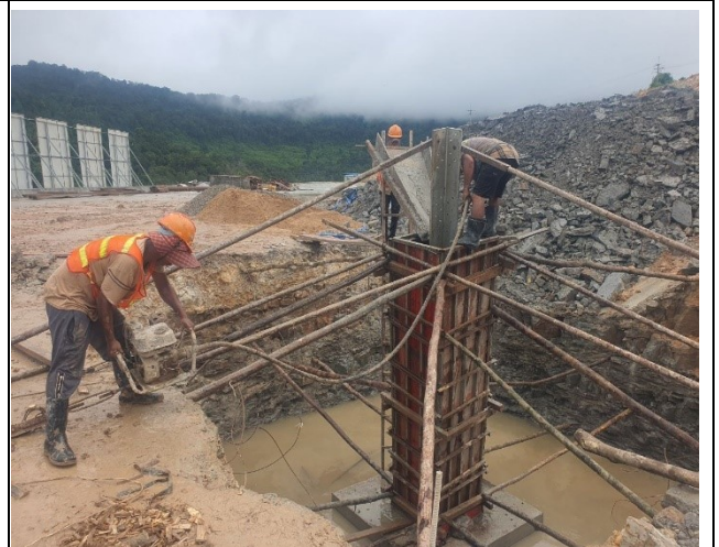
Concrete vibration.
