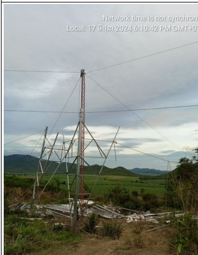
TA180 Tower erection
