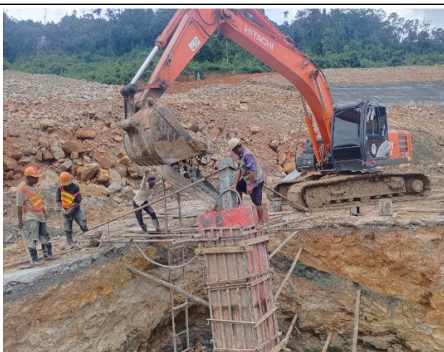
Casting concrete chimney .
