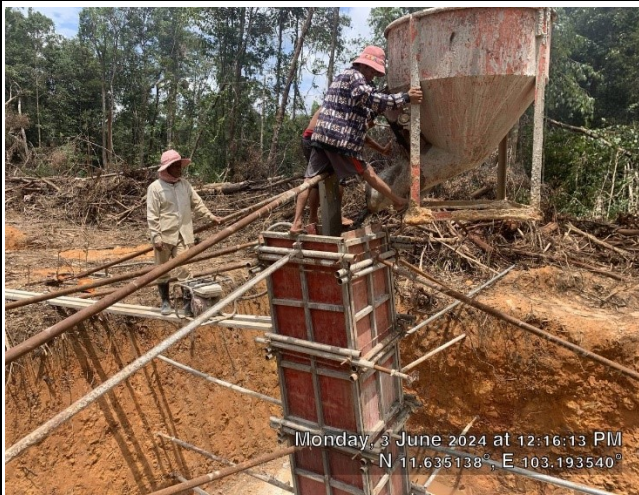
Casting concrete
