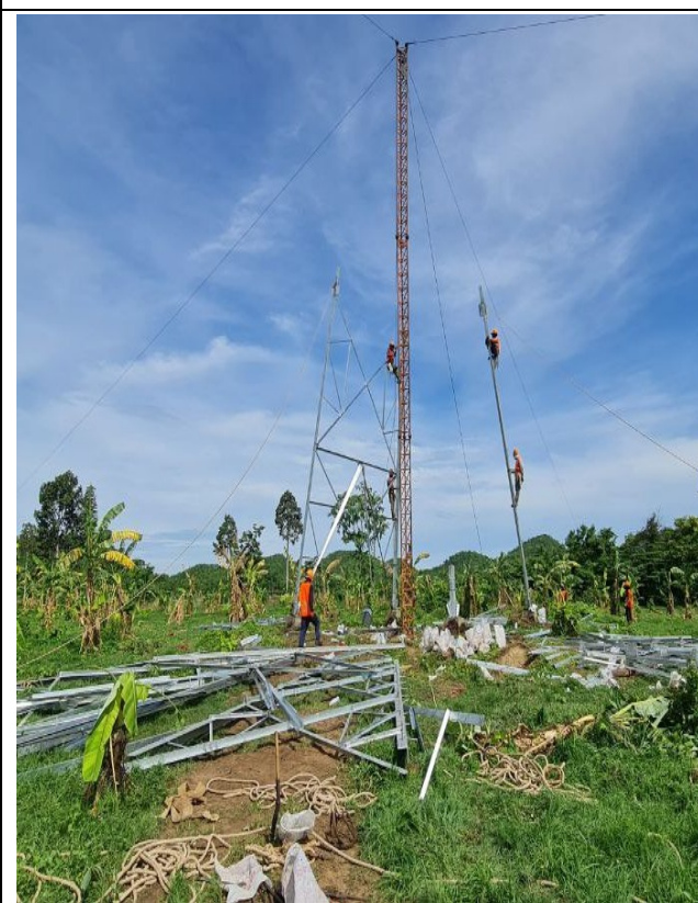
TA125 Tower erection
