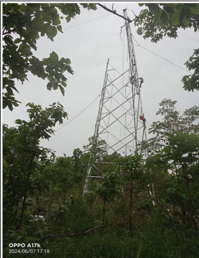
TA130 Tower erection.
