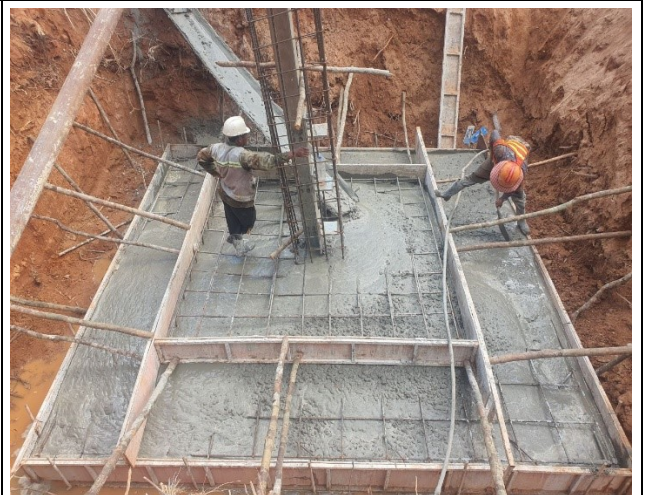
Concrete vibration base.
