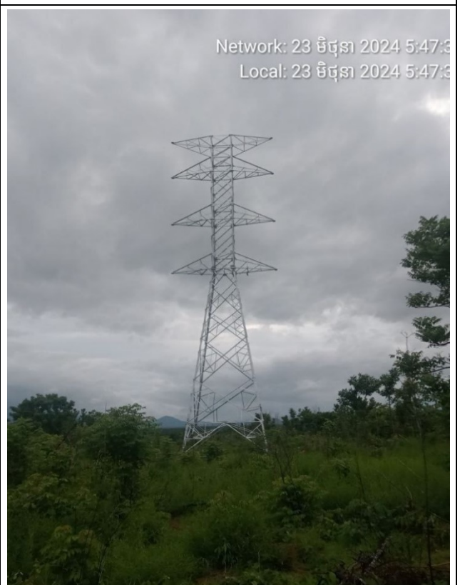
TA188 Erection completd.
