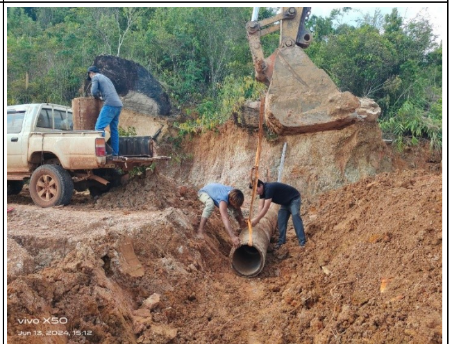
Access Road Work( Drainage pile)
