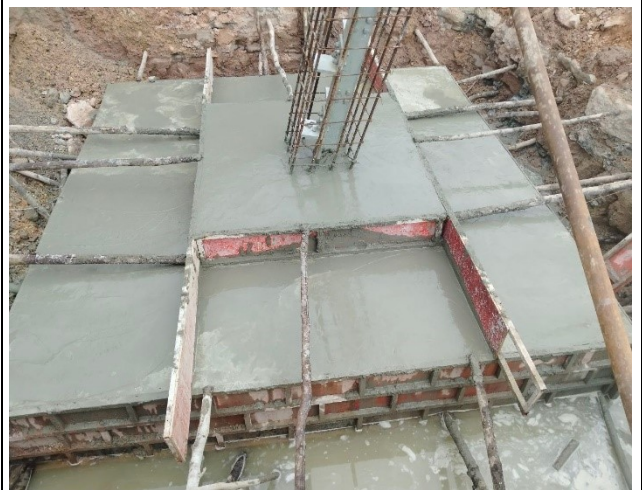
Casting concrete base finish.
