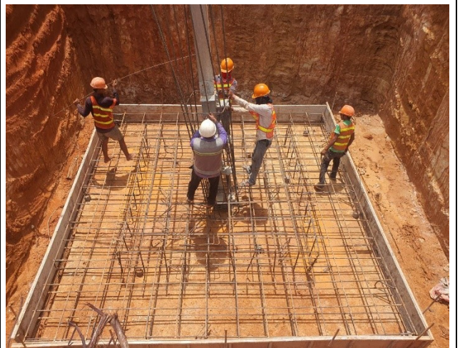
Install rebar of the column.
