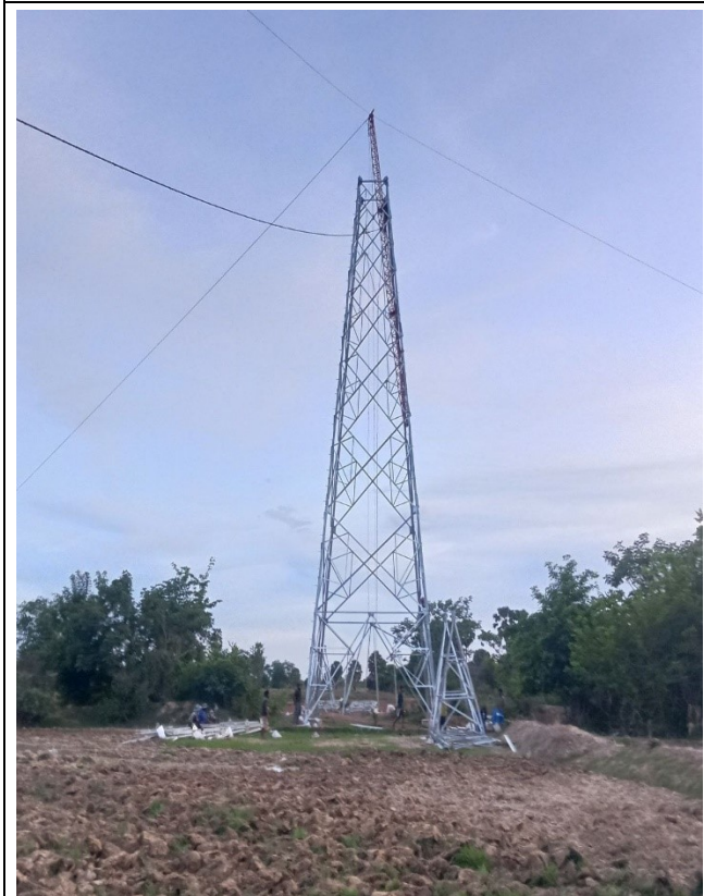
TA108 Tower erection
