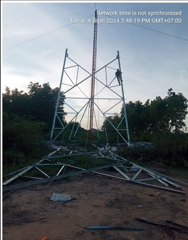
TA126 Tower erection.
