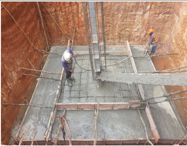
Concrete vibration base.
