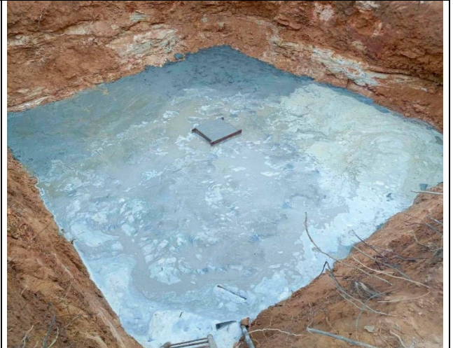
Casting concrete lean
