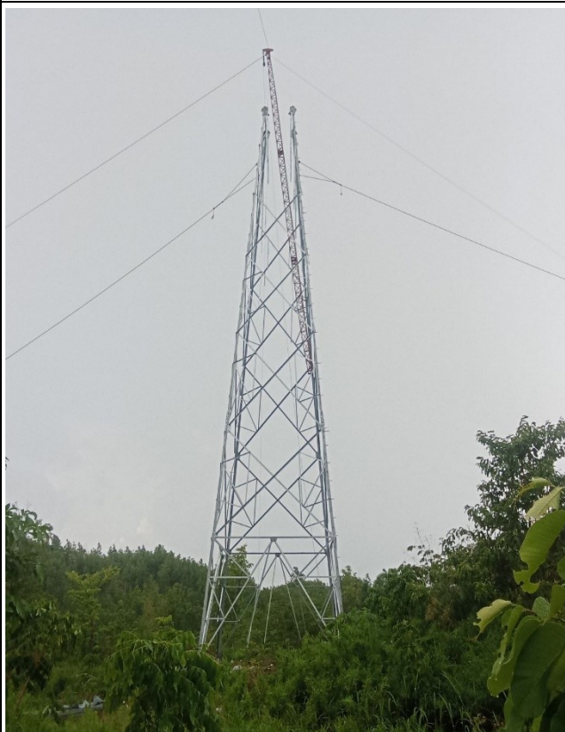
TA141 Tower erection.
