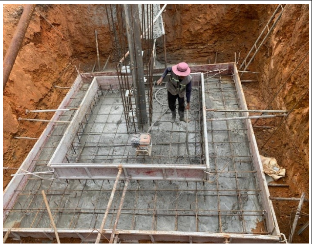
Casting concrete finish.
