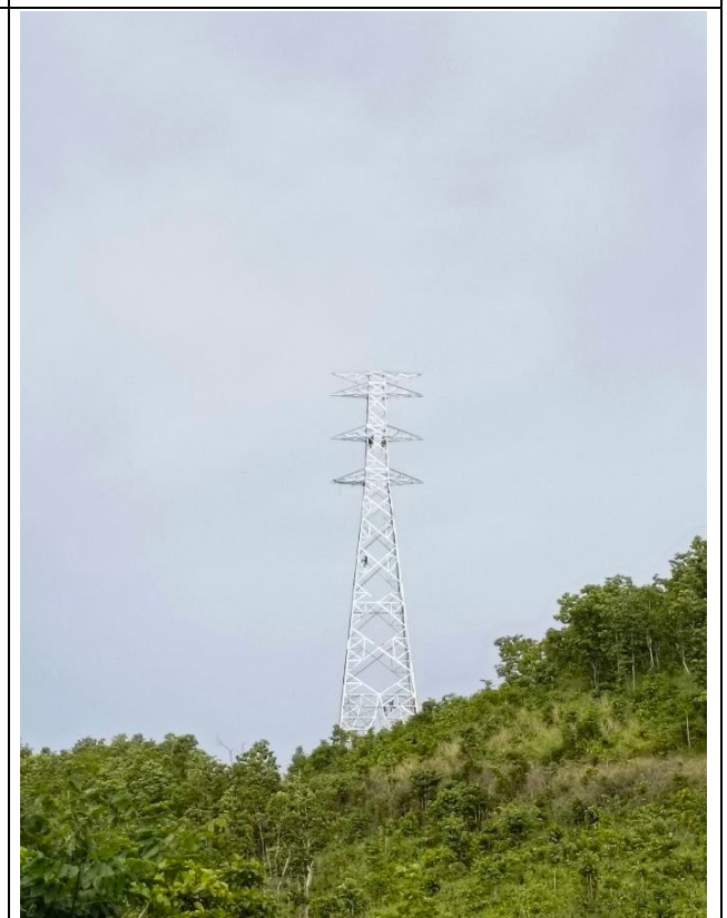
TA180 Erection completd.
