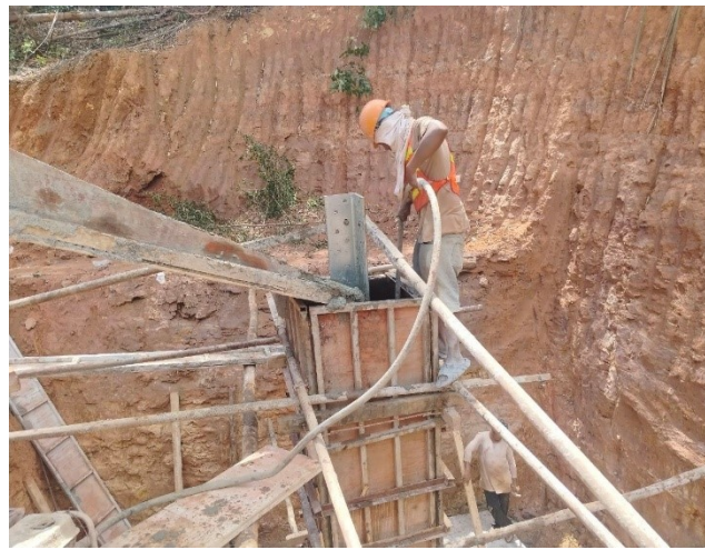
Concrete vibration.
