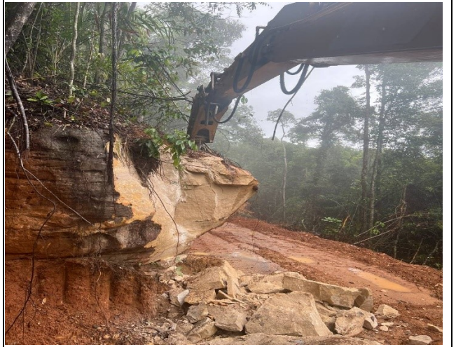
Access Road Work (Breaking stone)
