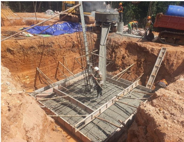
Concrete mixing for the base .
