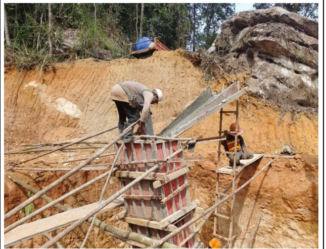
Concrete vibration.
