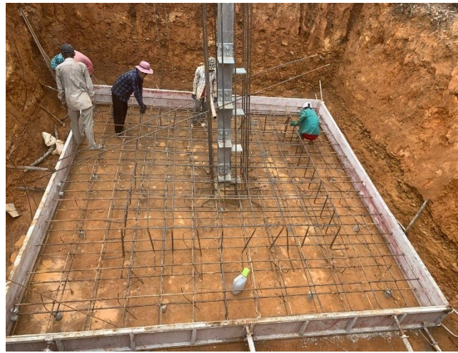
Installation rebar& formwork base.
