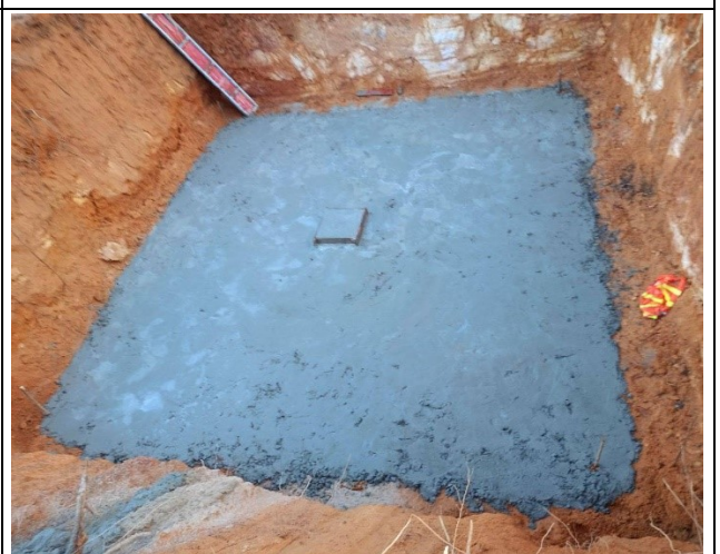
Casting concrete lean
