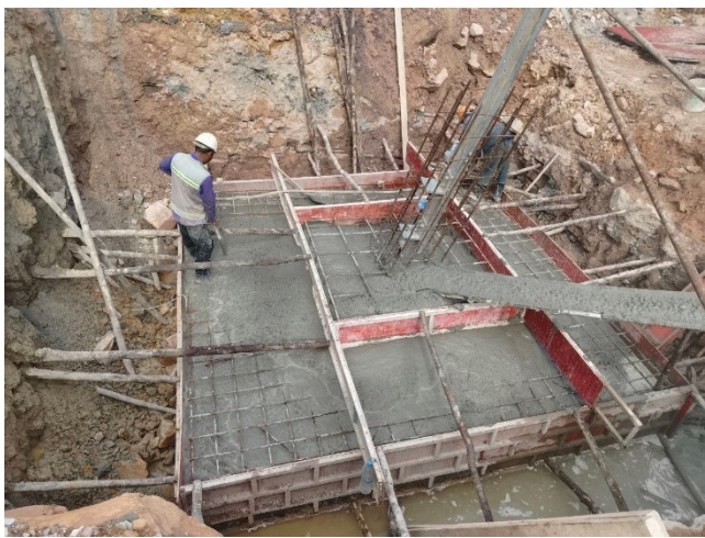
Casting concrete base .
