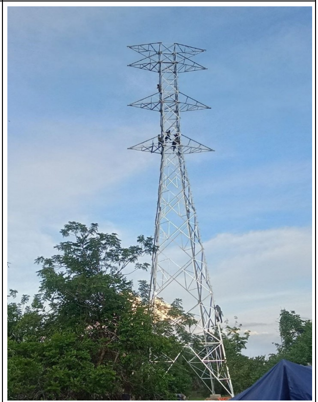
TA108 Erection completd.
