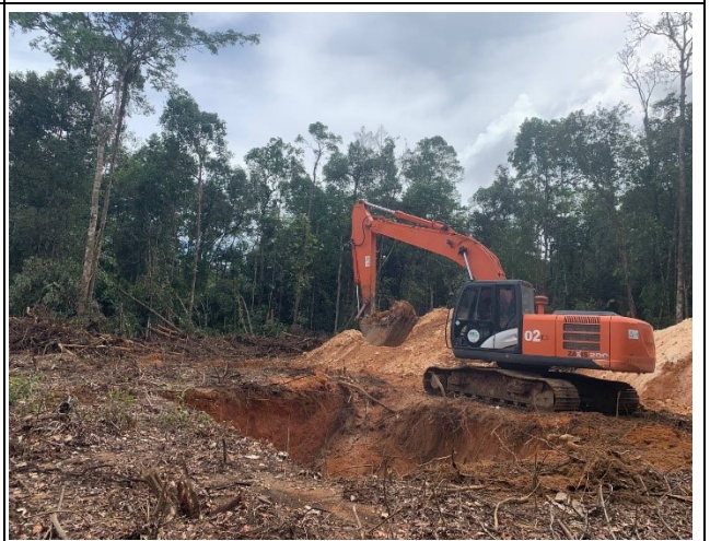
Soil excavatoin of the pit.
