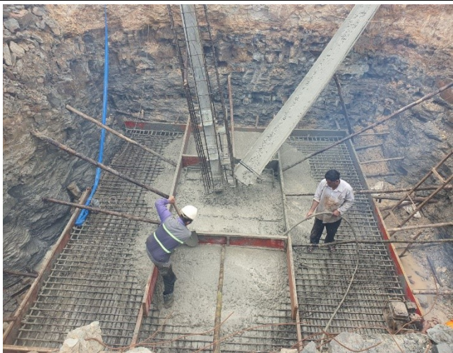
Casting concrete base .
