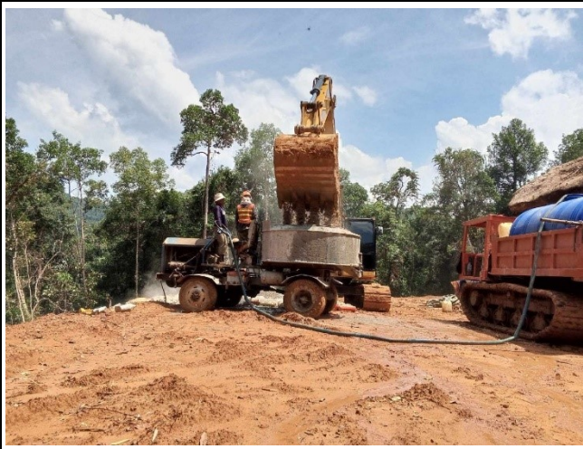
Concrete mixing
