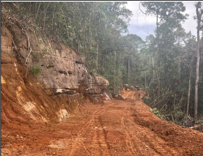
Access Road Work
