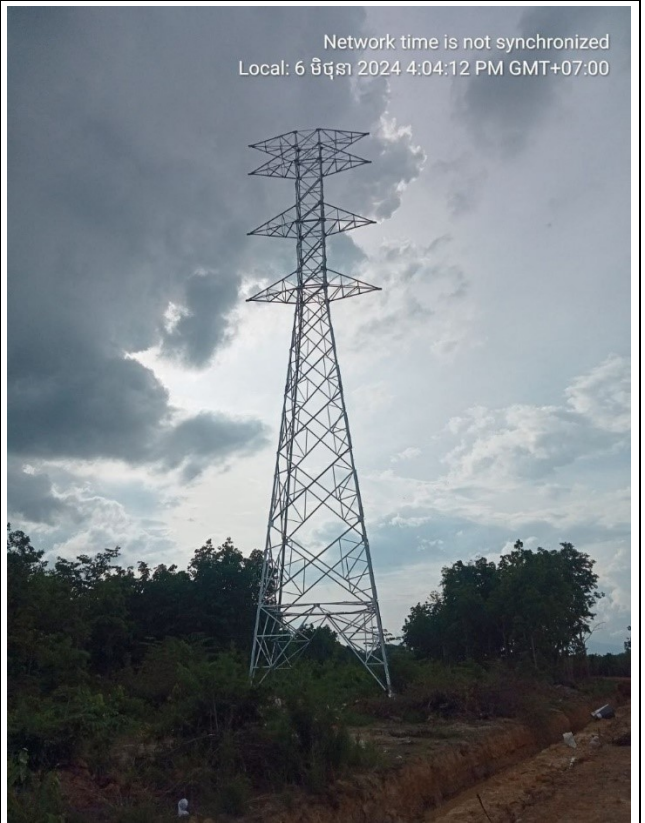
TA126 Erection completd.
