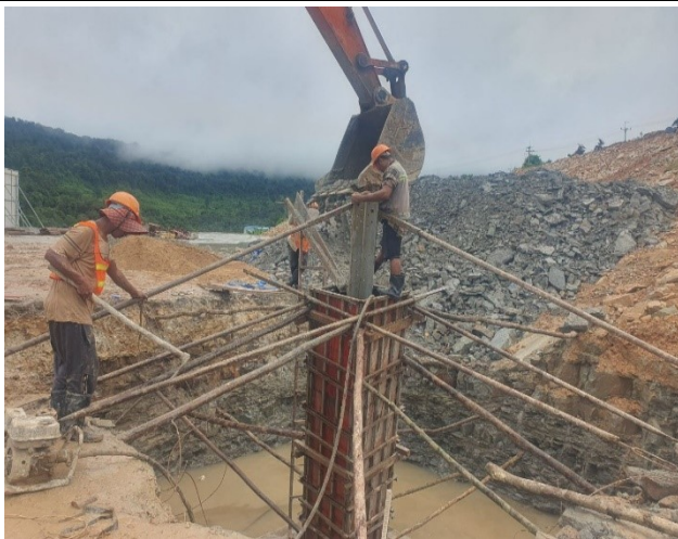
Casting concrete chimney .
