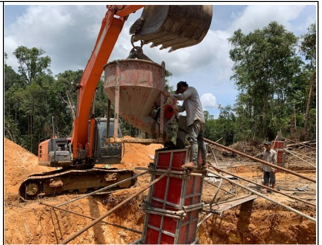
Casting concrete chimney
