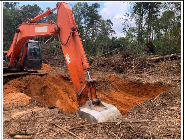
Soil excavatoin of the pit.
