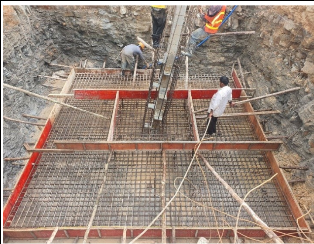
Rebar installation & formworks.
