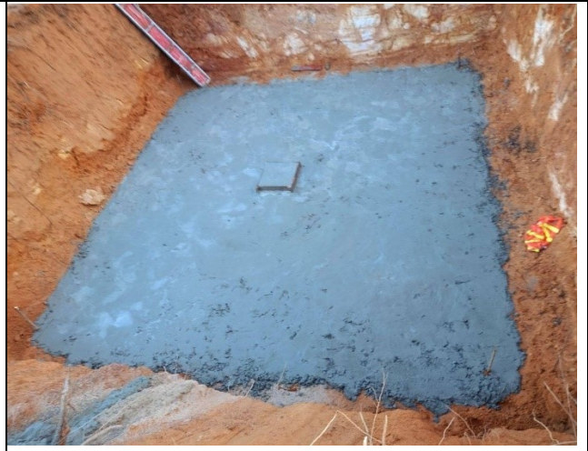
Casting concrete lean
