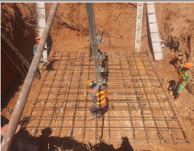
Install rebar.
