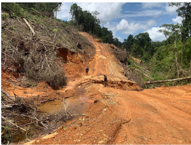
Access Road Work
