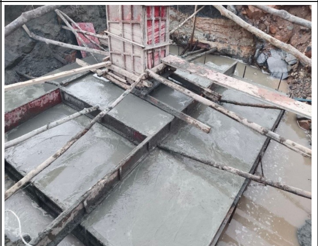
Casting concrete base finish.
