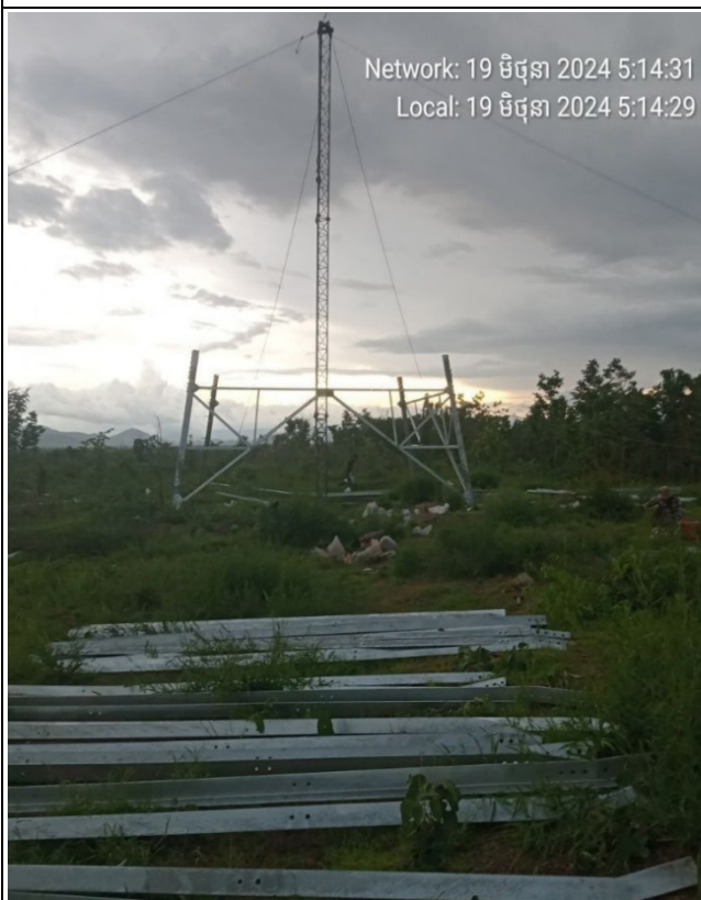
TA188 Tower erection
