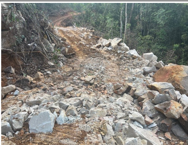
Access Road Work (Breaking stone)
