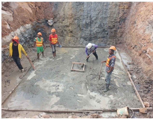
Casting concrete lean
