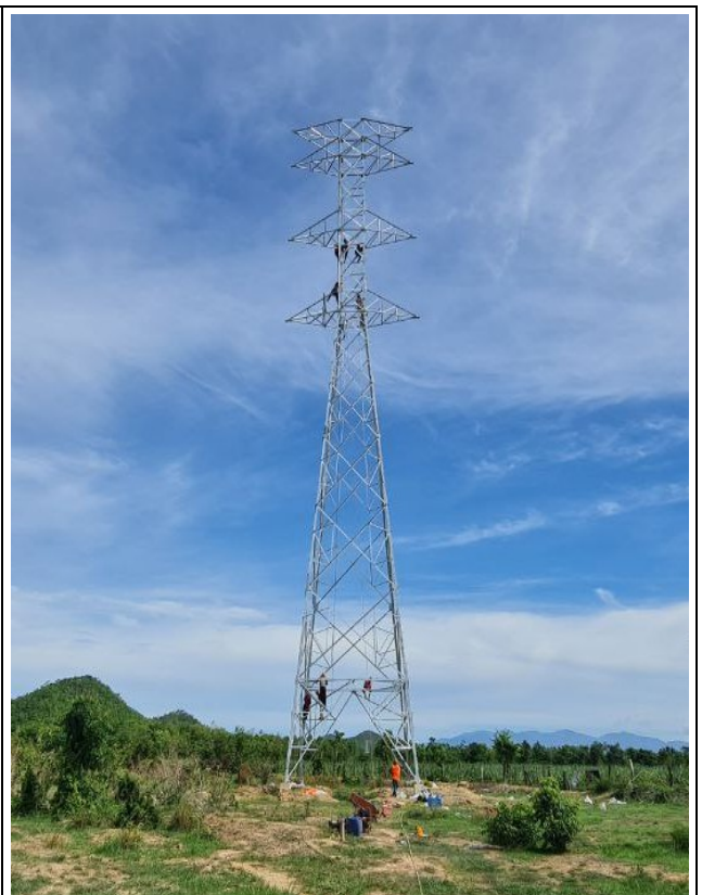
TA124 Erection completed.
