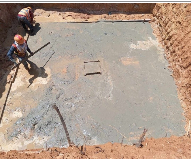
Casting concrete lean
