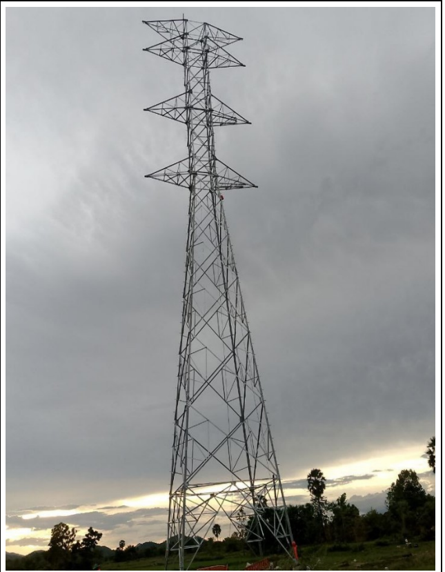
TA118 Erection completed.
