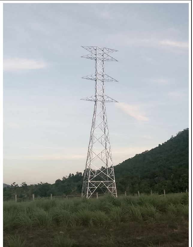
TA158 Erection completd.
