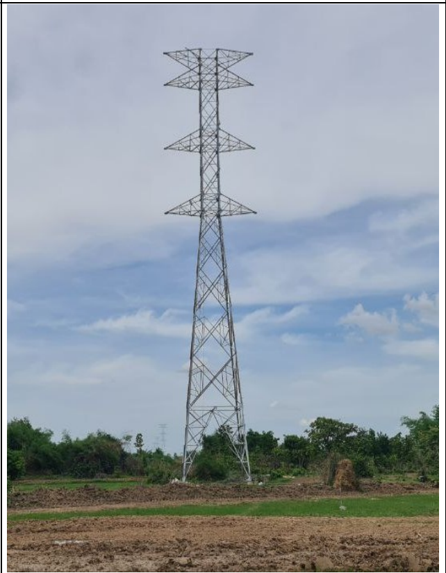
TA098 Erection completd.
