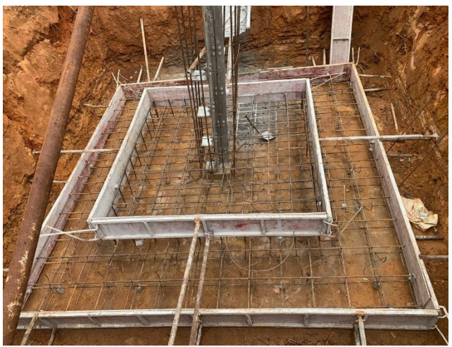
Installation rebar& formwork base.
