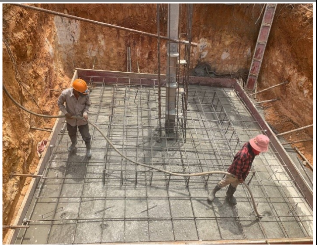
Concrete vibration
