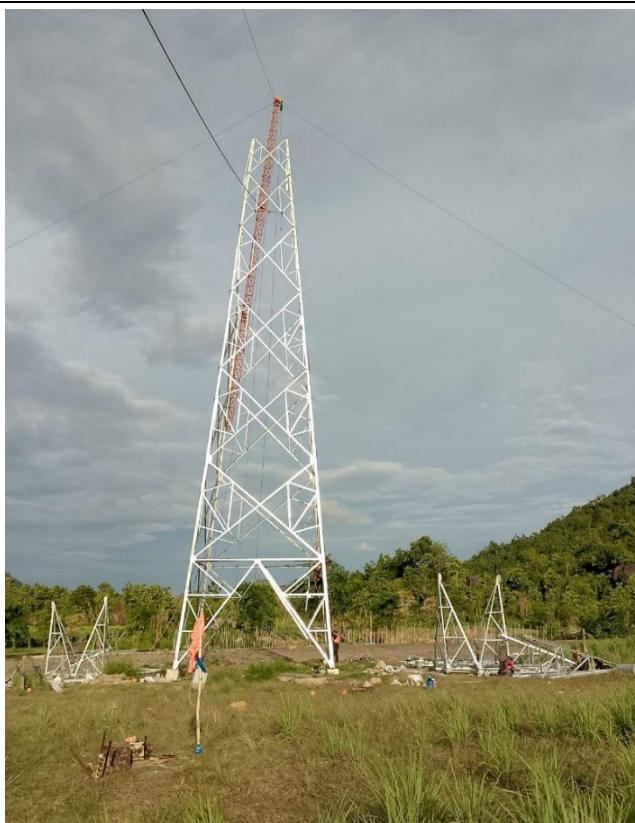
TA158 Tower erection
