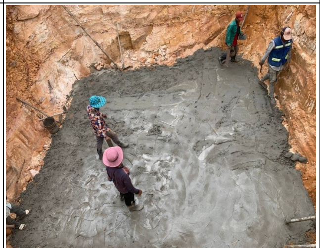
Casting concrete lean
