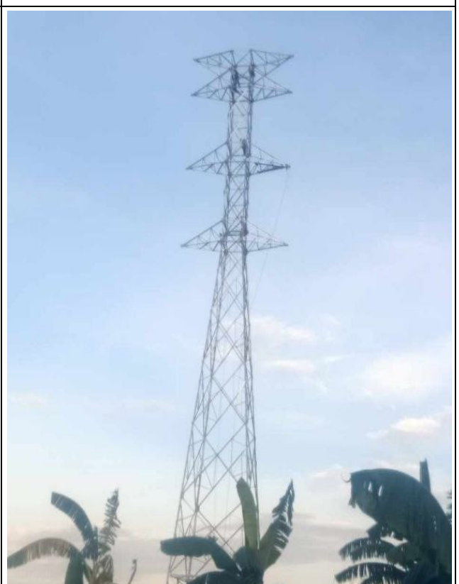
TA125 Erection completd.
