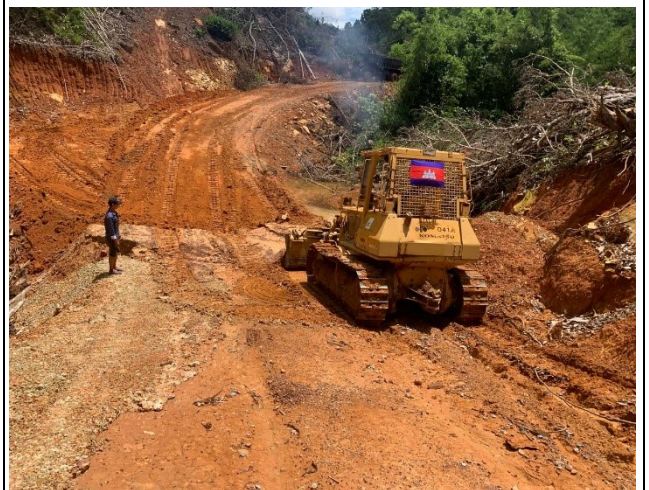
Access Road Work
