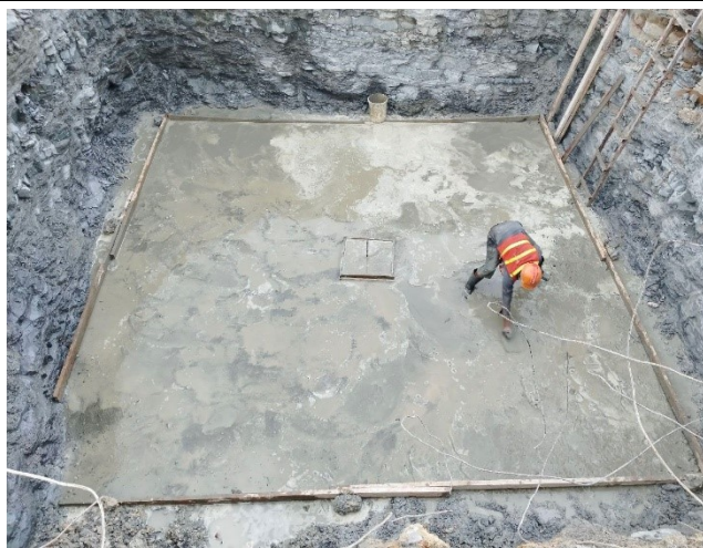
Casting concrete lean
