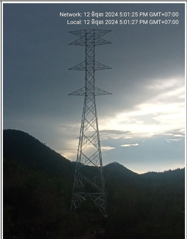
TA138 Erection completed.
