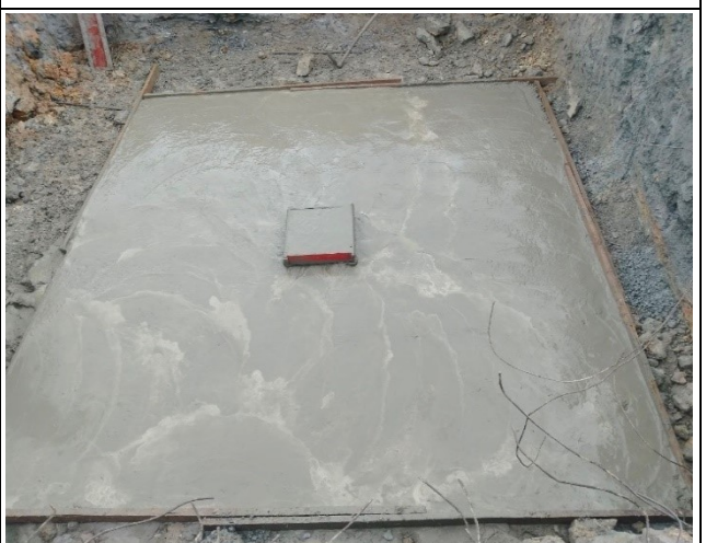
Casting concrete lean
