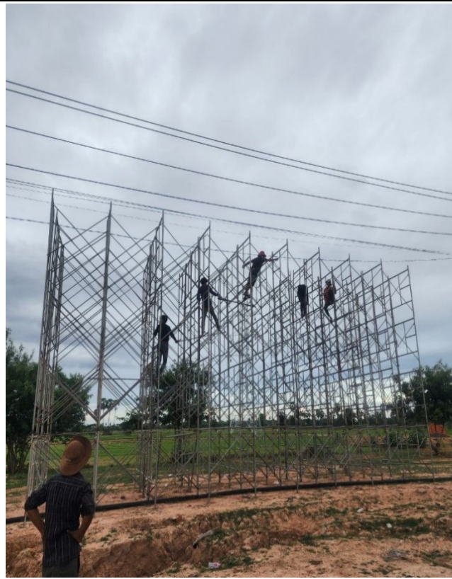
Installation scaffuding between T-A026, T-A026A
