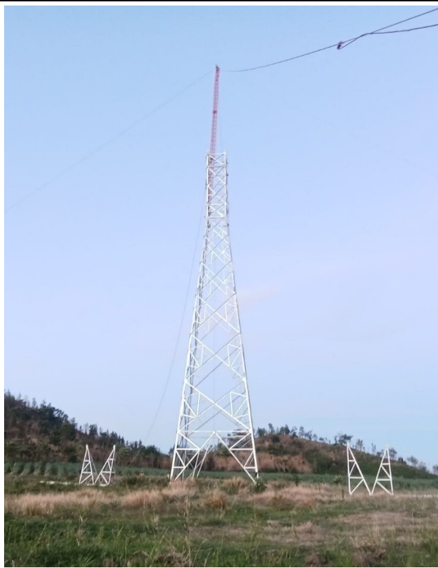
TA151 Tower erection.
