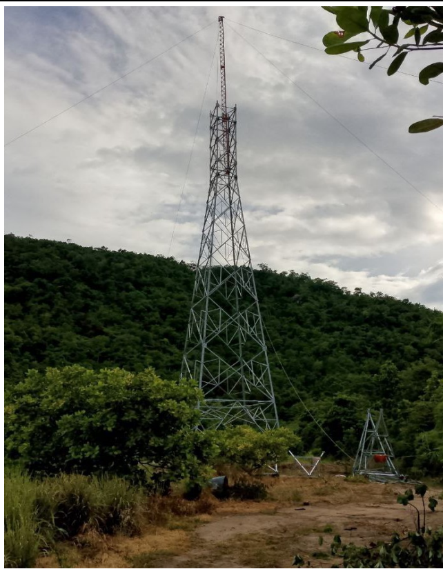
TA156 Tower erection
