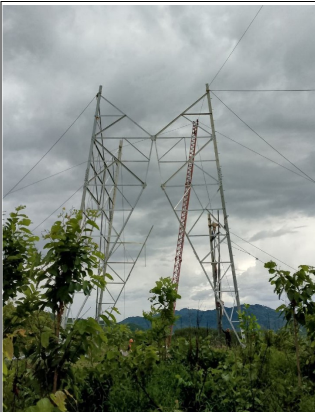
TA181 Tower erection
