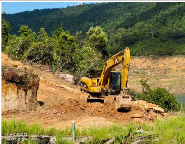
Repair access Road Work
