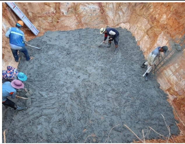
Casting concrete lean
