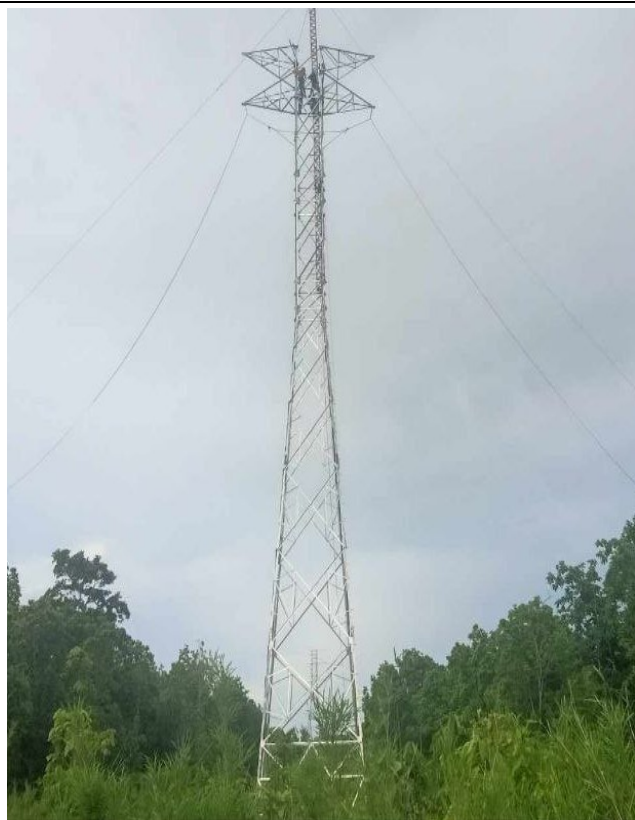
TA135 Tower erection.
