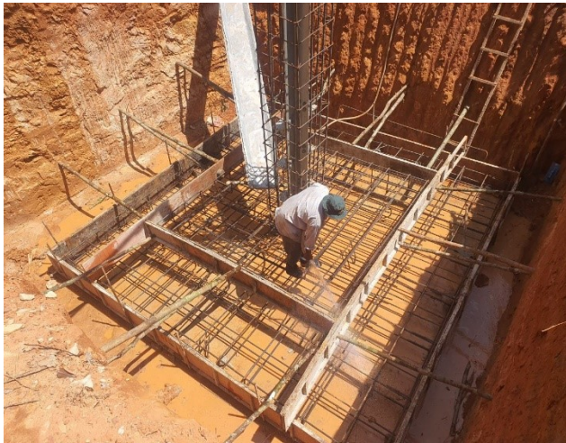
Install formworks of the base .
