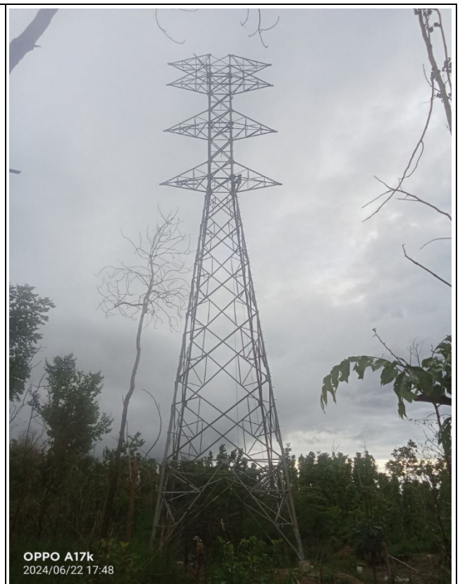
TA168 Erection completed.
