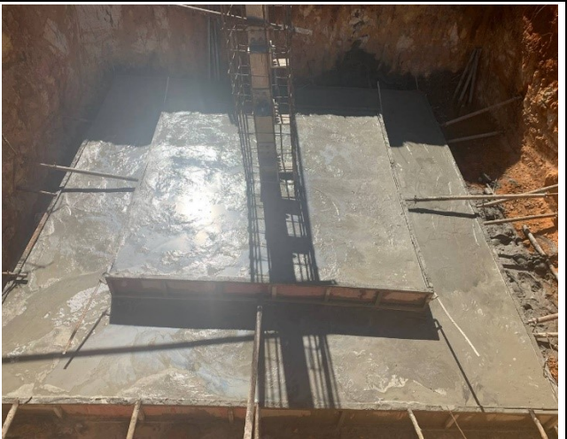
Casting leveling.
