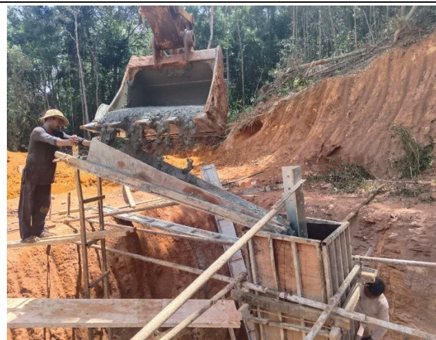
Casting concrete of the chimney.
