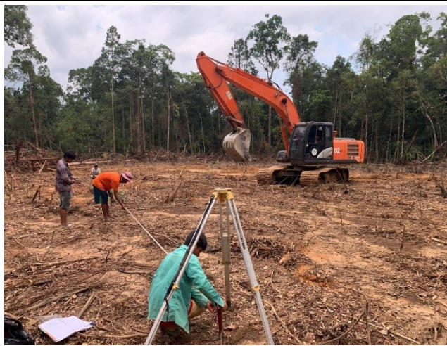
Measuring for excavatoin of the pit.
