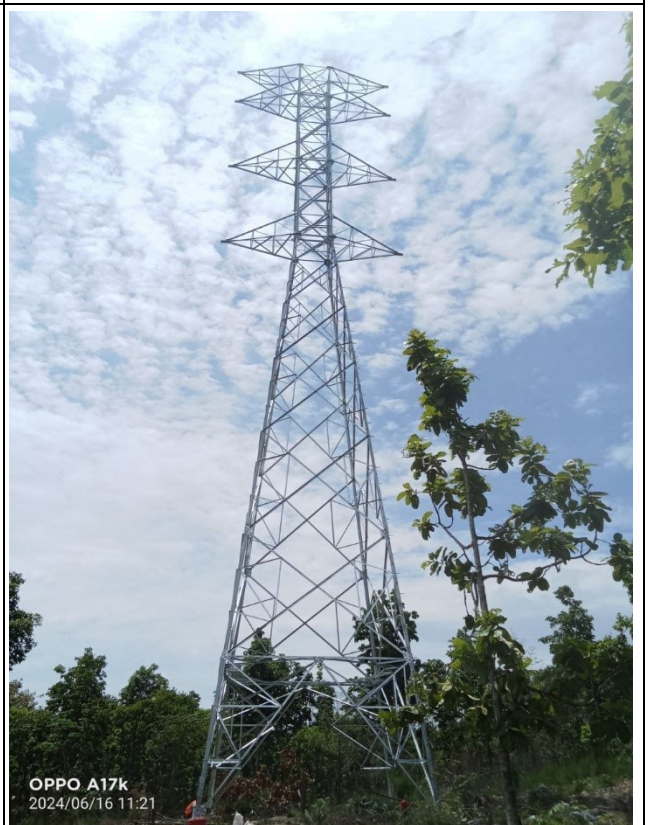
TA131 Erection completd.
