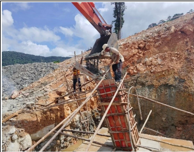
Casting concrete chimney .
