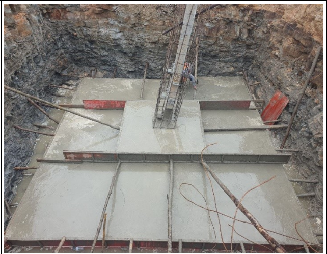
Casting concrete base finish.
