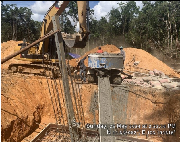
Casting concrete
