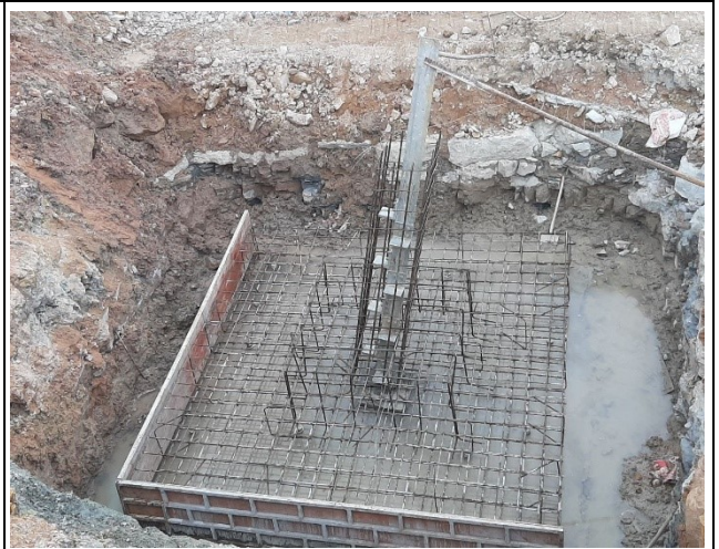
Rebar installation.
