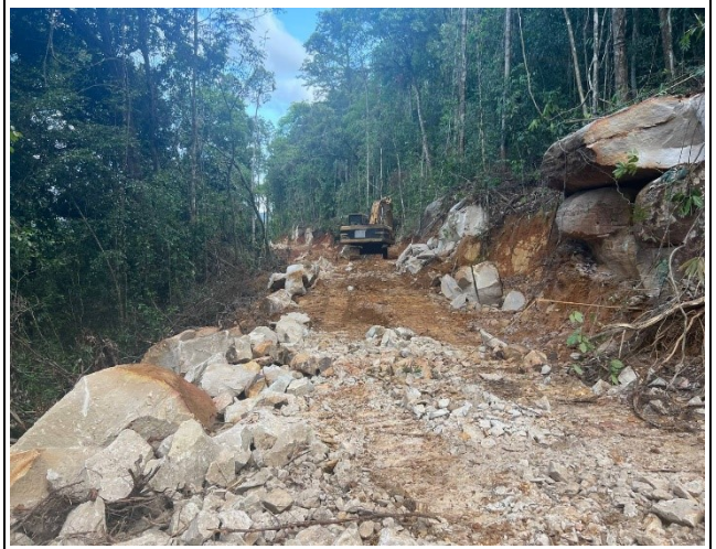
Access Road Work (Breaking stone)
