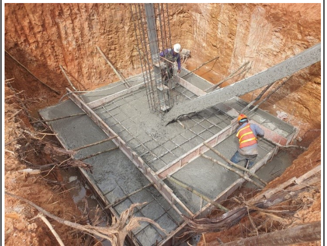
Casting concrete base
