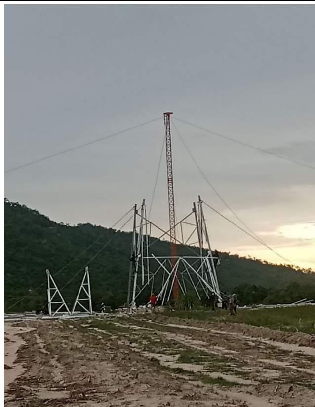
TA152 Tower erection.
