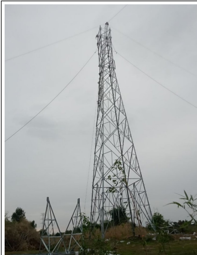
TA097 Tower erection
