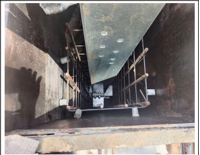
Concrete vibration base.
