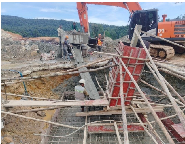
Casting concrete base .
