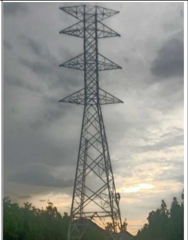
TA134 Erection completed.
