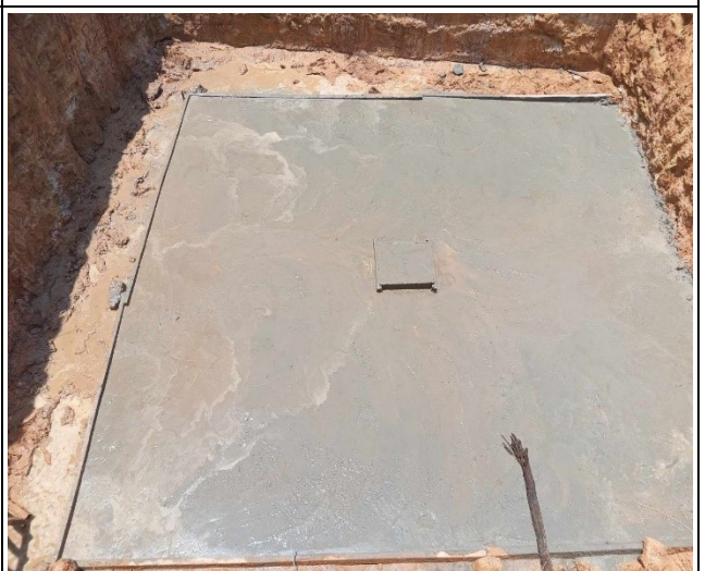
Casting concrete lean
