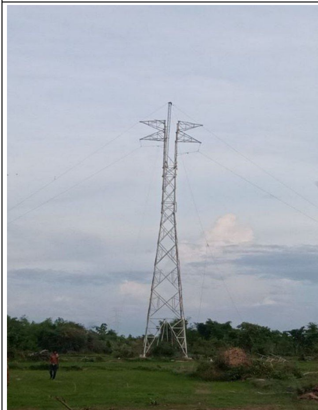
TA098 Tower erection
