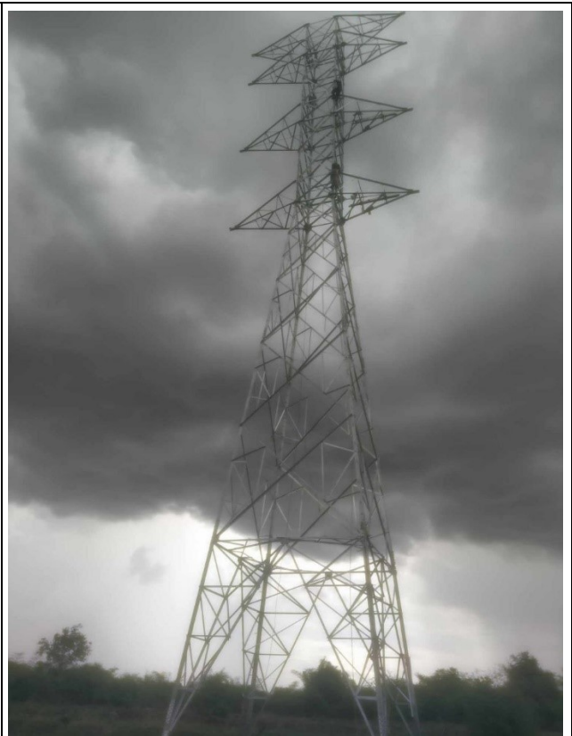
TA097 Erection completed.
