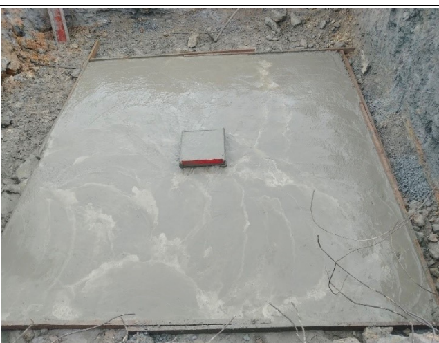
Casting concrete lean
