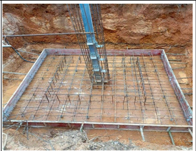
Installation formwork base.
