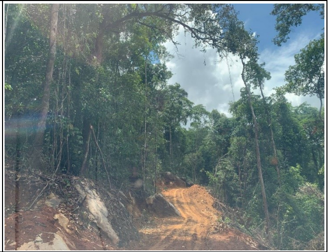
Access Road Work
