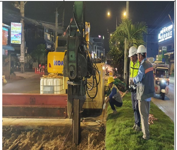
Sheet Pile Installation activity
