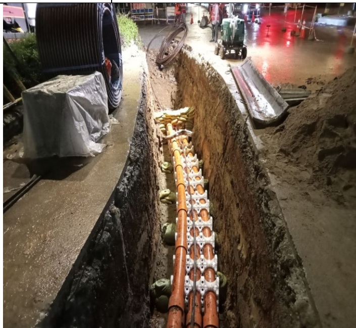
Photo: 22 Assembly PFP pipes and OFC pipe
