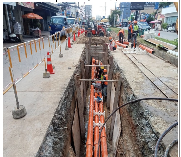
Photo: 06 Assembly PFP pipes and OFC pipe
