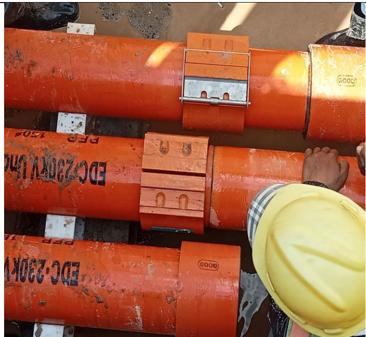
Photo: 08 Assembly PFP pipes and OFC pipe
