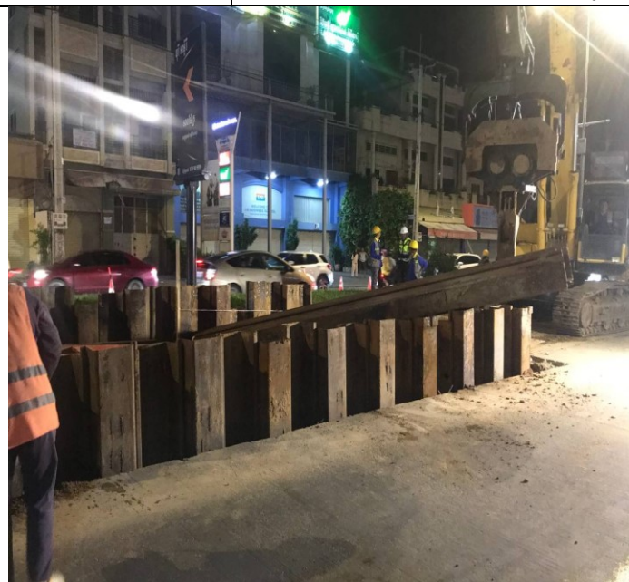
Sheet Pile Installation activity
