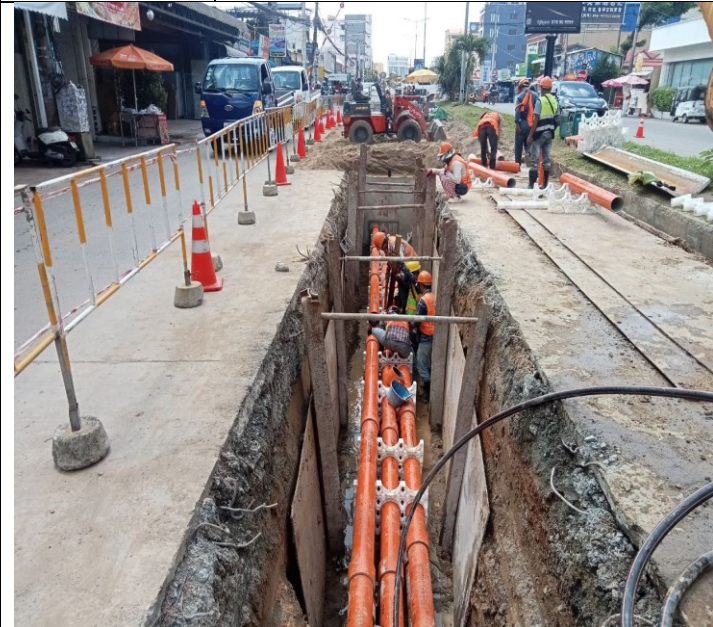
Photo: 09 Assembly PFP pipes and OFC pipe
