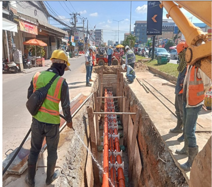
Photo: 12 Assembly PFP pipes and OFC pipe
