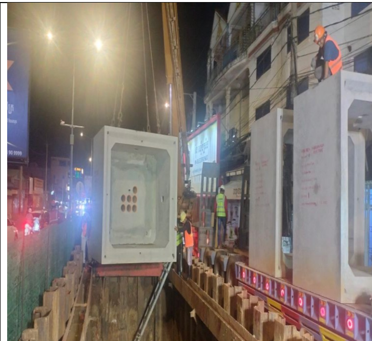
Photo: 19 Manhole Installation activity
