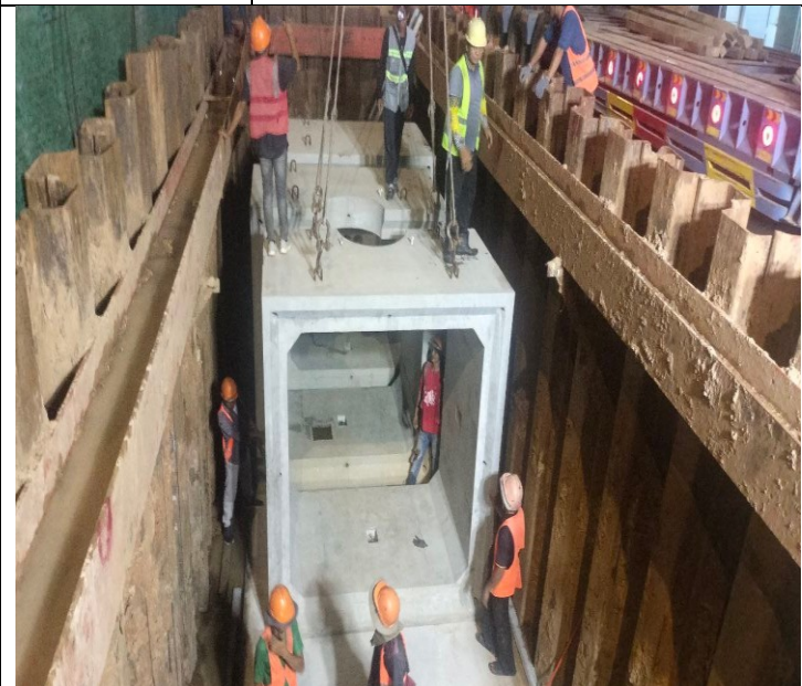
Photo: 21 Manhole Installation activity
