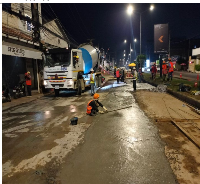
Photo: 10 Restoration of concrete road
