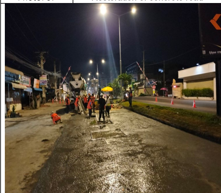
Photo: 09 Restoration of concrete road
