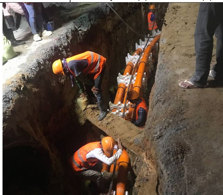
Photo: 28 Assembly PFP pipes and OFC pipe
