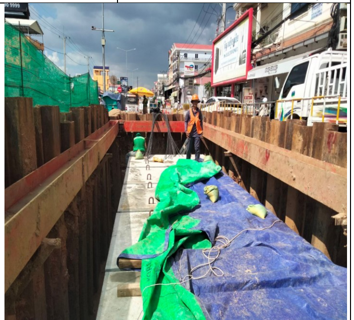
Photo: 24 Manhole Installation activity
