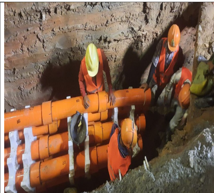
Photo: 25 Assembly PFP pipes and OFC pipe
