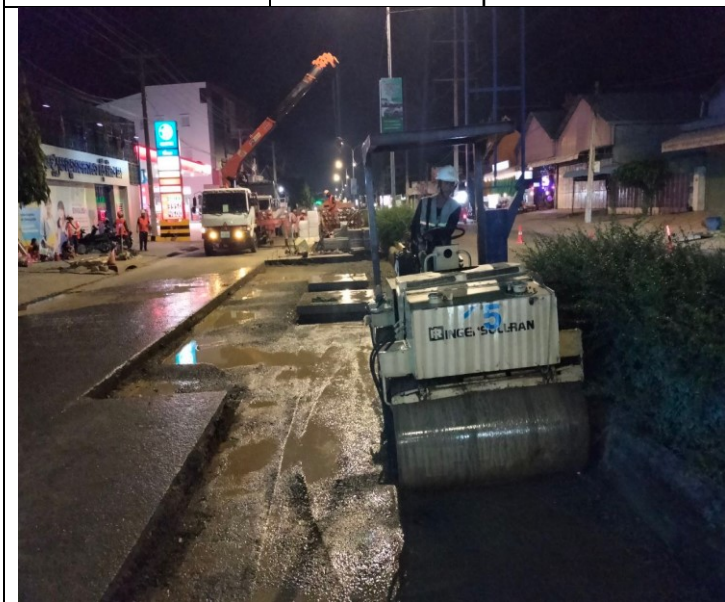
Base course backfilling and compaction
