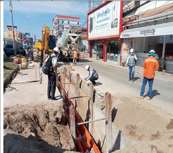
Photo: 11 Assembly PFP pipes and OFC pipe
