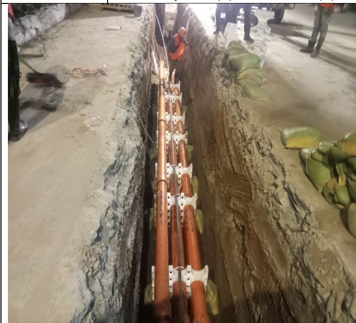
Photo: 17 Assembly PFP pipes and OFC pipe
