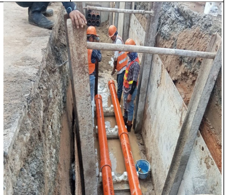
Photo: 04 Assembly PFP pipes and OFC pipe
