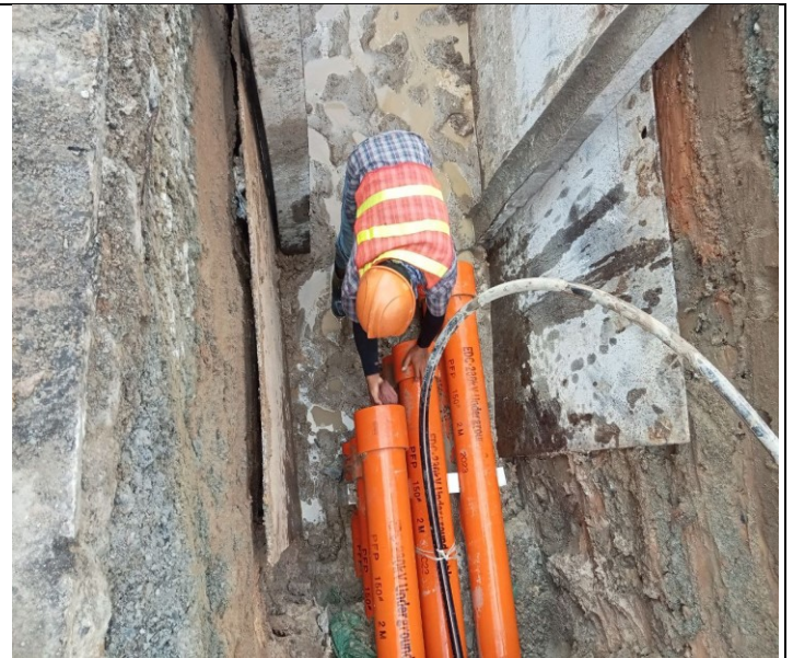
Photo: 02 Assembly PFP pipes and OFC pipe
