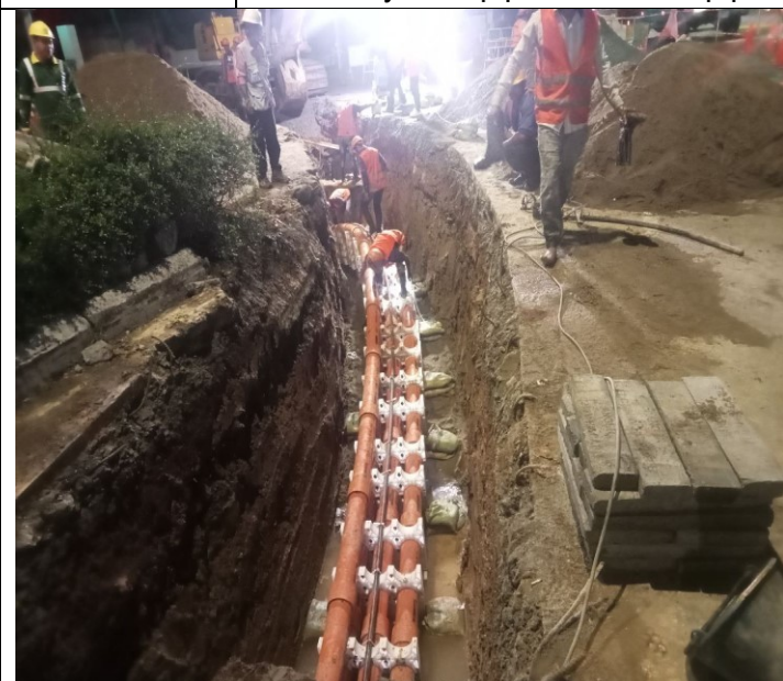
Photo: 27 Assembly PFP pipes and OFC pipe
