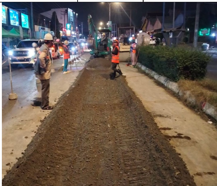
Base course backfilling and compaction
