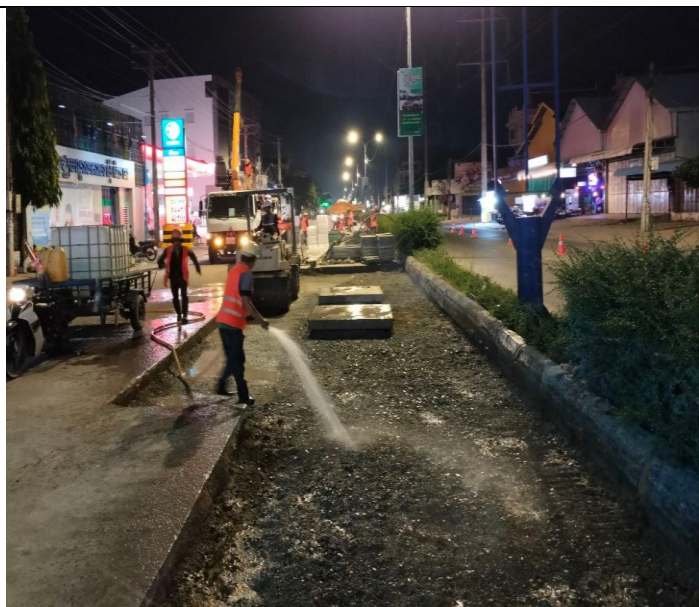
Base course backfilling and compaction
