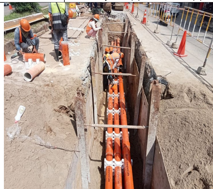
Photo: 05 Assembly PFP pipes and OFC pipe
