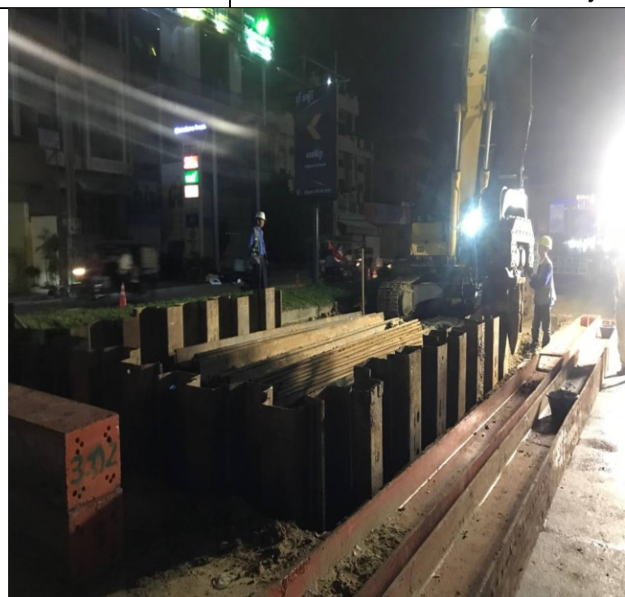
Sheet Pile Installation activity
