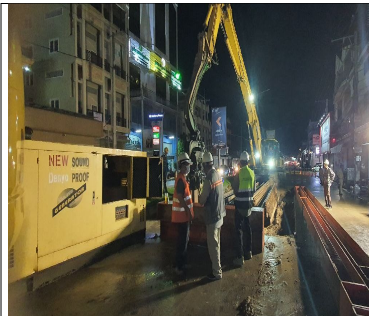
Sheet Pile Installation activity
