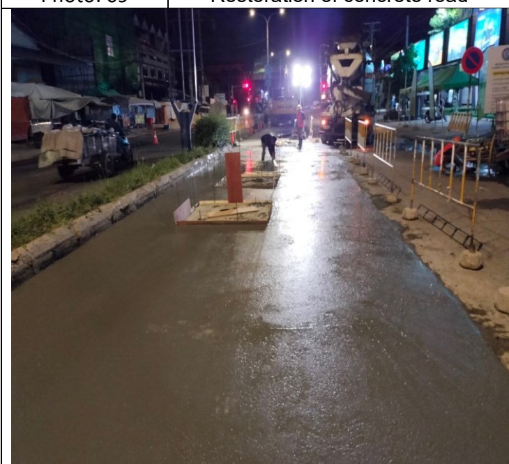
Photo: 11 Restoration of concrete road
