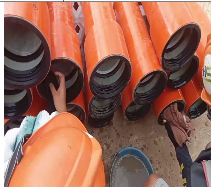
Photo: 03 Assembly PFP pipes and OFC pipe
