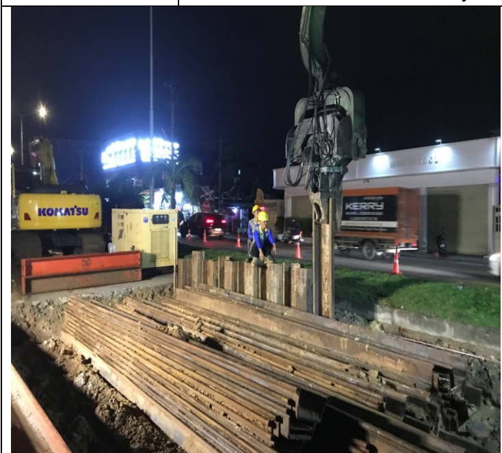
Sheet Pile Installation activity
