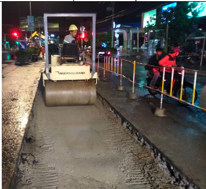
Base course backfilling and compaction
