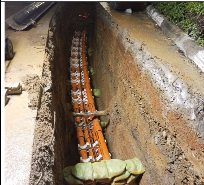
Photo: 21 Assembly PFP pipes and OFC pipe
