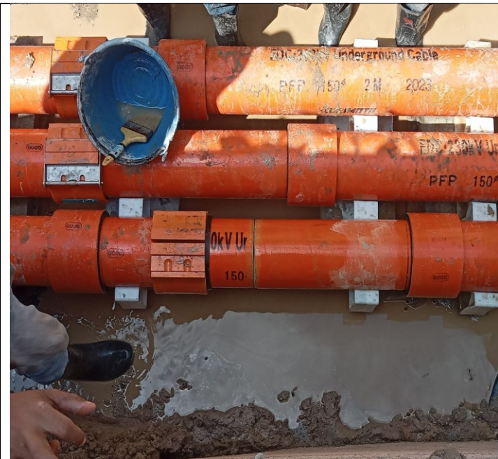
Photo: 07 Assembly PFP pipes and OFC pipe
