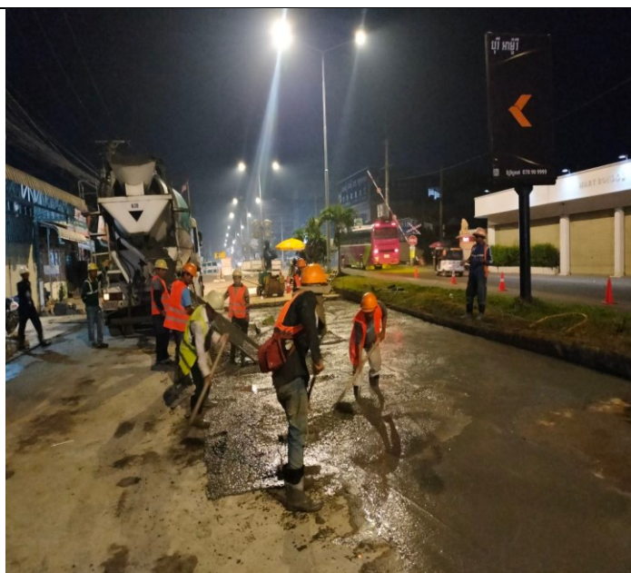
Photo: 08 Restoration of concrete road
