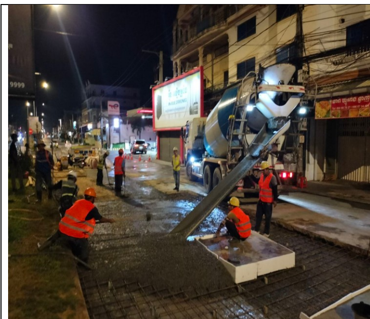
Photo: 07 Restoration of concrete road
