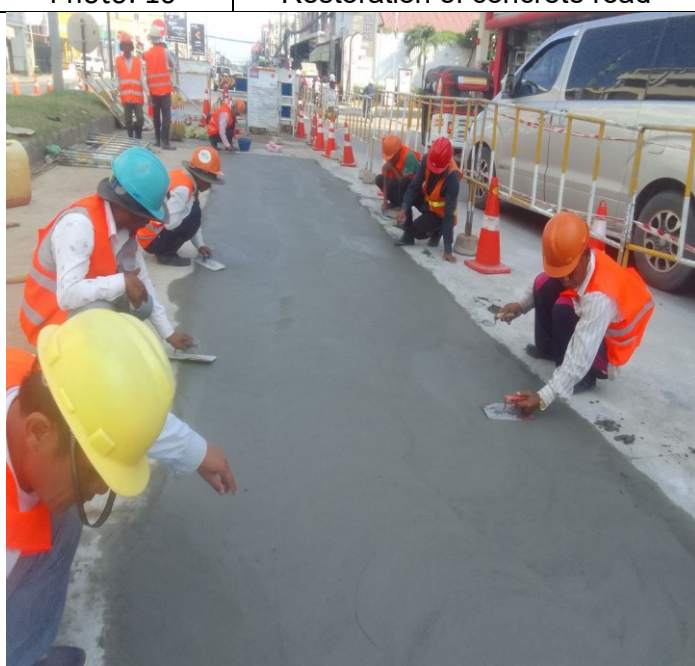
Photo: 12 Restoration of concrete road
