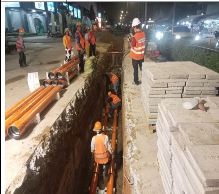
Photo: 15 Assembly PFP pipes and OFC pipe
