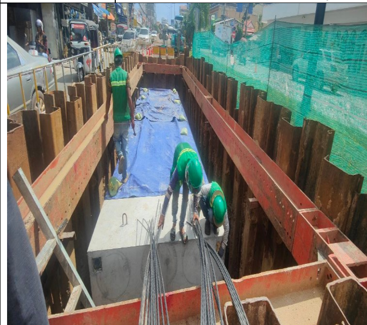
Photo: 23 Manhole Installation activity
