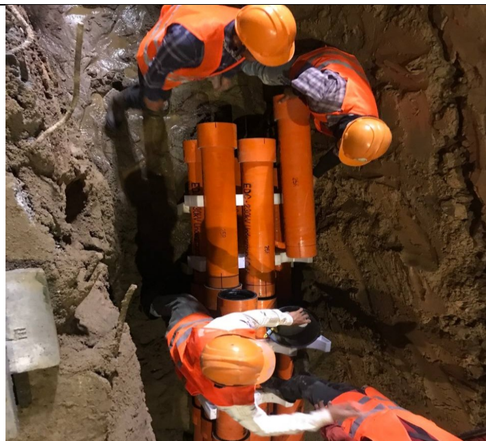
Photo: 26 Assembly PFP pipes and OFC pipe
