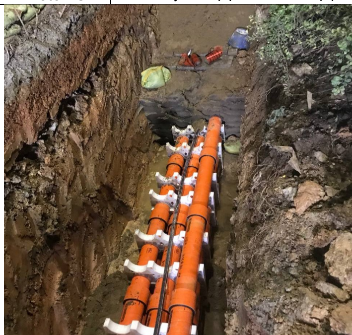
Photo: 30 Assembly PFP pipes and OFC pipe
