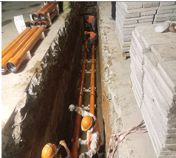
Photo: 16 Assembly PFP pipes and OFC pipe
