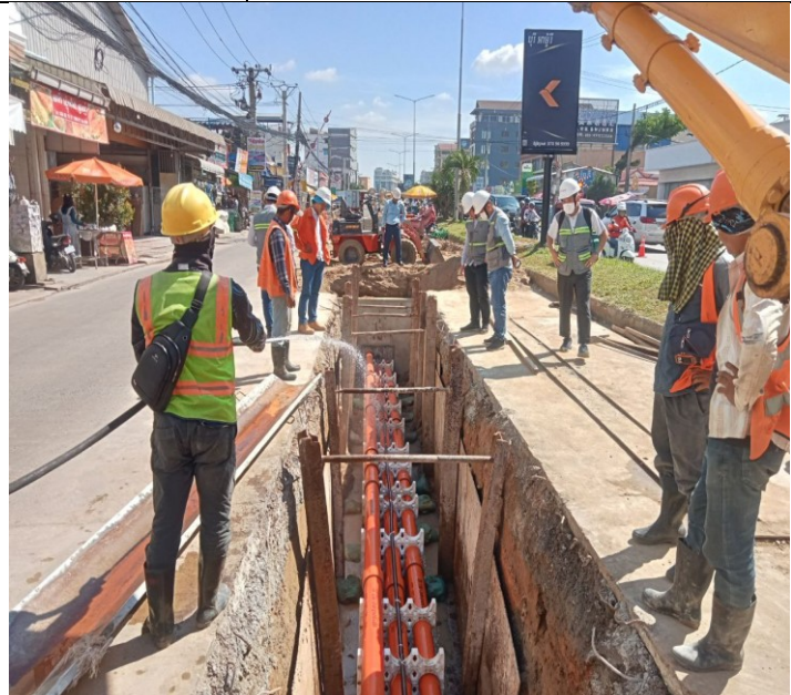
Photo: 10 Assembly PFP pipes and OFC pipe
