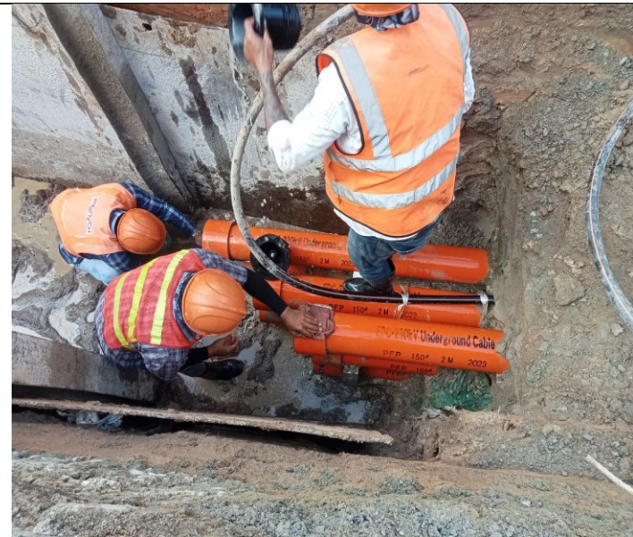
Photo: 01 Assembly PFP pipes and OFC pipe
