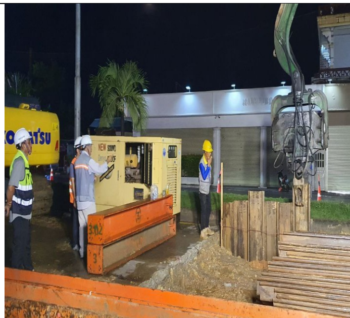
Sheet Pile Installation activity
