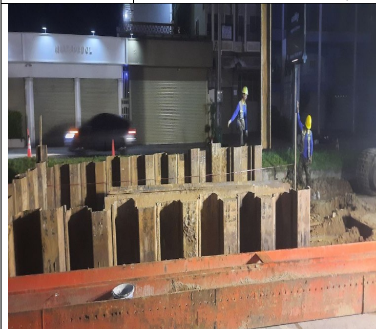
Sheet Pile Installation activity
