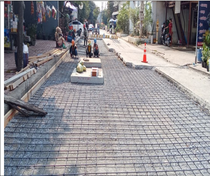
Photo: 07 Manhole of concrete road activity
