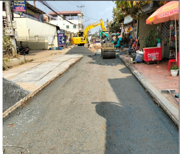
Photo: 04 | Manhole of concrete road activity
