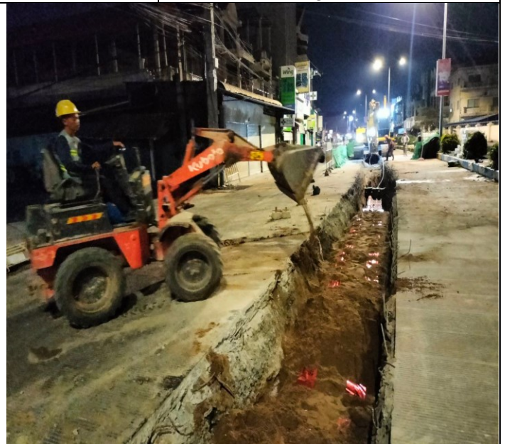
Photo: 04 Sand backfilling and compaction
