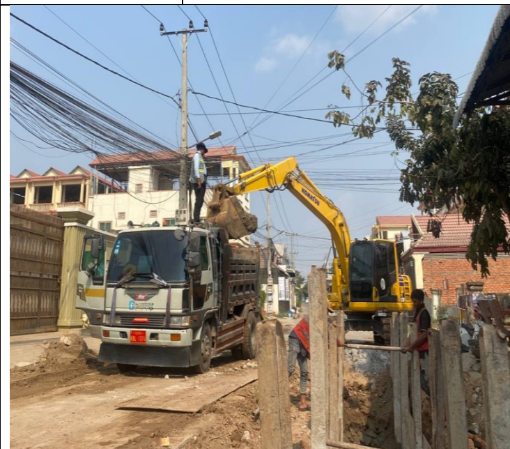
Photo: 15 Soil excavation and concrete road
