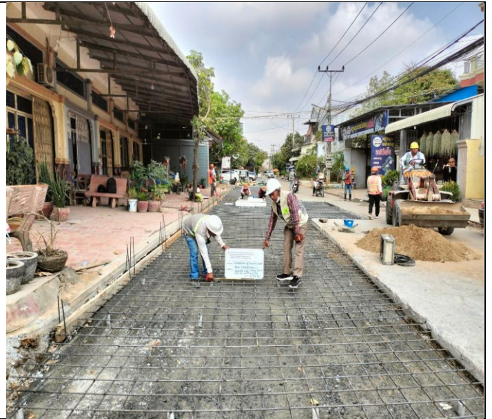
Photo: 08 Manhole of concrete road activity
