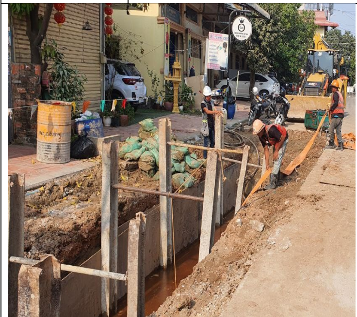
Photo: 11 Soil excavation and concrete road
