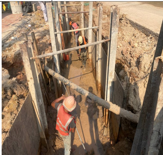
Photo: 18 Soil excavation and concrete road
