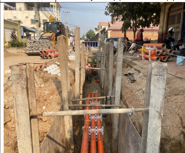
Photo: 05 Assembly PFP pipes and OFC pipe
