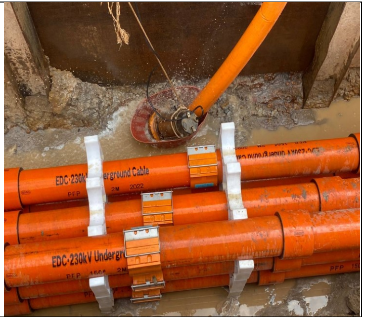
Photo: 02 Assembly PFP pipes and OFC pipe
