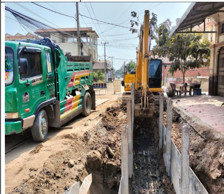
Photo: 09 Soil excavation and concrete road
