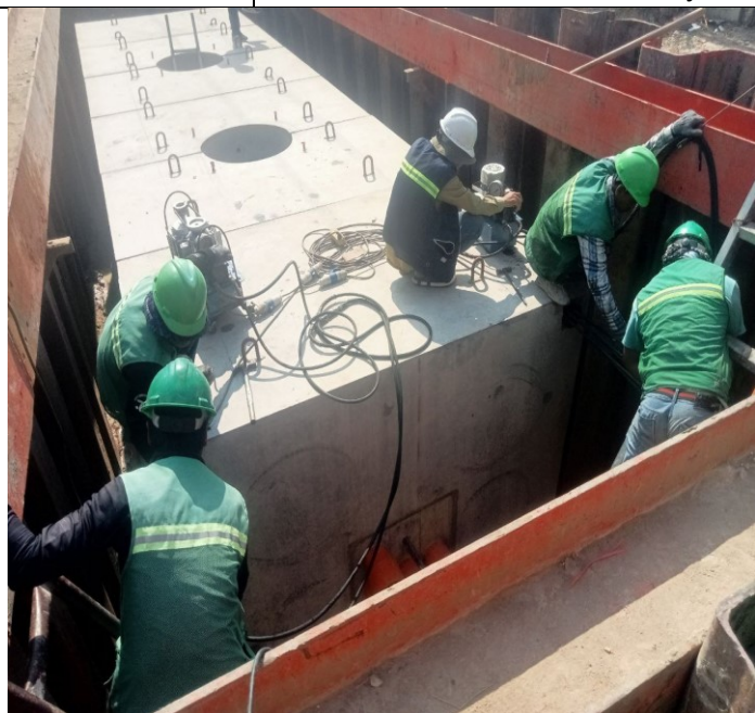
Photo: 48 Manhole Installation activity
