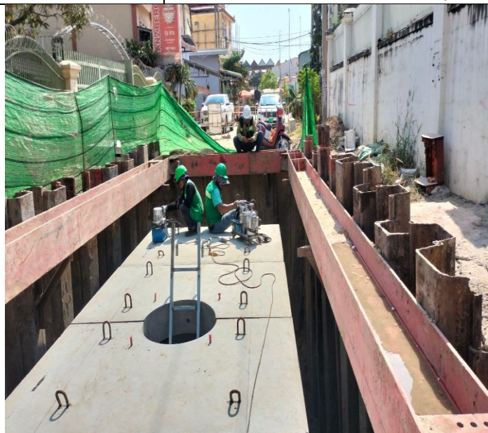
Photo: 46 Manhole Installation activity
