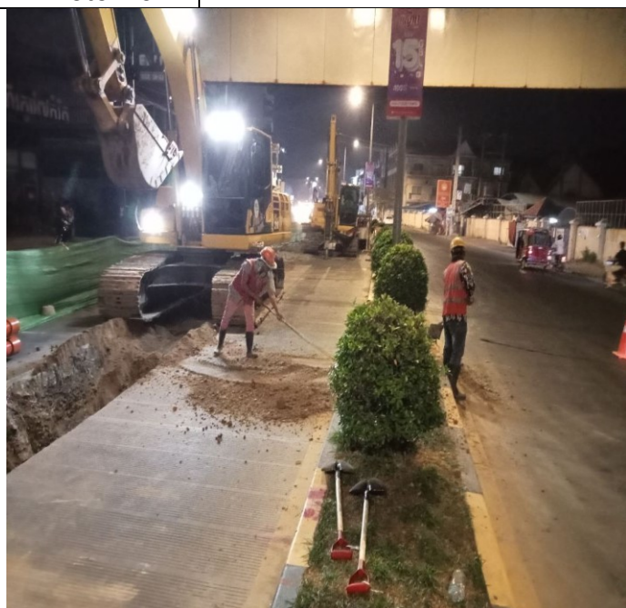
Photo: 22 Soil excavation and concrete road
