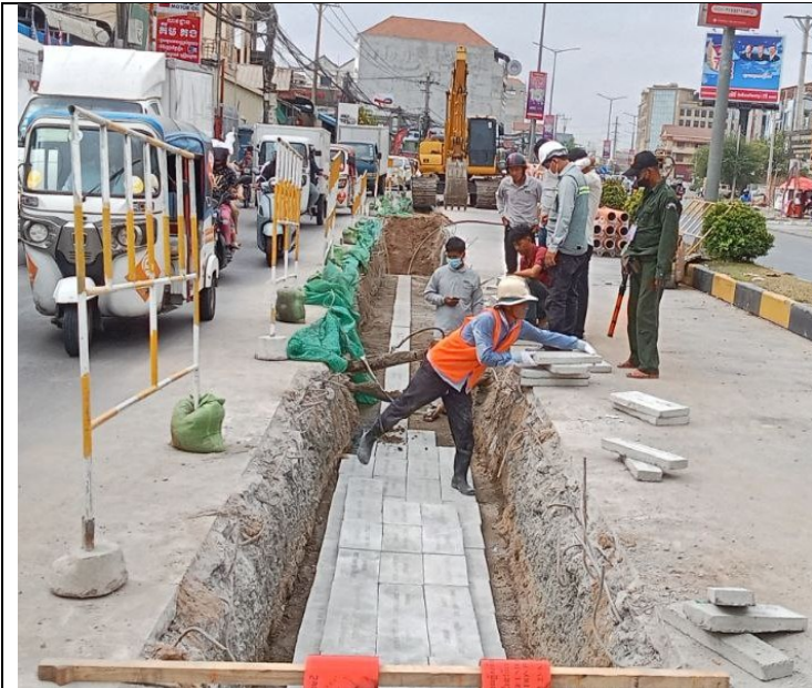
Laying concrete protection slab and warning tap
