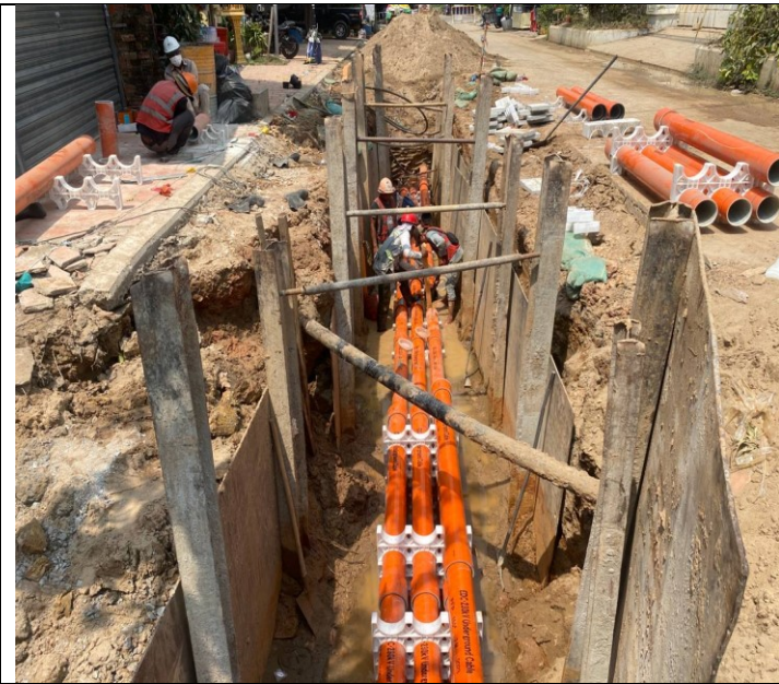
Photo: 01 Assembly PFP pipes and OFC pipe
