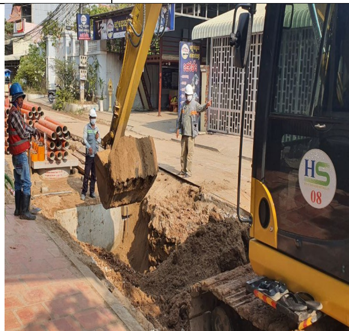
Photo: 12 Soil excavation and concrete road
