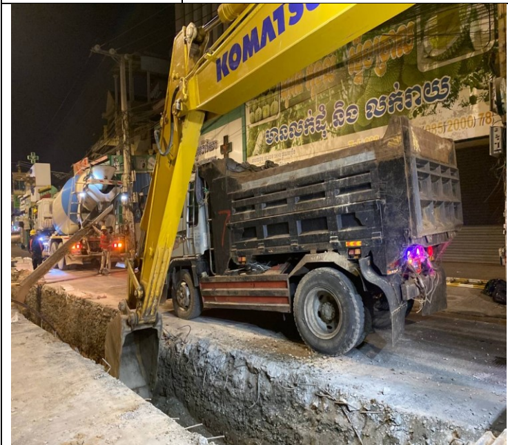
Photo: 29 Soil excavation and concrete road
