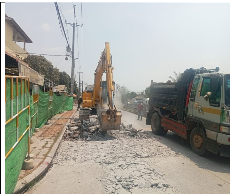
Photo: 19 Soil excavation and concrete road
