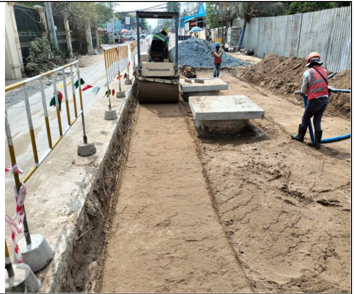
Photo: 02 | Manhole of concrete road activity
