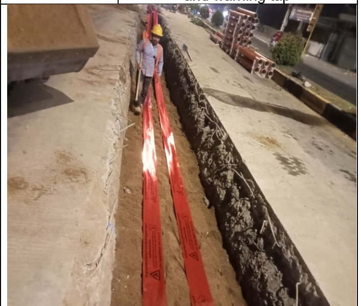
Laying concrete protection slab and warning tap
