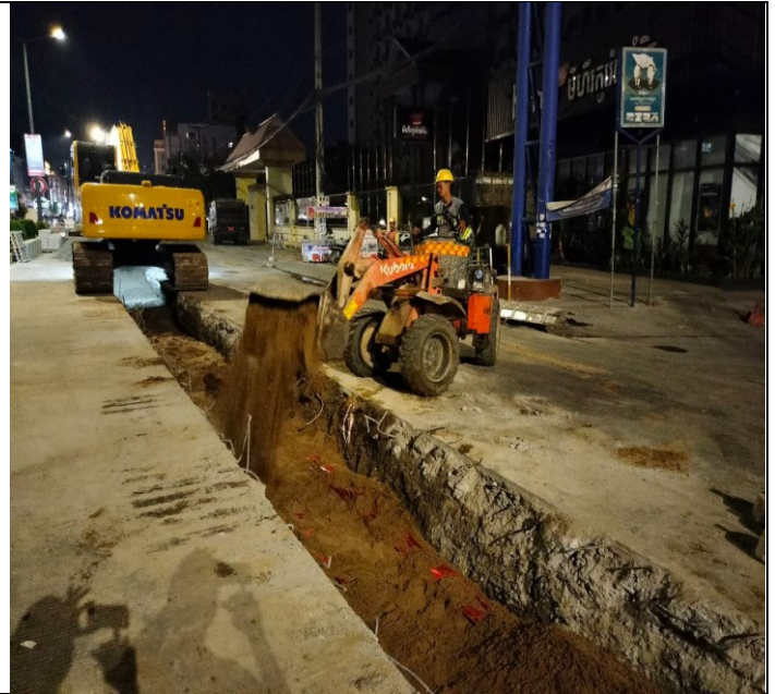
Photo: 02 Sand backfilling and compaction
