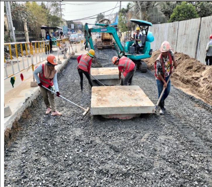
Photo: 05 | Manhole of concrete road activity
