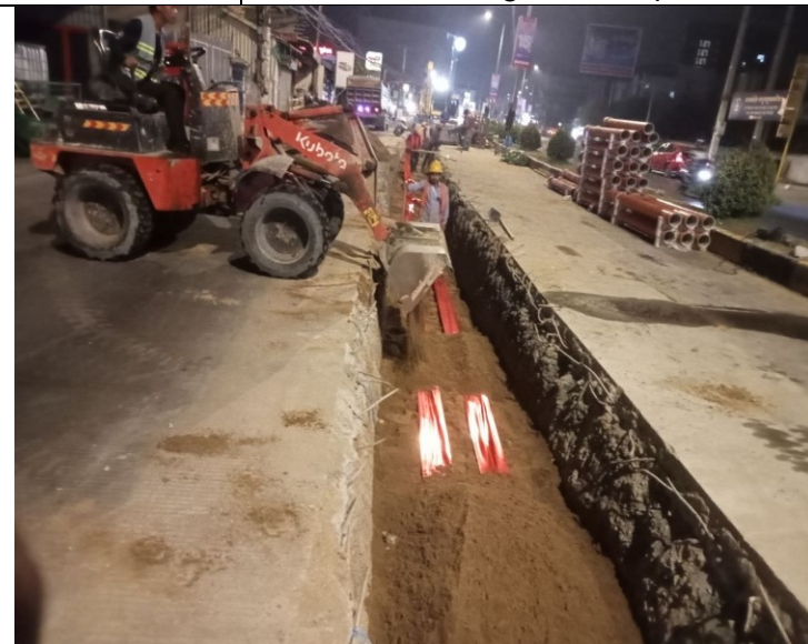
Photo: 05 Sand backfilling and compaction
