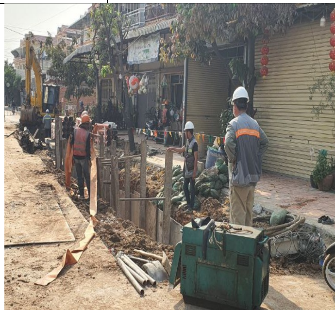
Photo: 10 Soil excavation and concrete road
