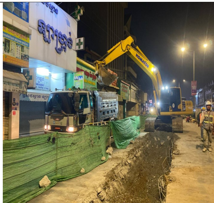
Photo: 26 Soil excavation and concrete road
