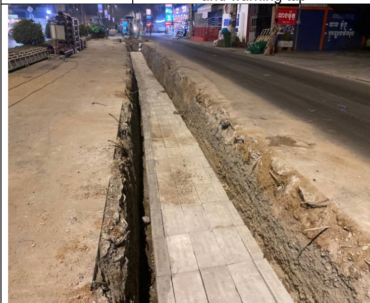
Laying concrete protection slab and warning tap
