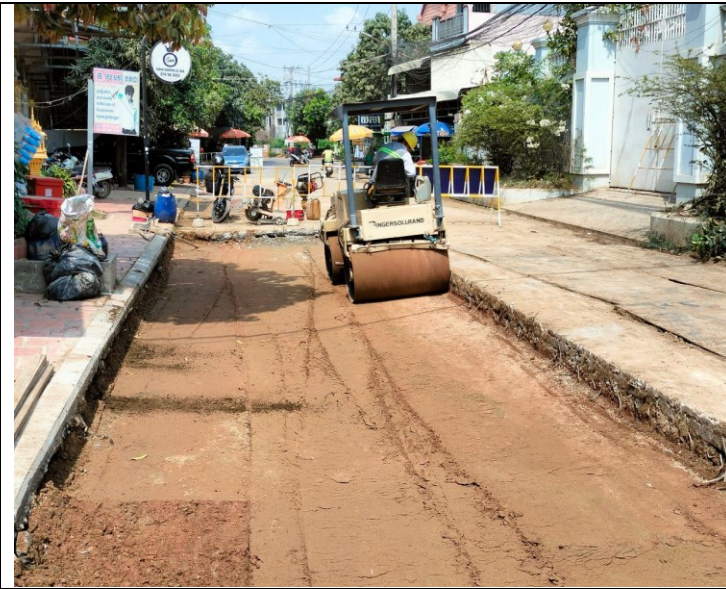
Photo: 01 | Manhole of concrete road activity
