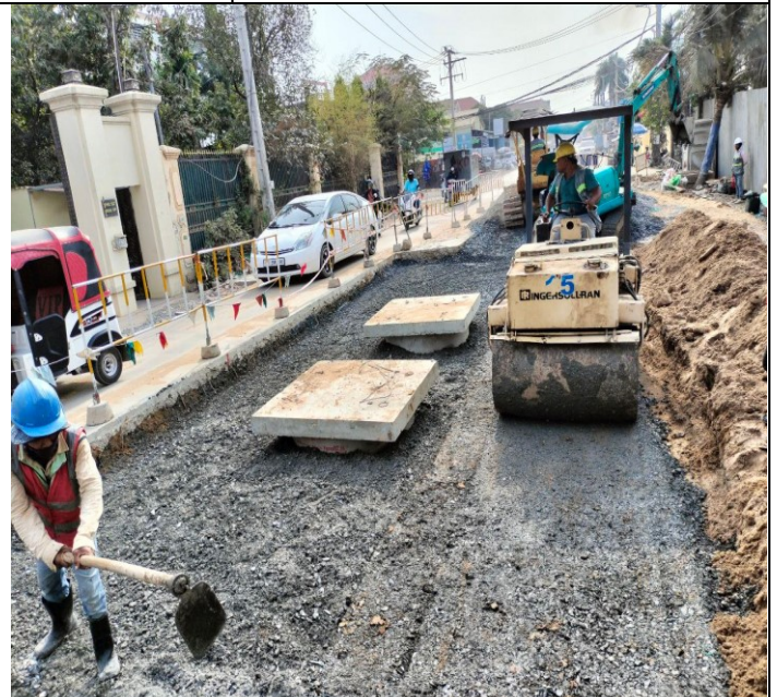
Photo: 06 | Manhole of concrete road activity
