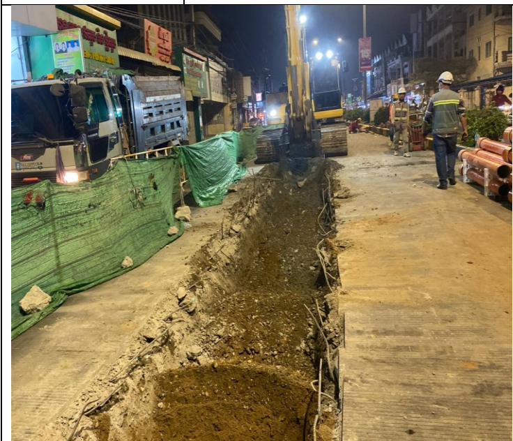
Photo: 27 Soil excavation and concrete road
