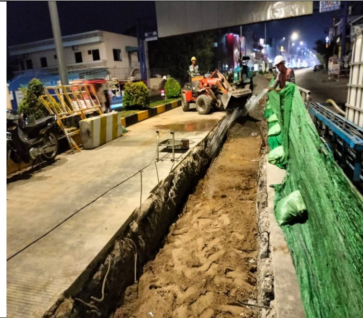
Photo: 01 Sand backfilling and compaction
