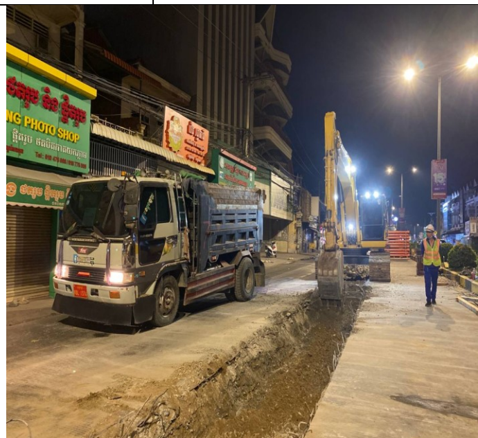
Photo: 28 Soil excavation and concrete road
