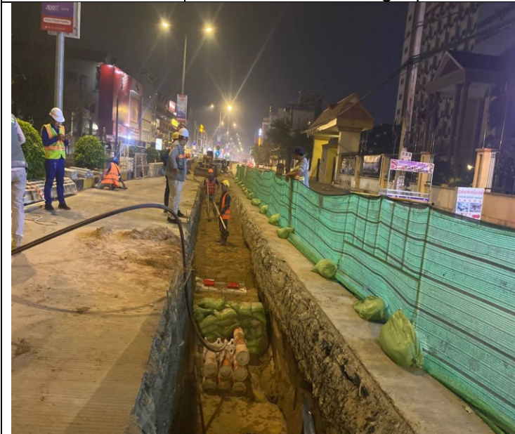
Laying concrete protection slab and warning tap
