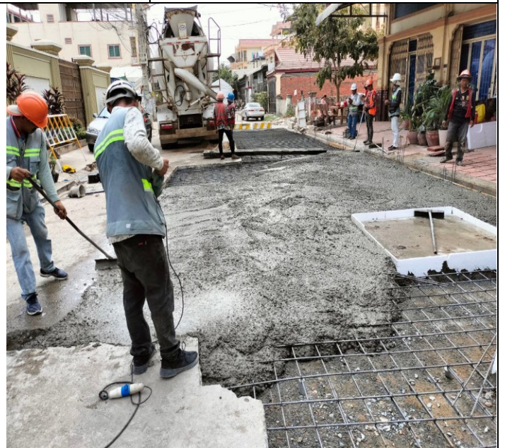
Photo: 12 Manhole of concrete road activity
