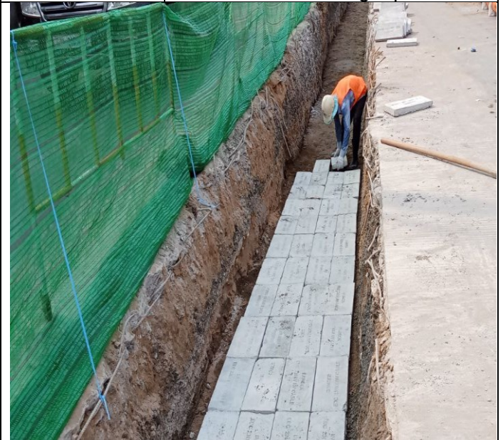
Laying concrete protection slab and warning tap
