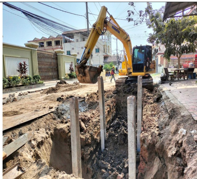
Photo: 08 Soil excavation and concrete road
