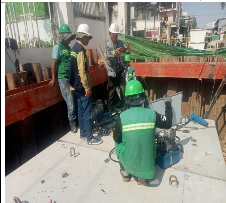
Photo: 47 Manhole Installation activity
