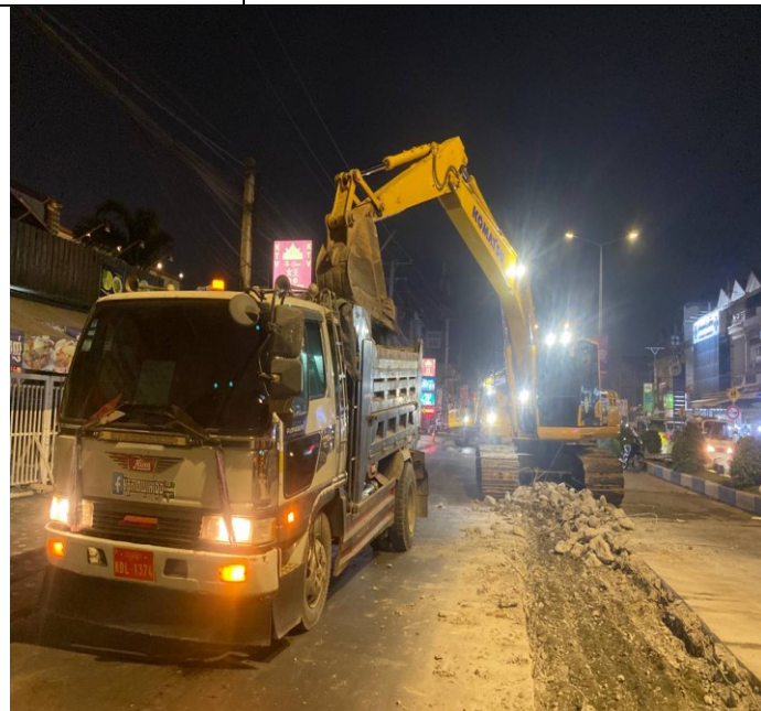
Photo: 30 Soil excavation and concrete road
