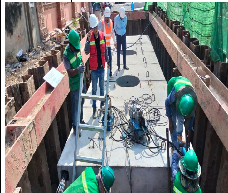
Photo: 45 Manhole Installation activity
