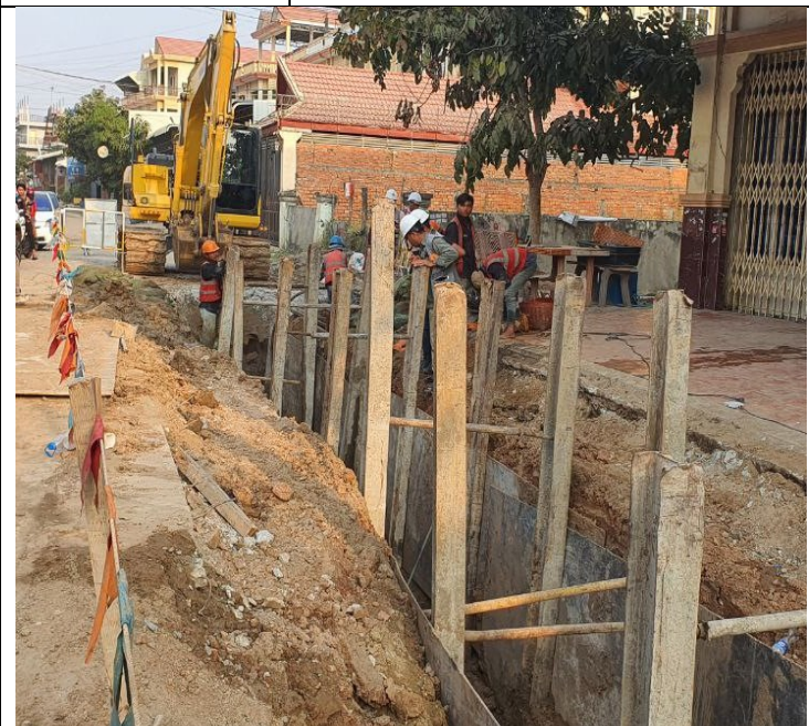
Photo: 17 Soil excavation and concrete road
