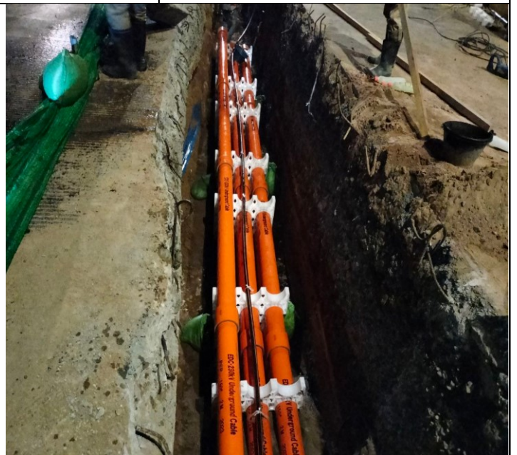
Photo: 10 Assembly PFP pipes and OFC pipe
