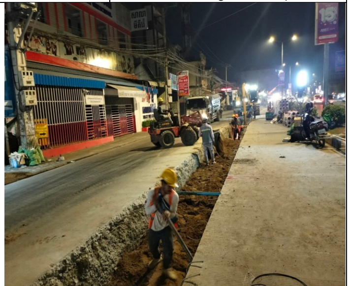
Photo: 06 Sand backfilling and compaction
