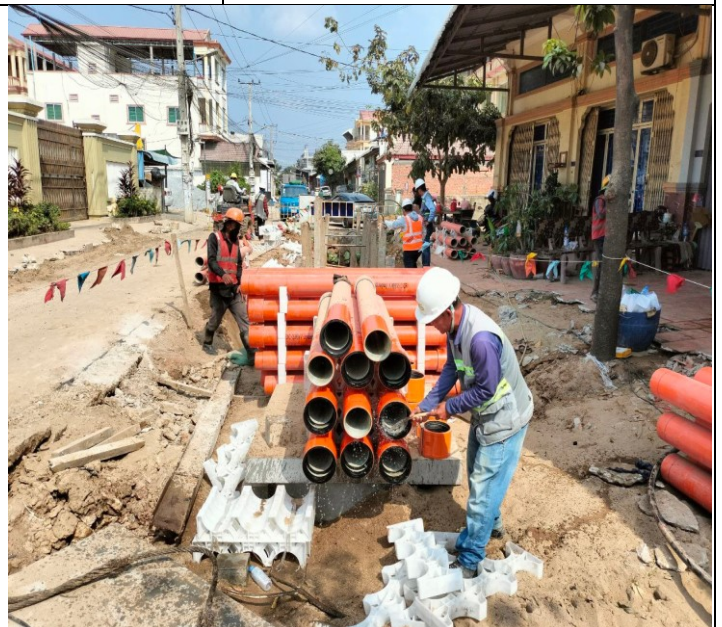
Photo: 04 Assembly PFP pipes and OFC pipe
