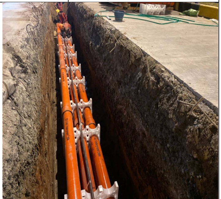
Photo: 16 Assembly PFP pipes and OFC pipe
