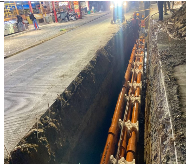
Photo: 19 Assembly PFP pipes and OFC pipe
