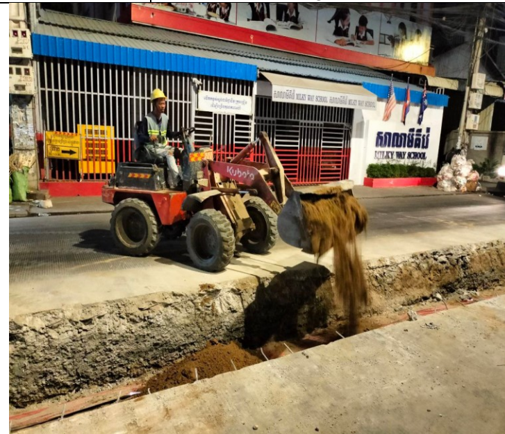
Photo: 03 Sand backfilling and compaction
