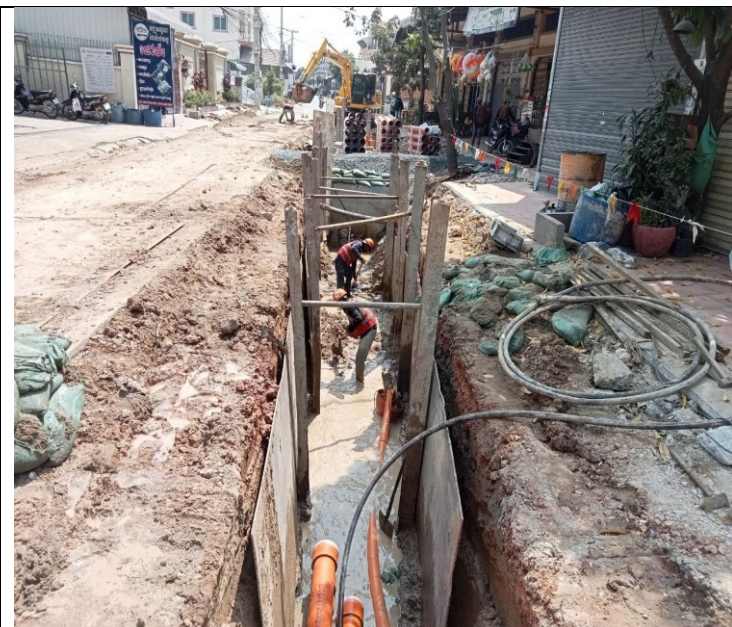
Photo: 13 Soil excavation and concrete road
