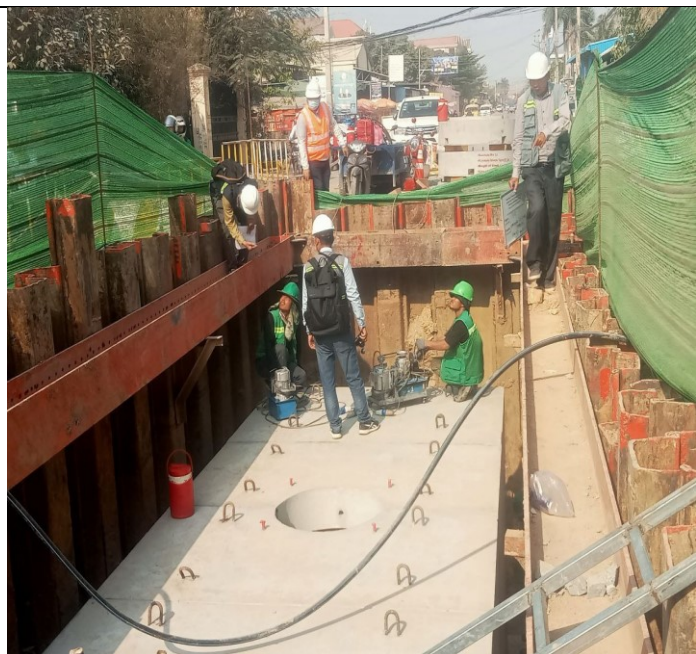
Photo: 44 Manhole Installation activity
