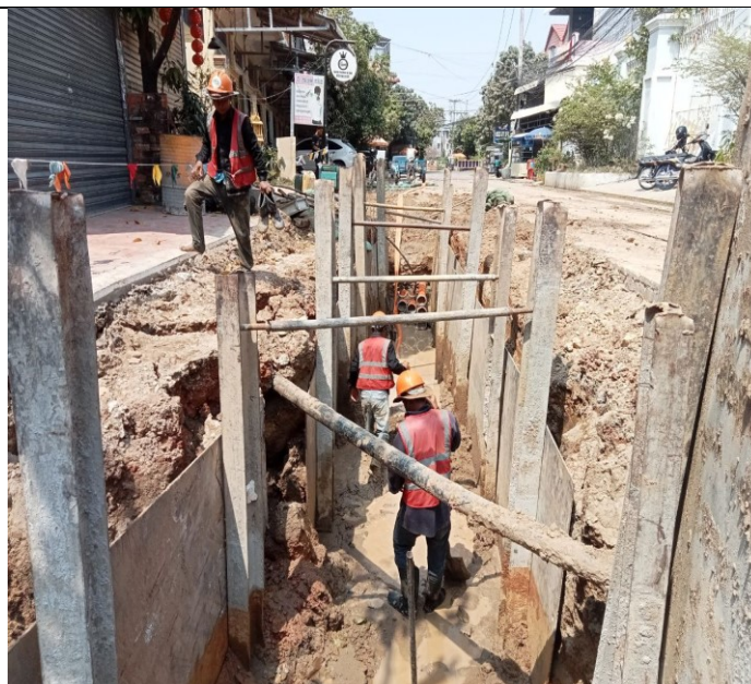
Photo: 14 Soil excavation and concrete road
