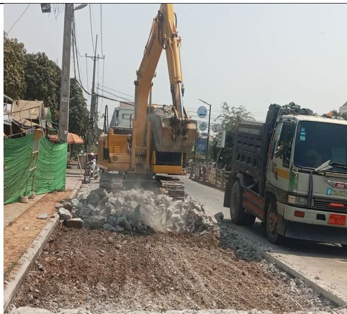
Photo: 20 Soil excavation and concrete road
