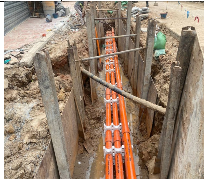
Photo: 03 Assembly PFP pipes and OFC pipe
