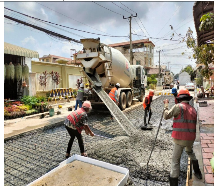
Photo: 11 Manhole of concrete road activity
