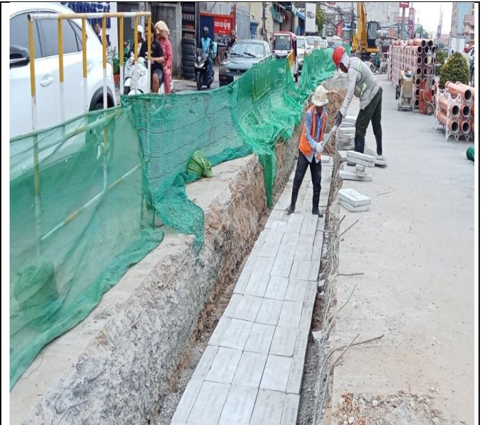
Laying concrete protection slab and warning tap
