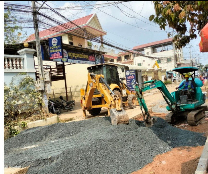
Photo: 03 | Manhole of concrete road activity
