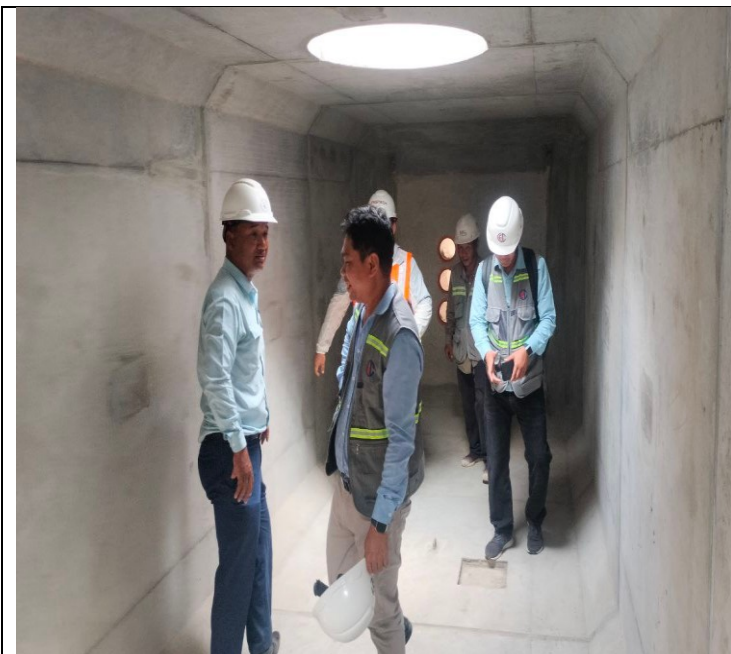
Photo: 43 Manhole Installation activity
