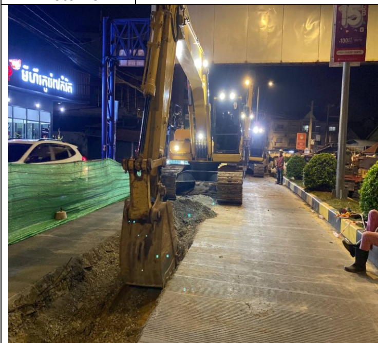
Photo: 21 Soil excavation and concrete road
