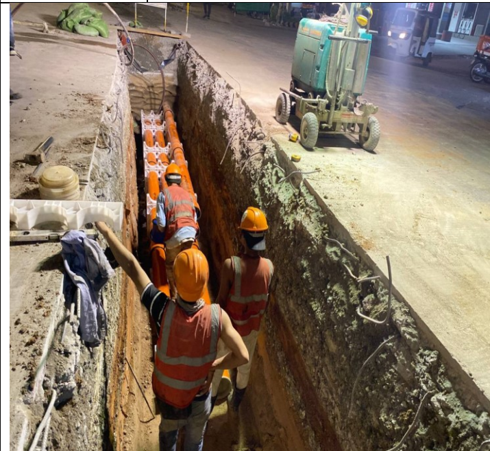
Photo: 23 Assembly PFP pipes and OFC pipe
