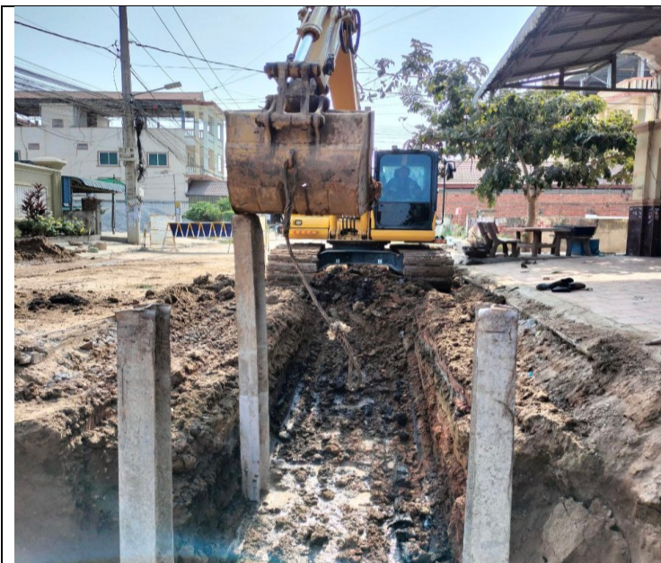
Photo: 07 Soil excavation and concrete road
