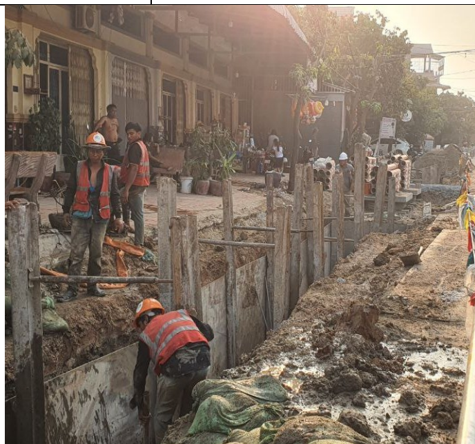
Photo: 16 Soil excavation and concrete road
