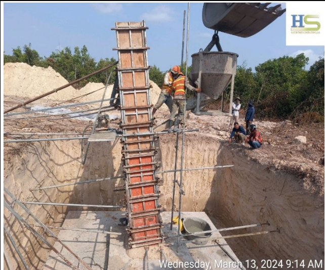
Casting concrete chimney leg C.
