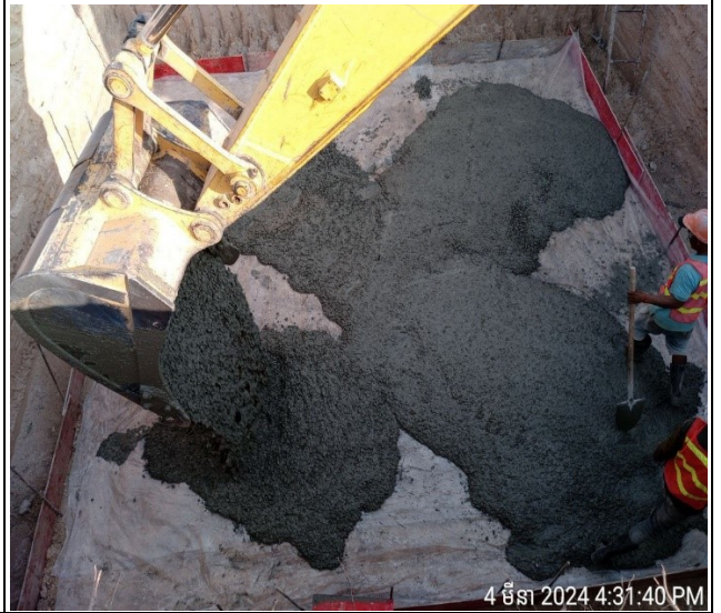
Lean casting concrete B.
