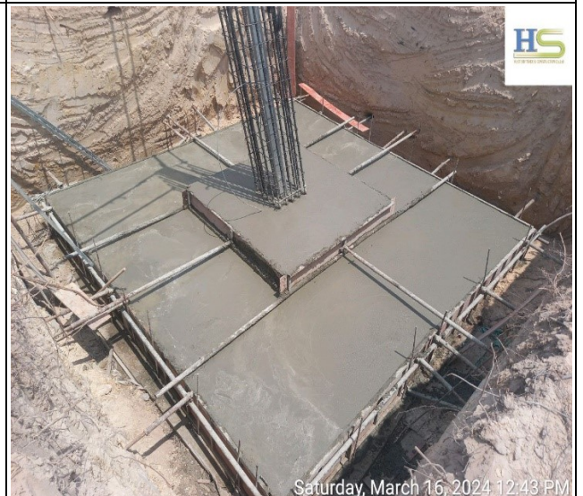
Casting concrete base of the leg D.
