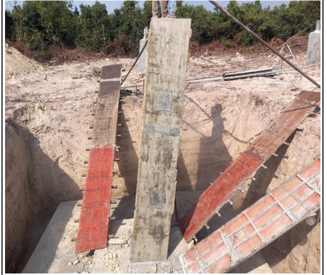
Remove formwork chimney leg A.
