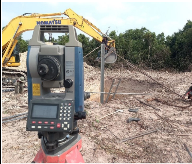
Stub setting of the leg A.
