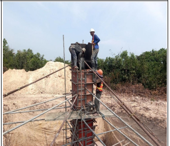
Chimney casting concrete of the leg A.
