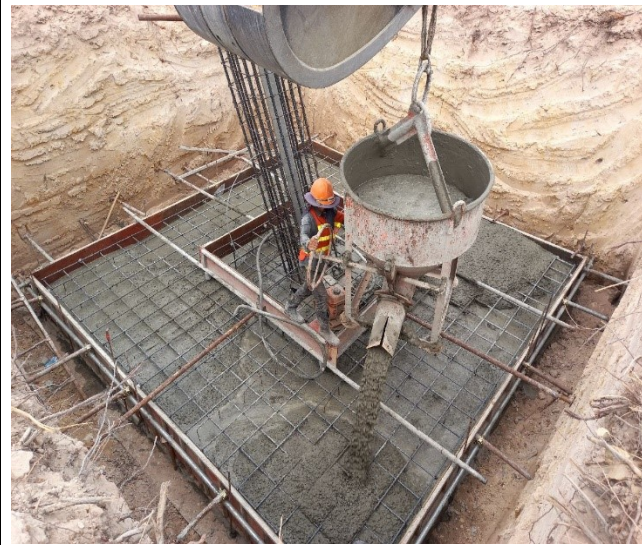
Base casting concrete of the leg A.
