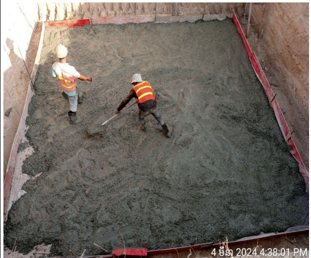
Lean casting concrete B.
