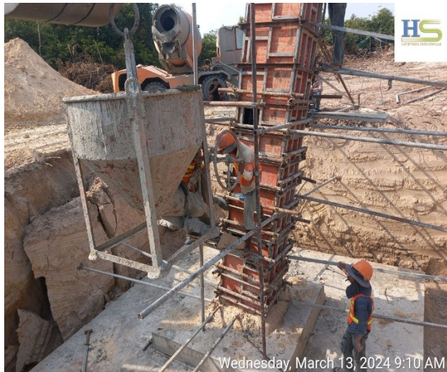
Chimney casting concrete of the leg B.
