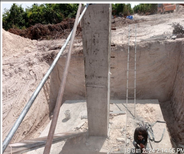
Remove formwork chimney leg B.
