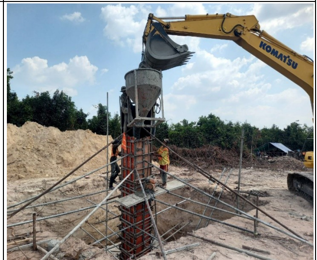
Casting concrete chimney leg D.
