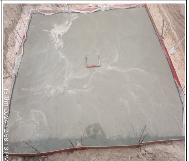
Lean casting concrete of the leg D.
