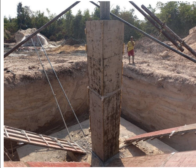
Remove formwork chimney leg A.
