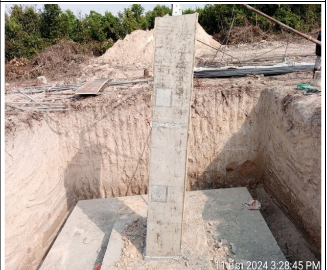
Remove formwork chimney leg D.
