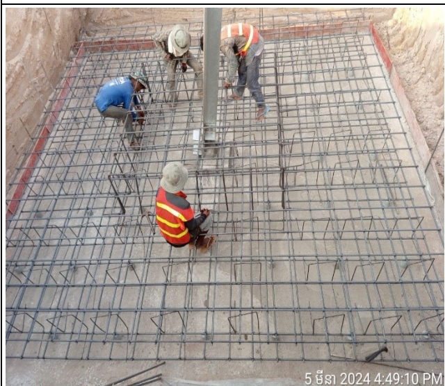
Rebar arrangement of the leg A.
