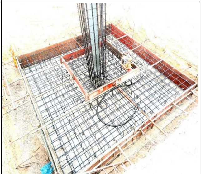
Formwork installation of the leg A.
