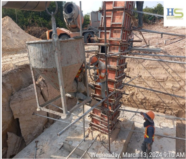
Casting concrete chimney leg C.
