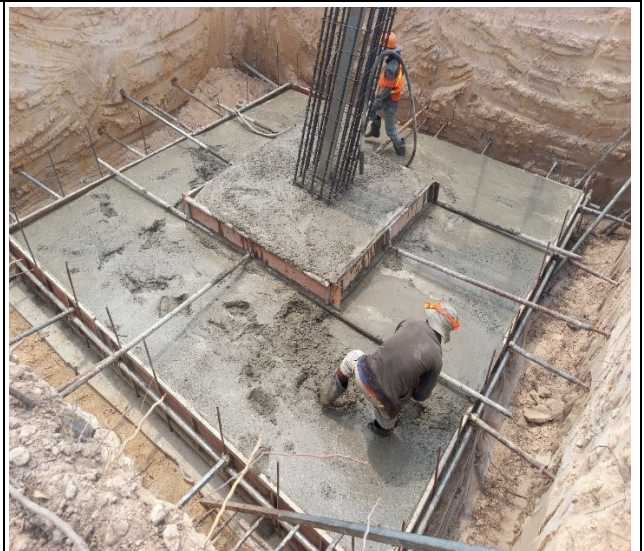
Base casting concrete of the leg B.
