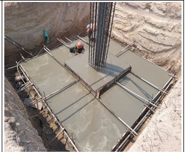
Casting concrete base of the leg C.
