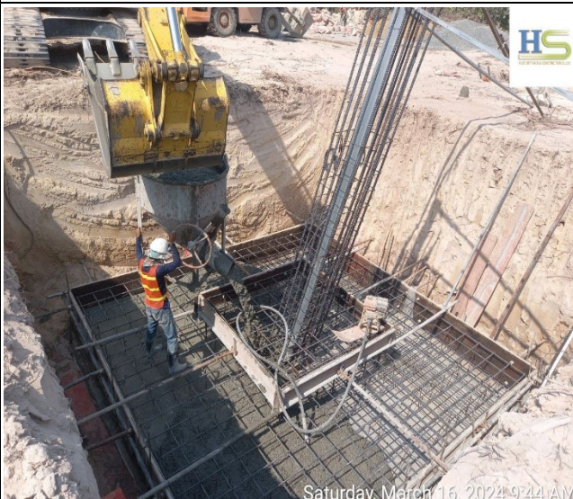
Casting concrete base of the leg D.
