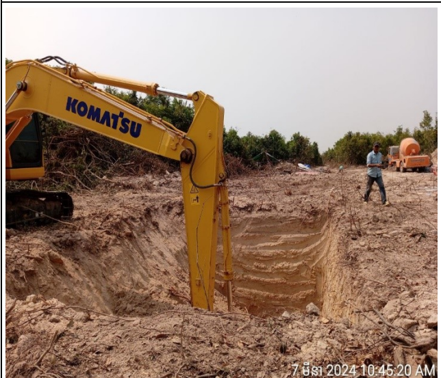
Soil excavation of the leg A.
