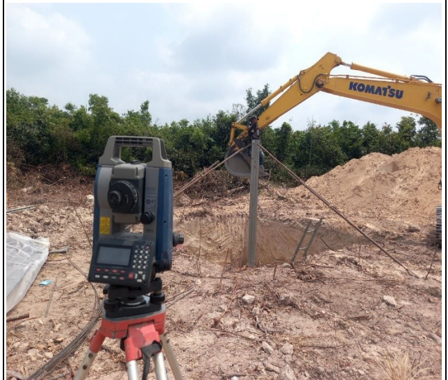
Stub setting of the leg B.
