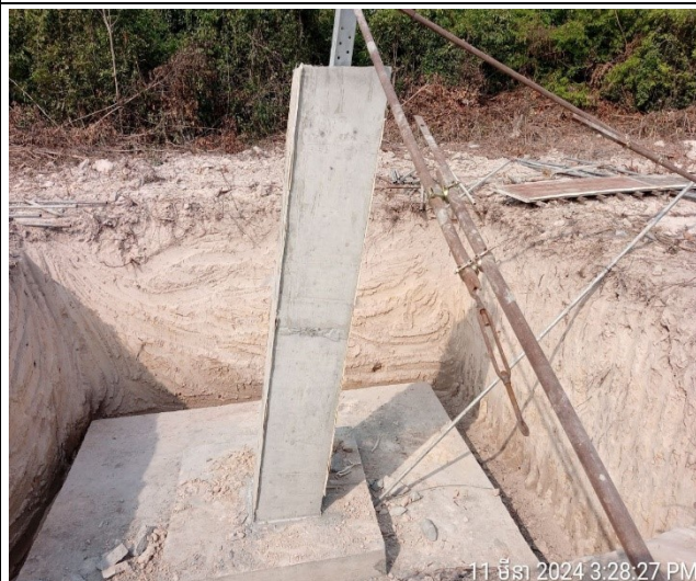
Remove formwork chimney leg D.
