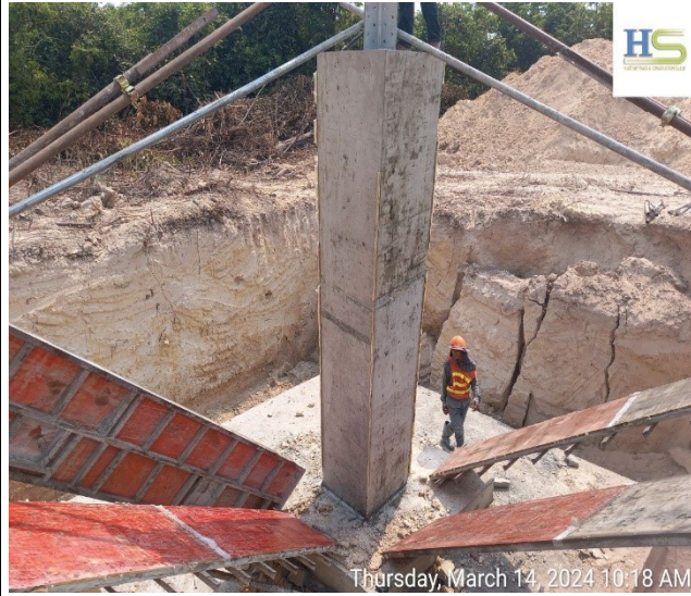
Remove formwork chimney leg C
