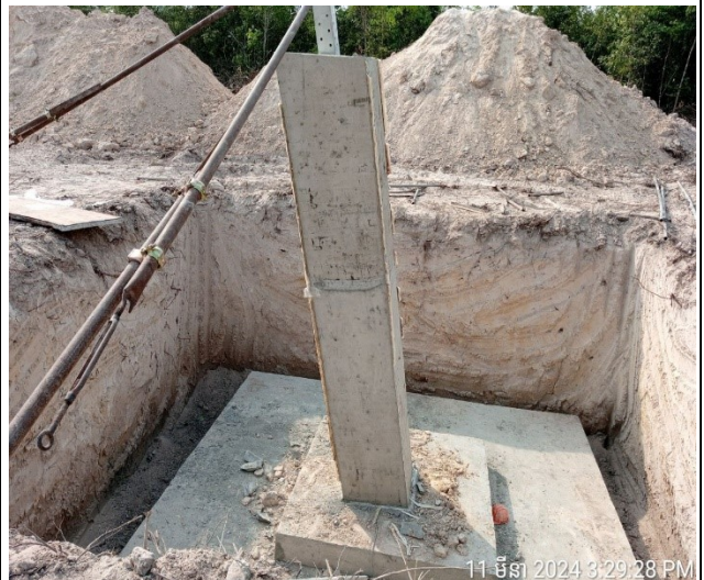
Remove formwork chimney leg D.
