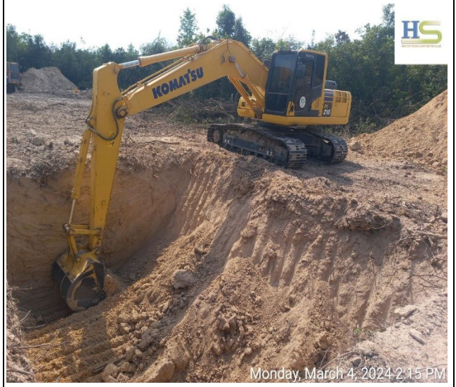
Soil excavation of the leg B
