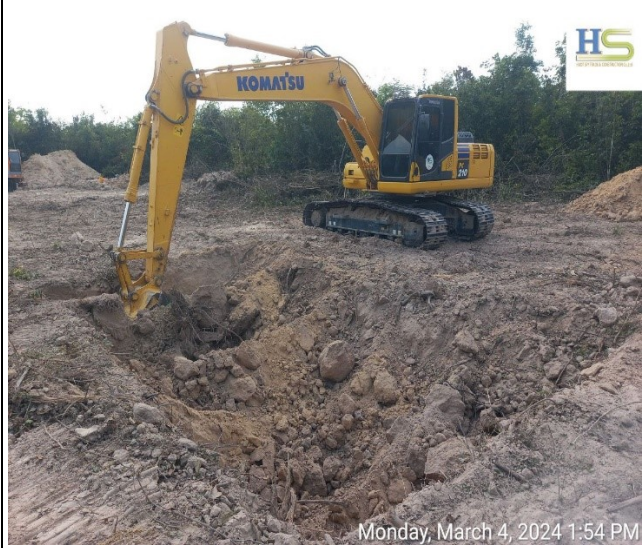
Soil excavation of the leg B
