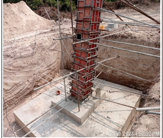
Chimney formwork installation of the leg B.
