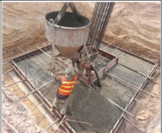
Base casting concrete of the leg B.
