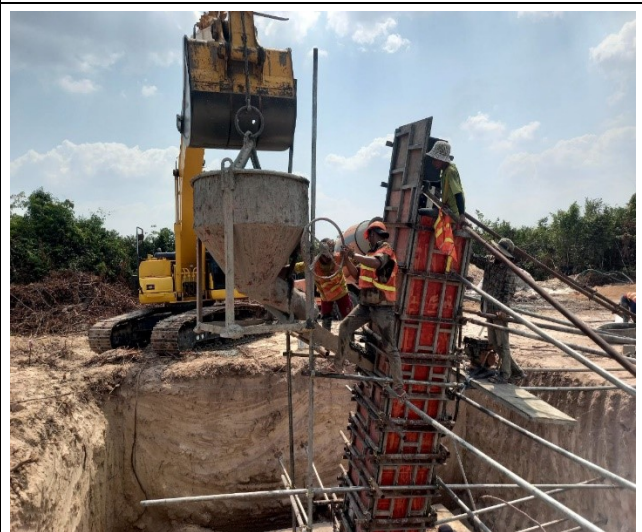
Casting concrete chimney leg D.
