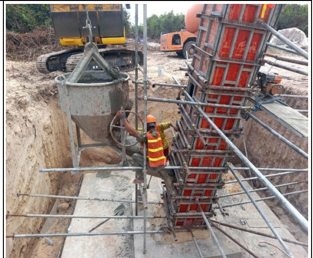
Chimney casting concrete of the leg D.
