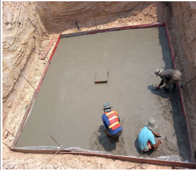
Lean casting concrete C.
