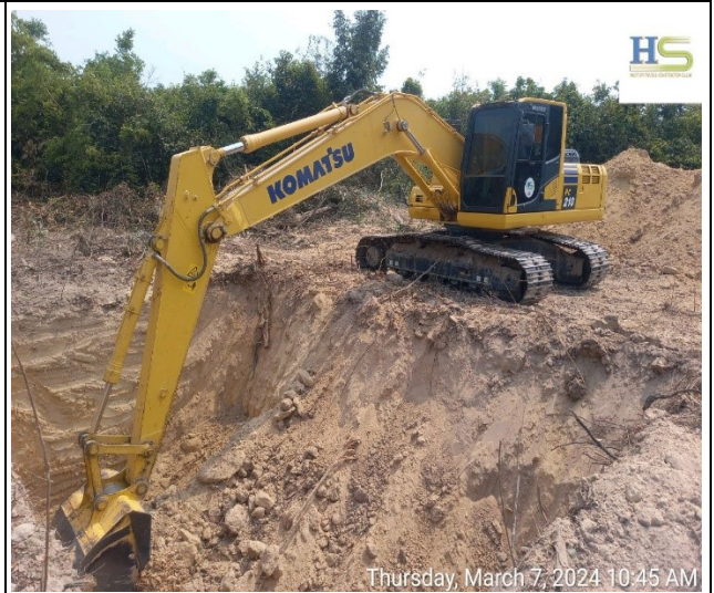
Soil excavation of the leg C.
