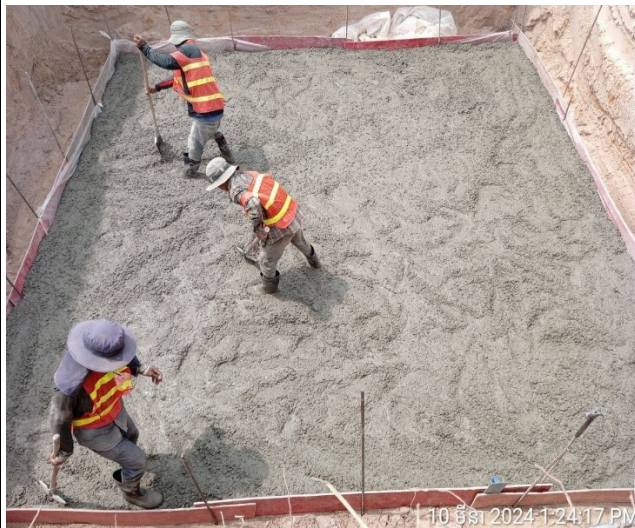
Lean casting concrete of the leg A.
