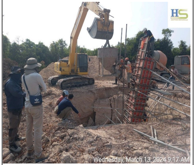
Casting concrete chimney leg C.
