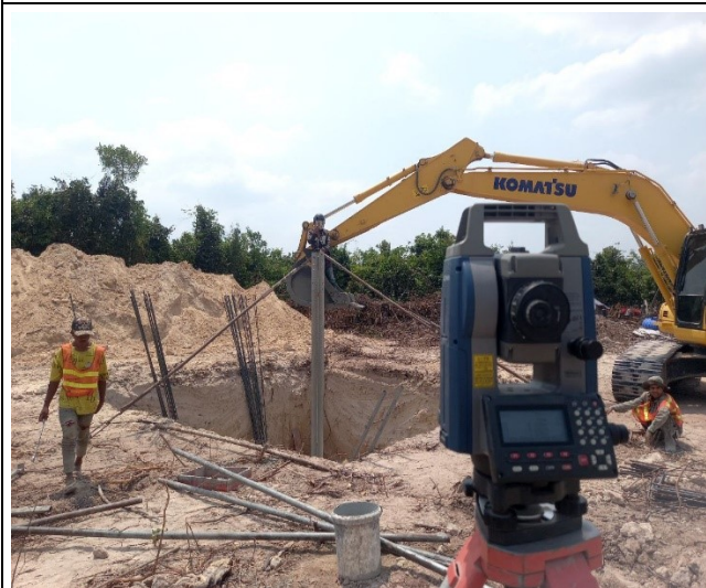
Stub setting of the leg C.
