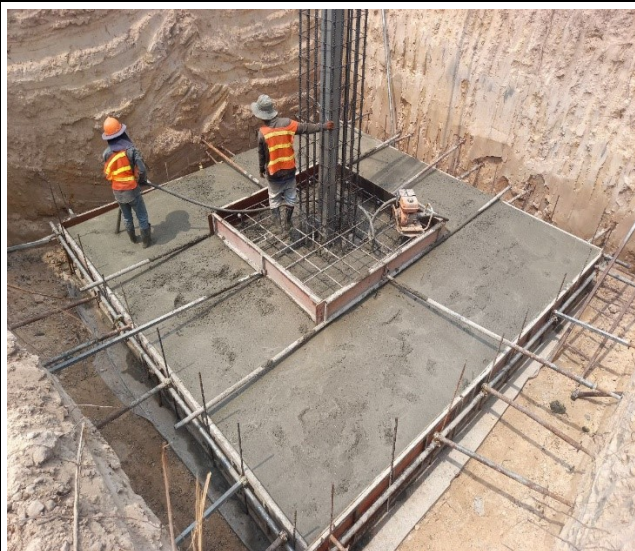
Base casting concrete of the leg B.
