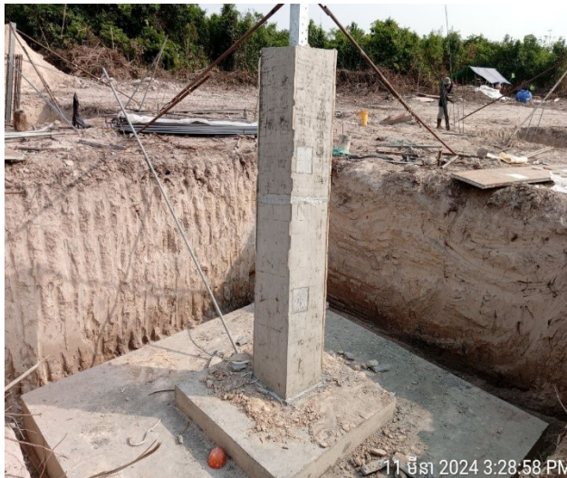
Remove formwork chimney leg D.
