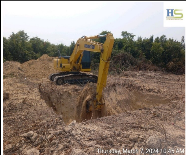
Soil excavation of the leg C.
