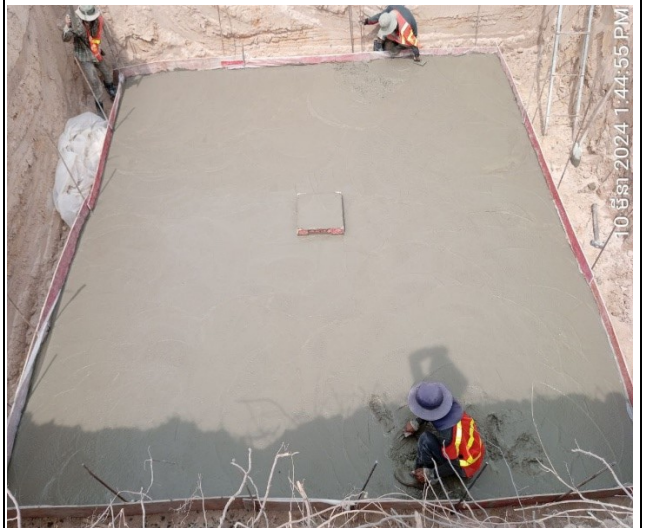
Lean casting concrete of the leg A.
