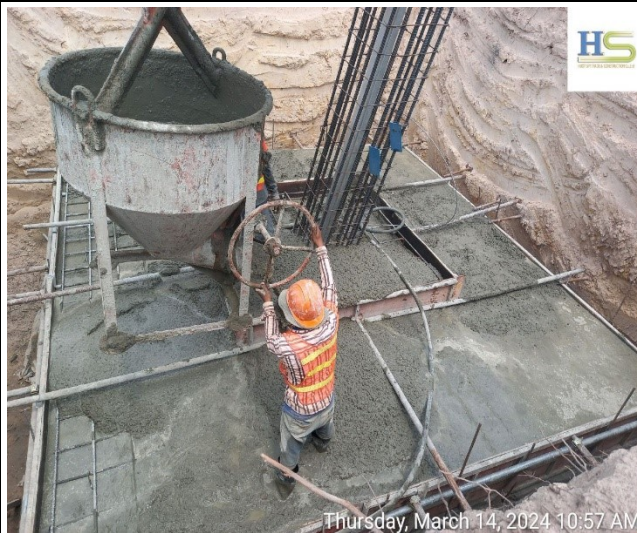
Casting concrete base of the leg C.
