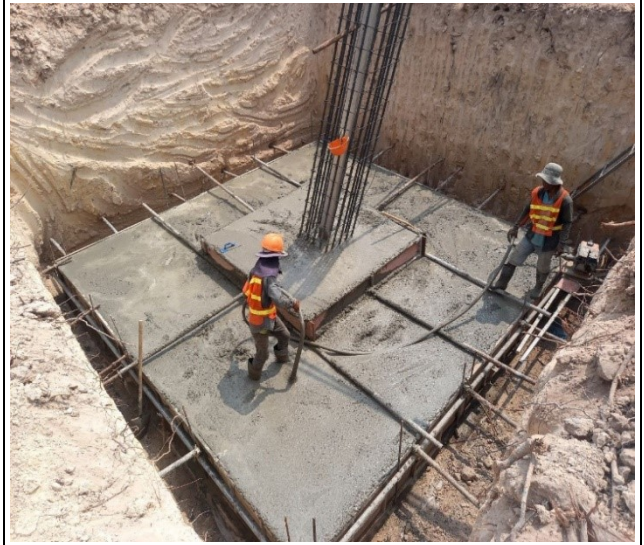
Base casting concrete of the leg A.
