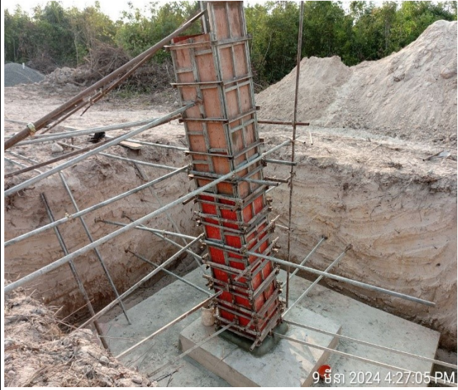
Chimney formwork installation of the leg A.
