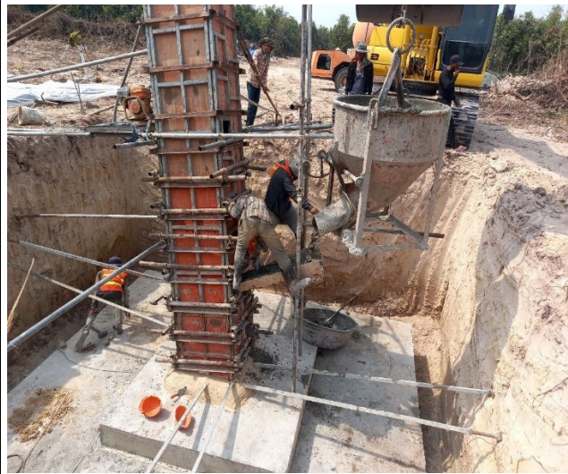
Chimney casting concrete of the leg A.
