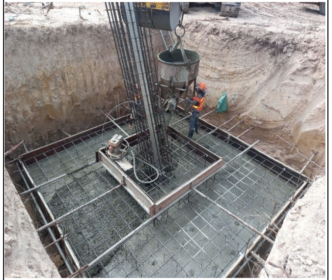
Casting concrete base of the leg C.
