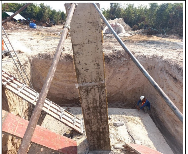
Remove formwork chimney leg A.
