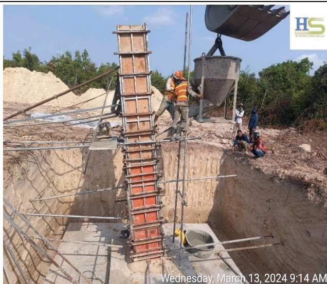
Chimney casting concrete of the leg B.
