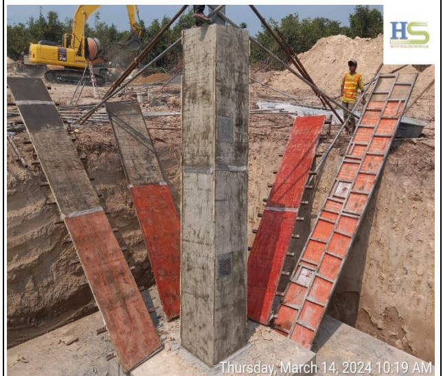
Remove formwork chimney leg C
