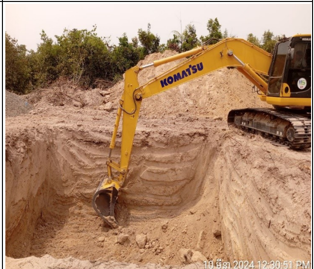
Soil excavation of the leg A.
