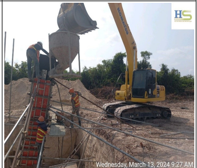
Chimney casting concrete of the leg B.
