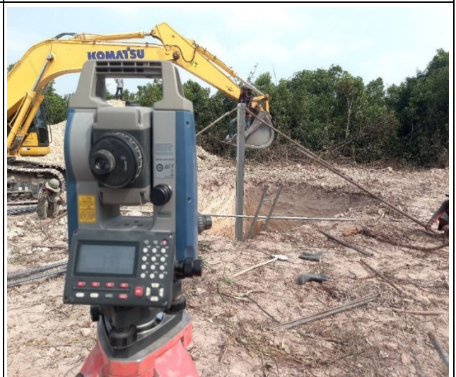
Stub setting of the leg D.
