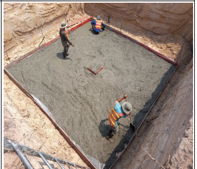
Lean casting concrete C.
