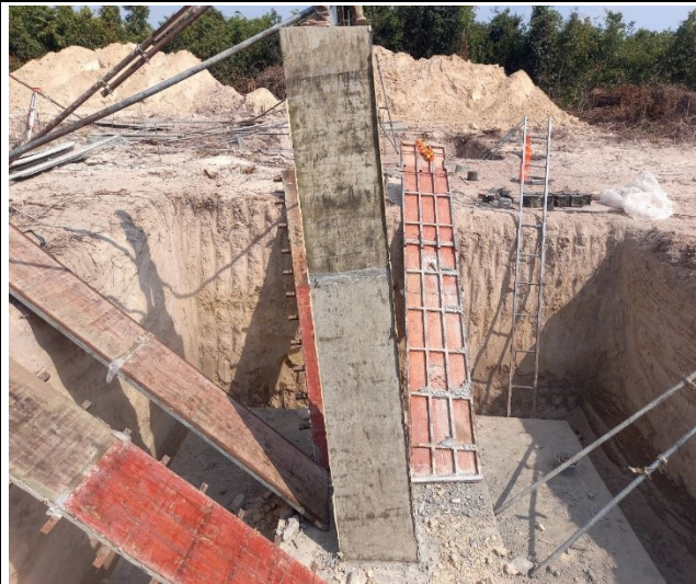
Remove formwork chimney leg A.
