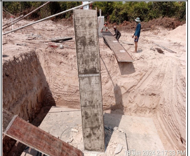
Remove formwork chimney leg B.
