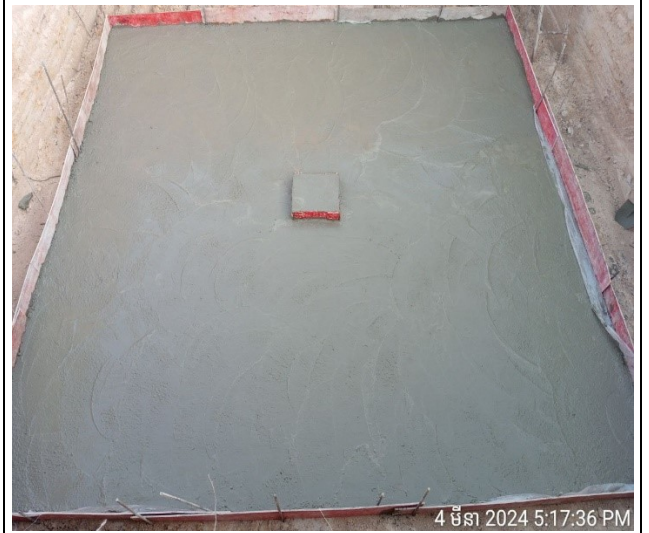
Lean casting concrete B.
