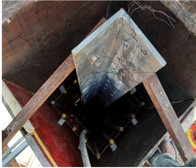
Chimney formwork installation of the leg B.
