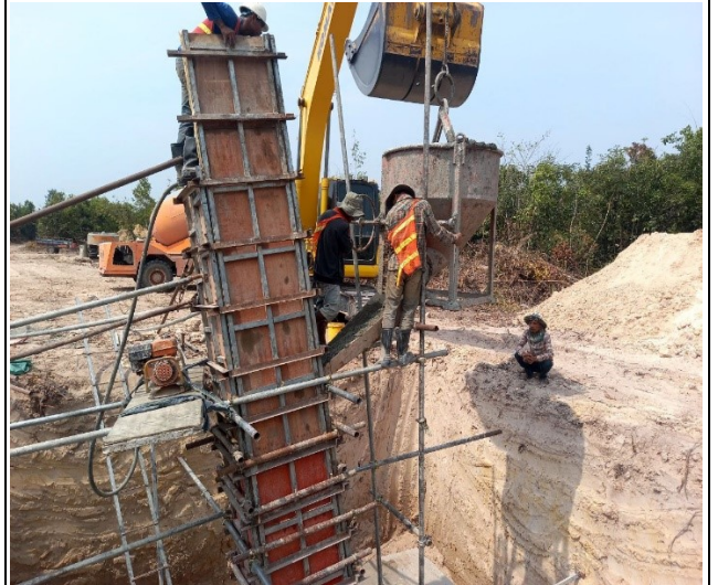
Chimney casting concrete of the leg A.
