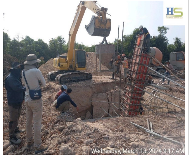
Chimney casting concrete of the leg B.
