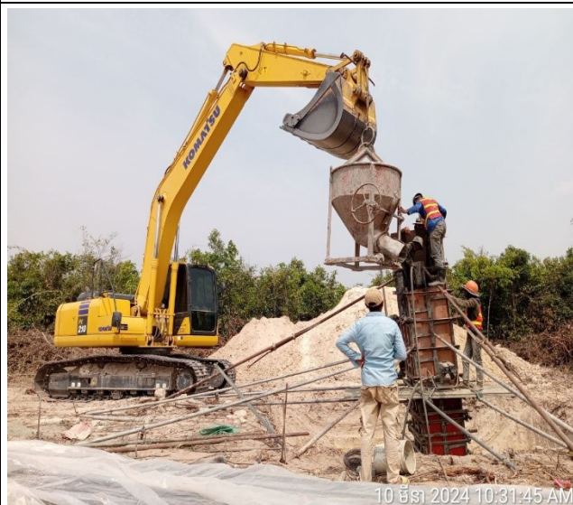
Chimney casting concrete of the leg A.
