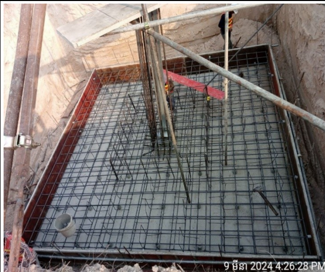
Base casting concrete of the leg B.
