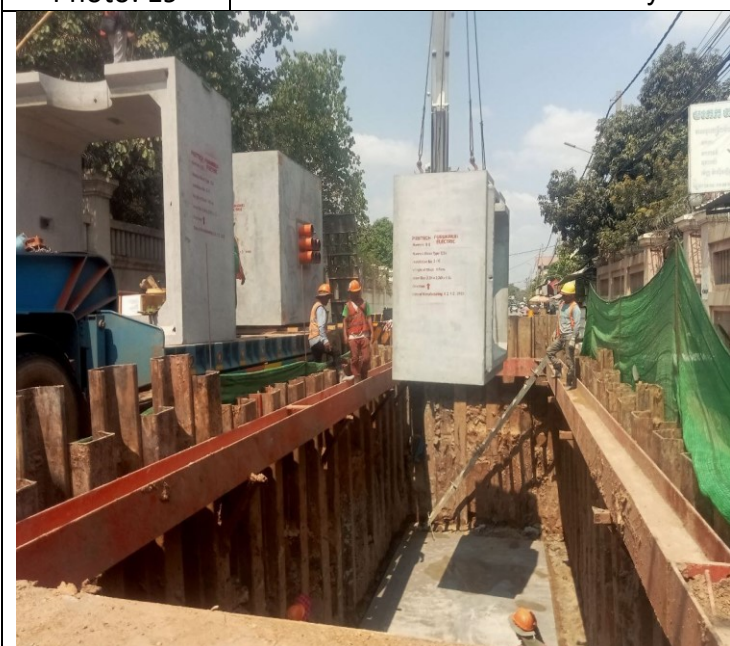
Photo: 21 Manhole Installation activity
