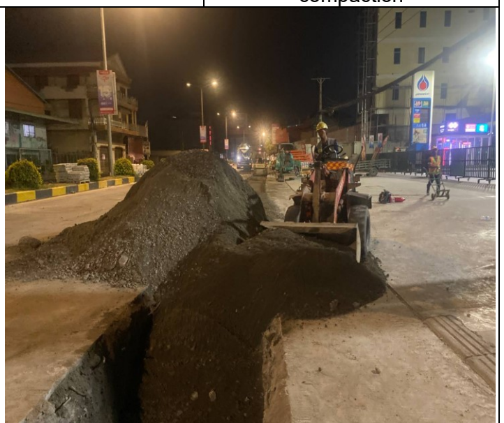
Base course backfilling and compaction
