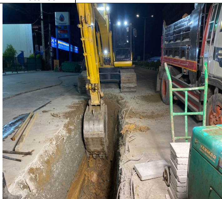
Photo: 10 Soil excavation and concrete road
