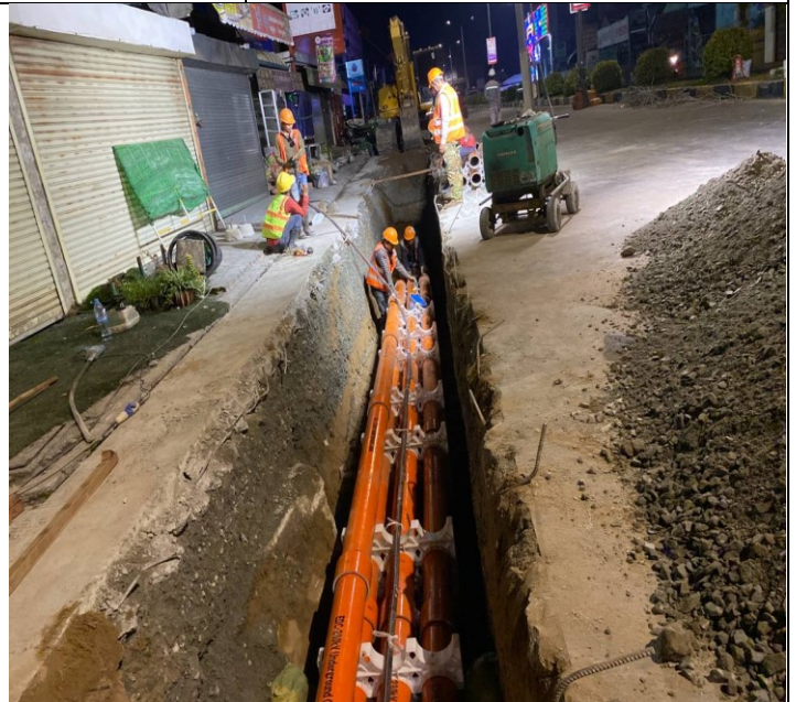
Photo: 18 Assembly PFP pipes and OFC pipe
