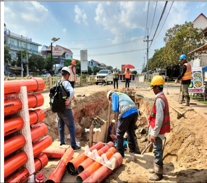
Photo: 13 Assembly PFP pipes and OFC pipe
