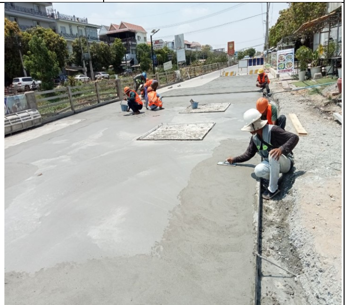
Photo: 22 Manhole of concrete road activity
