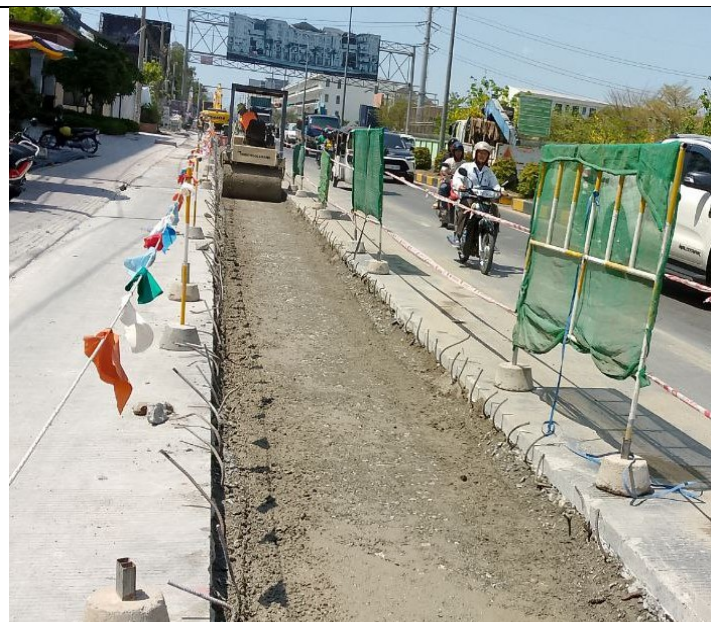
Base course backfilling and compaction
