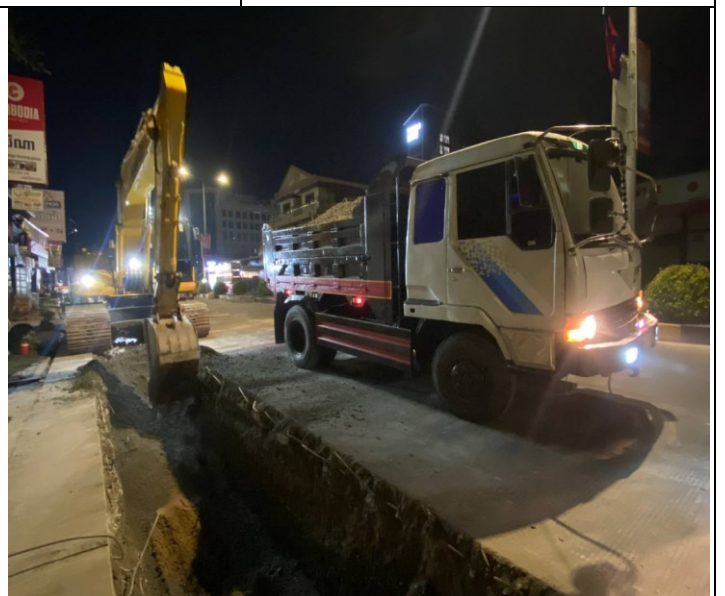
Photo: 06 Soil excavation and concrete road
