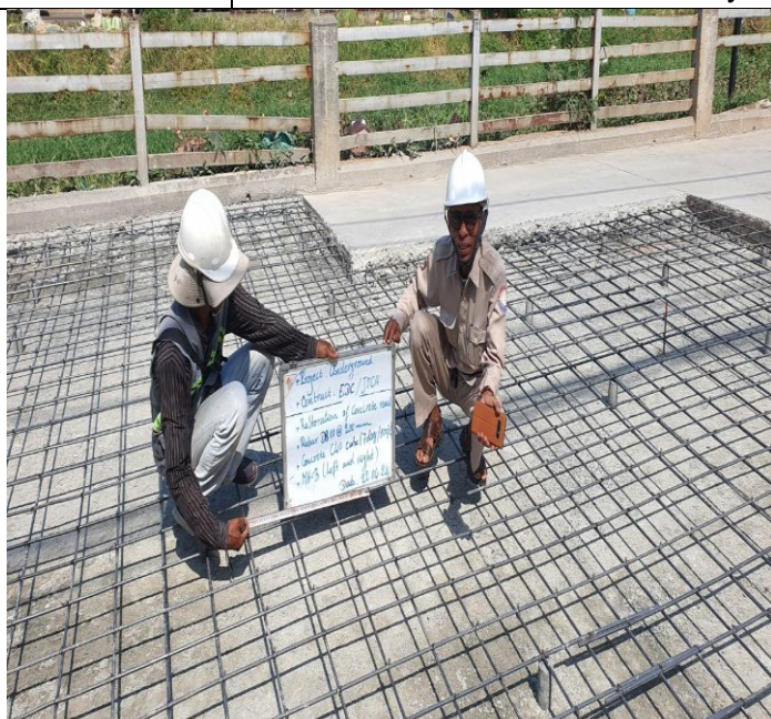
Photo: 10 Manhole of concrete road activity
