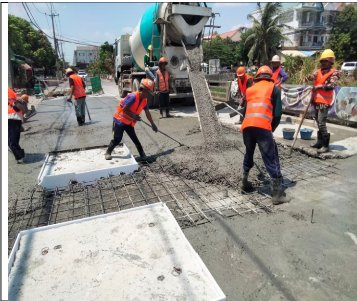
Photo: 19 Manhole of concrete road activity
