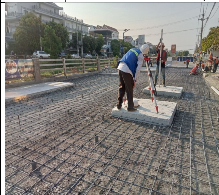
Photo: 09 Manhole of concrete road activity
