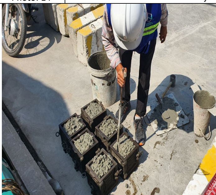
Photo: 16 Manhole of concrete road activity
