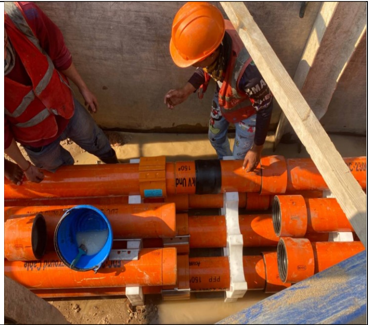
Photo: 14 Assembly PFP pipes and OFC pipe
