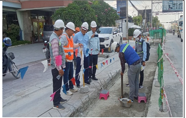
Photo: 02 Plate test of compaction road
