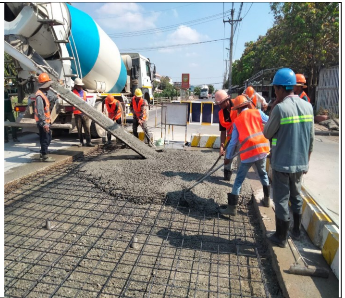
Photo: 20 Manhole of concrete road activity
