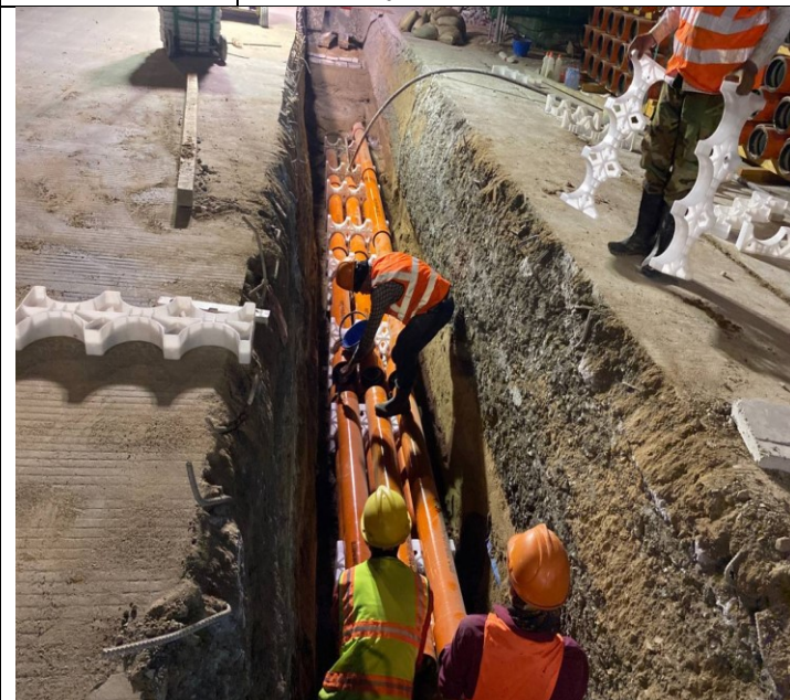
Photo: 27 Assembly PFP pipes and OFC pipe
