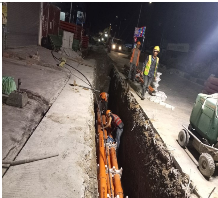
Photo: 26 Assembly PFP pipes and OFC pipe
