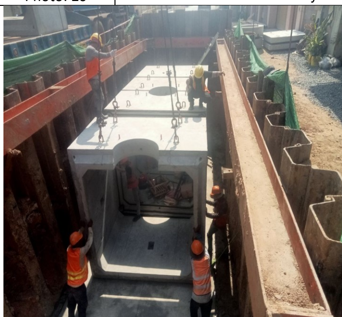
Photo: 22 Manhole Installation activity
