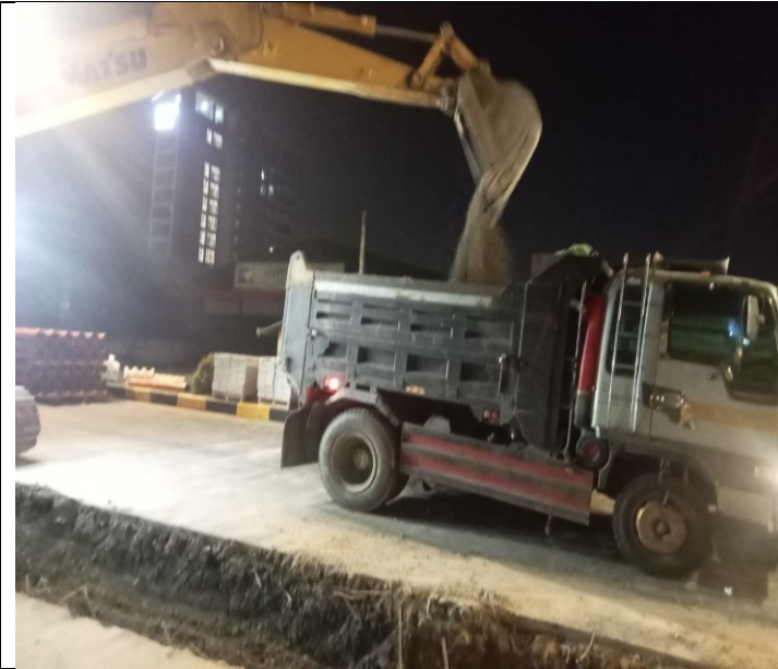
Photo: 01 Soil excavation and concrete road
