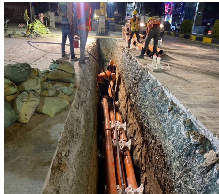
Photo: 29 Assembly PFP pipes and OFC pipe
