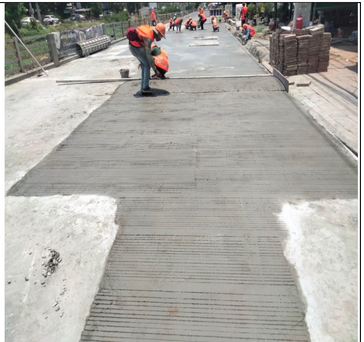
Photo: 26 Manhole of concrete road activity
