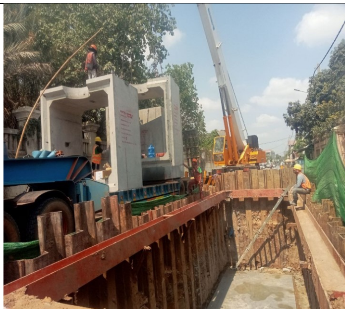
Photo: 20 Manhole Installation activity
