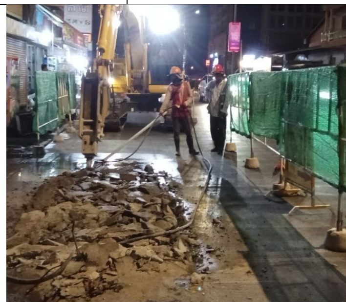
Demolition of concrete road
