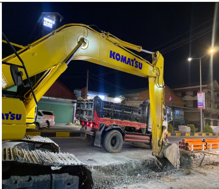
Photo: 14 Soil excavation and concrete road
