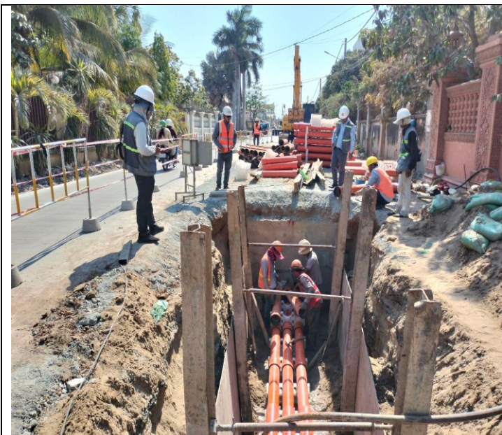
Photo: 19 Assembly PFP pipes and OFC pipe
