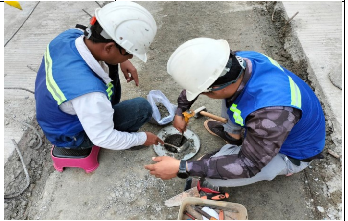
Photo: 06 Plate test of compaction road
