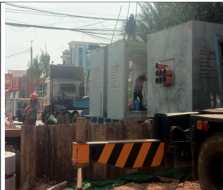
Photo: 19 Manhole Installation activity
