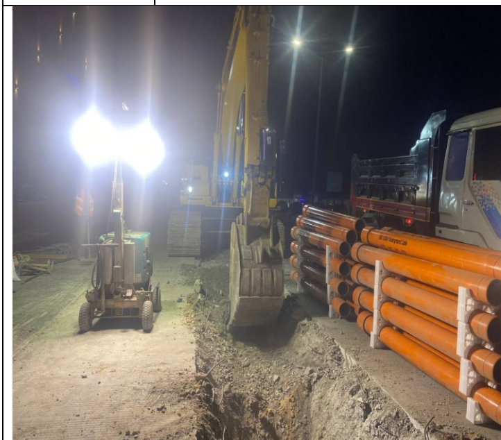
Photo: 17 Soil excavation and concrete road
