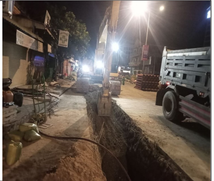
Photo: 02 Soil excavation and concrete road
