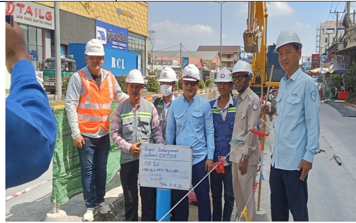
Photo: 05 Plate test of compaction road
