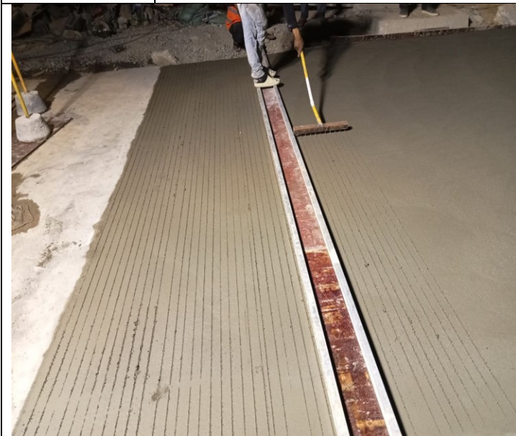
Photo: 27 Manhole of concrete road activity
