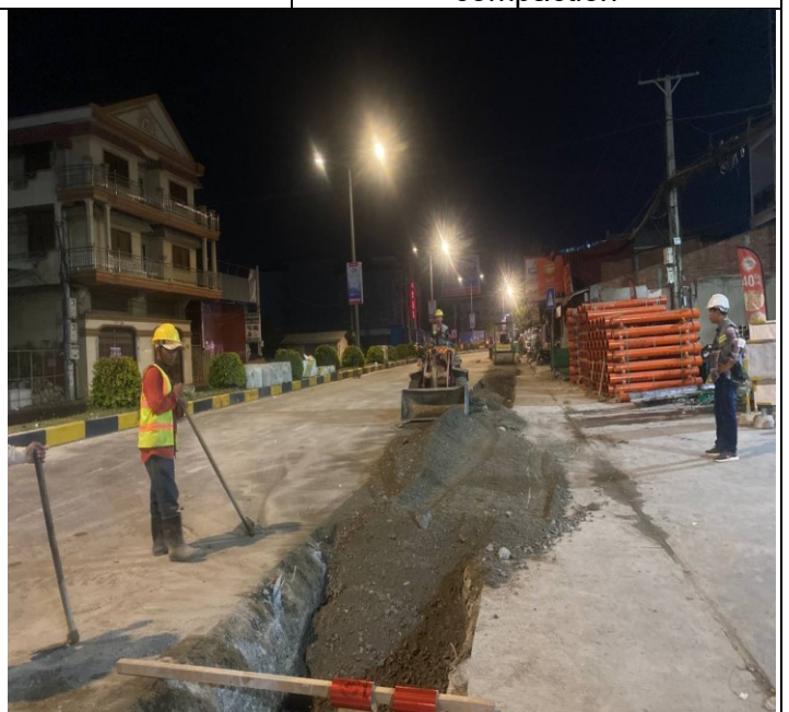
Base course backfilling and compaction
