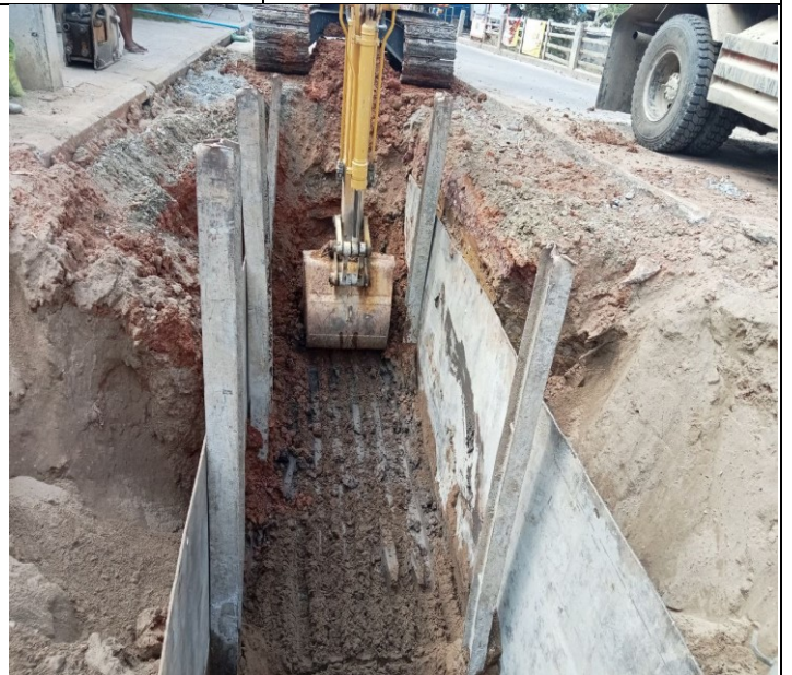
Photo: 04 Soil excavation and concrete road
