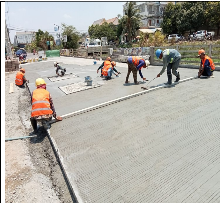
Photo: 25 Manhole of concrete road activity
