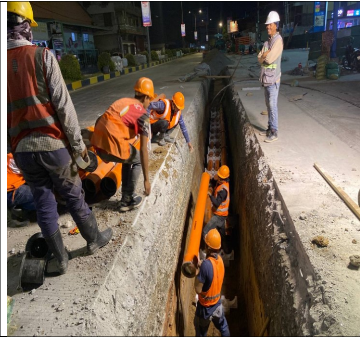
Photo: 31 Assembly PFP pipes and OFC pipe
