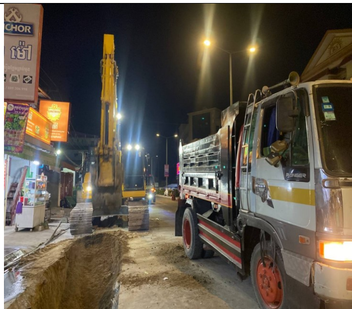
Photo: 08 Soil excavation and concrete road
