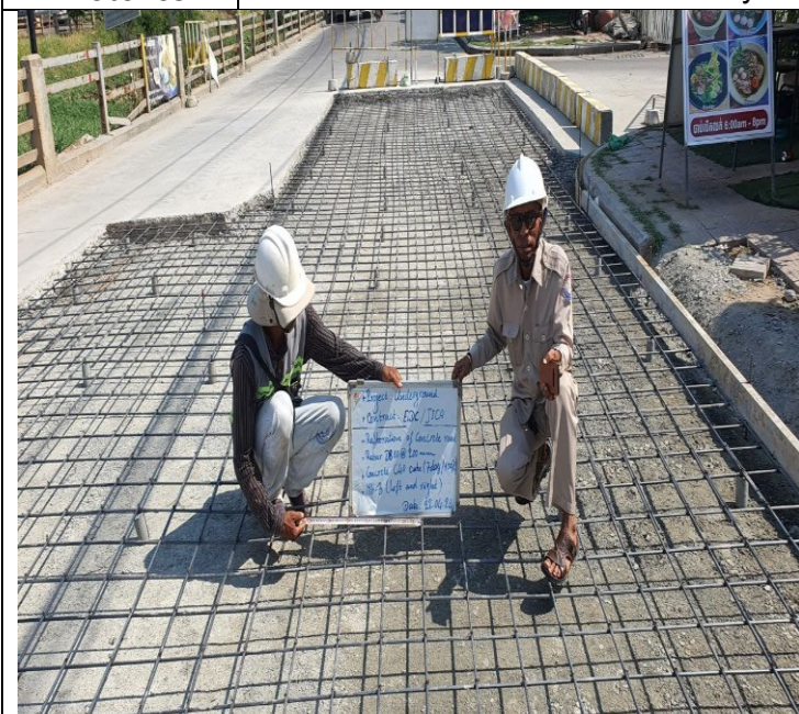
Photo: 11 Manhole of concrete road activity
