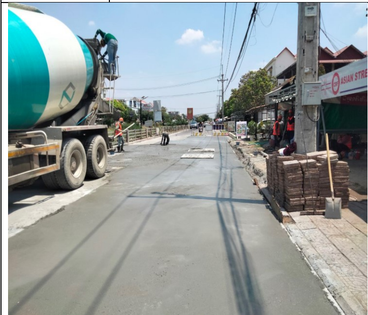
Photo: 21 Manhole of concrete road activity
