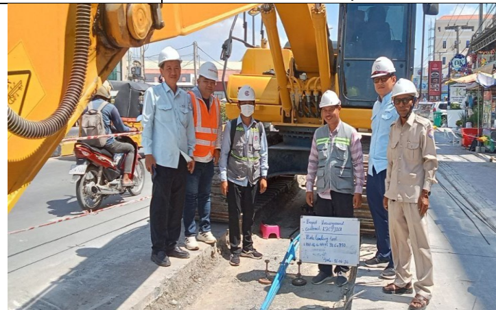
Photo: 07 Plate test of compaction road
