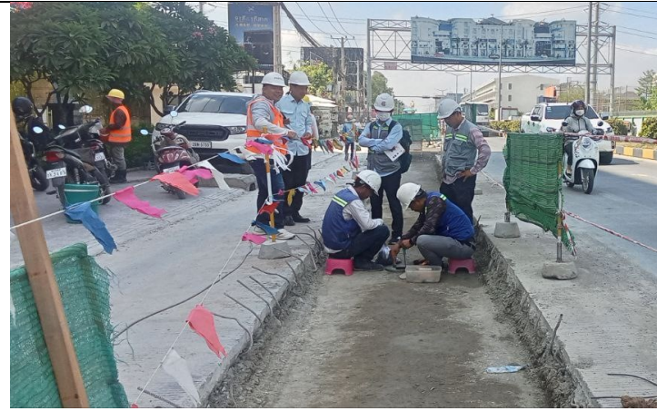
Photo: 01 Plate test of compaction road
