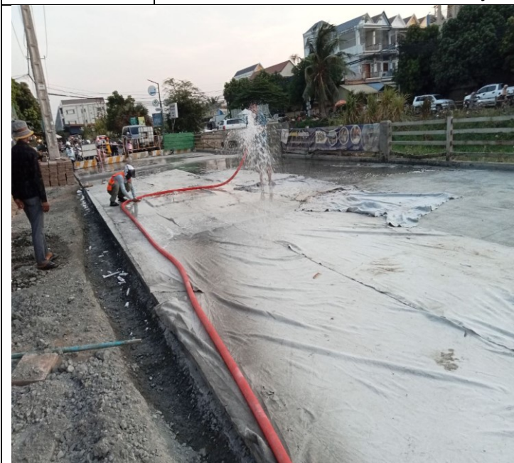
Photo: 29 Manhole of concrete road activity
