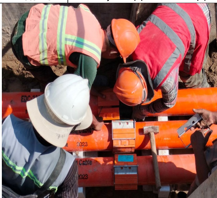
Photo: 22 Assembly PFP pipes and OFC pipe
