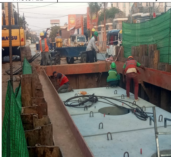
Photo: 24 Manhole Installation activity
