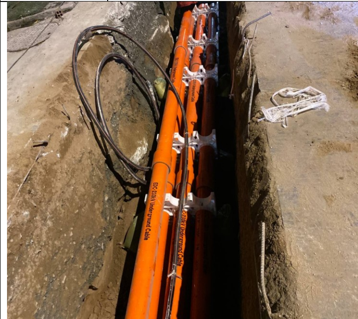
Photo: 17 Assembly PFP pipes and OFC pipe
