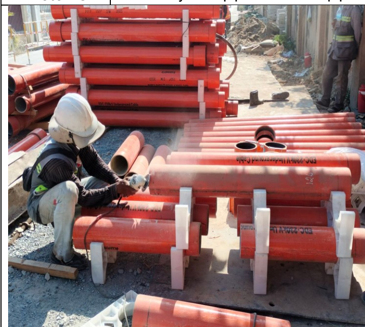
Photo: 21 Assembly PFP pipes and OFC pipe
