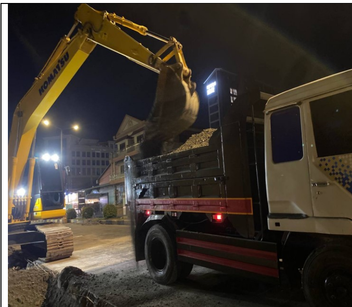
Photo: 07 Soil excavation and concrete road
