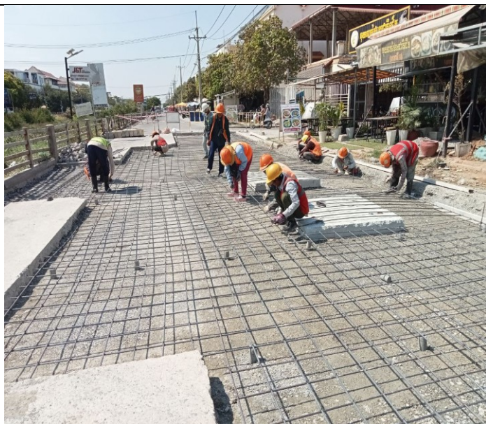
Photo: 08 Manhole of concrete road activity
