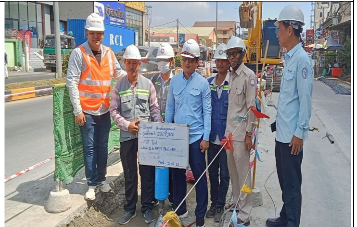
Photo: 04 Plate test of compaction road
