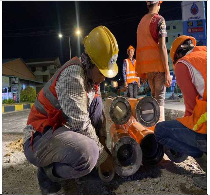
Photo: 32 Assembly PFP pipes and OFC pipe
