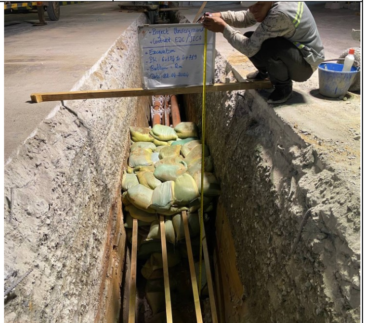
Photo: 34 Assembly PFP pipes and OFC pipe
