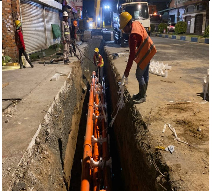
Photo: 16 Assembly PFP pipes and OFC pipe
