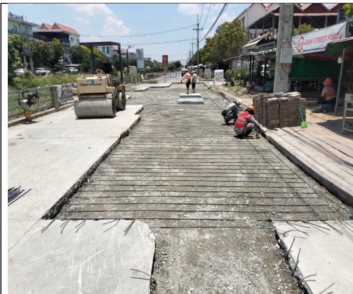
Photo: 07 Manhole of concrete road activity
