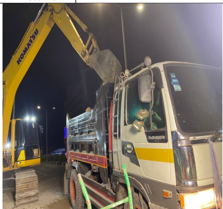
Photo: 12 Soil excavation and concrete road
