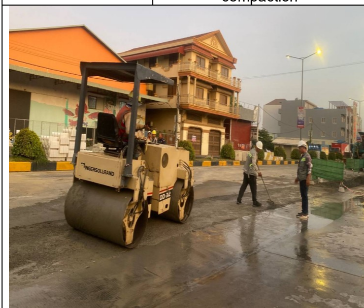
Base course backfilling and compaction
