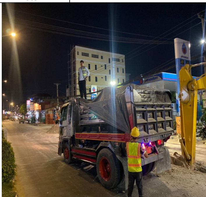
Photo: 16 Soil excavation and concrete road
