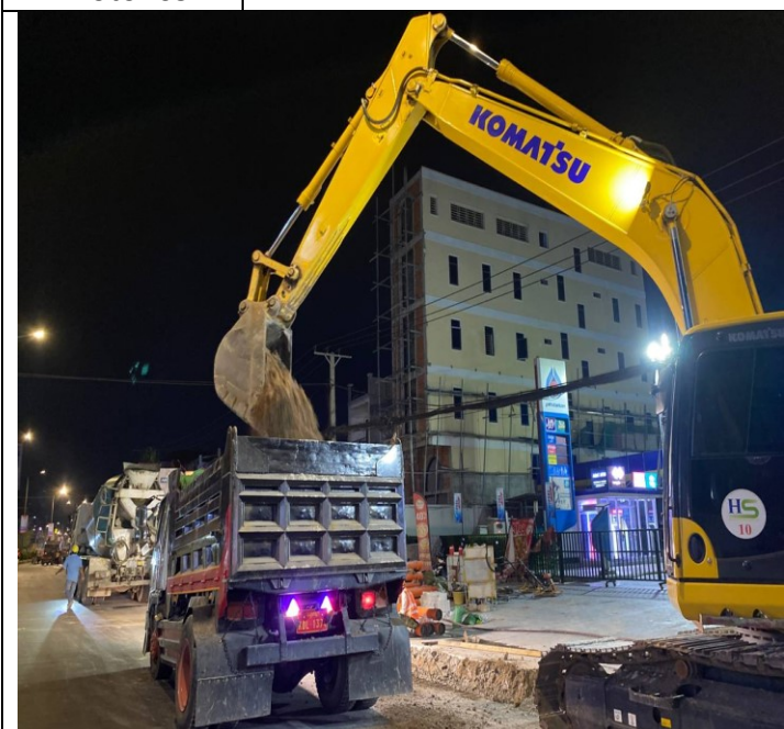
Photo: 11 Soil excavation and concrete road
