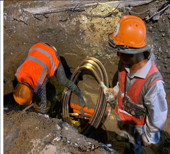
Photo: 15 Assembly PFP pipes and OFC pipe
