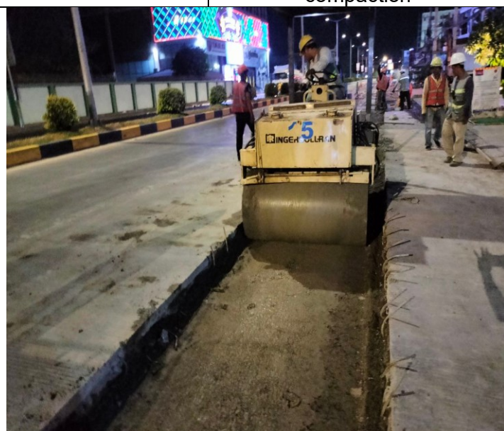
Base course backfilling and compaction
