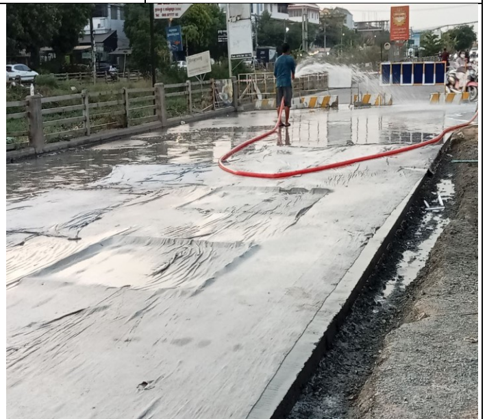
Photo: 28 Manhole of concrete road activity
