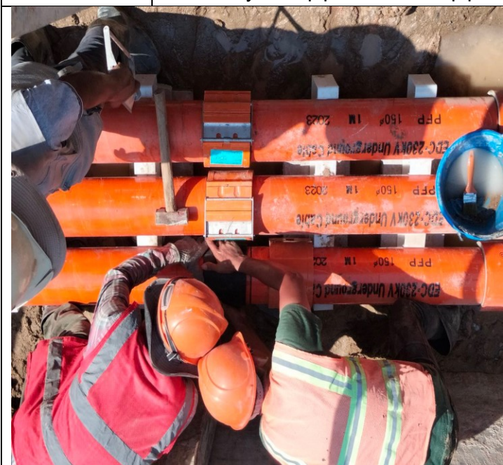
Photo: 23 Assembly PFP pipes and OFC pipe
