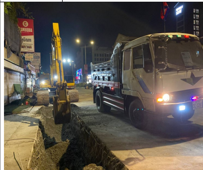
Photo: 05 Soil excavation and concrete road
