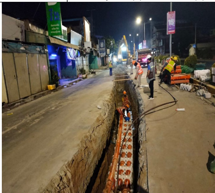
Photo: 30 Assembly PFP pipes and OFC pipe
