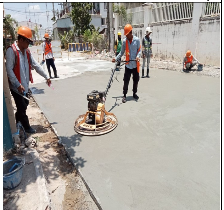
Photo: 24 Manhole of concrete road activity
