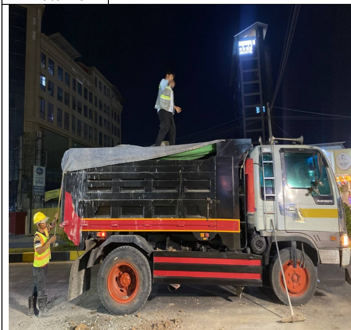
Photo: 15 Soil excavation and concrete road
