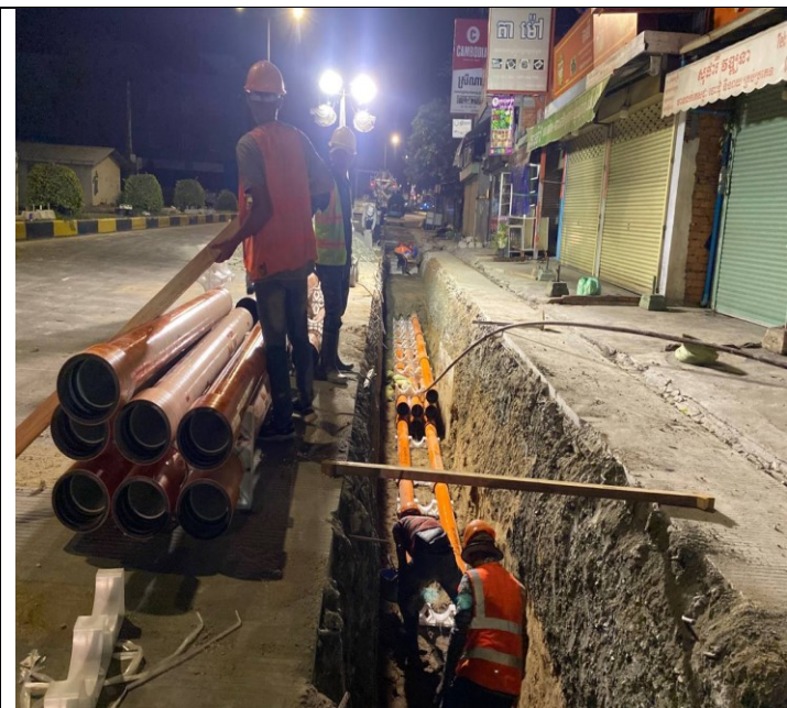
Photo: 25 Assembly PFP pipes and OFC pipe
