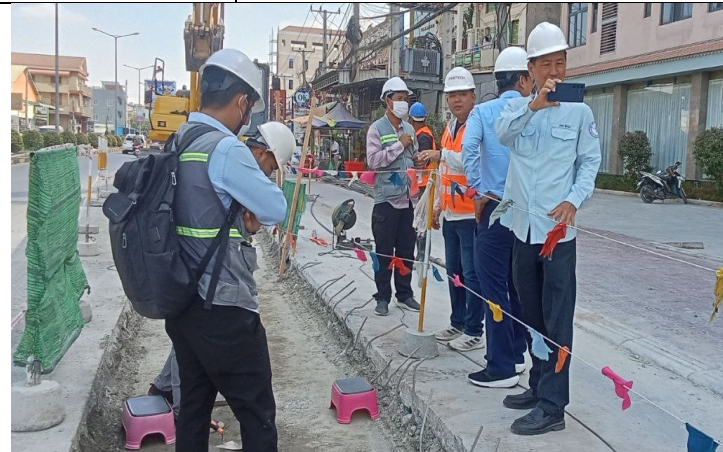
Photo: 03 Plate test of compaction road
