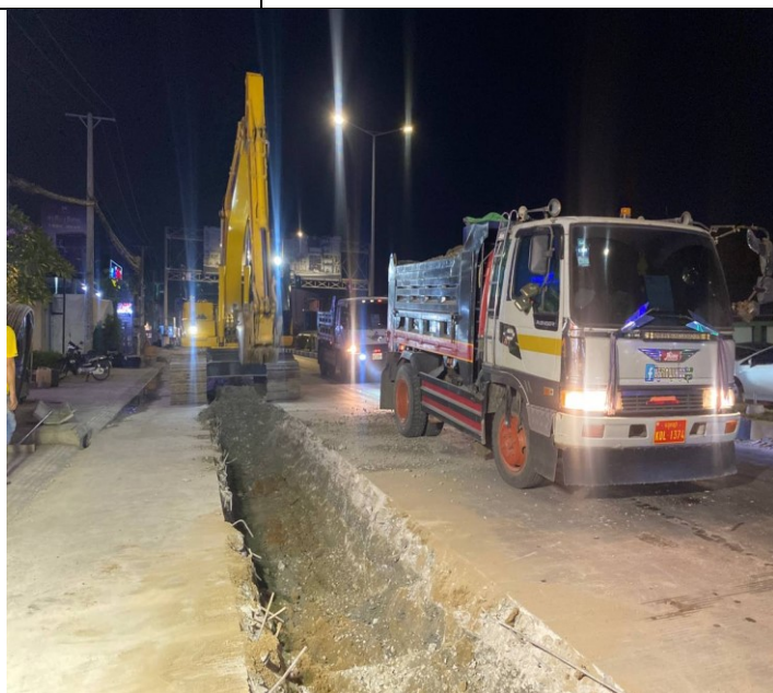
Photo: 18 Soil excavation and concrete road
