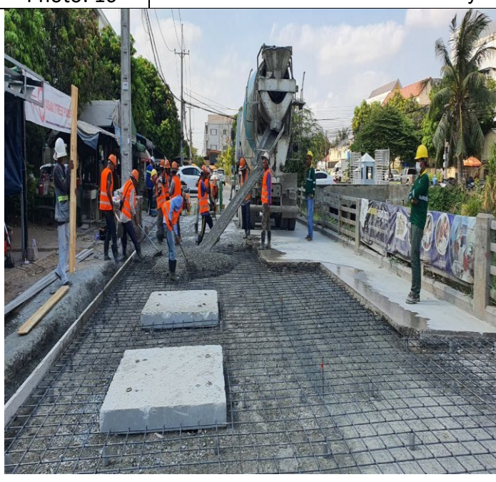
Photo: 18 Manhole of concrete road activity
