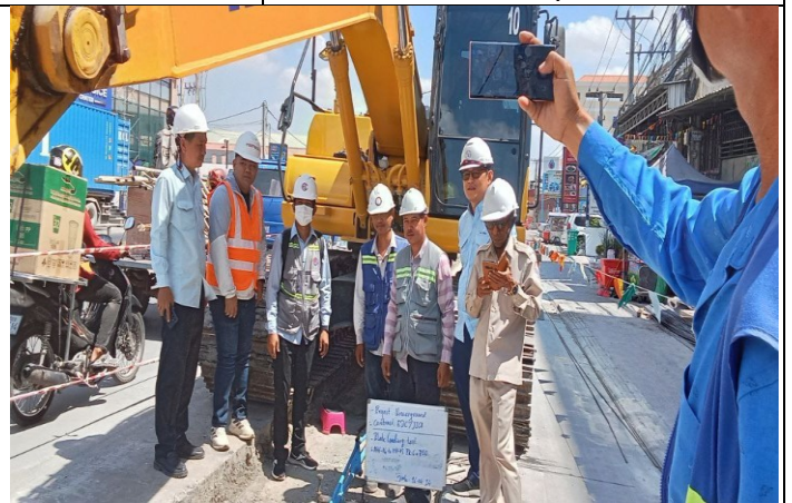
Photo: 08 Plate test of compaction road
