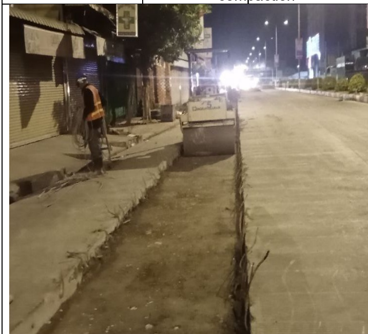
Base course backfilling and compaction
