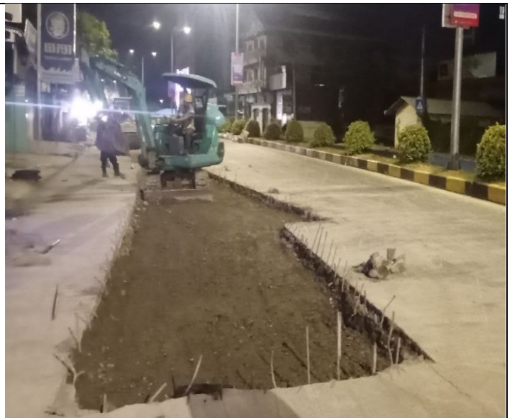
Base course backfilling and compaction
