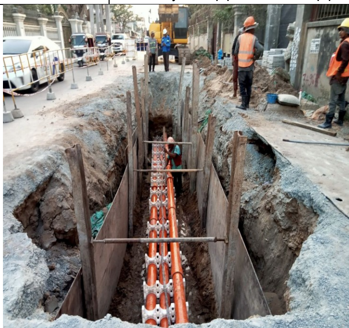
Photo: 24 Assembly PFP pipes and OFC pipe
