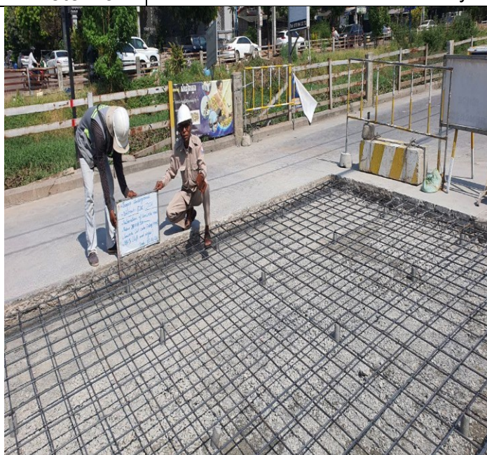
Photo: 12 Manhole of concrete road activity
