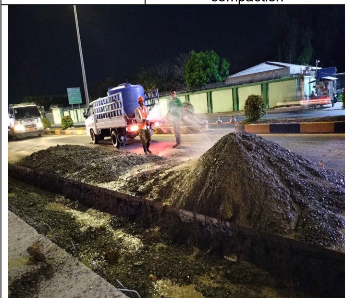
Base course backfilling and compaction
