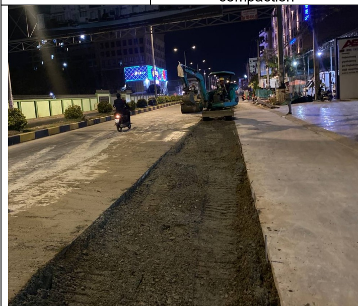
Base course backfilling and compaction
