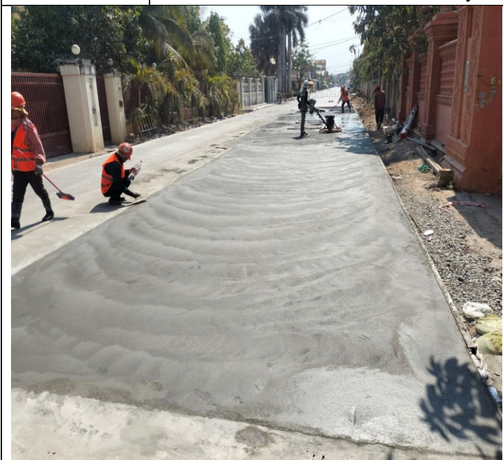
Photo: 23 Manhole of concrete road activity
