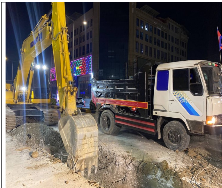
Photo: 13 Soil excavation and concrete road
