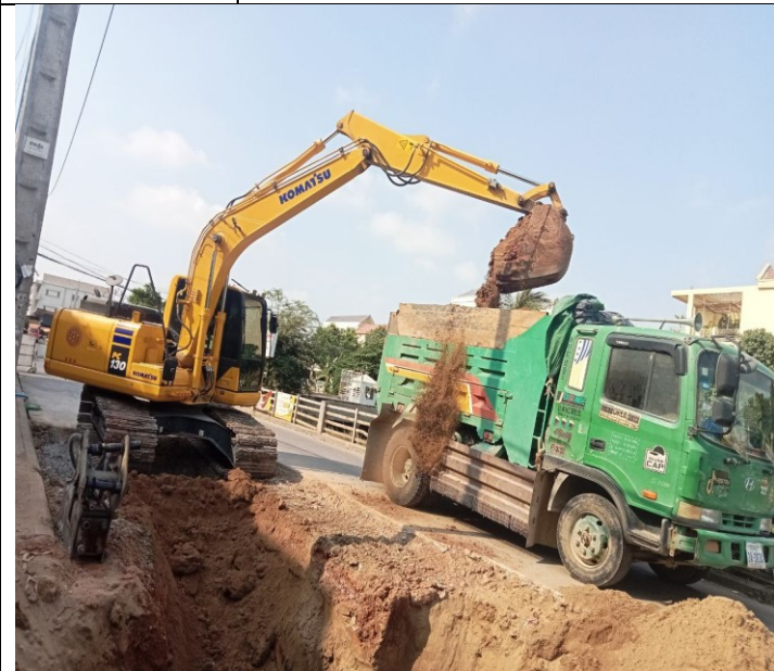
Photo: 03 Soil excavation and concrete road
