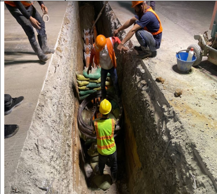
Photo: 33 Assembly PFP pipes and OFC pipe
