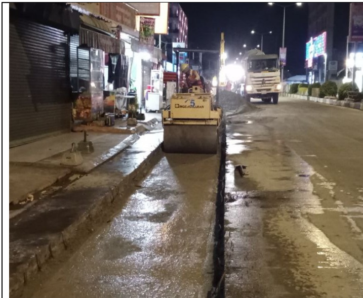
Base course backfilling and compaction
