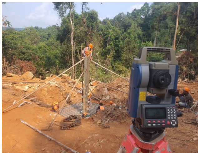
Set stub for the leg A.
