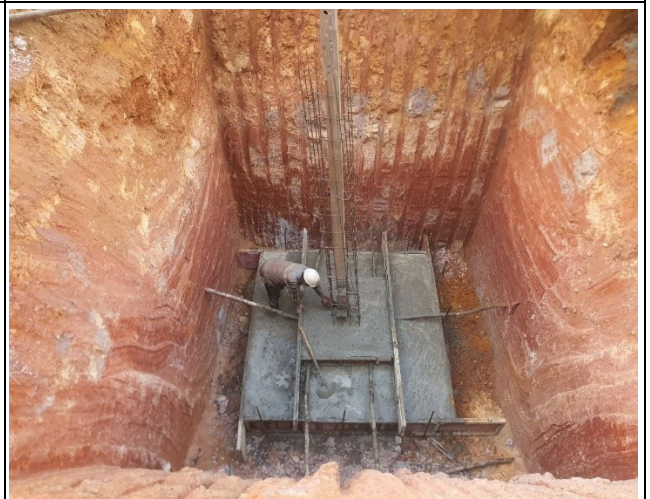
Casting concrete base for the leg B.
