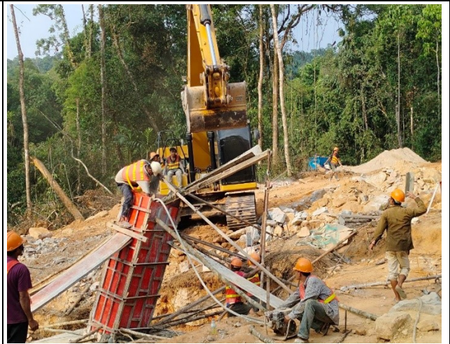
Soil excavation base for the leg B.
