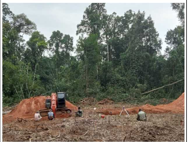
Soil excavation for the leg B.
