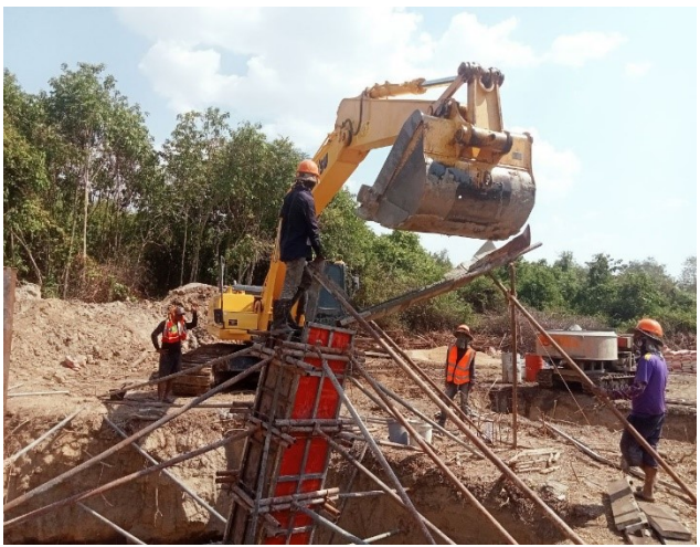
Casting concrete chimney for the leg D.
