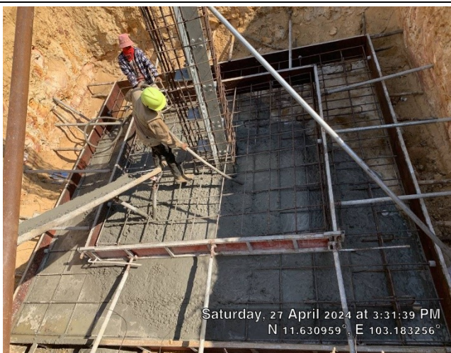
Casting concrete Base for the leg D.
