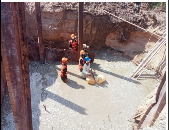
Soil excavation for the leg D.
