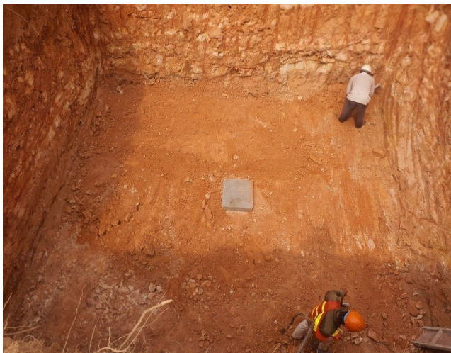
Soil excavation for the leg C.
