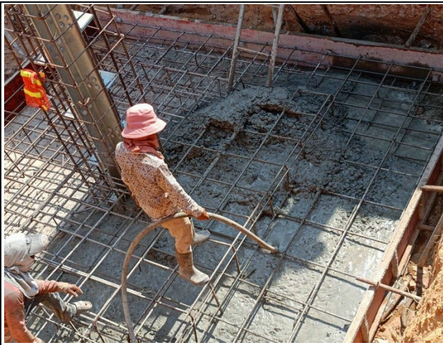
Casting concrete Base for the leg A.
