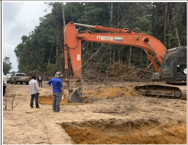
Soil excavation for the leg D.
