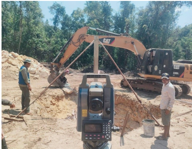
Stub setting for the leg B.
