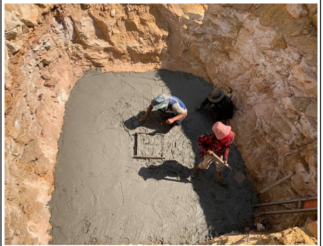
Casting concrete Lean for the leg A.
