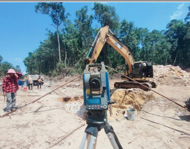
Stub setting for the leg D.
