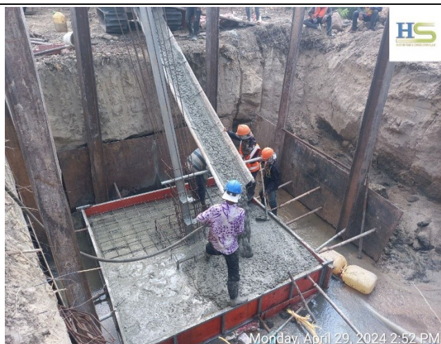
Casting concrete base for the leg C.
