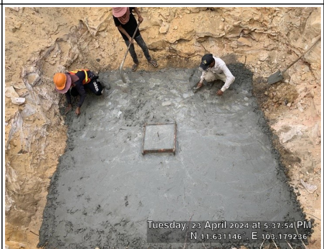
Casting concrete Lean for the leg C.
