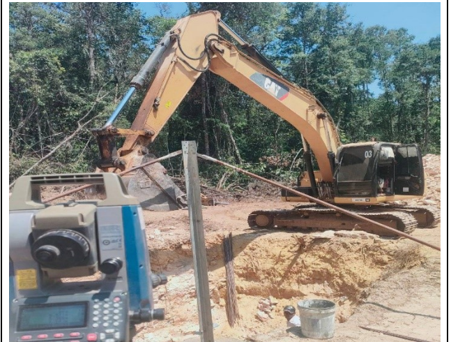
Stub setting for the leg C.
