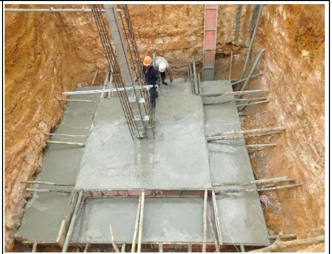
Casting concrete Base for the leg C.
