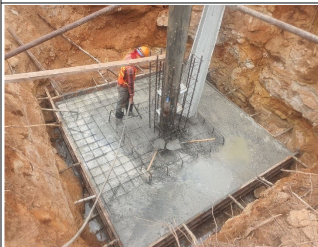
Casting concrete base for the leg C.
