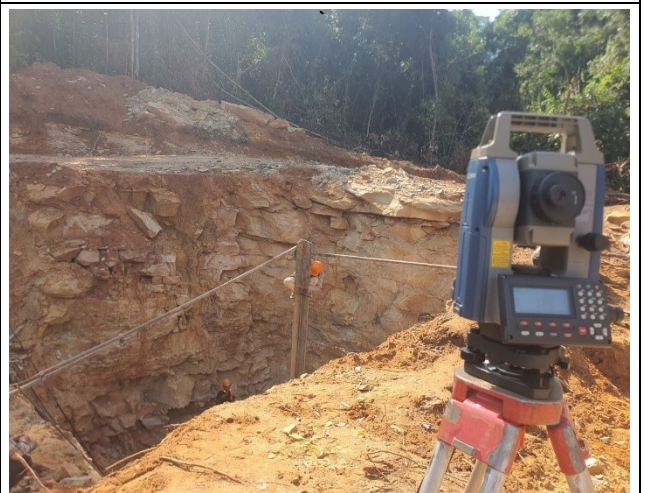
Set stub for the leg D.
