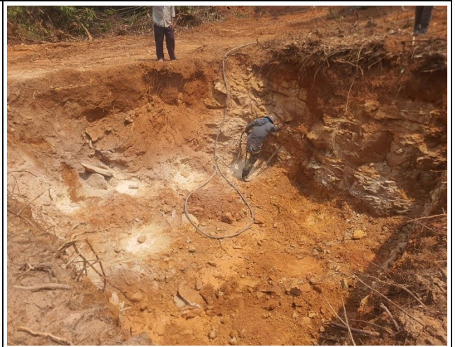
Soil excavation for the leg B.
