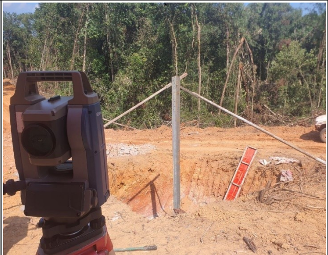
Stub setting for the leg B.
