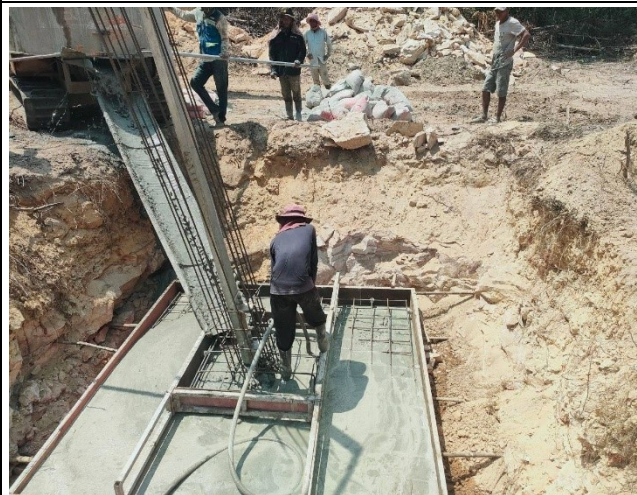
Casting concrete base for the leg B.
