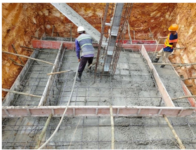
Casting concrete Base for the leg A.
