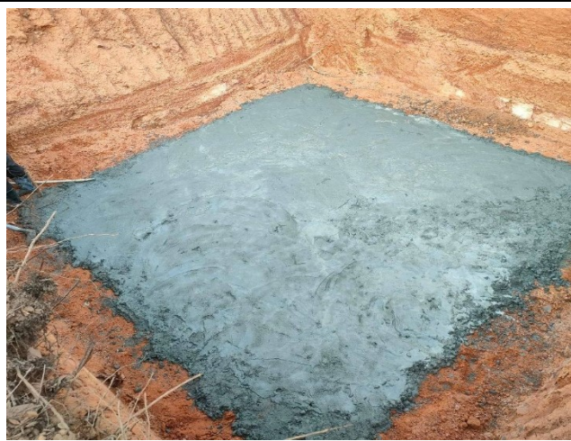
Casting concrete lean for the leg C.
