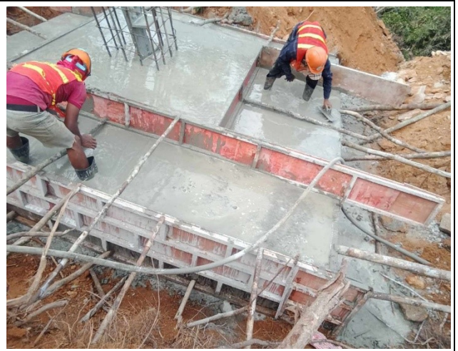
Soil excavation base for the leg A.
