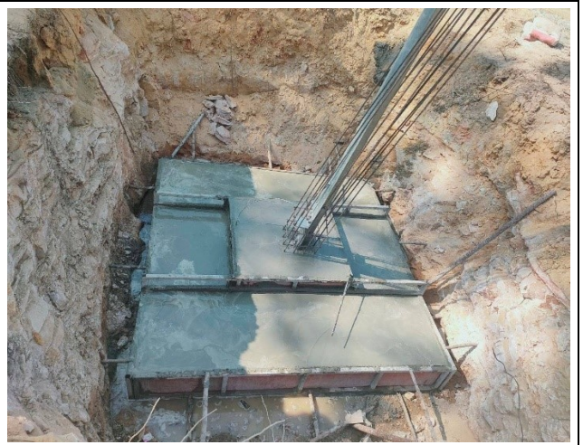
Casting concrete base for the leg D.
