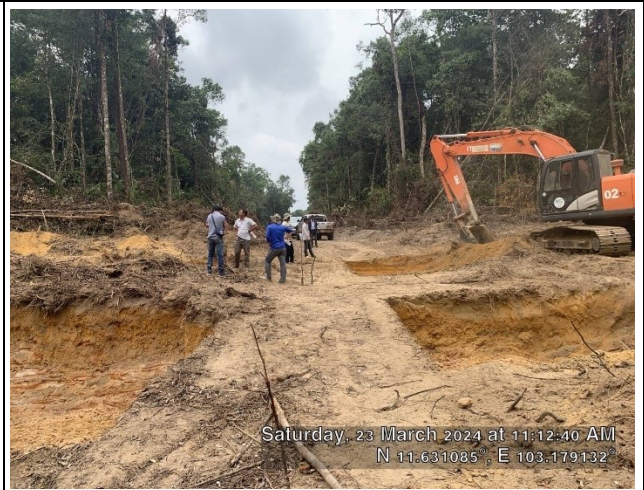
Soil excavation for the leg B.
