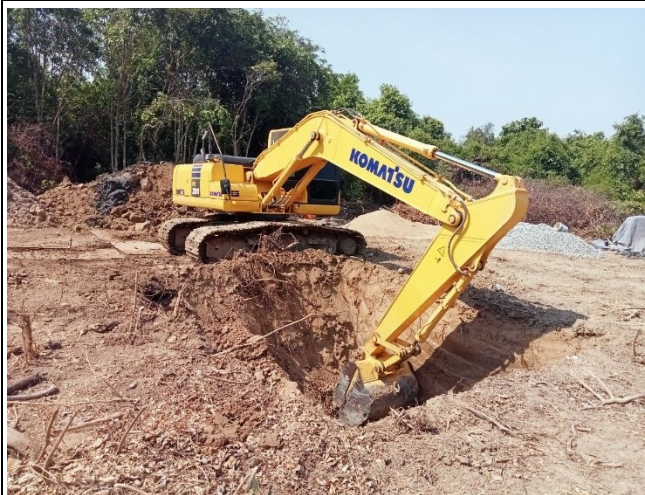
Soil excavation for the leg A.
