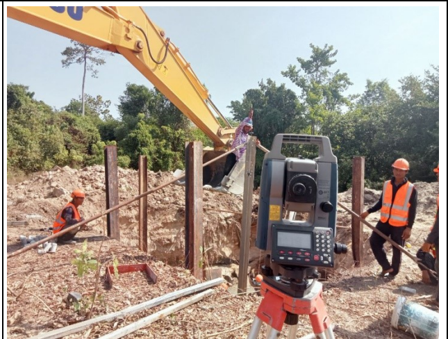
Set stub for the leg D.
