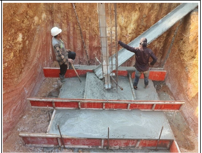
Casting concrete base for the leg A.
