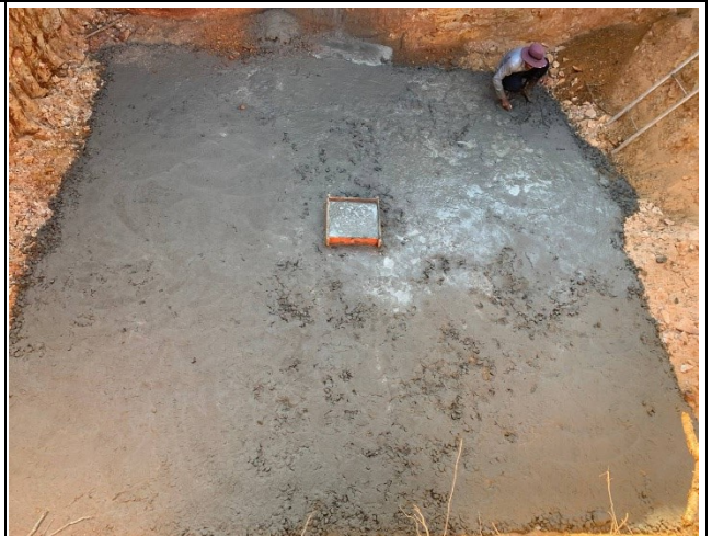
Casting concrete lean for the leg C.
