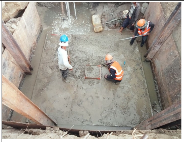
Casting concrete Lean for the leg D.
