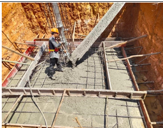
Casting concrete Base for the leg D.
