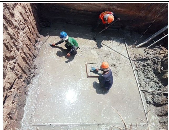
Casting concrete Lean for the leg B.
