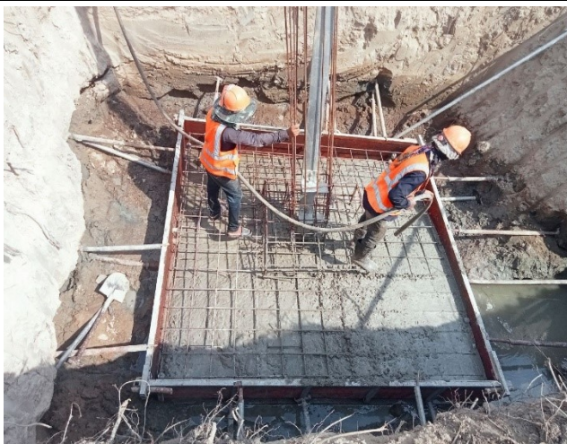
Casting concrete base for the leg A.
