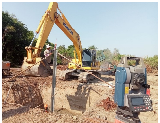
Soil excavation for the leg B.
