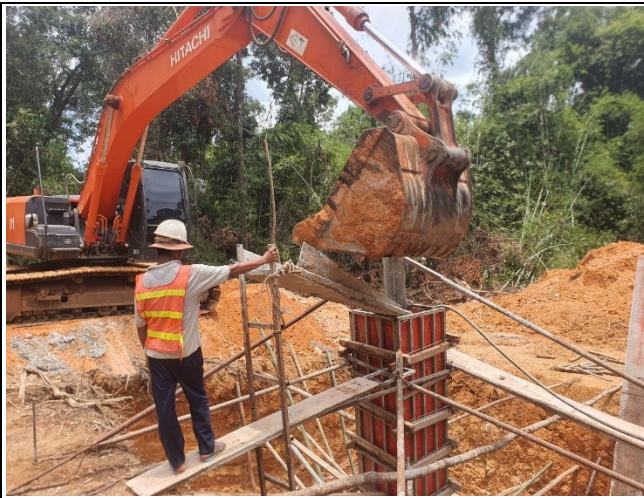
Casting concrete chimney for the leg D.
