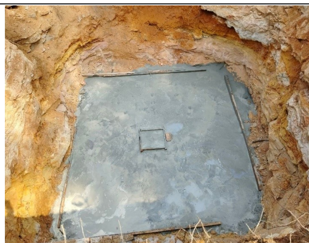
Casting concrete lean for the leg A.
