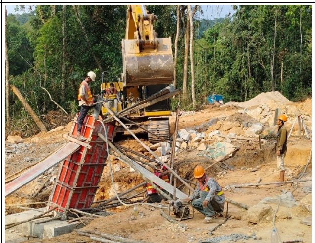
Casting concrete chimney for the leg A.
