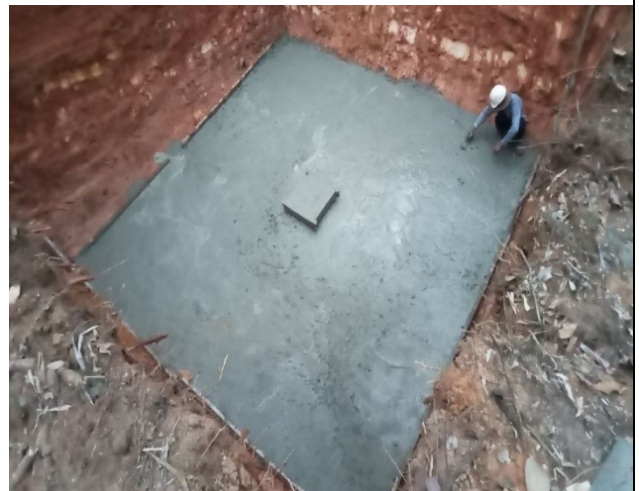
Casting concrete lean for the leg B.
