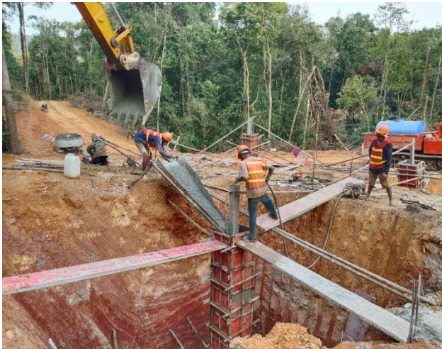
Casting concrete chimney for the leg A.
