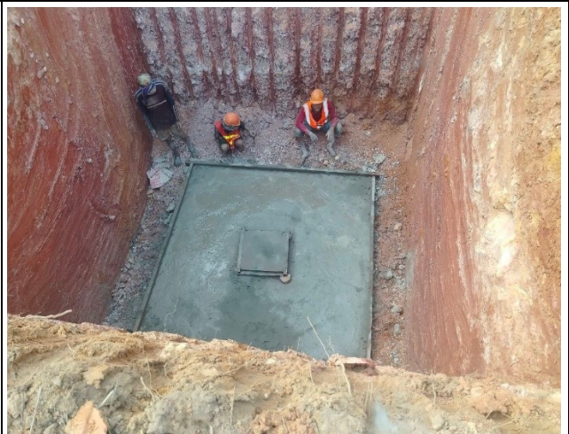
Casting concrete lean for the leg D.
