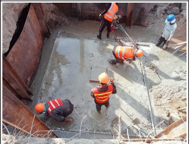
Casting concrete Lean for the leg C.
