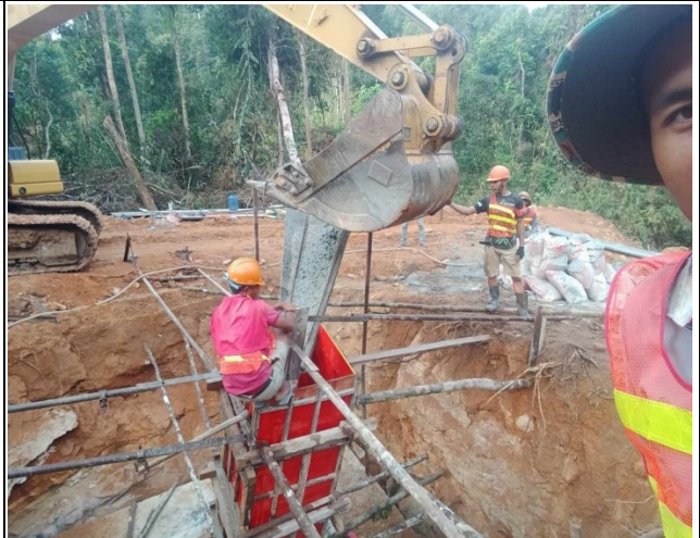
Casting concrete chimney for the leg C.
