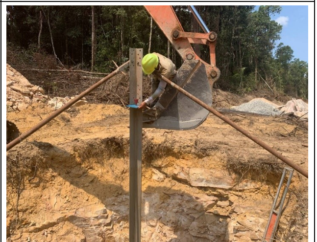
Stub setting for the leg A.
