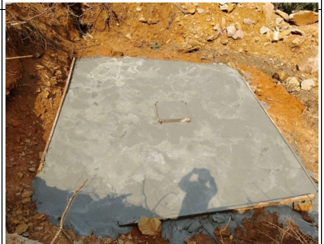
Casting concrete lean for the leg B.
