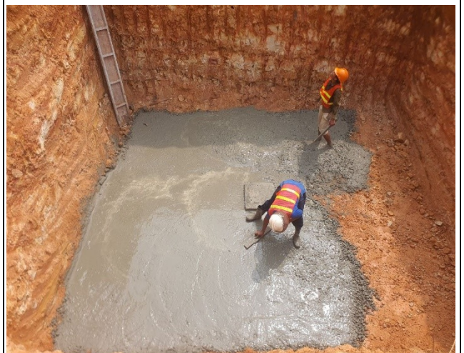
Casting concrete lean for the leg D.
