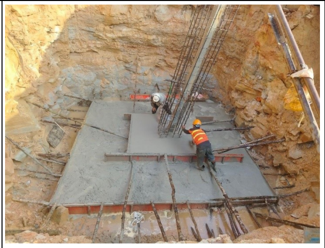
Soil excavation base for the leg D.
