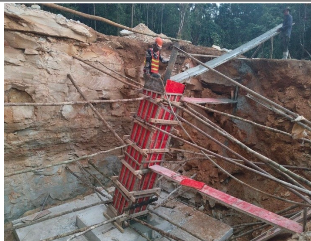
Casting concrete chimney for the leg C.
