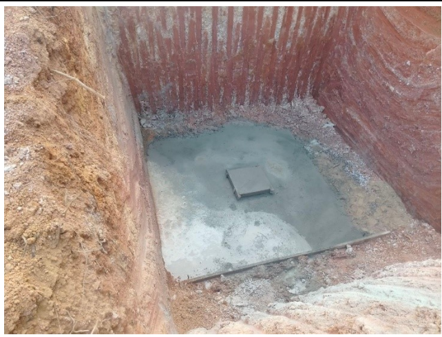
Casting concrete lean for the leg C.
