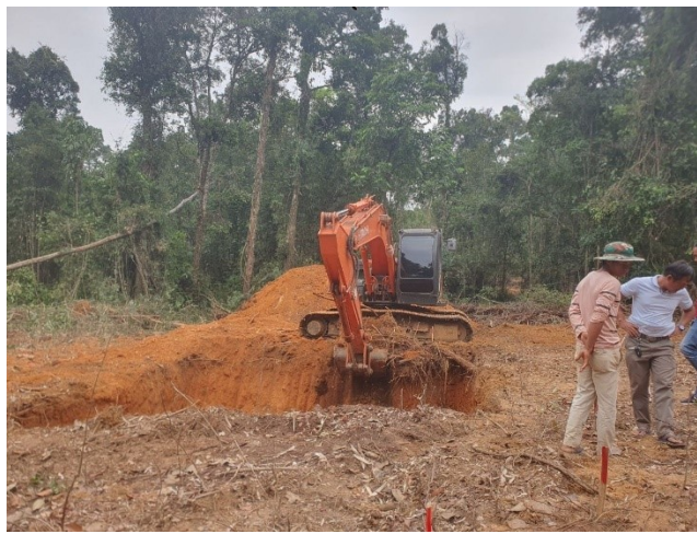
Soil excavation for the leg A.
