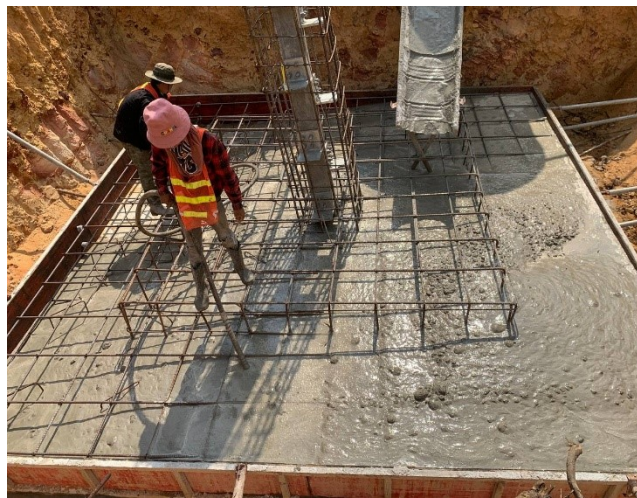
Casting concrete Base for the leg C.
