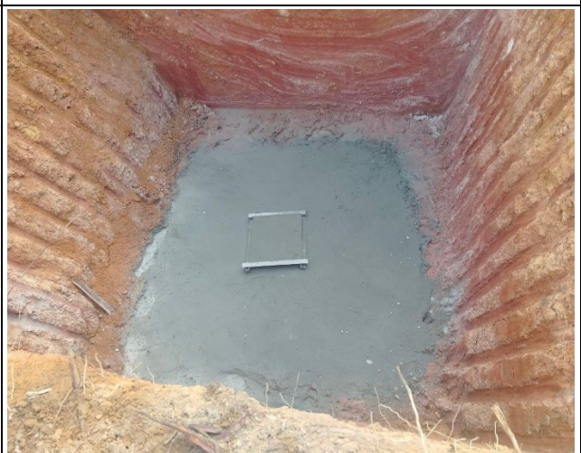
Casting concrete lean for the leg B.
