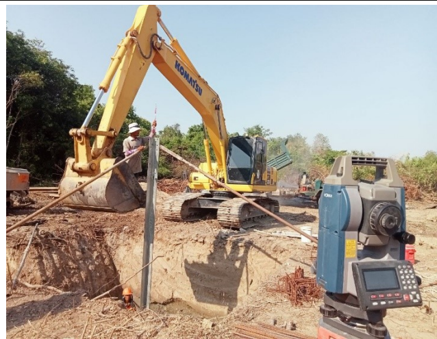
Soil excavation for the leg A.
