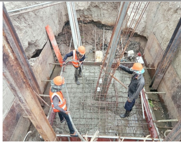
Casting concrete base for the leg D.
