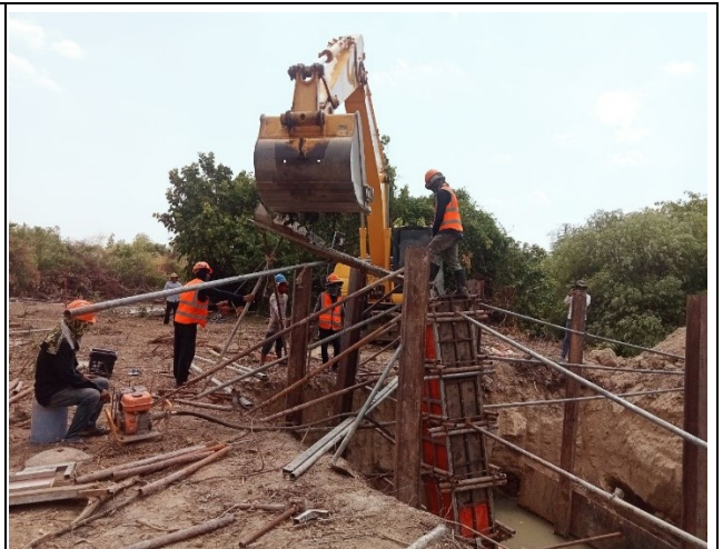
Casting concrete chimney for the leg C.
