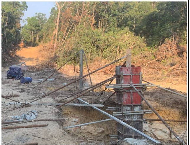
Casting concrete Chimney for the leg B.
