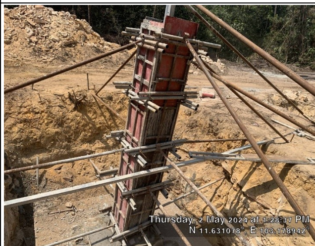
Casting concrete Chimney for the leg C.
