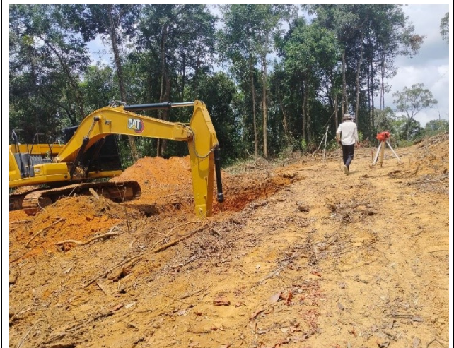
Siol excavation for the leg D.
