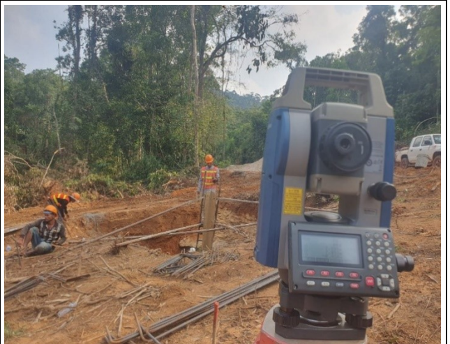
Set stub for the leg B.
