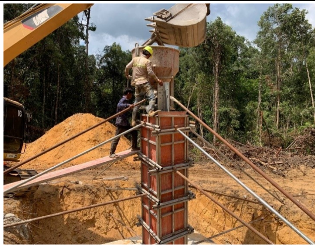
Casting concrete Chimney for the leg D.
