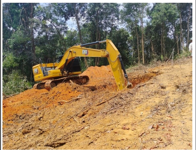
Siol excavation for the leg B.
