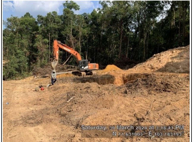
Soil excavation for the leg B.
