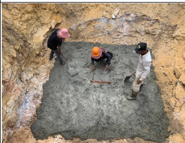
Casting concrete Lean for the leg B.
