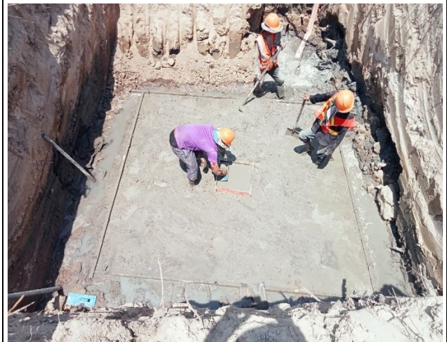
Casting concrete Lean for the leg A.
