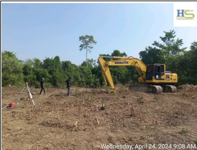
Soil excavation for the leg C.
