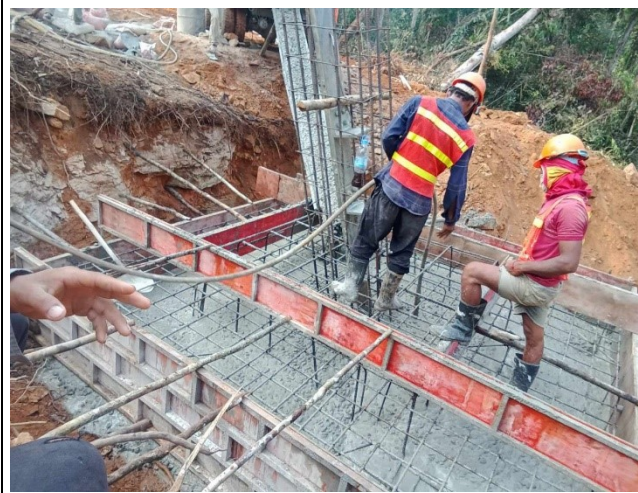
Casting concrete base for the leg B.
