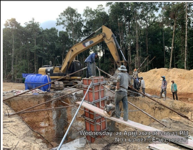
Casting concrete Chimney for the leg B.
