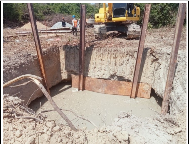
Soil excavation for the leg C.
