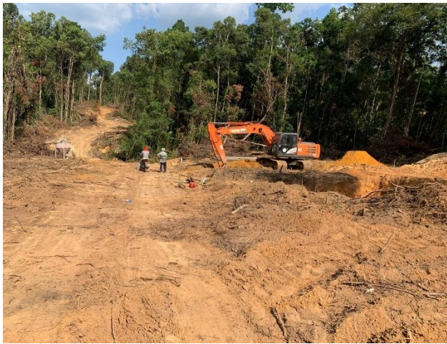
Soil excavation for the leg A.
