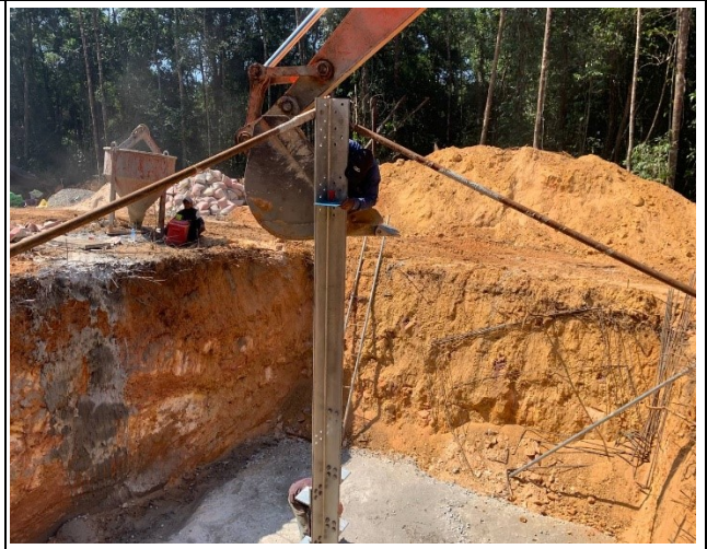
Set stub for the leg C.
