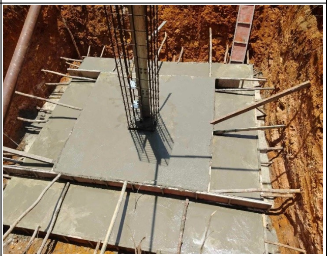
Casting concrete Base for the leg D.
