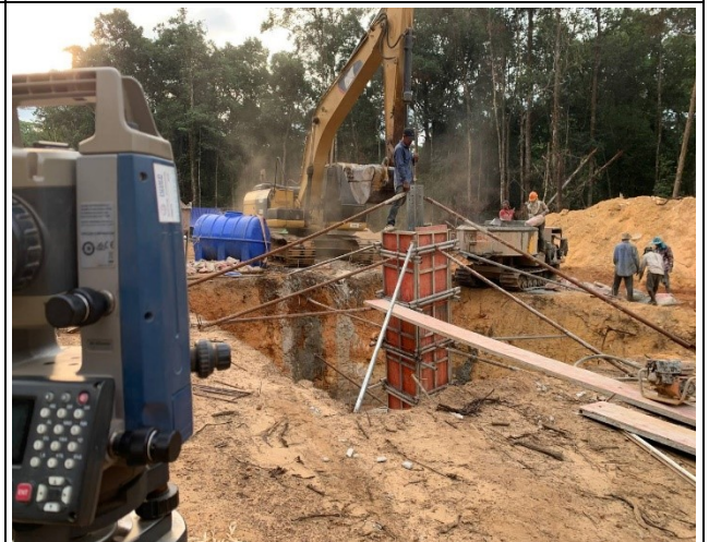
Casting concrete Chimney for the leg B.
