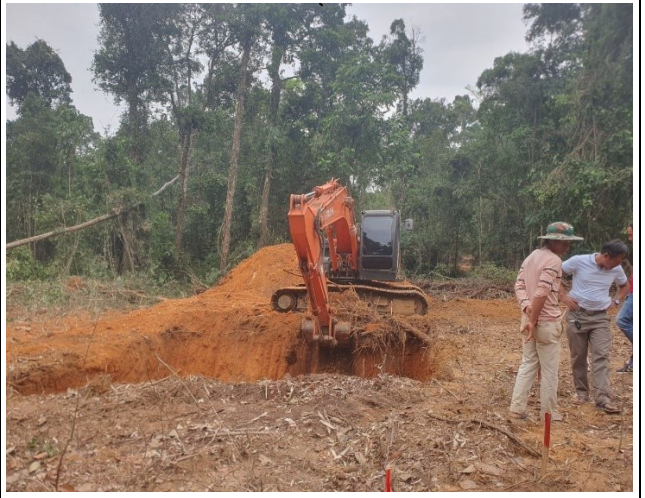
Soil excavation for the leg D.
