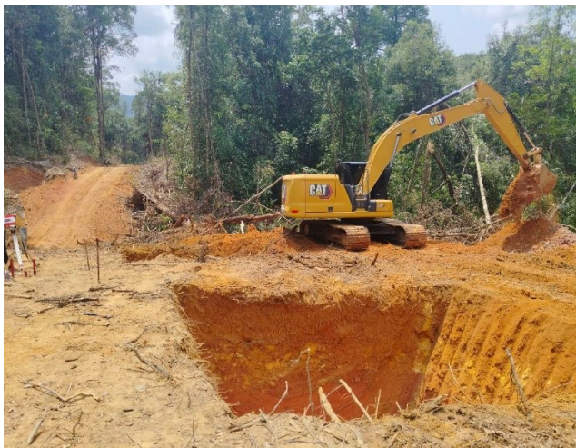
Siol excavation for the leg C.
