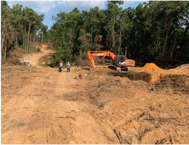
Soil excavation for the leg C.
