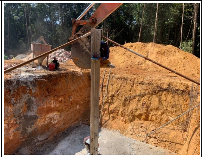
Set stub for the leg D.
