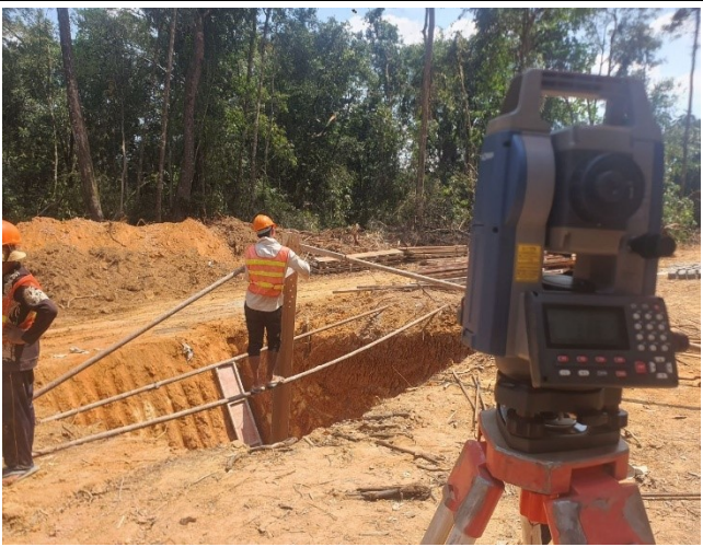
Stub setting for the leg A.
