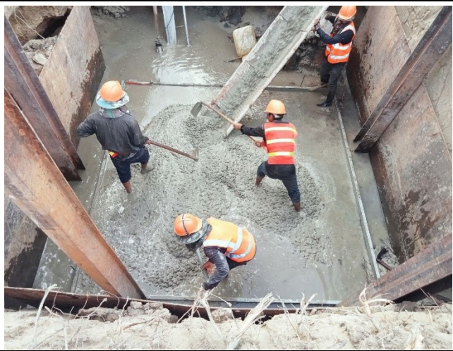
Casting concrete Lean for the leg D.
