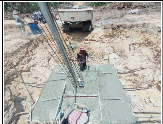
Casting concrete base for the leg B.
