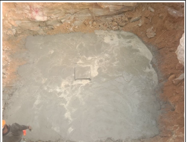
Soil excavation for the leg D.
