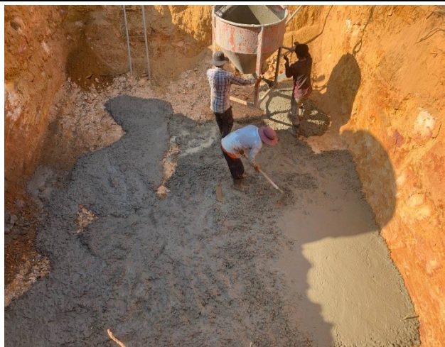
Casting concrete lean for the leg B.
