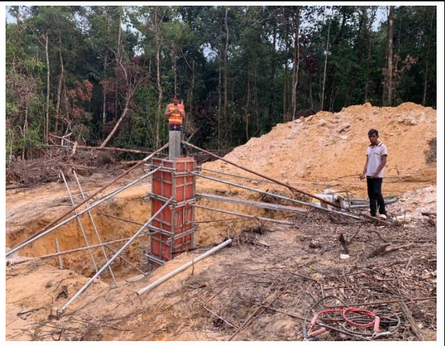
Casting concrete Chimney for the leg D.
