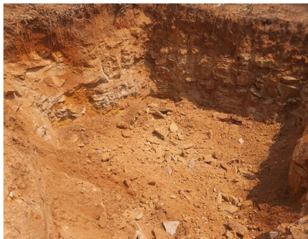
Soil excavation for the leg C.
