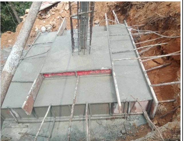
Casting concrete base for the leg B.
