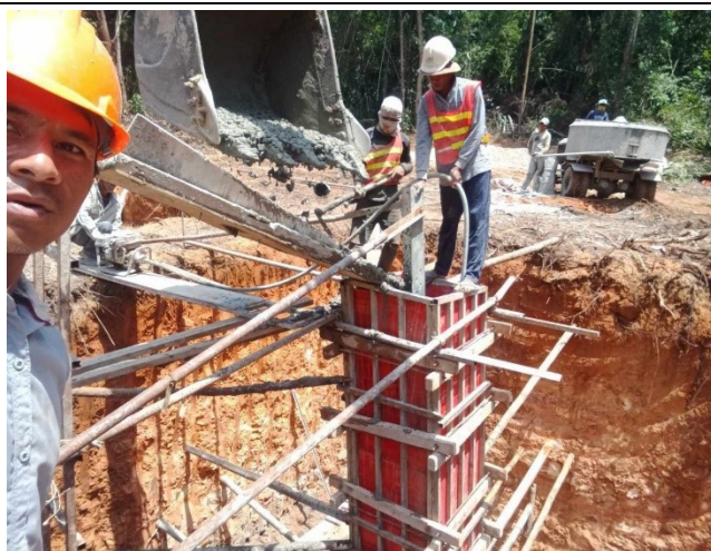
Casting concrete chimney for the leg B.
