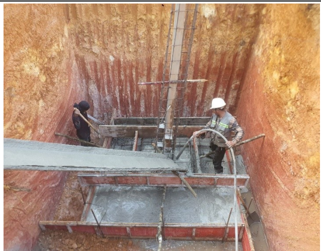
Casting concrete base for the leg B.
