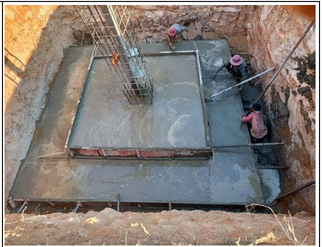
Casting concrete Base for the leg A.
