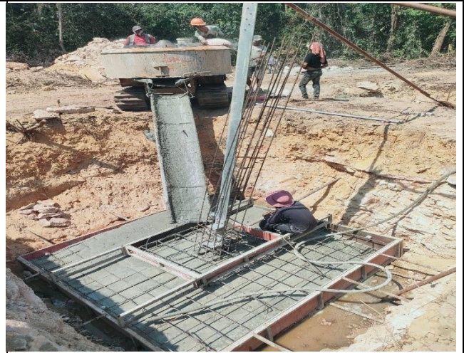
Casting concrete base for the leg A.
