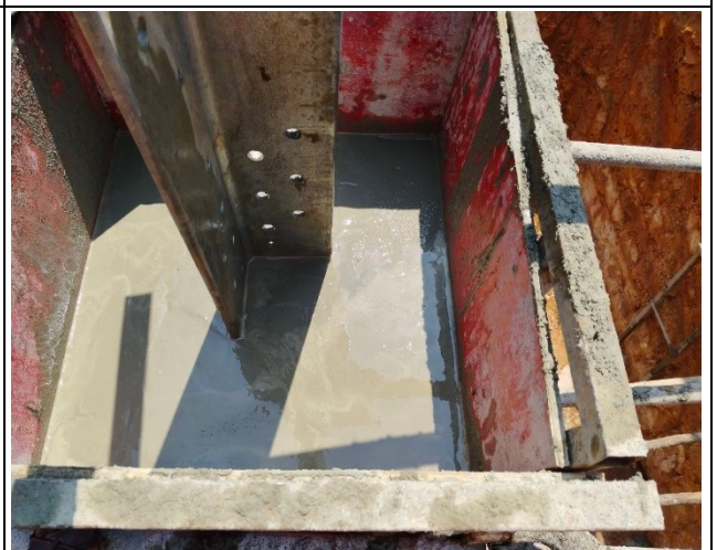
Casting concrete chimney for the leg C.
