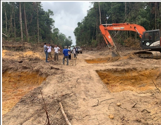
Soil excavation for the leg C.
