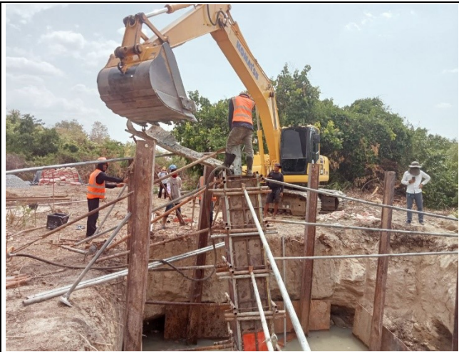
Casting concrete chimney for the leg C.
