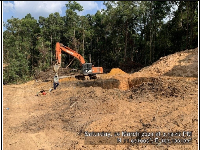
Soil excavation for the leg D.
