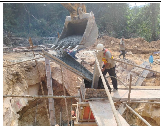
Casting concrete chimney for the leg A.
