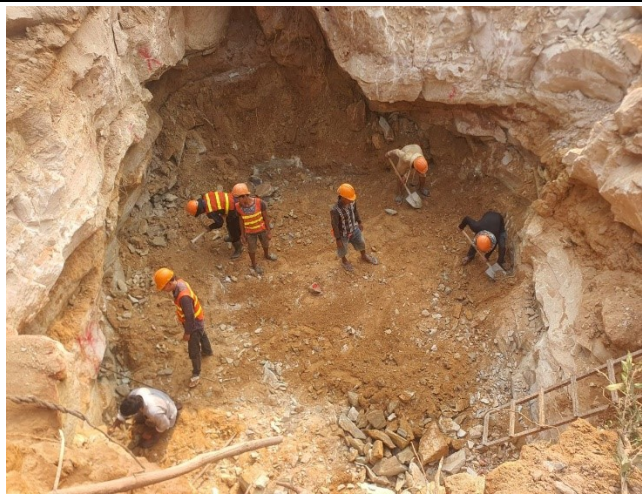
Soil excavation for the leg A.
