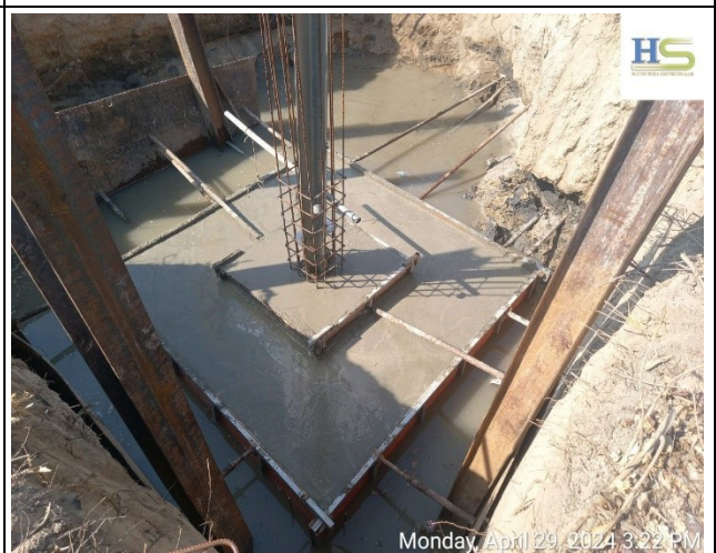
Casting concrete base for the leg C.
