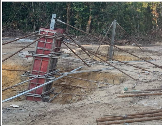
Casting concrete Chimney for the leg A.
