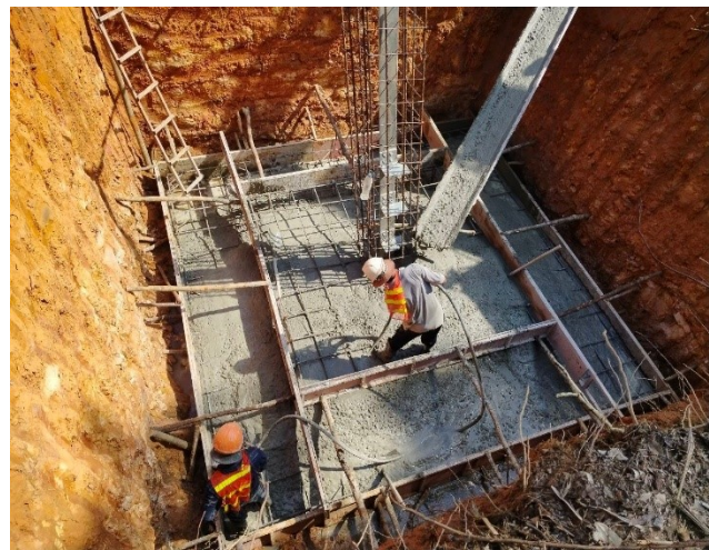
Casting concrete Base for the leg B.
