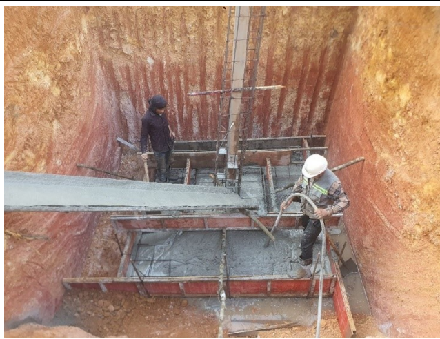
Casting concrete base for the leg A.
