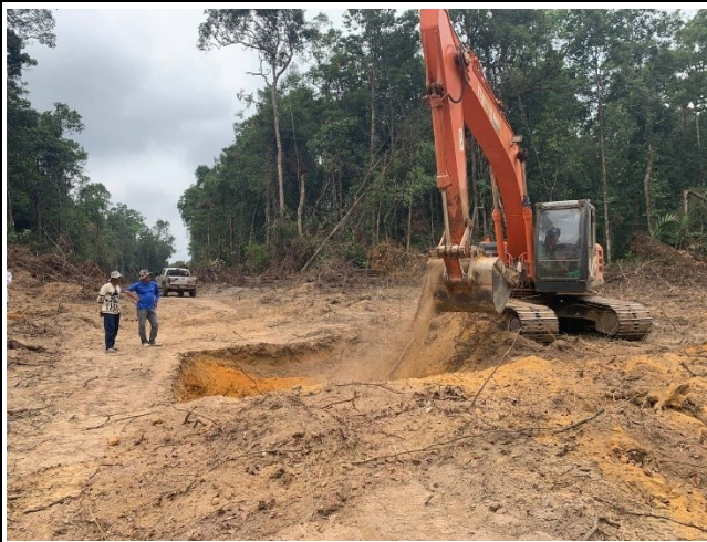
Soil excavation for the leg A.
