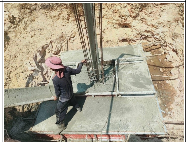
Casting concrete base for the leg C.
