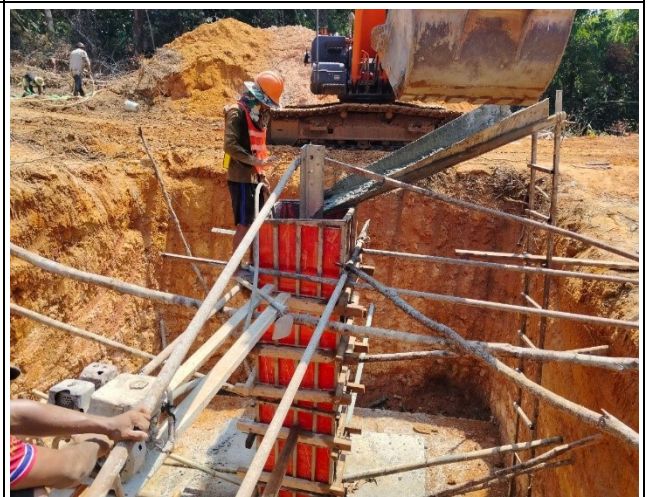
Casting concrete chimney for the leg C.
