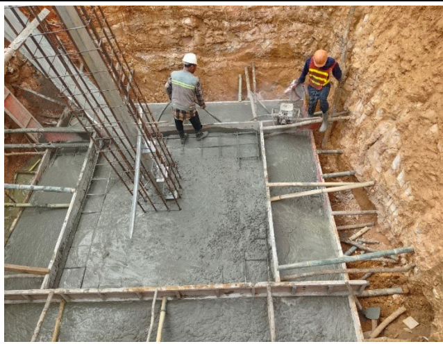
Casting concrete Base for the leg C.
