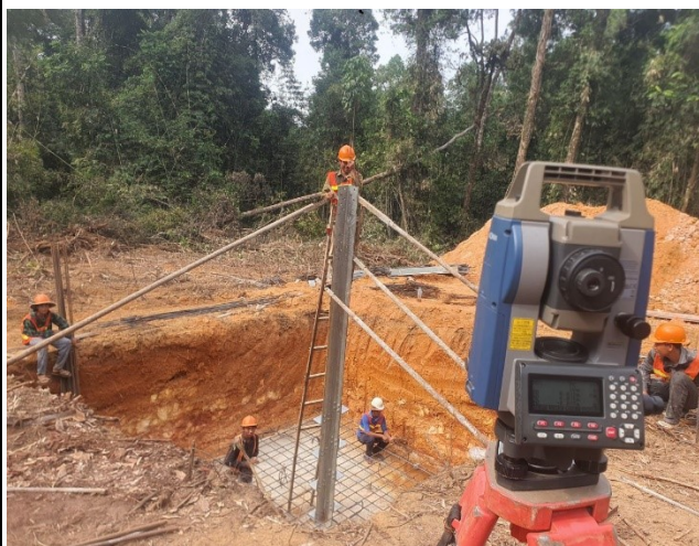
Stub setting for the leg A.
