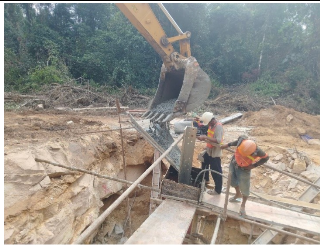
Casting concrete base for the leg B.
