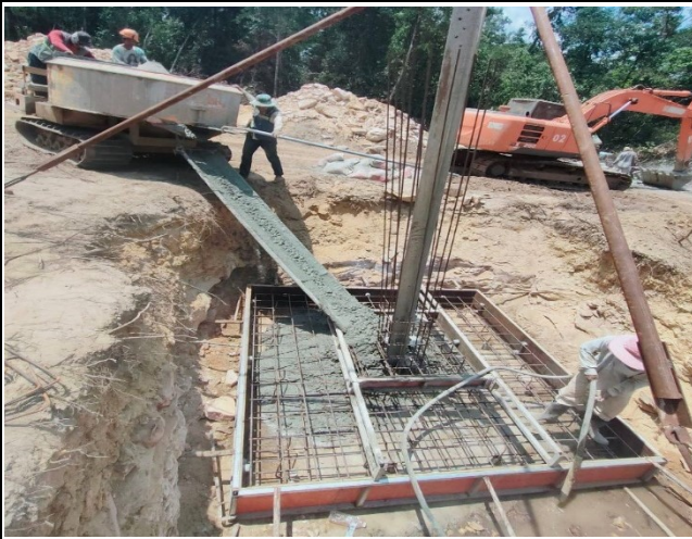
Casting concrete base for the leg A.
