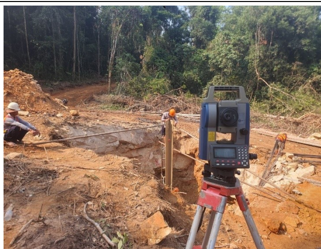
Set stub for the leg C.
