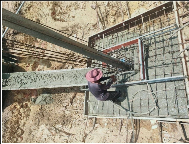
Casting concrete base for the leg D.
