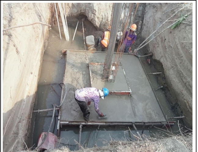
Casting concrete base for the leg B.
