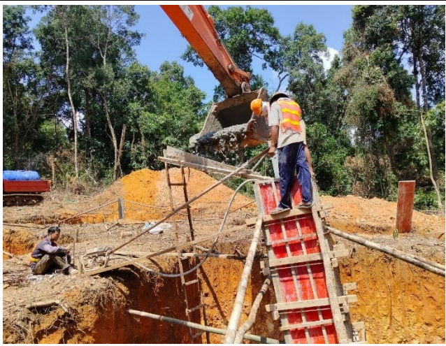
Casting concrete chimney for the leg A.
