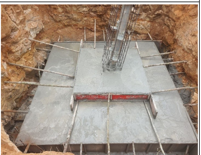
Casting concrete base for the leg C.
