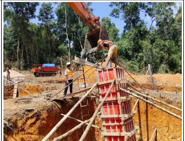
Casting concrete chimney for the leg A.
