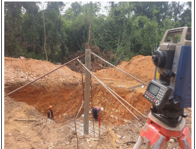
Stub setting for the leg B.
