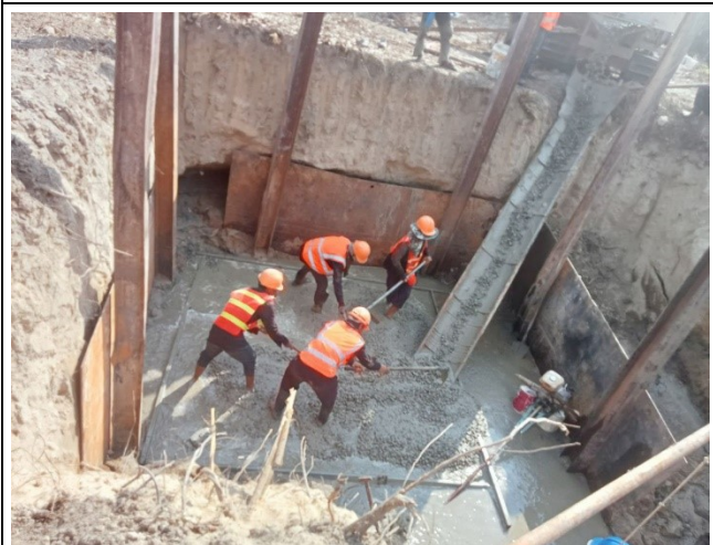
Casting concrete Lean for the leg C.
