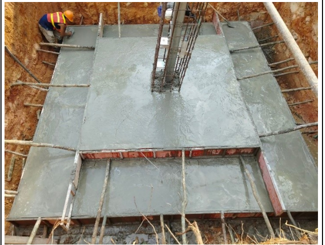
Casting concrete Base for the leg A.
