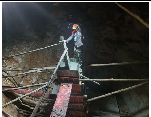
Casting concrete chimney for the leg D.
