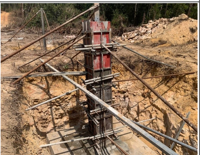
Casting concrete base for the leg D.
