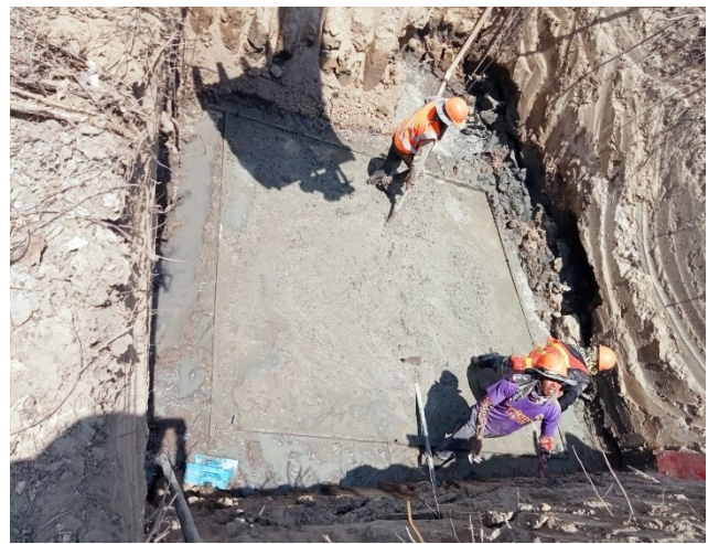
Casting concrete Lean for the leg A.
