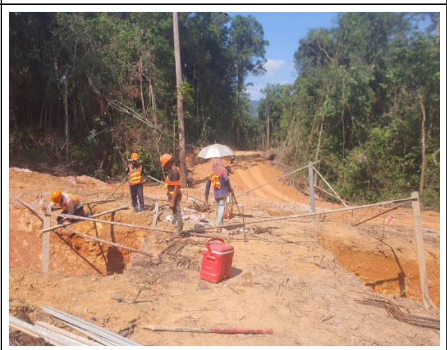
Stub setting for the leg D.
