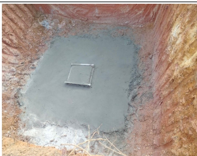
Casting concrete lean for the leg A.
