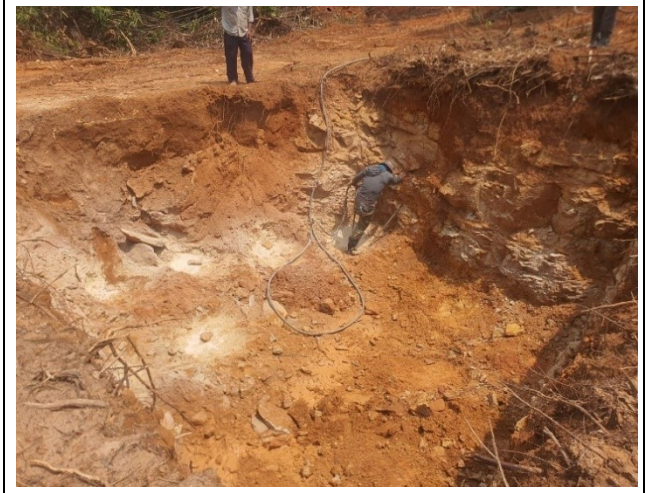
Soil excavation for the leg D.
