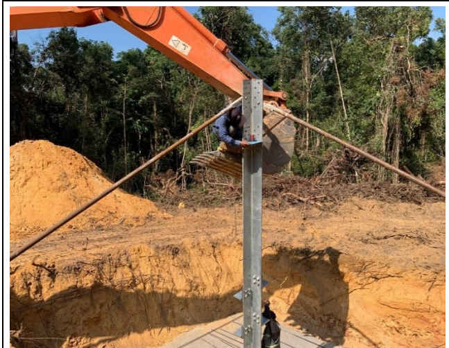
Set stub for the leg A.
