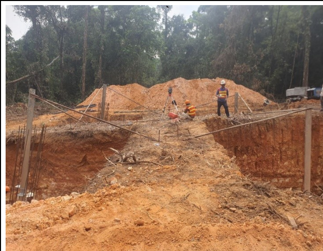
Stub setting for the leg C.
