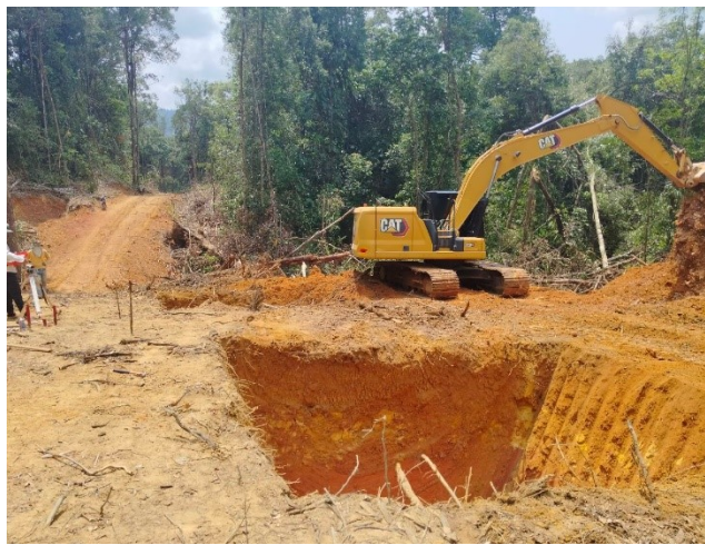
Siol excavation for the leg A.
