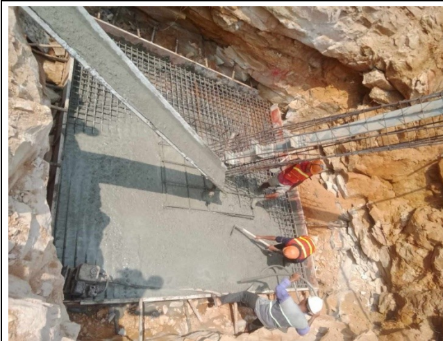
Casting concrete base for the leg A.
