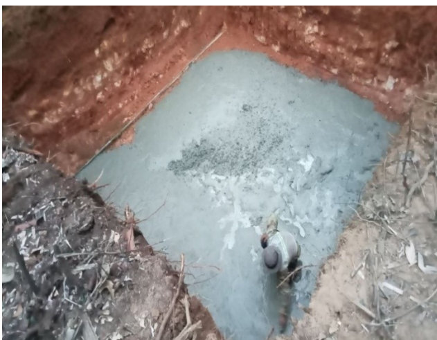
Casting concrete lean for the leg A.
