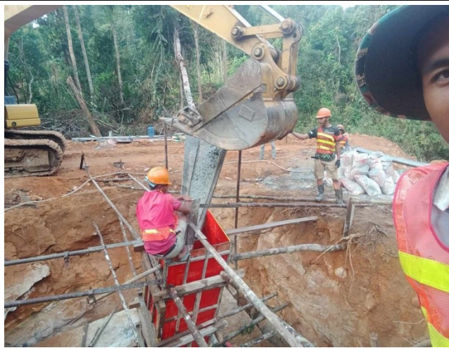
Casting concrete chimney for the leg C.
