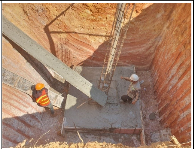
Casting concrete base for the leg D.
