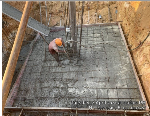
Casting concrete Base for the leg B.
