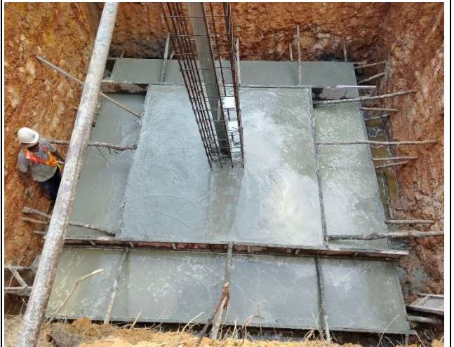
Casting concrete Base for the leg B.
