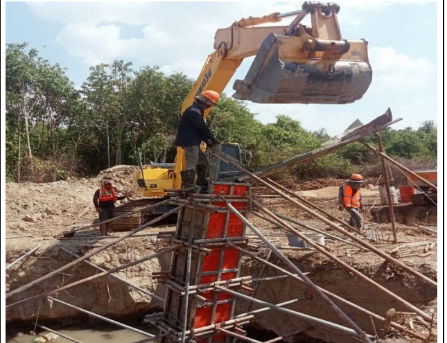
Casting concrete chimney for the leg D.
