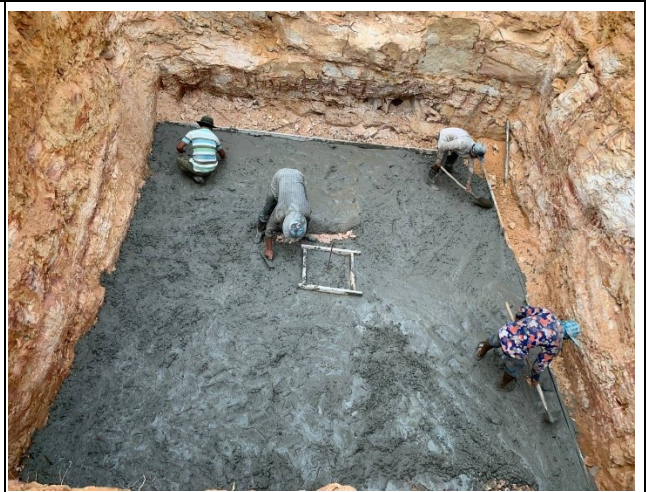
Casting concrete lean for the leg A.
