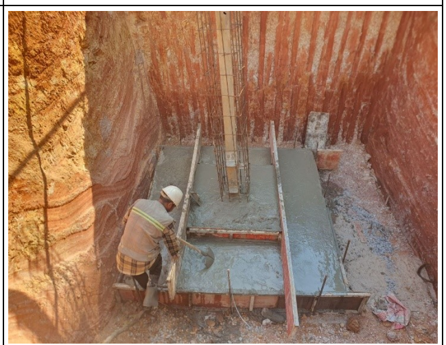
Casting concrete base for the leg C.
