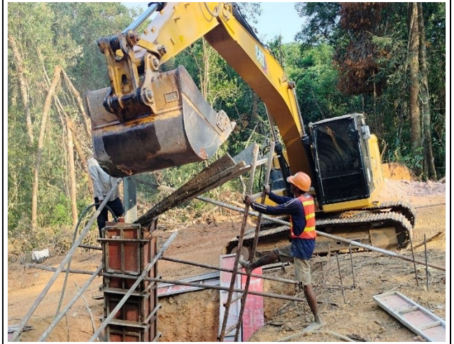
Casting concrete chimney for the leg B.
