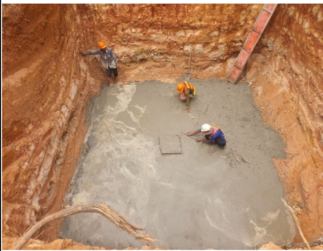
Casting concrete lean for the leg C.
