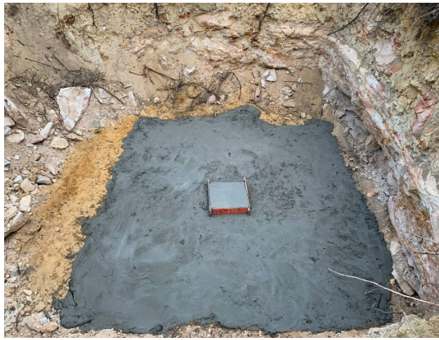
Casting concrete Lean for the leg D.
