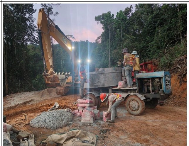
Casting concrete base for the leg D.
