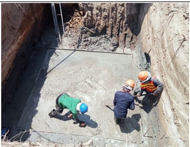
Casting concrete Lean for the leg B.
