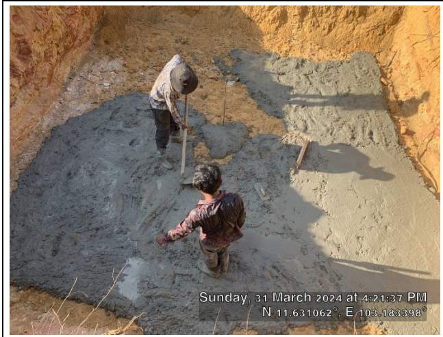
Casting concrete lean for the leg D.
