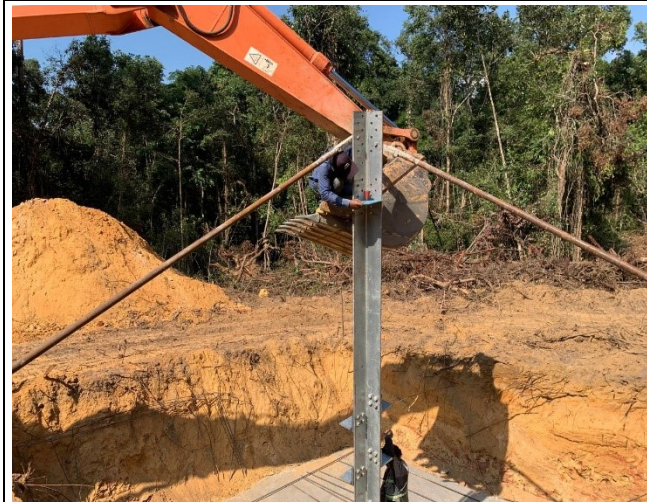
Set stub for the leg B.
