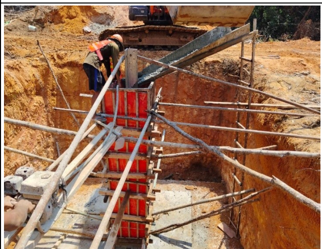
Casting concrete chimney for the leg C.
