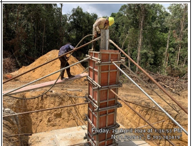
Casting concrete Chimney for the leg C.
