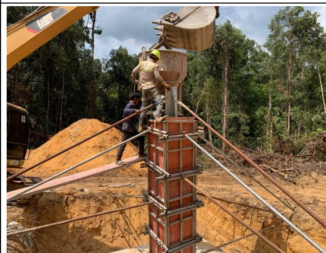
Casting concrete Chimney for the leg C.
