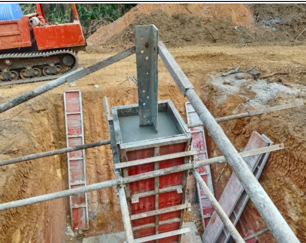
Casting concrete chimney for the leg C.
