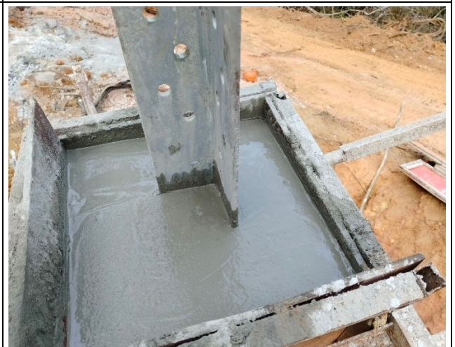
Casting concrete chimney for the leg D.
