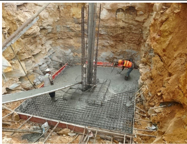
Casting concrete base for the leg D.
