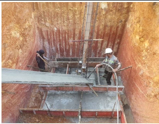
Casting concrete base for the leg D.
