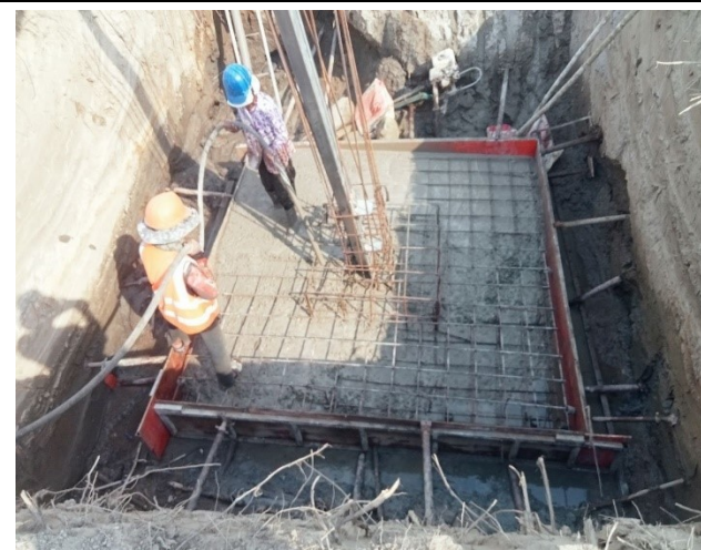
Casting concrete base for the leg B.
