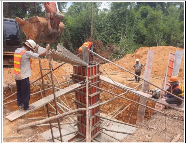
Casting concrete chimney for the leg D.
