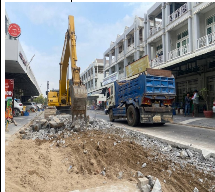
Photo: 11 Soil excavation and concrete road
