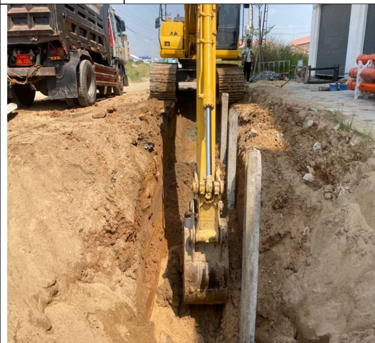
Photo: 05 Soil excavation and concrete road
