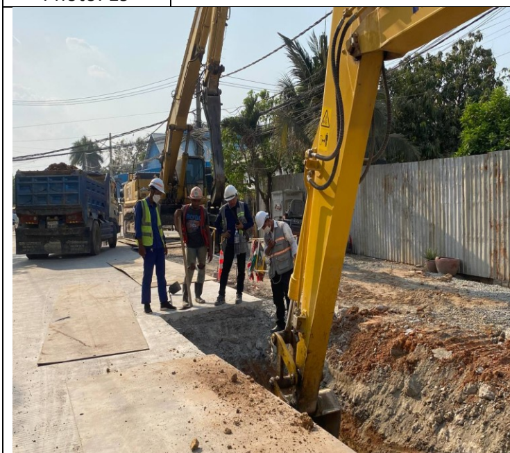
Photo: 21 Soil excavation and concrete road
