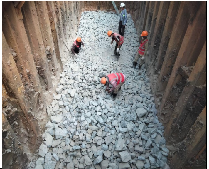
Photo: 02 Manhole Installation activity
