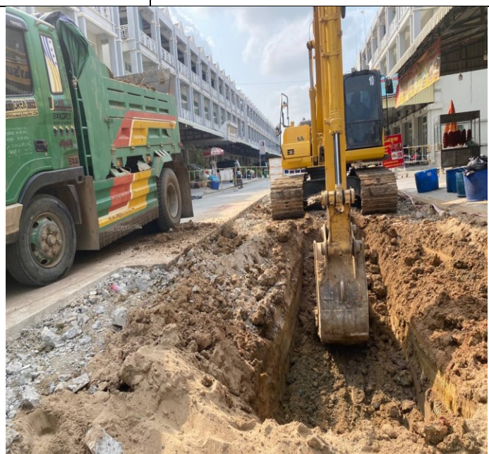
Photo: 16 Soil excavation and concrete road
