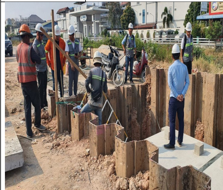
Manhole Installation activity
