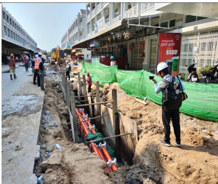
Photo: 20 | Assembly PFP pipes and OFC pipe
