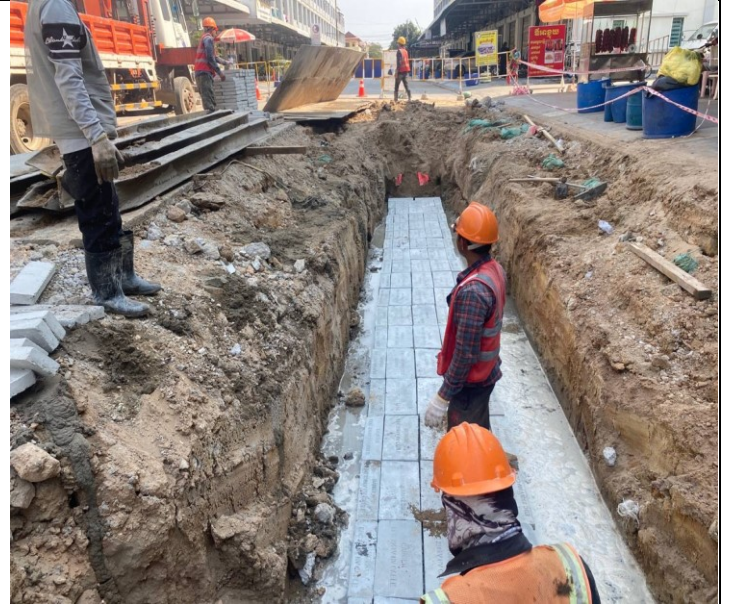
Photo: 10 Laying concrete protection slab and warning tap
