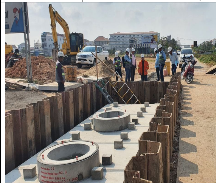
Manhole Installation activity
