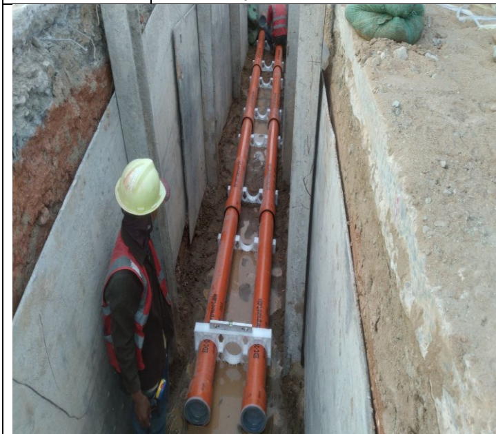
Photo: 03 Assembly PFP pipes and OFC pipe
