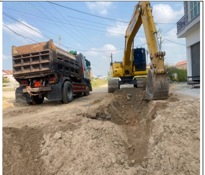
Photo: 02 Soil excavation and concrete road
