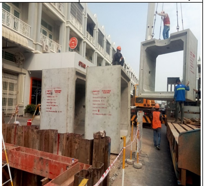
Photo: 06 Manhole Installation activity
