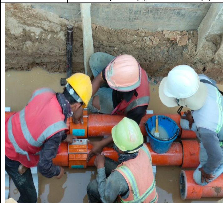
Photo: 15 Assembly PFP pipes and OFC pipe
