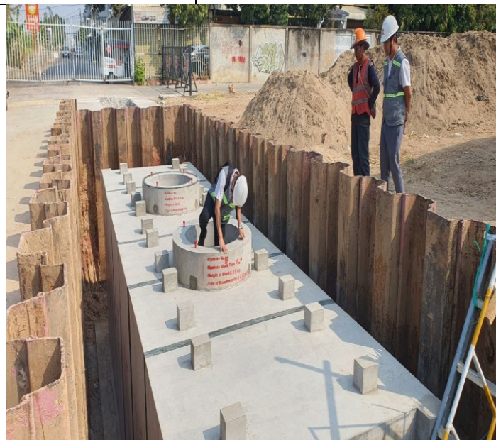
Manhole Installation activity
