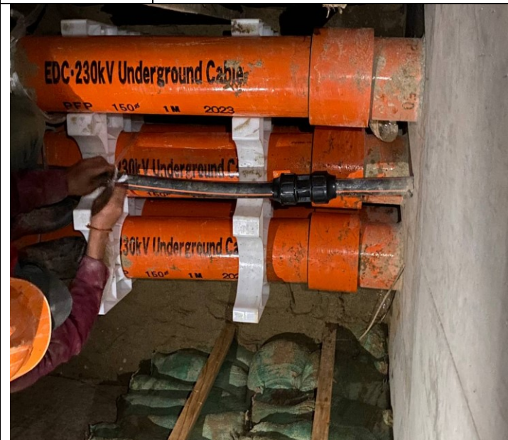
Photo: 11 Assembly PFP pipes and OFC pipe
