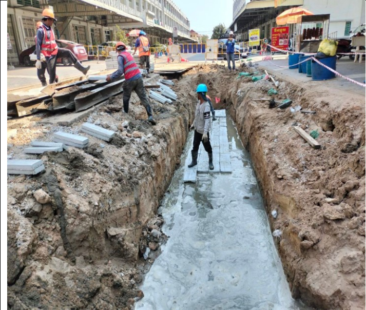
Photo: 09 Laying concrete protection slab and warning tap
