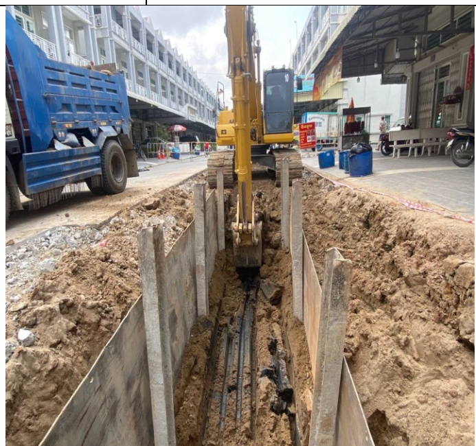
Photo: 18 Soil excavation and concrete road
