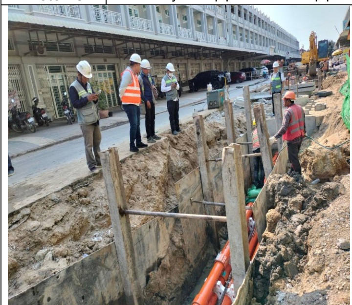
Photo: 21 | Assembly PFP pipes and OFC pipe
