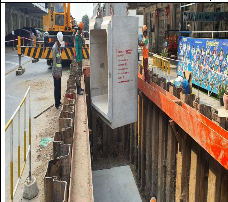
Photo: 05 Manhole Installation activity
