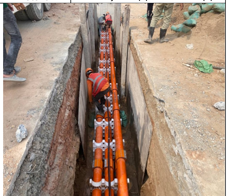
Photo: 06 Assembly PFP pipes and OFC pipe
