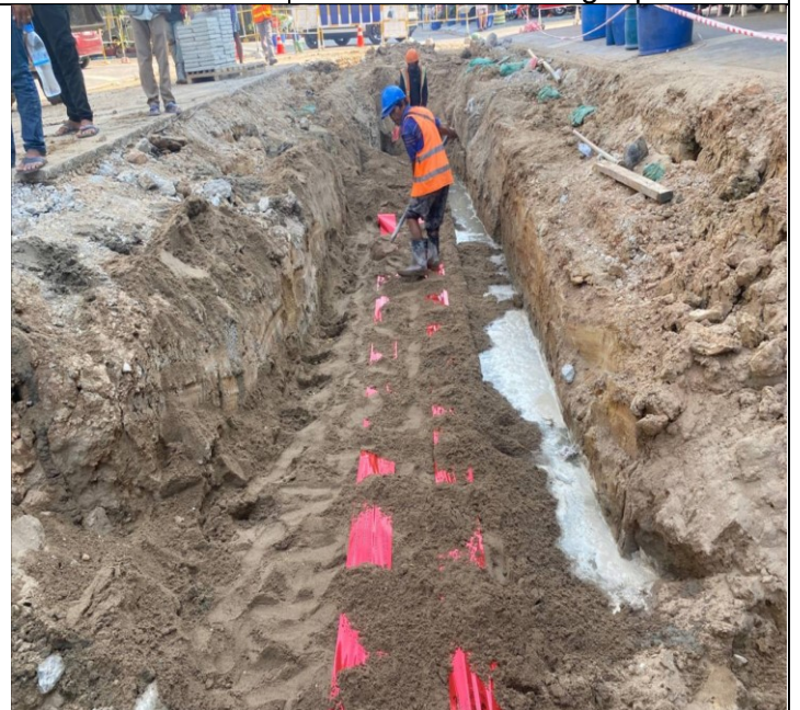
Photo: 12 Laying concrete protection slab and warning tap
