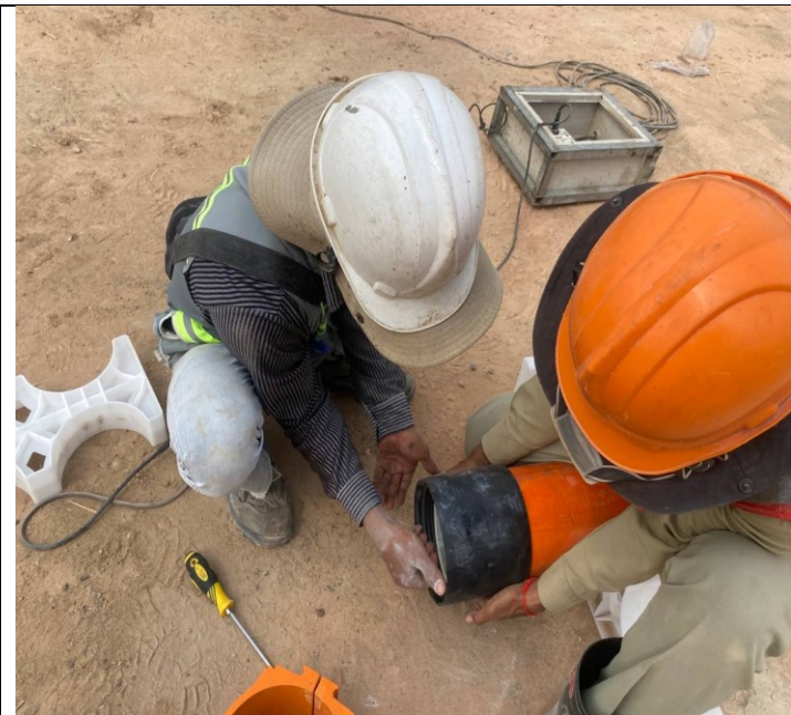
Photo: 07 Assembly PFP pipes and OFC pipe
