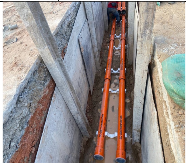
Photo: 04 Assembly PFP pipes and OFC pipe
