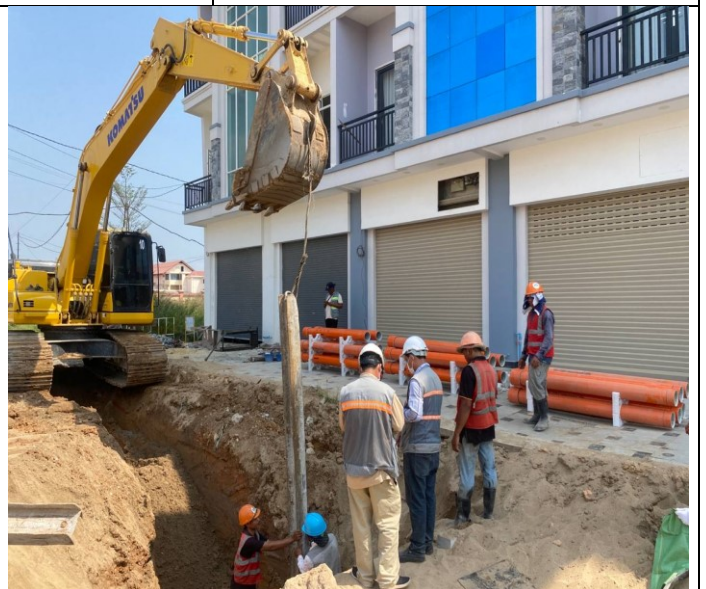
Photo: 04 Soil excavation and concrete road
