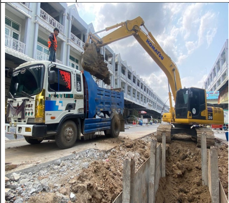
Photo: 17 Soil excavation and concrete road
