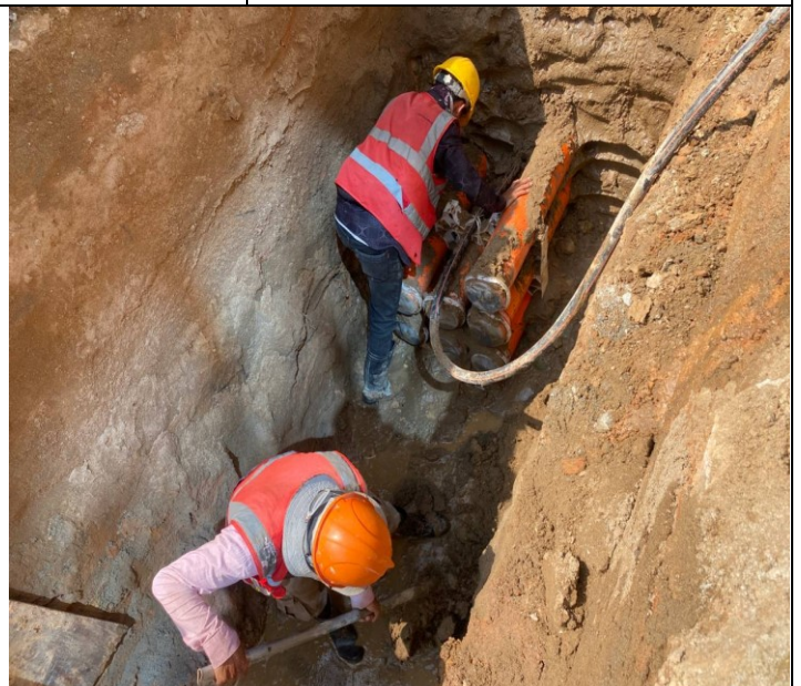
Photo: 12 Assembly PFP pipes and OFC pipe
