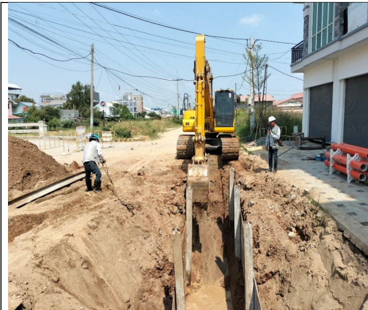
Photo: 07 Soil excavation and concrete road
