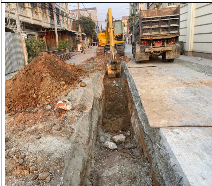
Photo: 23 Soil excavation and concrete road
