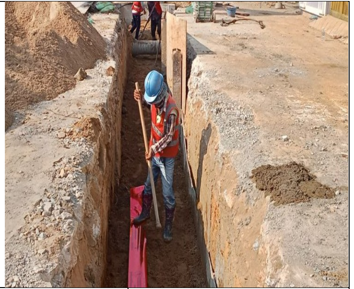
Photo: 08 Laying concrete protection slab and warning tap
