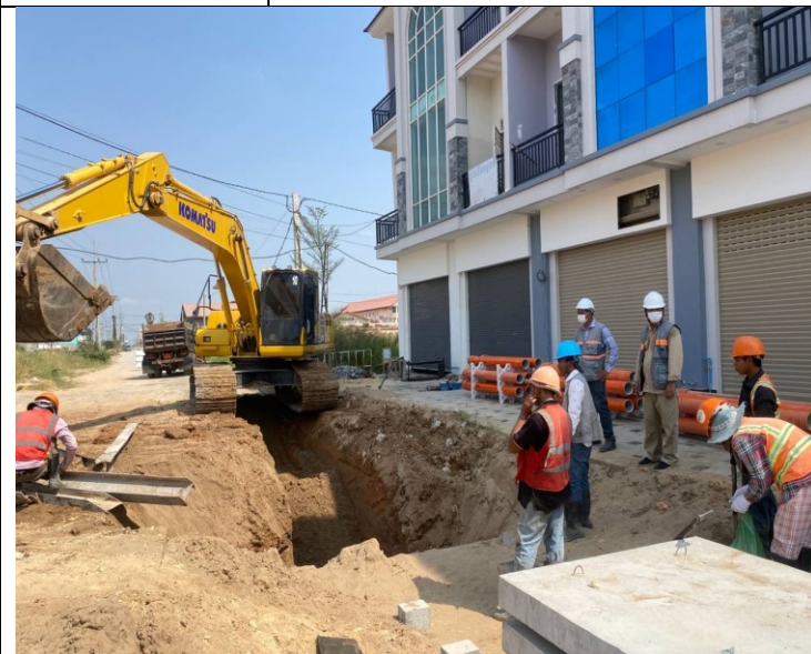
Photo: 03 Soil excavation and concrete road
