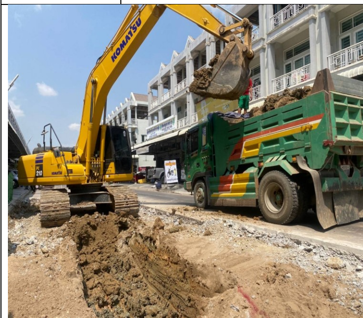
Photo: 15 Soil excavation and concrete road
