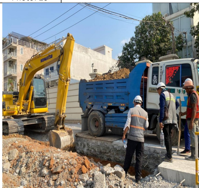
Photo: 22 Soil excavation and concrete road
