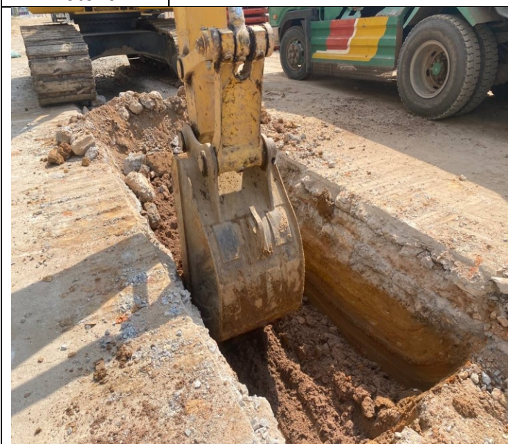
Photo: 09 Soil excavation and concrete road
