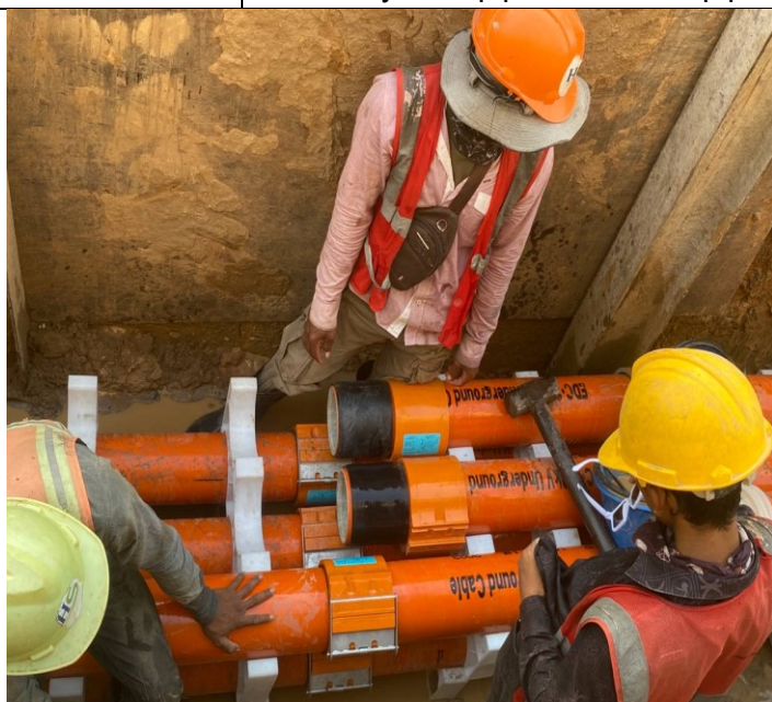
Photo: 18 Assembly PFP pipes and OFC pipe
