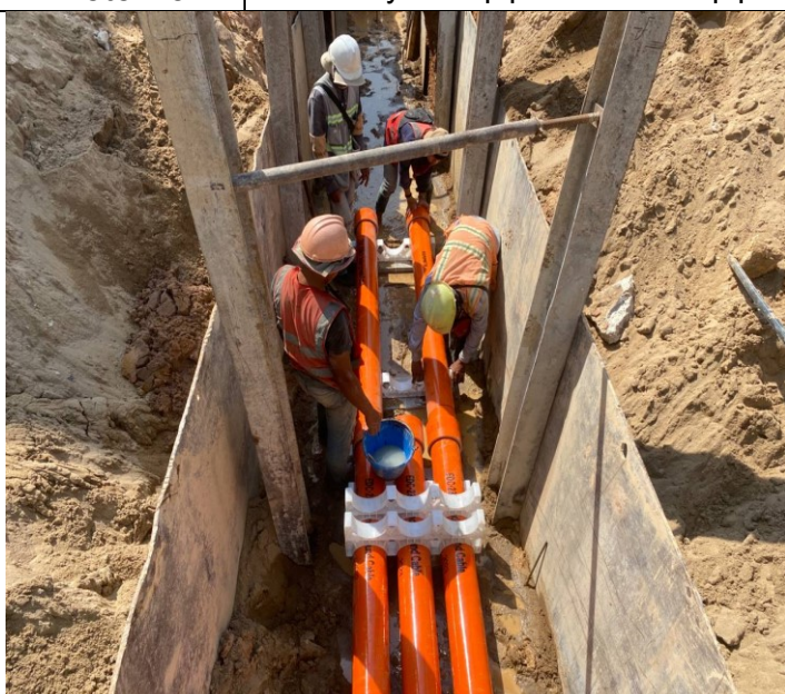
Photo: 22 | Assembly PFP pipes and OFC pipe
