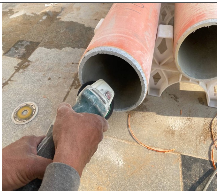
Photo: 14 Assembly PFP pipes and OFC pipe
