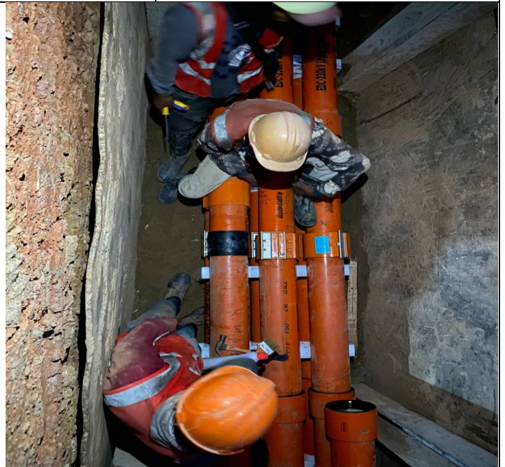
Photo: 10 Assembly PFP pipes and OFC pipe
