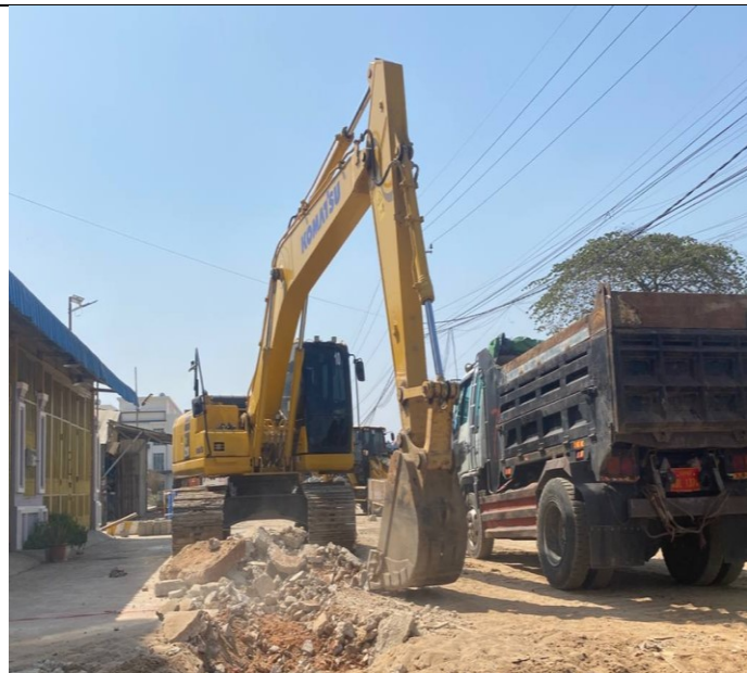
Photo: 08 Soil excavation and concrete road
