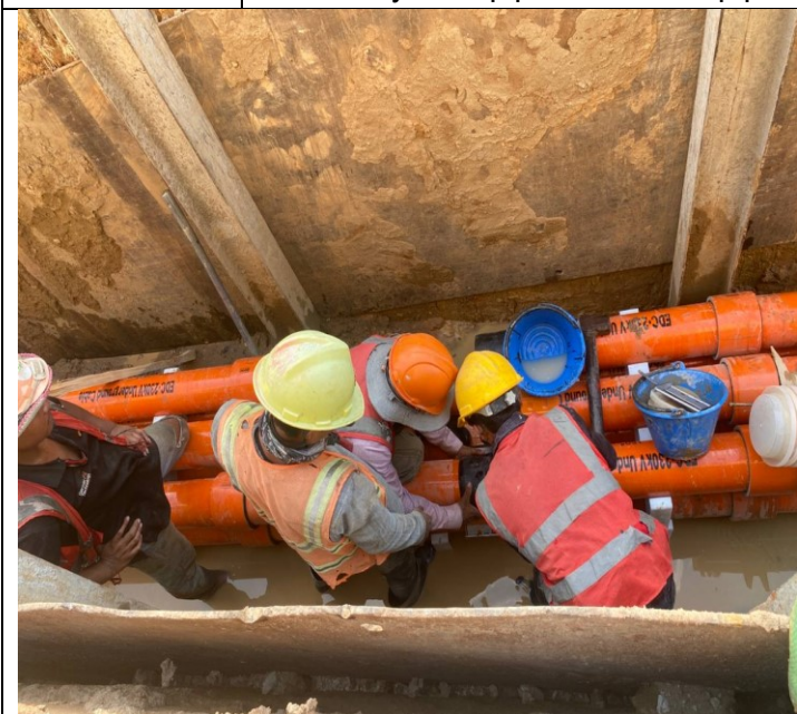
Photo: 17 Assembly PFP pipes and OFC pipe
