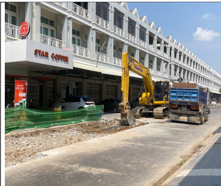
Photo: 13 Soil excavation and concrete road
