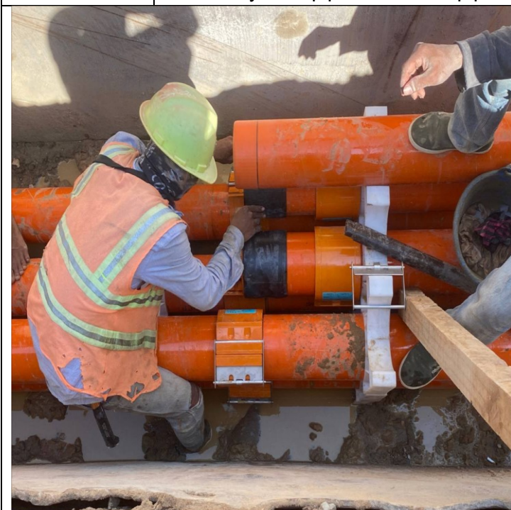
Photo: 23 | Assembly PFP pipes and OFC pipe
