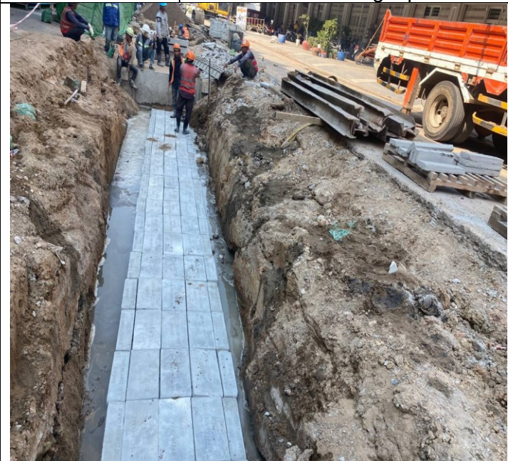
Photo: 11 Laying concrete protection slab and warning tap
