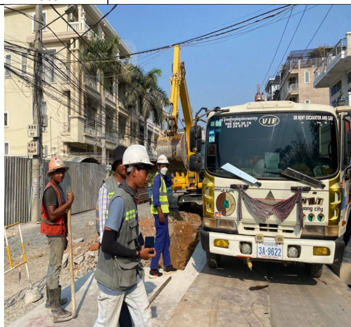
Photo: 24 Soil excavation and concrete road
