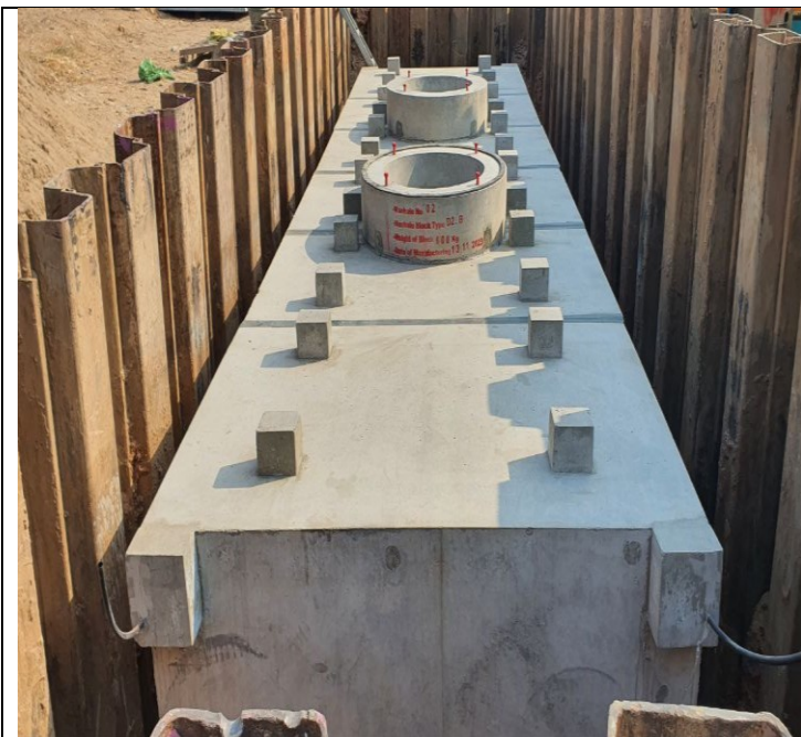
Manhole Installation activity
