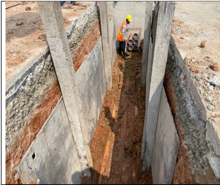
Photo: 01 Assembly PFP pipes and OFC pipe
