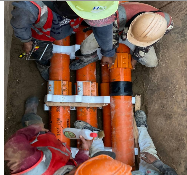
Photo: 09 Assembly PFP pipes and OFC pipe
