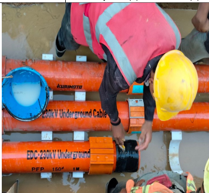
Photo: 16 Assembly PFP pipes and OFC pipe
