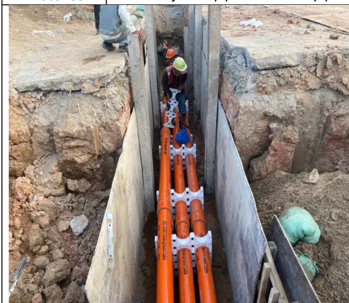
Photo: 05 Assembly PFP pipes and OFC pipe
