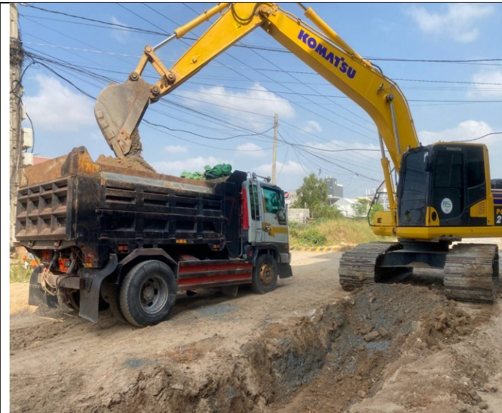
Photo: 01 Soil excavation and concrete road
