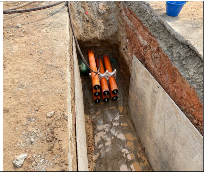
Photo: 02 Assembly PFP pipes and OFC pipe
