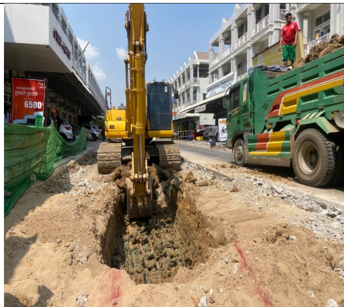
Photo: 14 Soil excavation and concrete road
