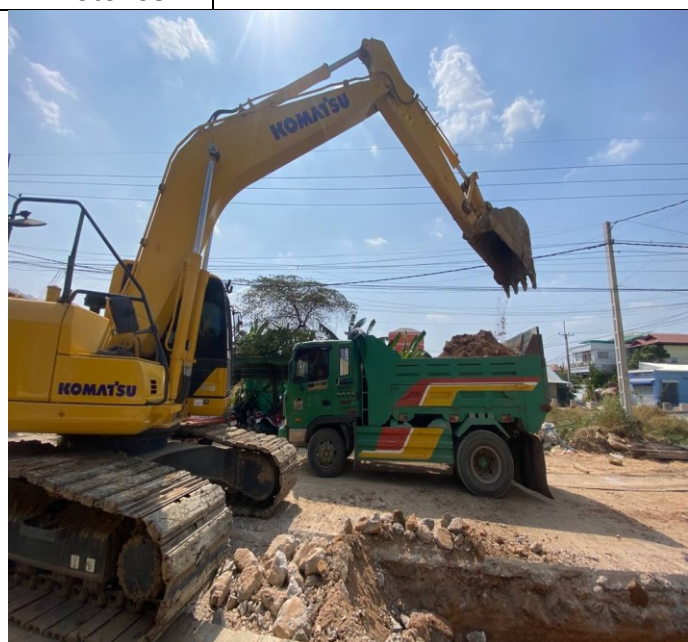
Photo: 10 Soil excavation and concrete road
