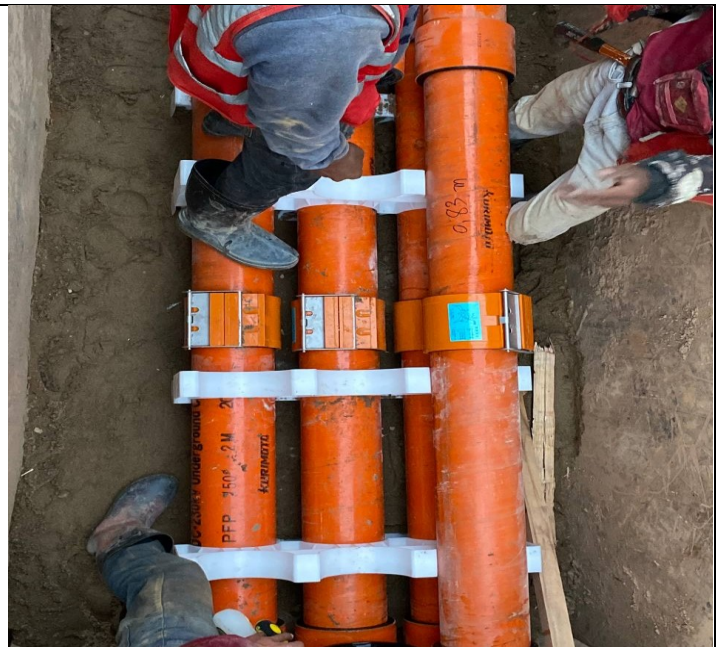
Photo: 08 Assembly PFP pipes and OFC pipe
