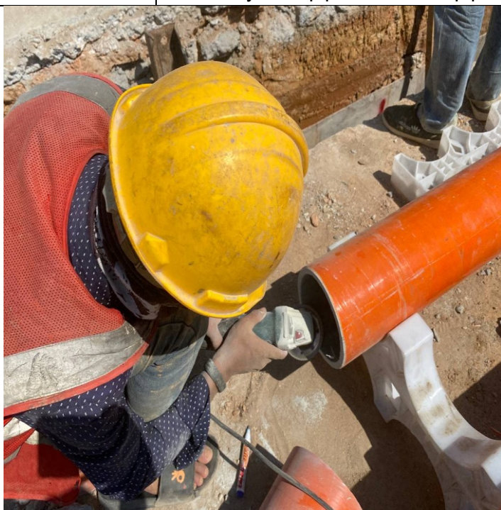
Photo: 24 | Assembly PFP pipes and OFC pipe
