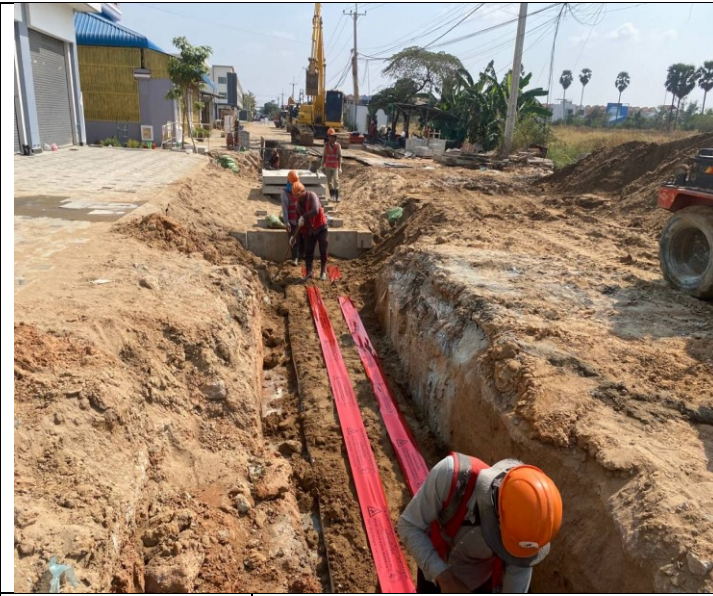
Photo: 07 Laying concrete protection slab and warning tap
