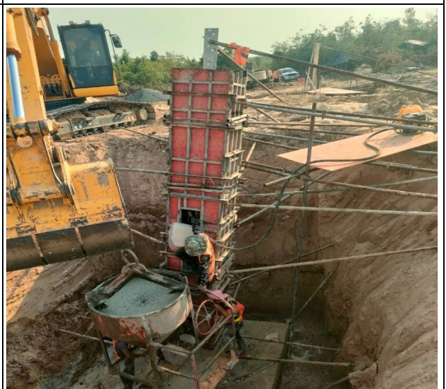
Chimney casting concrete pit leg B.
