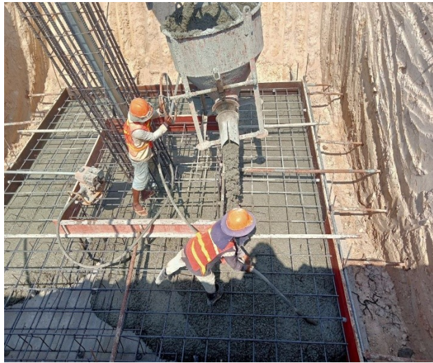
Base casting concrete of the pit leg A.
