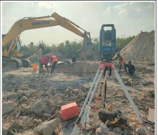
Chimney casting concrete pit leg D.
