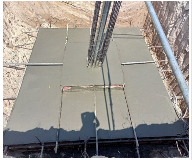
Base casting concrete of the pit leg A.
