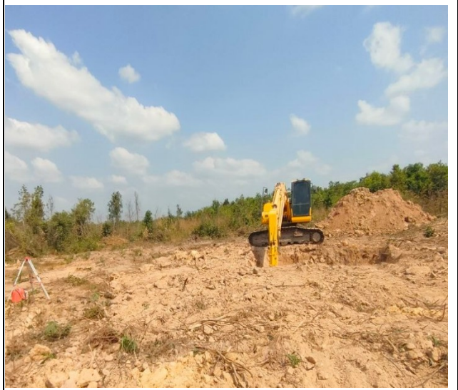
Soil excavation pit leg C.
