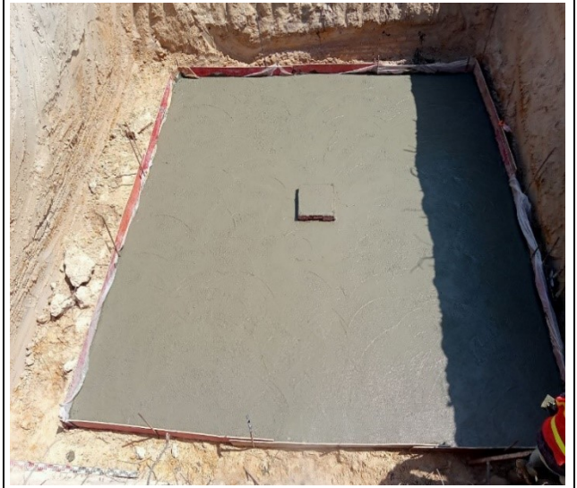
Lean casting concrete pit leg D.
