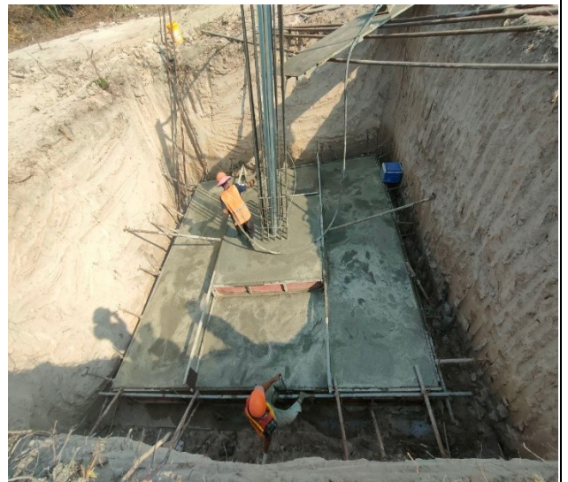
Base concrete of the pit leg B.
