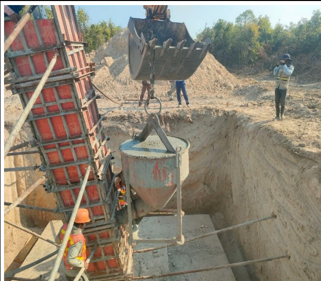
Chimney casting concrete pit leg C.
