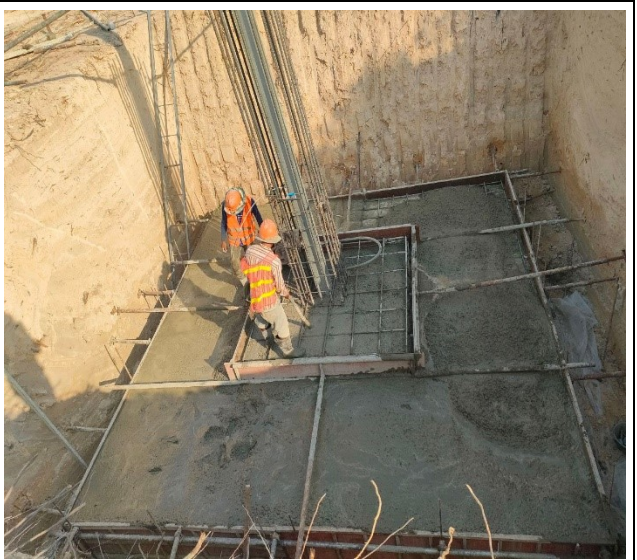
Base casting concrete of the pit leg C.
