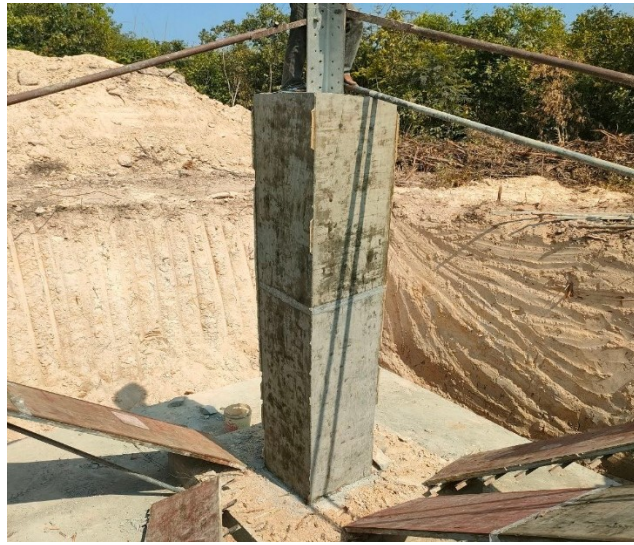
Remove Chimney form box of the pit leg A.
