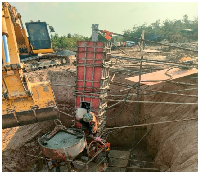
Chimney casting concrete pit leg A.
