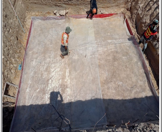
Soil excavation of the pit leg C.
