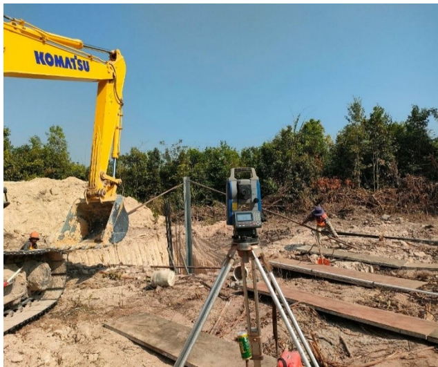
Stub setting of the pit leg A.
