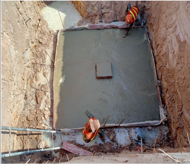
Lean casting concrete pit leg C.
