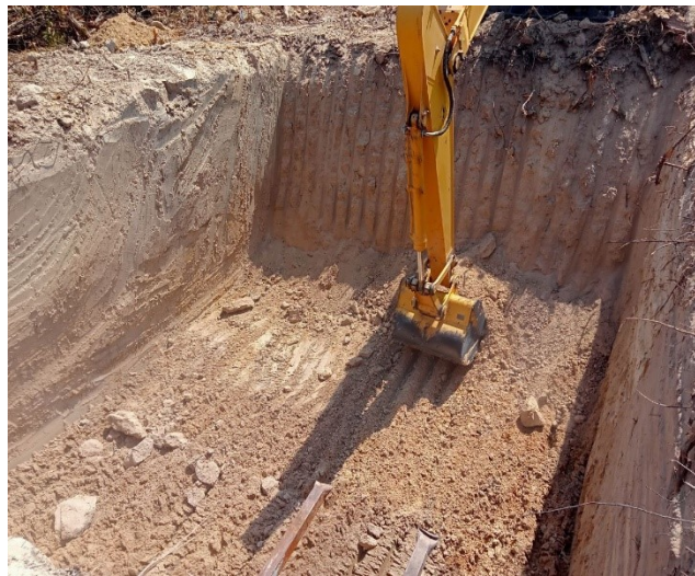
Soil excavation of the pit leg C.
