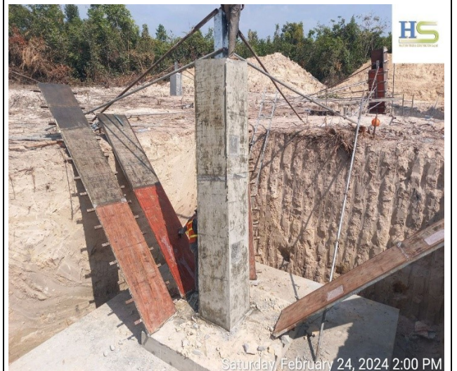
Remove Chimney form box of the pit leg C.
