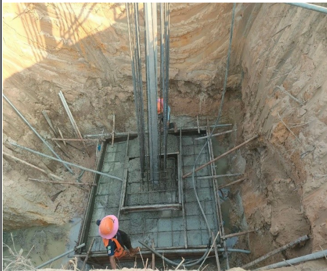
Base casting concrete pit leg C.
