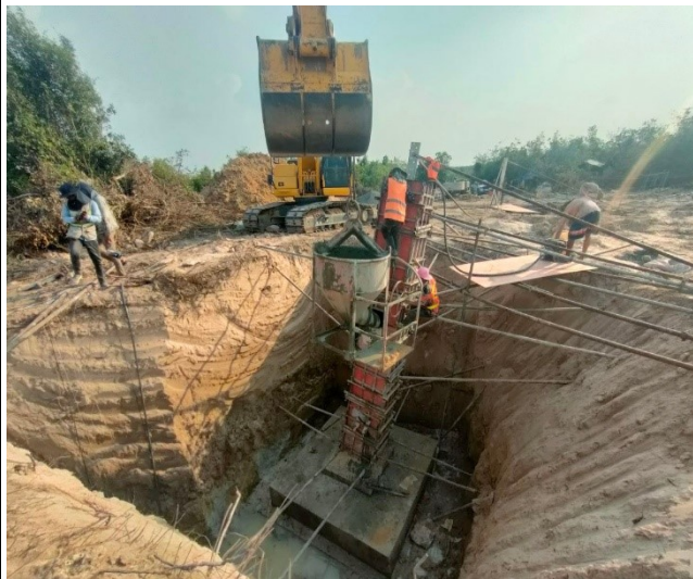
Chimney casting concrete pit leg B.
