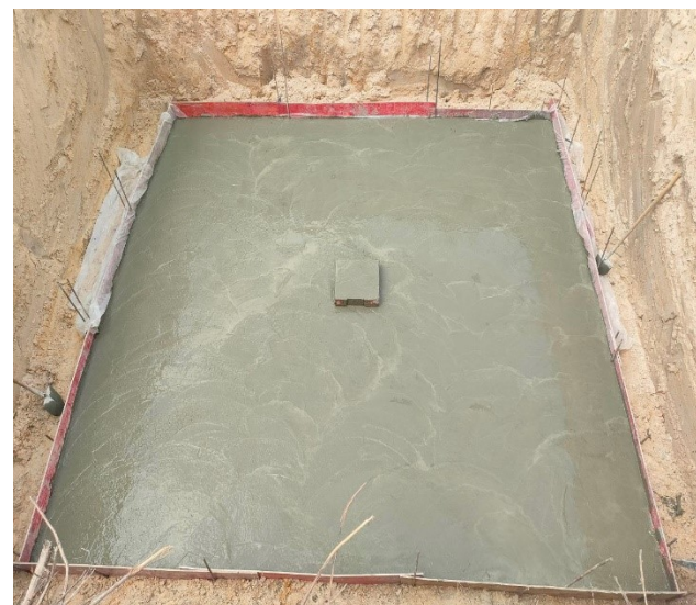
Lean casting concrete pit leg A.
