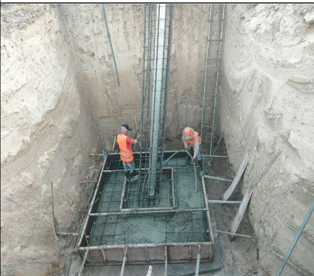
Base casting concrete pit leg C.
