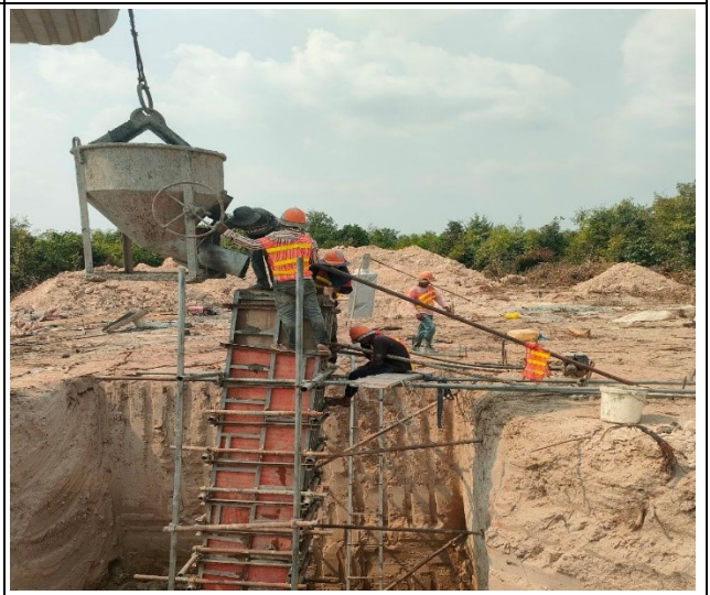
Chimney casting concrete pit leg D.
