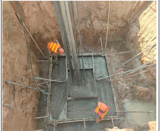
Base casting concrete pit leg C.
