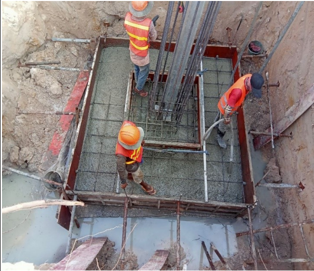
Base casting concrete pit leg A.
