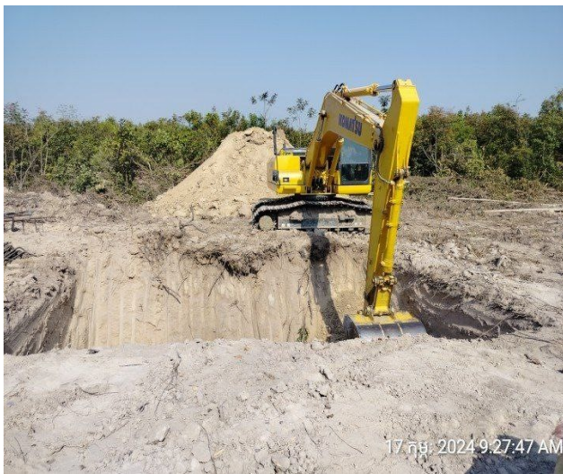
Soil excavation of the pit leg A.
