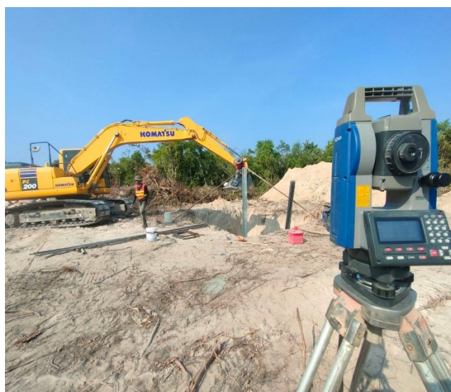
Stub setting of the pit leg C.
