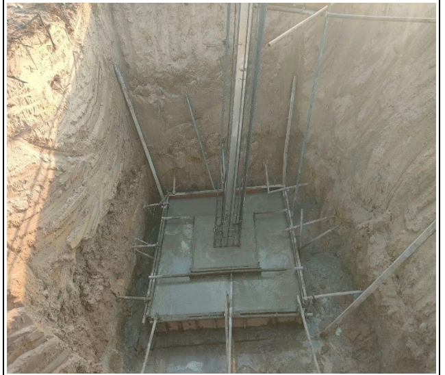
Base casting concrete pit leg B.
