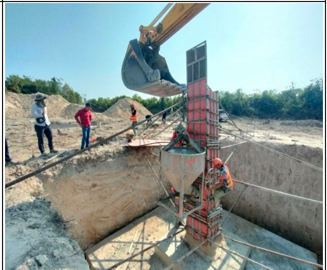
Chimney casting concrete pit leg B.
