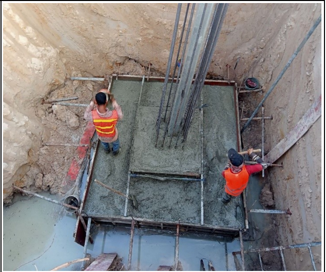
Base casting concrete pit leg B.
