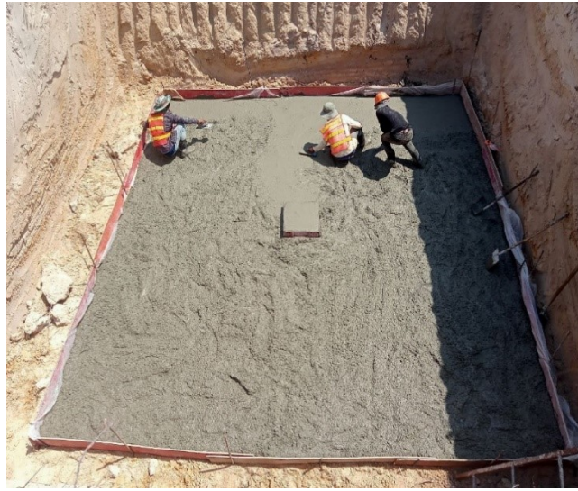
Lean casting concrete pit leg C.
