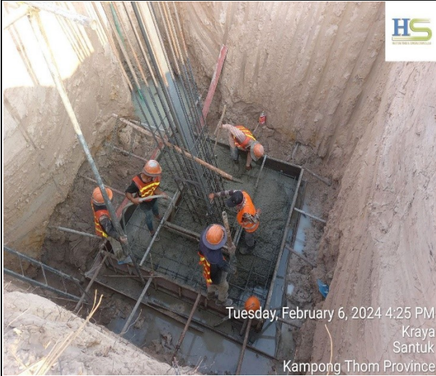
Base casting concrete pit leg D.
