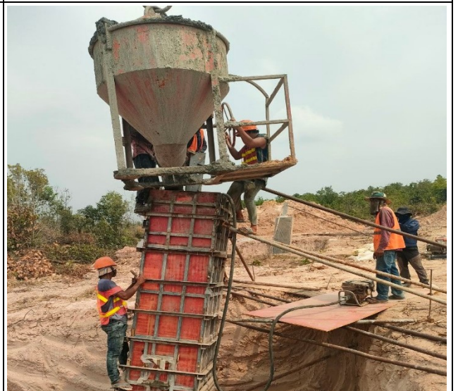
Chimney casting concrete pit leg D.
