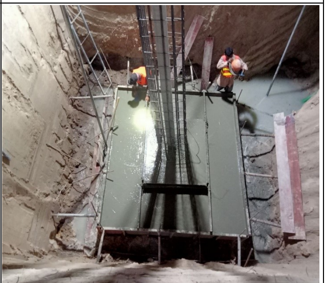
Base casting concrete pit leg C.
