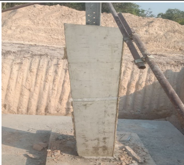
Remove Chimney form box of the pit leg D.
