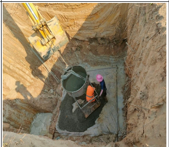
Lean casting concrete pit leg C.
