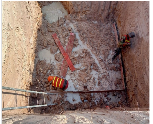
Soil excavation pit leg D.
