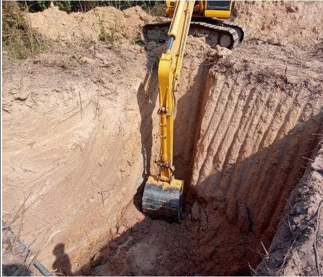
Soil excavation pit leg A.
