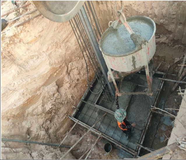
Base casting concrete pit leg D.
