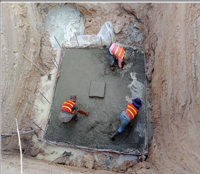
Lean casting concrete pit leg A.
