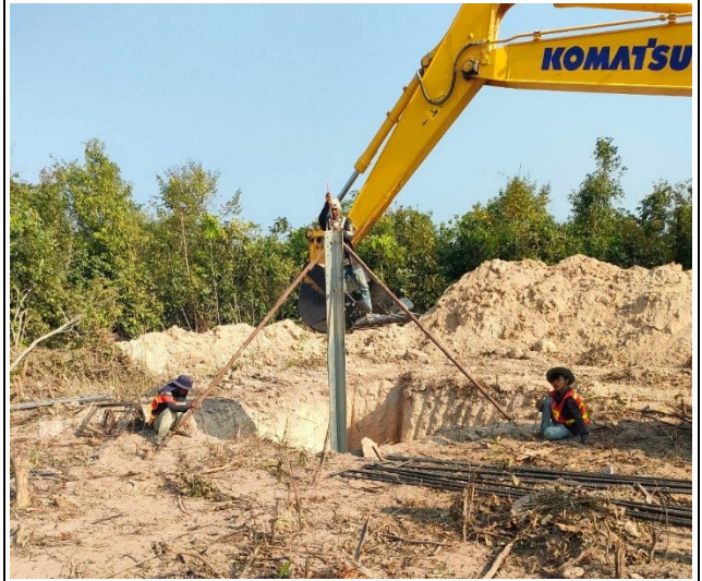
Stub setting pit leg B.
