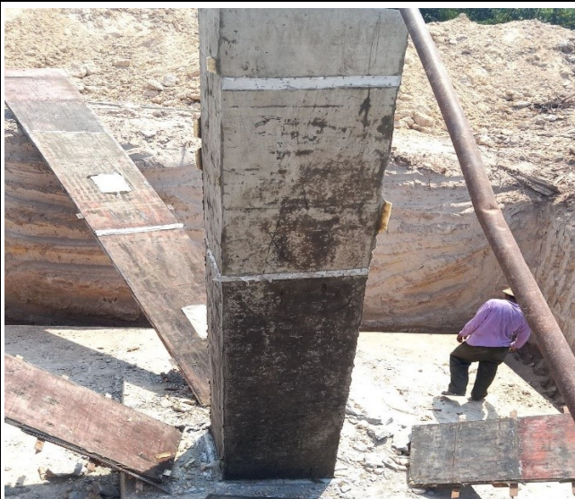
Remove chimney form box of the pit leg D.
