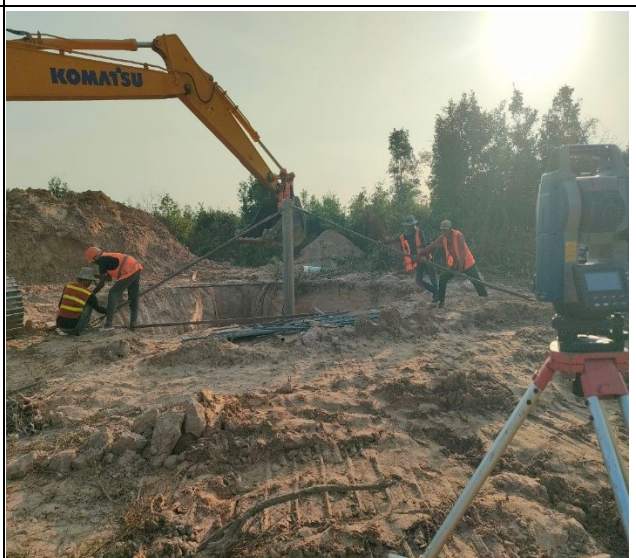
Stub setting pit leg D.
