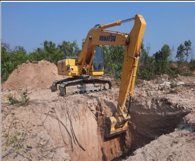
Soil excavation pit leg A.
