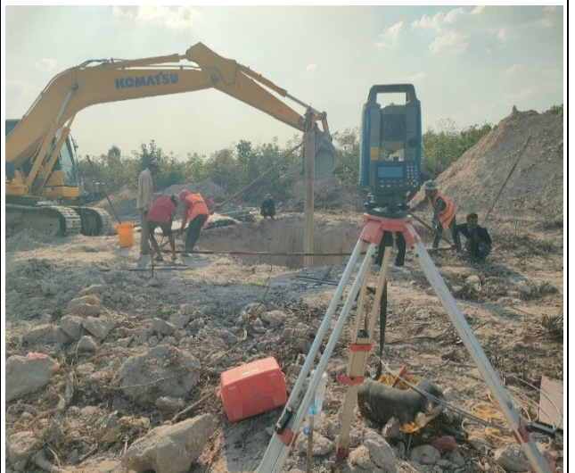
Stub setting of the pit leg B.
