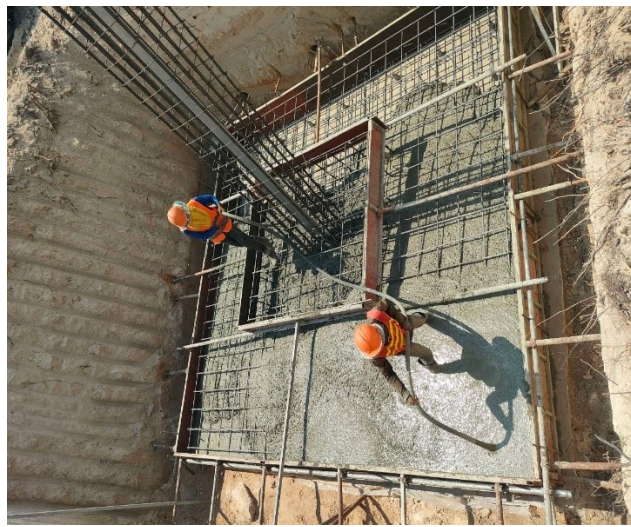
Base casting concrete of the pit leg B.
