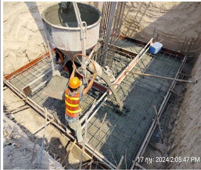
Base concrete of the pit leg B.
