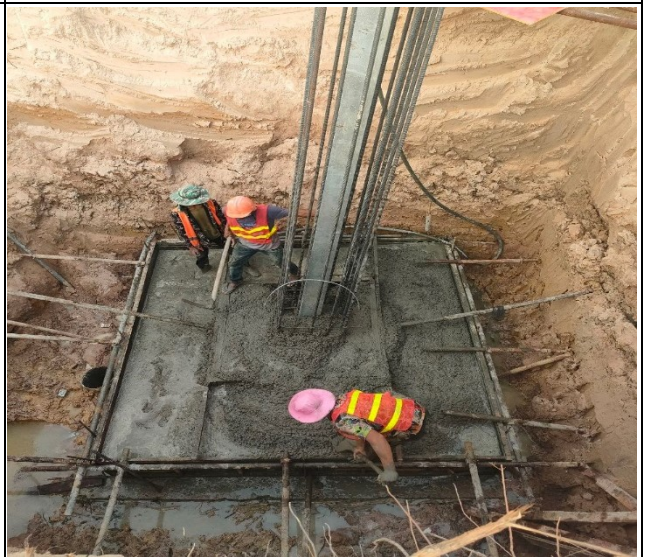
Base casting concrete pit leg A.
