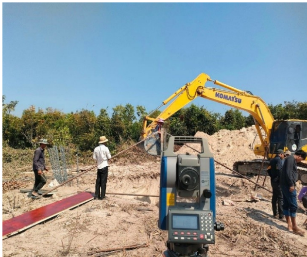
Stub setting of the pit leg A.
