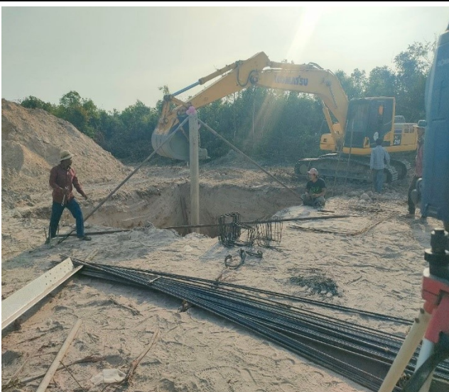
Stub setting of the pit leg C.
