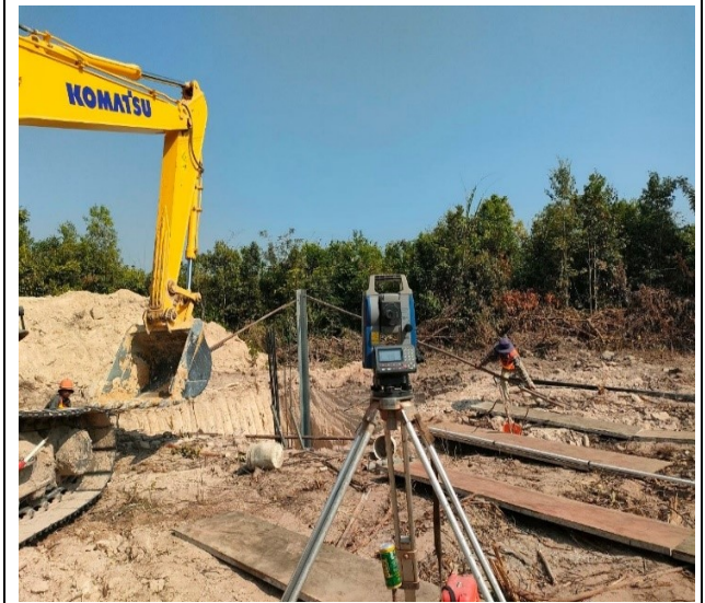
Stub setting of the pit leg D.
