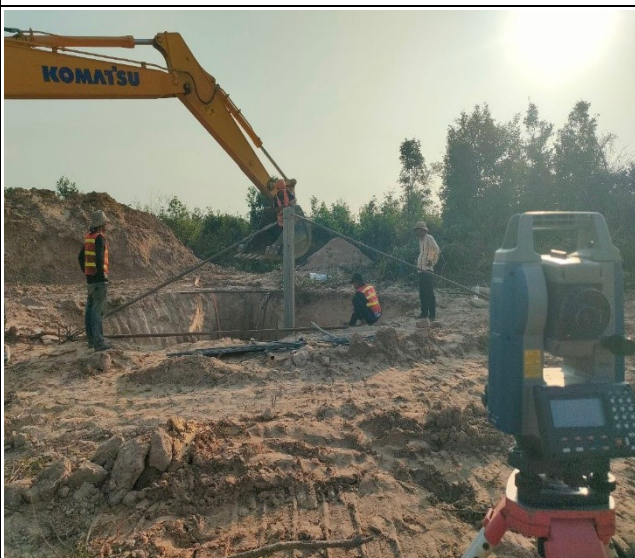
Stub setting pit leg A.
