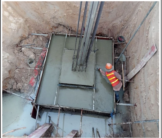
Base casting concrete pit leg A.
