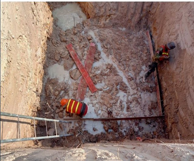
Soil excavation pit leg C.
