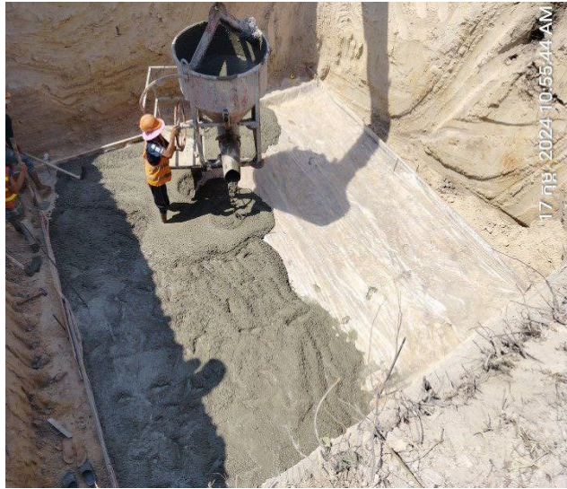
Lean concrete of the pit leg C.
