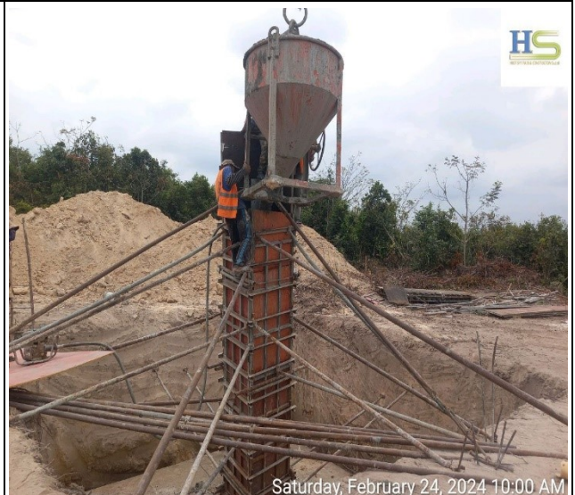
Chimney casting concrete pit leg D.
