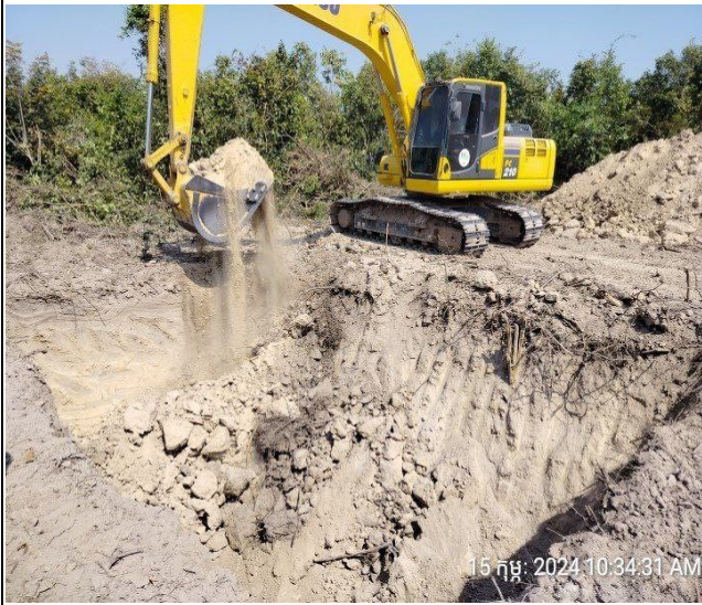
Soil excavation of the pit leg A.
