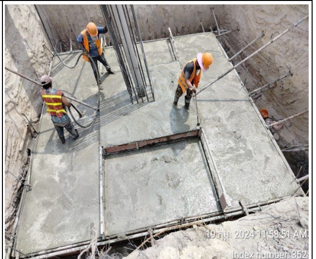
Base concrete of the pit leg A.
