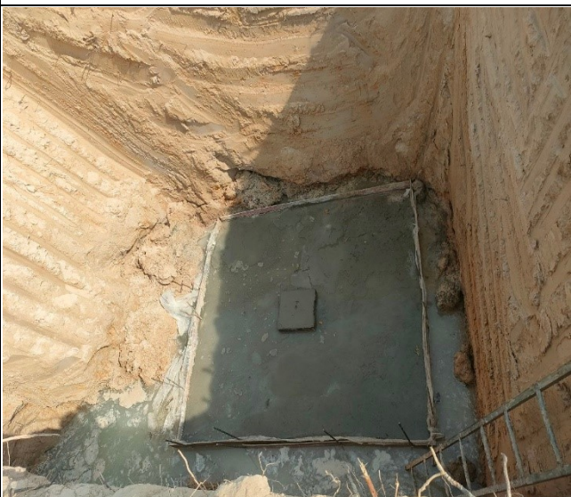
Lean casting concrete pit leg B.
