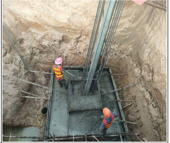
Base casting concrete pit leg D.
