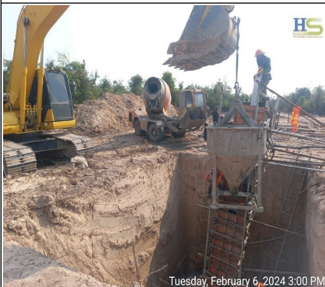
Chimney casting concrete pit leg A.
