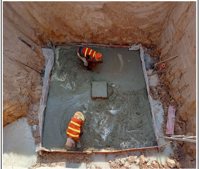
Lean casting concrete pit leg D.
