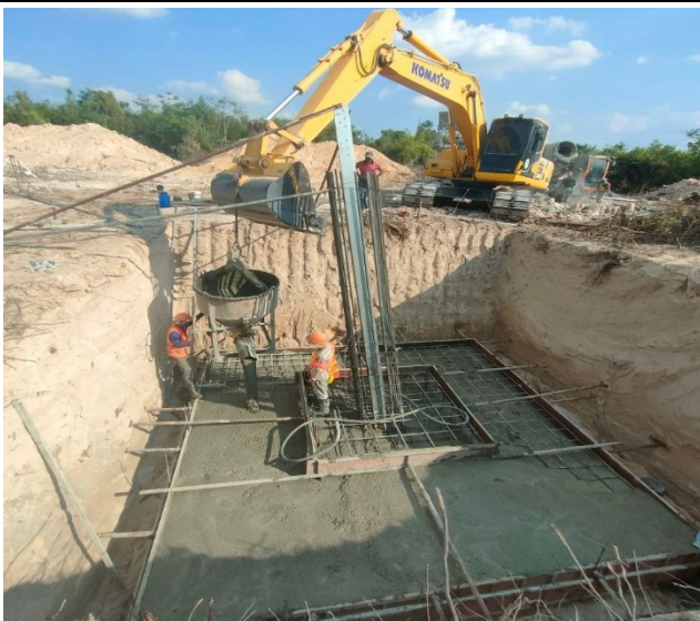
Base casting concrete of the pit leg C.
