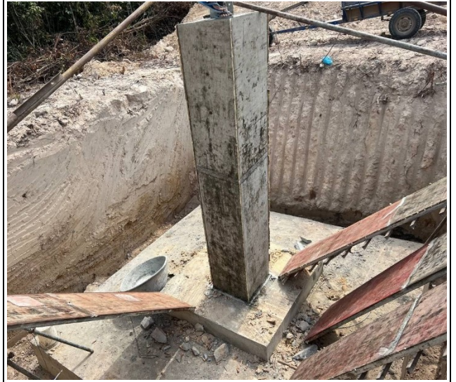
Remove Chimney form box of the pit leg B.
