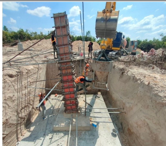
Chimney casting concrete of the pit leg C.
