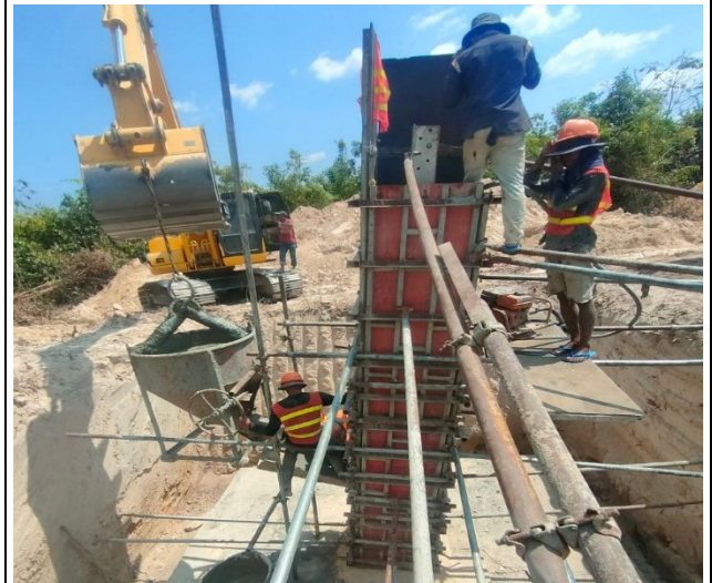
Chimney casting concrete of the pit leg B.
