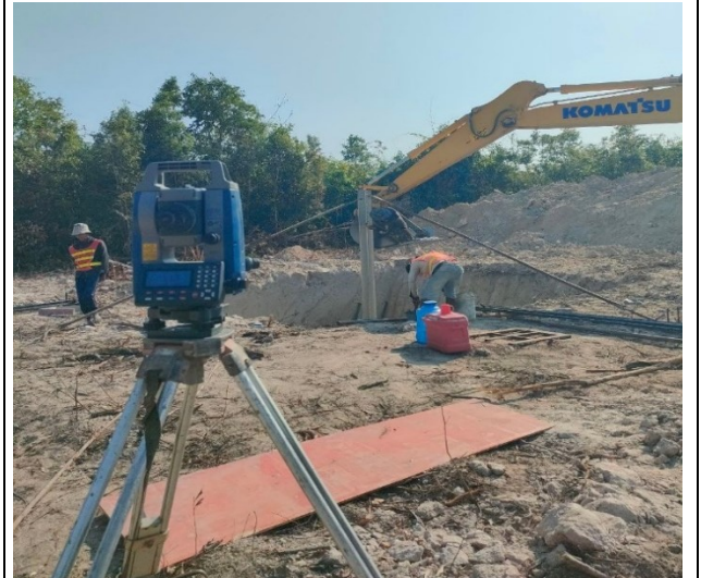
Stub setting of the pit leg B.
