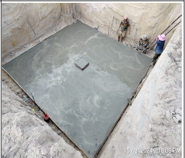
Lean concrete of the pit leg B.
