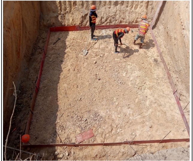
Soil excavation of the pit leg B.
