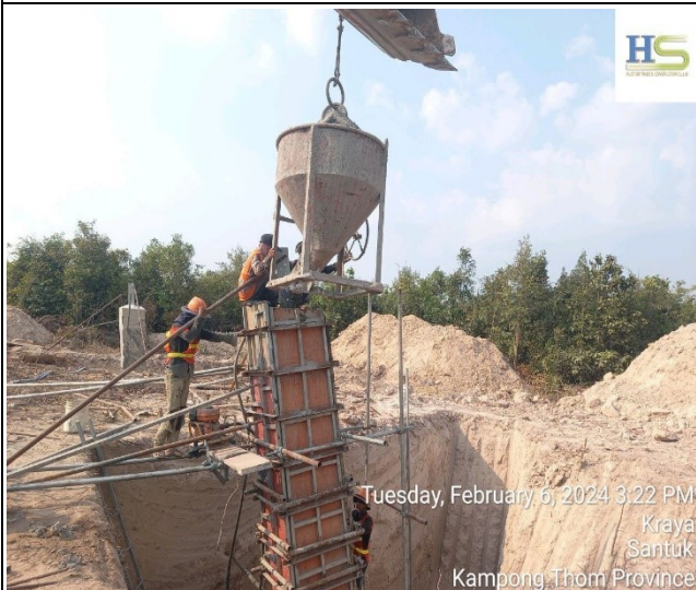
Chimney casting concrete pit leg C.
