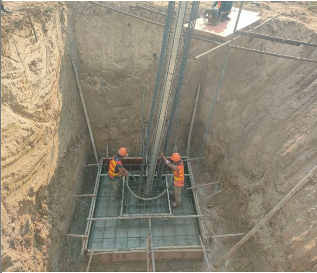
Base casting concrete pit leg B.
