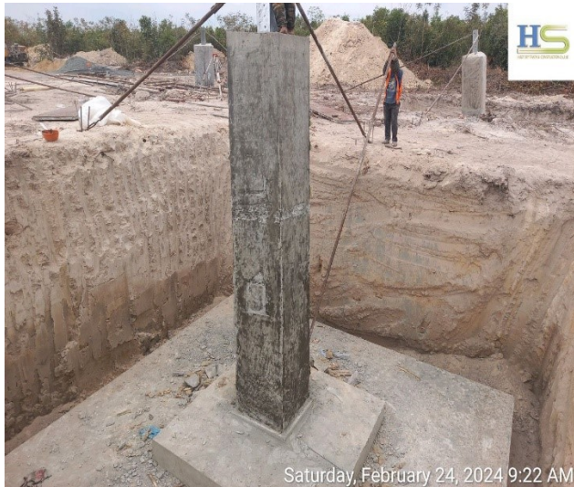
Remove chimney form box of the pit leg C.
