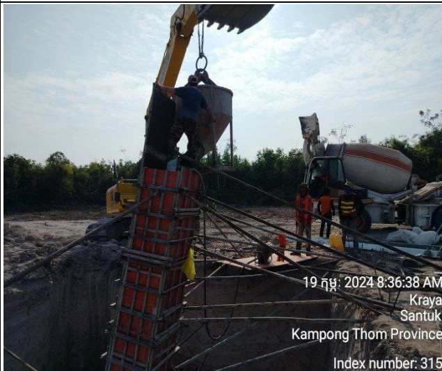
Chimney casting concrete pit leg A.
