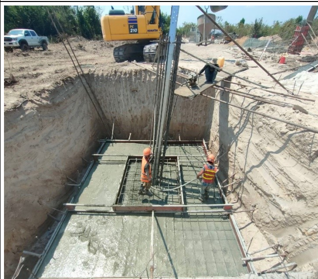
Chimney casting concrete pit leg C.
