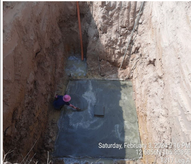
Lean casting concrete pit leg A.
