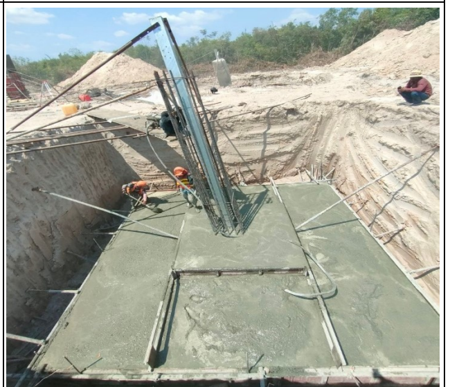
Chimney casting concrete pit leg C.
