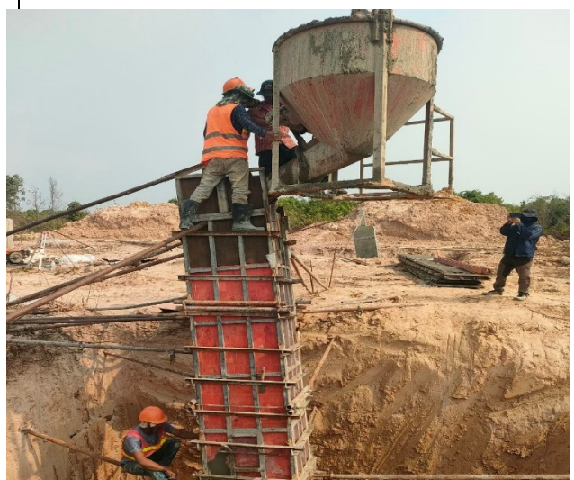
Chimney casting concrete pit leg C.
