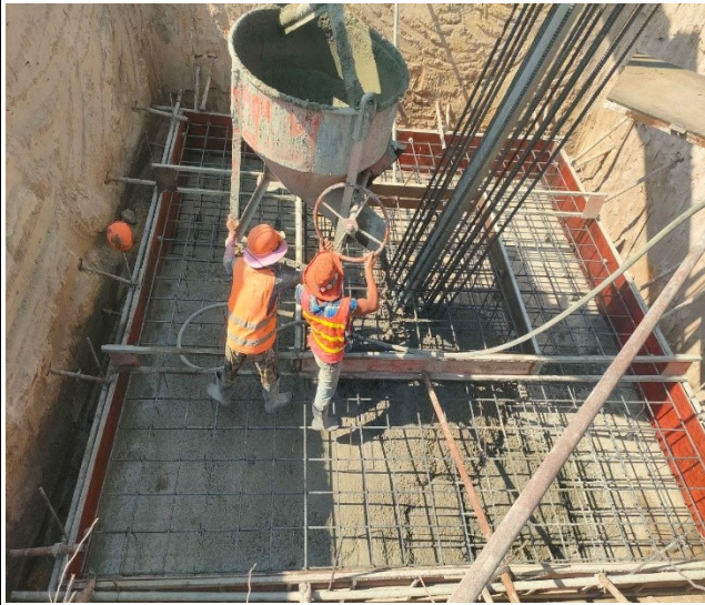
Base casting concrete of the pit leg D.
