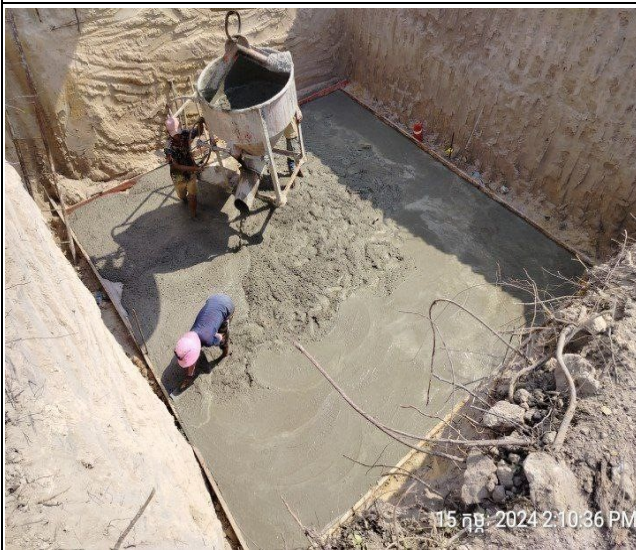
Lean concrete of the pit leg A.
