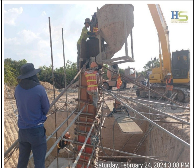
Chimney casting concrete of the pit leg D.
