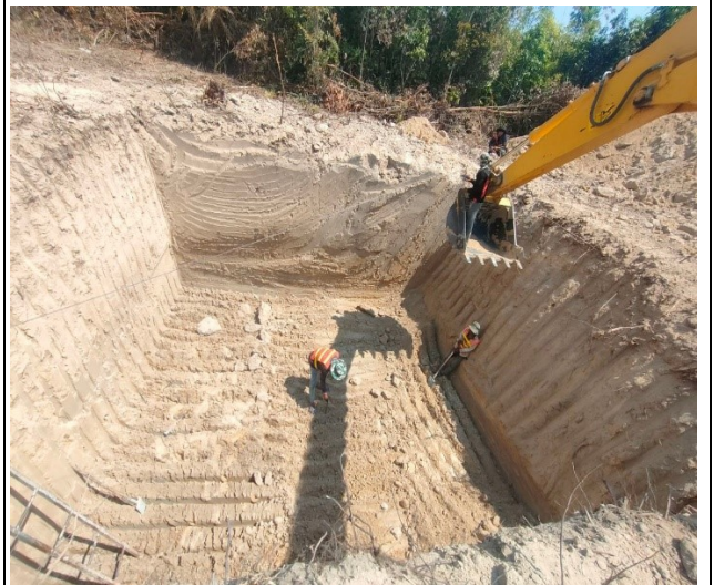
Soil excavation of the pit leg A.
