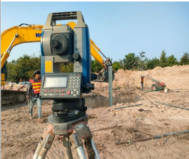
Stub setting pit leg A.
