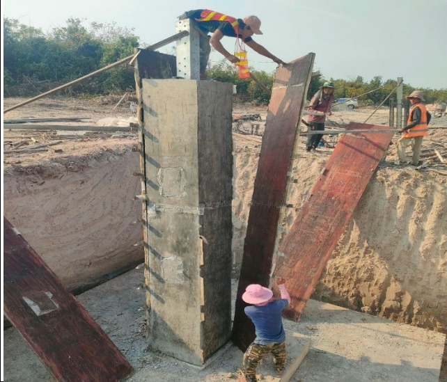
Remove chimney form box of the pit leg B.
