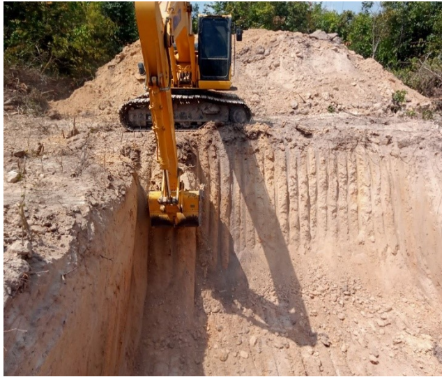
Soil excavation of the pit leg B.
