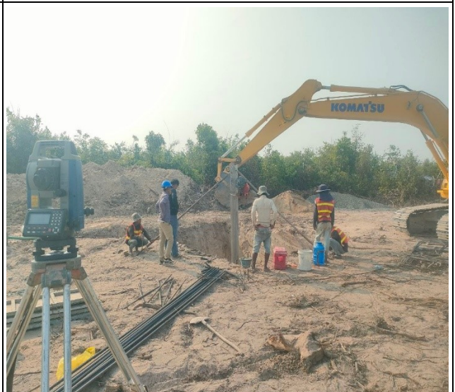
Stub setting pit leg D.
