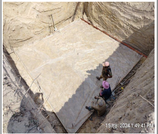
Soil excavation of the pit leg B.
