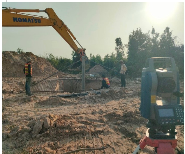
Stub setting pit leg C.
