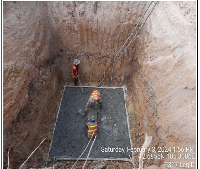
Lean casting concrete pit leg D.
