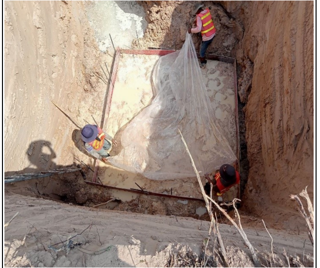
Soil excavation pit leg B.
