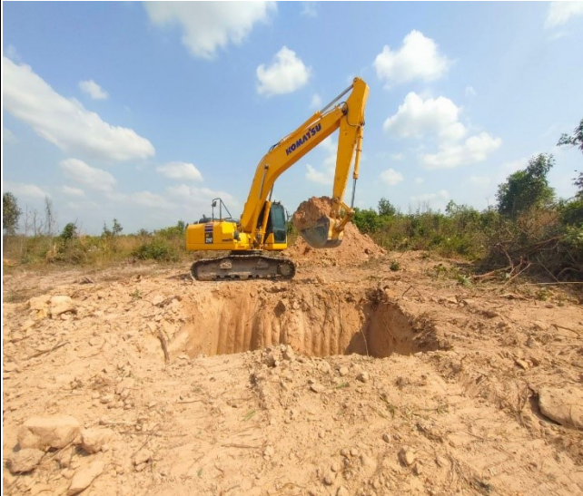
Soil excavation pit leg B.
