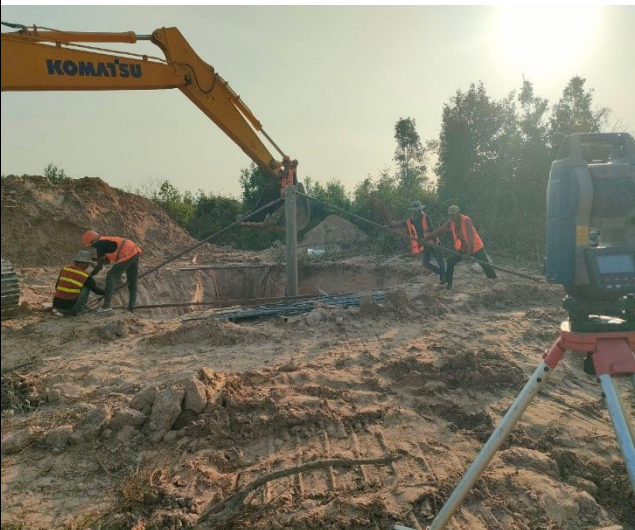
Stub setting pit leg B.
