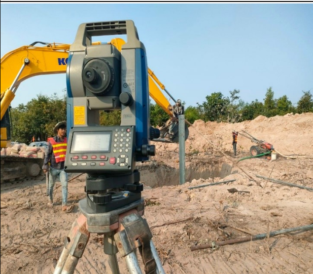
Stub setting pit leg C.
