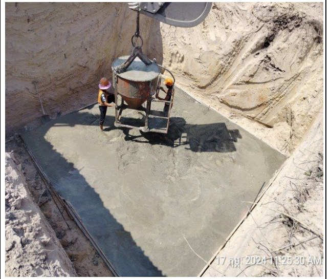
Lean concrete of the pit leg D.
