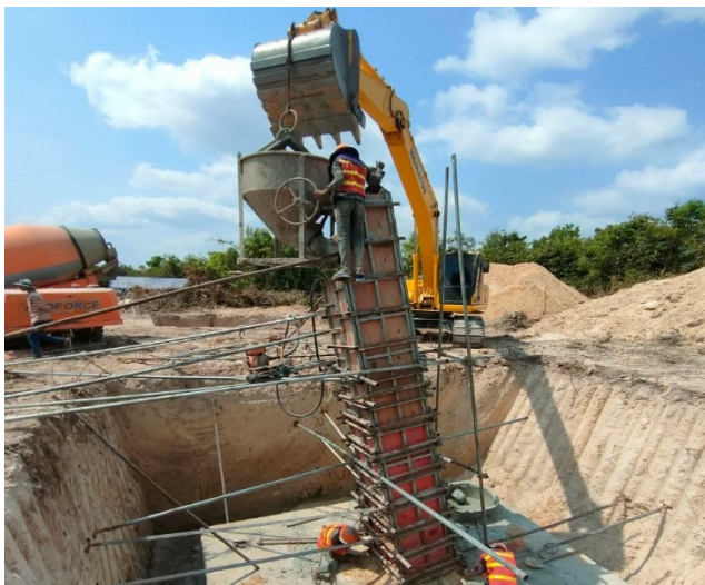
Chimney casting concrete of the pit leg A.
