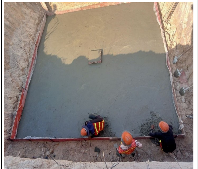
Chimney casting concrete pit leg B.
