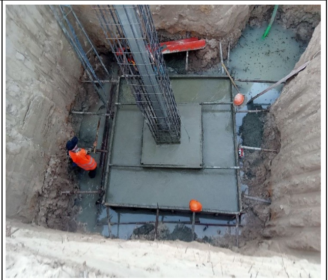
Base casting concrete pit leg D.
