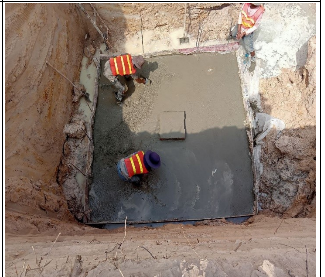
Lean casting concrete pit leg B.
