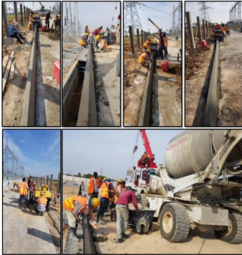
Road Kerb for Substation
