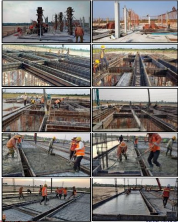
Column Beam & Slab Roof of Control Building for Substation
