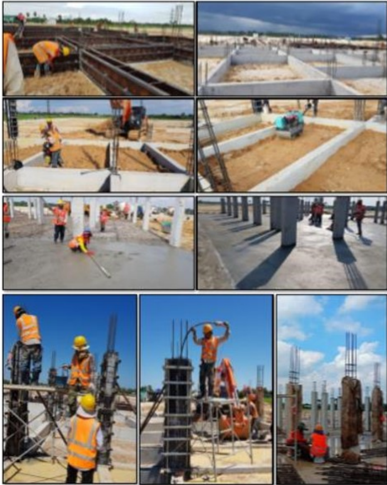
Ground Floor Beam & Column of Control Building for Substation
