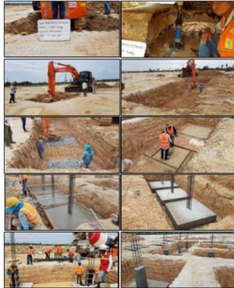
Footing of Control Building for Substation
