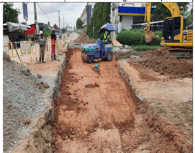
Photo: 06 Sand backfilling and compaction
