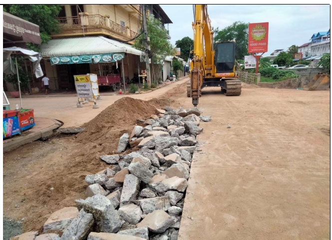
Photo: 02 Demolition of concrete road
