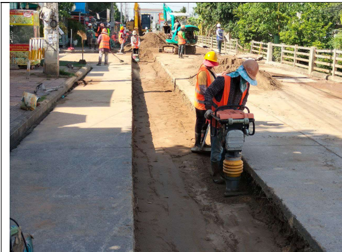
Photo: 11 Sand backfilling and compaction
