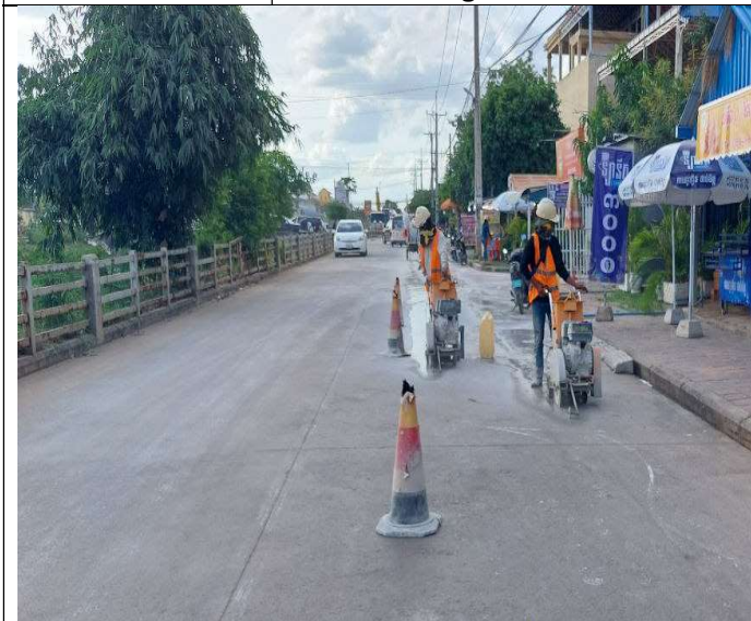
Photo: 09 Saw cutting of concrete road
