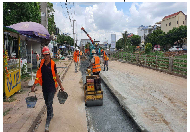
Base course backfilling and compaction
