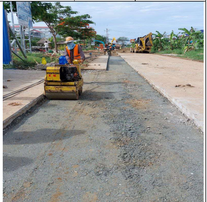
Base course backfilling and compaction
