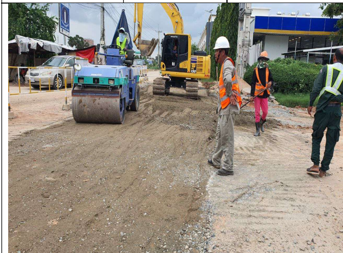
Base course backfilling and compaction
