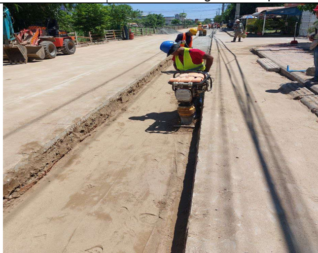
Photo: 14 Sand backfilling and compaction
