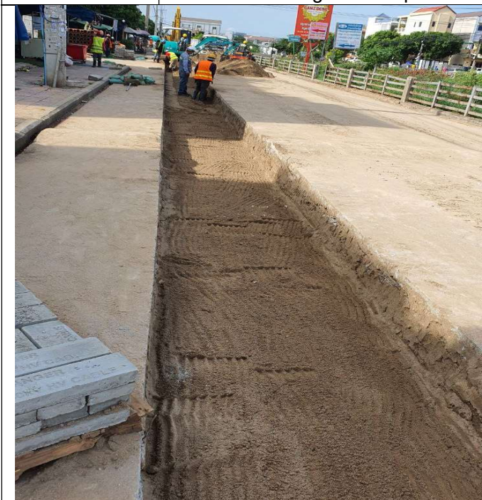
Photo: 15 Sand backfilling and compaction
