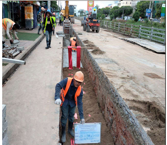
Photo: 010 Laying concrete protection slab and warning tap
