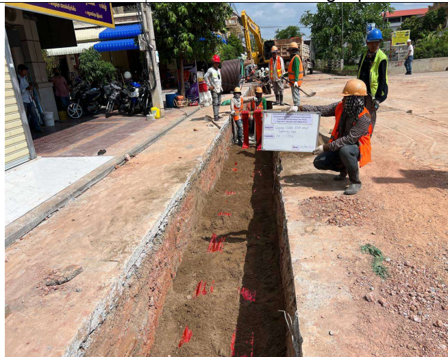
Photo: 03 Laying concrete protection slab and warning tap
