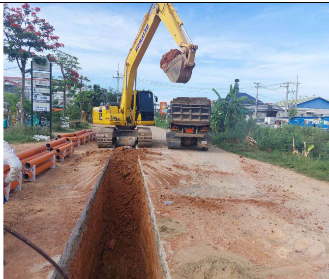
Photo: 10 Soil excavation and concrete road
