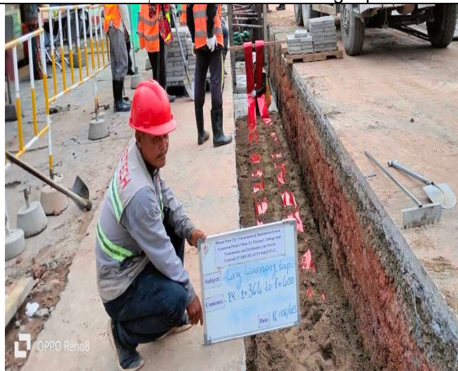
Photo: 05 Laying concrete protection slab and warning tap
