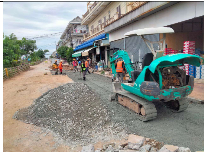
Base course backfilling and compaction
