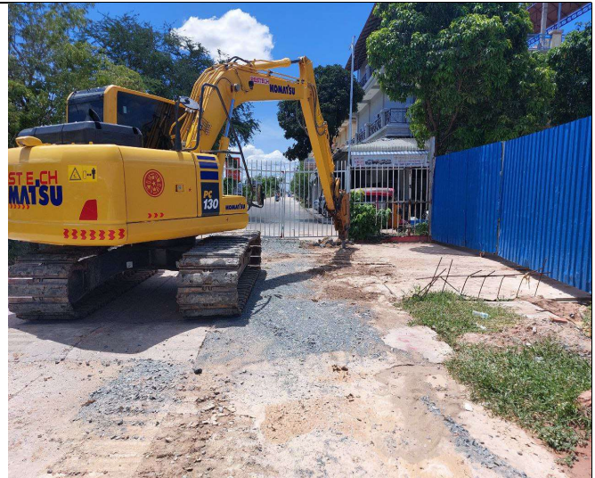
Demolition of concrete road
