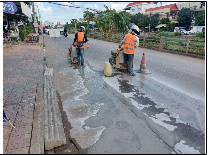
Photo: 08 Saw cutting of concrete road
