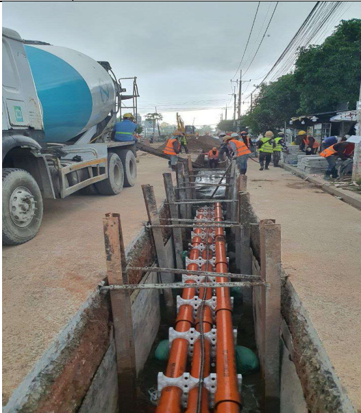
Photo: 21 CBS casting (mortar)
