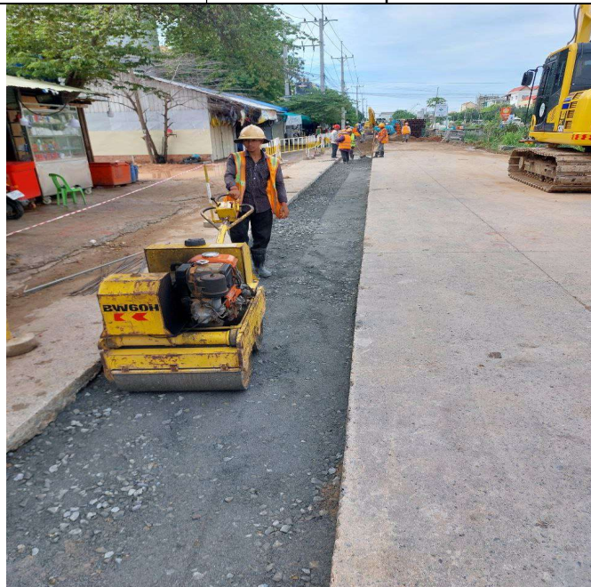
Base course backfilling and compaction
