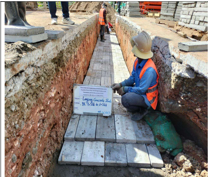
Photo: 07 Laying concrete protection slab and warning tap
