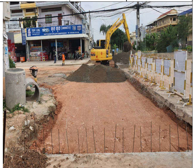
Base course backfilling and compaction
