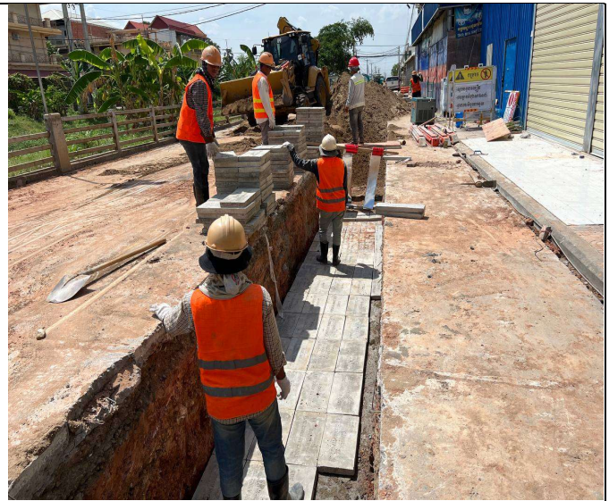
Photo: 02 Laying concrete protection slab and warning tap
