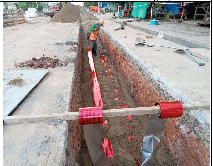
Photo: 06 Laying concrete protection slab and warning tap
