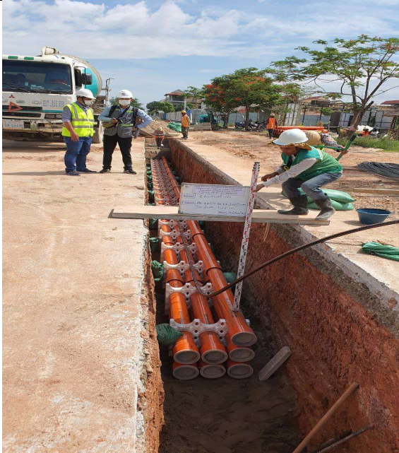
Photo: 19 CBS casting (mortar)
