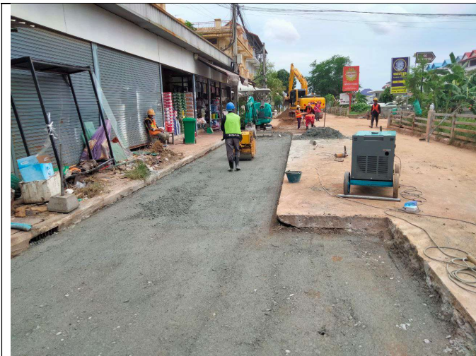
Base course backfilling and compaction
