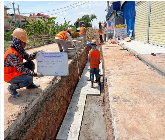
Photo: 01 Laying concrete protection slab and warning tap
