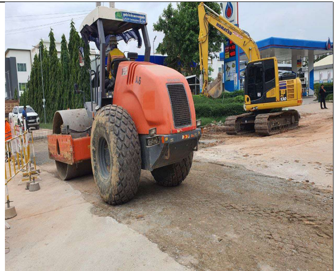
Base course backfilling and compaction
