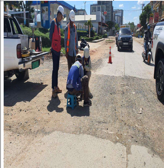
Density of base course backfilling and compaction
