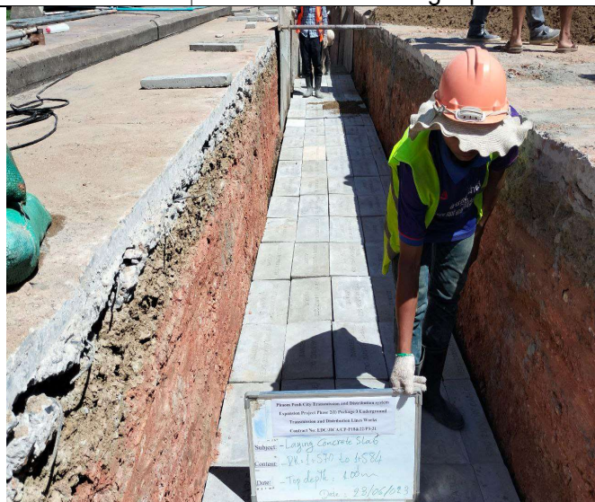
Photo: 11 Laying concrete protection slab and warning tap
