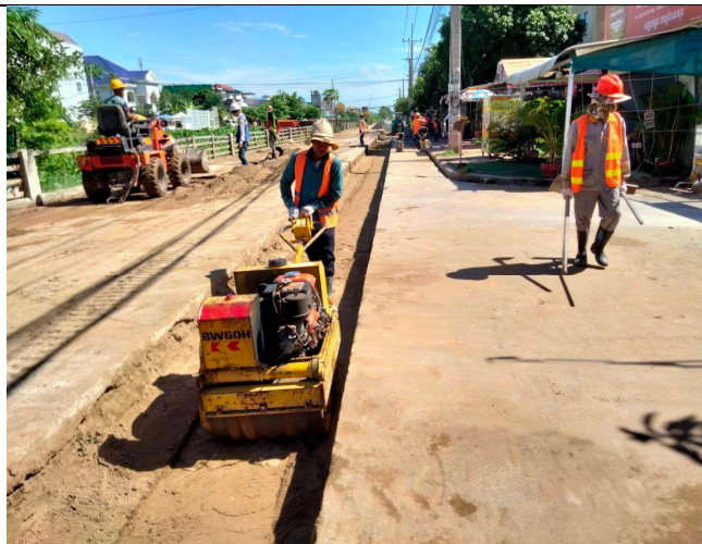
Photo: 12 Sand backfilling and compaction
