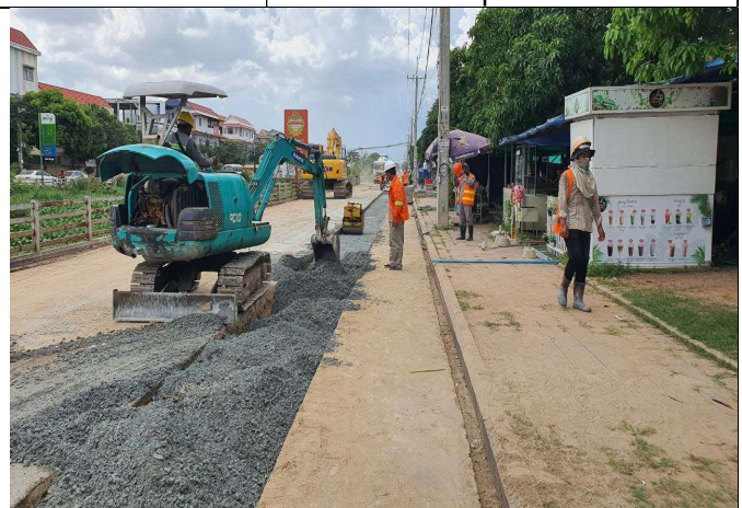
Base course backfilling and compaction
