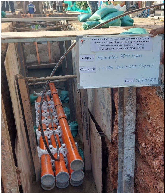
Photo: 04 Assembly PFP pipes and OFC pipe
