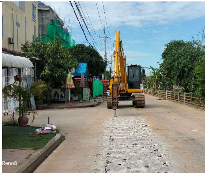
Demolition of concrete road
