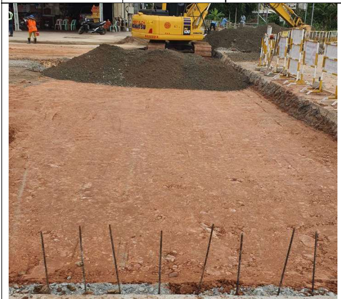
Base course backfilling and compaction
