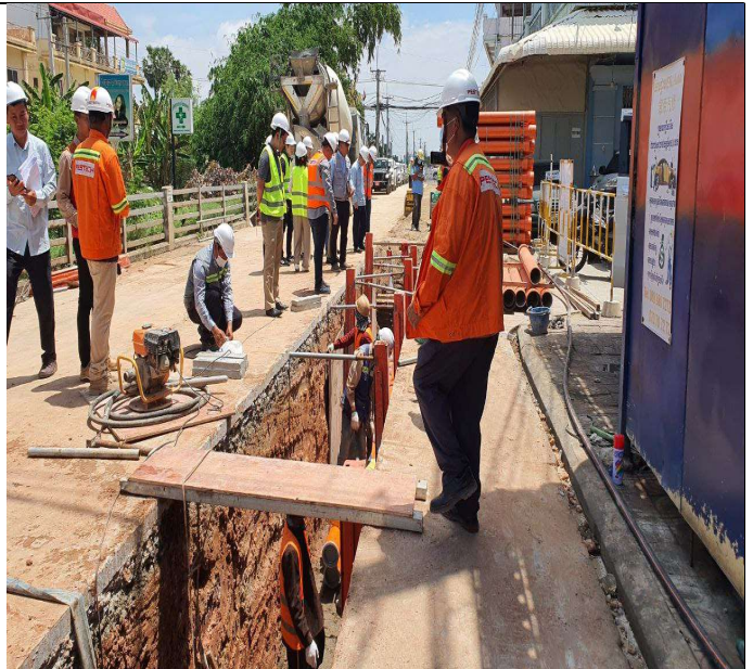
Photo: 16 Assembly PFP pipes and OFC pipe
