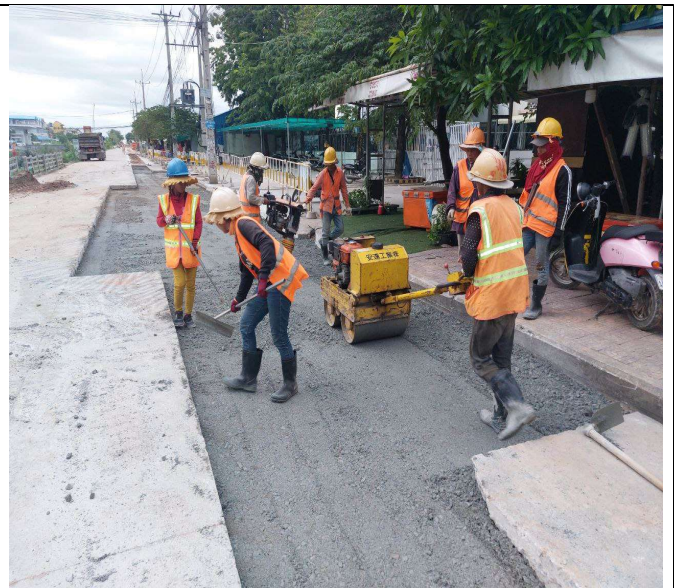
Base course backfilling and compaction
