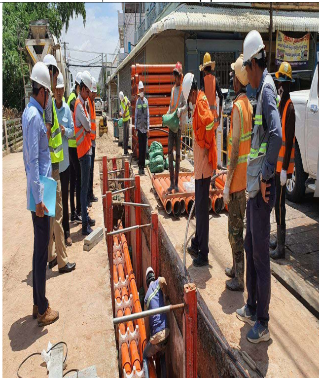
Photo: 17 Assembly PFP pipes and OFC pipe
