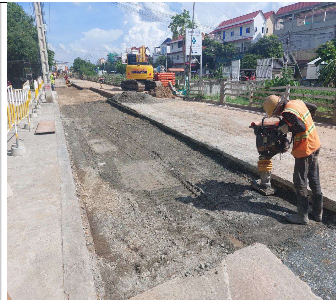
Base course backfilling and compaction
