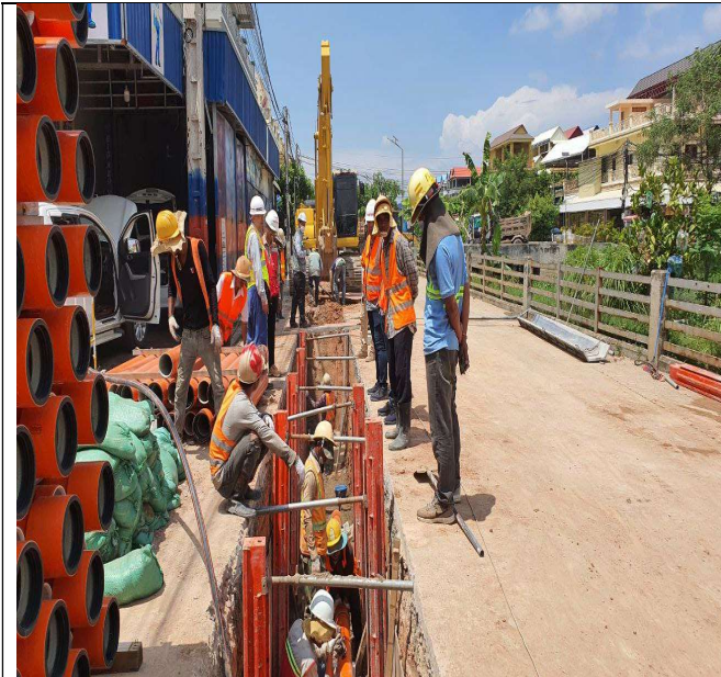
Photo: 15 Assembly PFP pipes and OFC pipe
