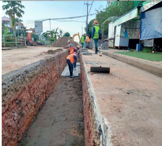
Photo: 09 Laying concrete protection slab and warning tap
