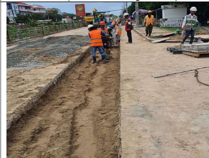
Photo: 13 Sand backfilling and compaction
