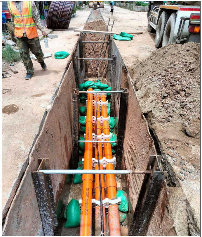
Photo: 02 Assembly PFP pipes and OFC pipe
