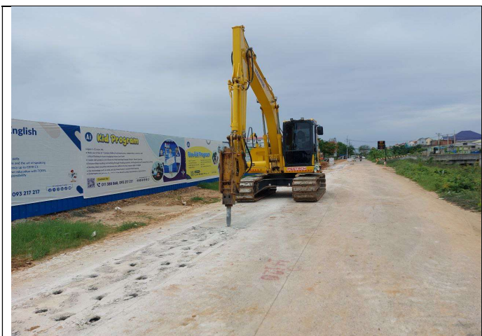
Photo: 01 Demolition of concrete road
