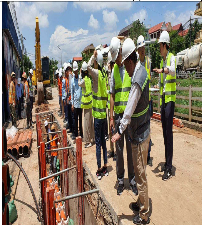
Photo: 18 Assembly PFP pipes and OFC pipe
