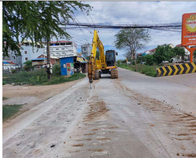
Demolition of concrete road
