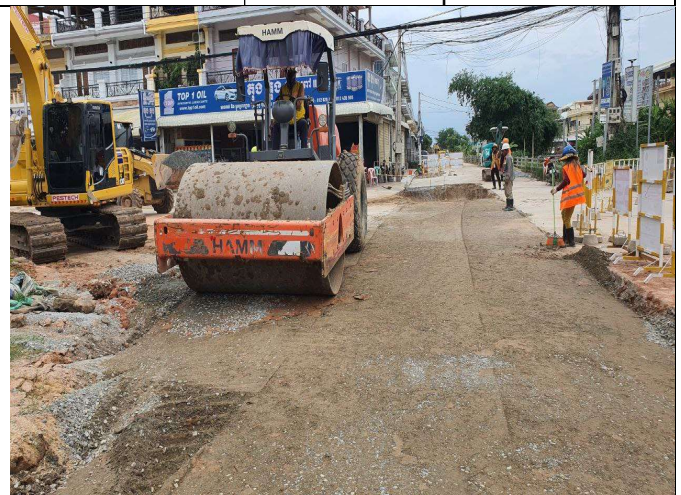
Base course backfilling and compaction
