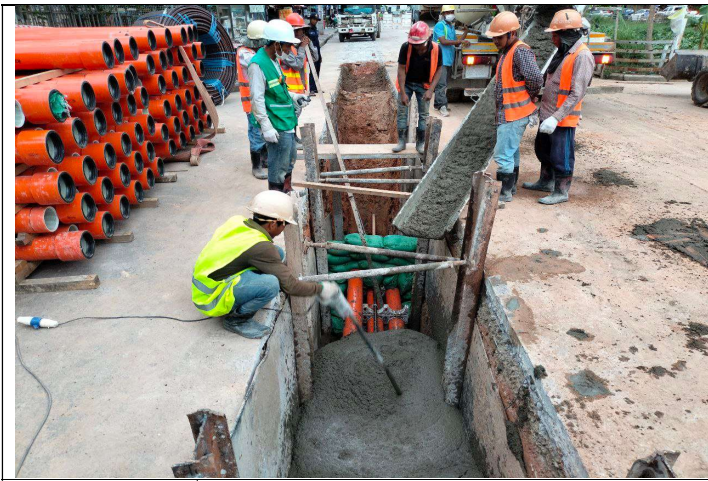
Photo: 17 CBS casting (mortar)
