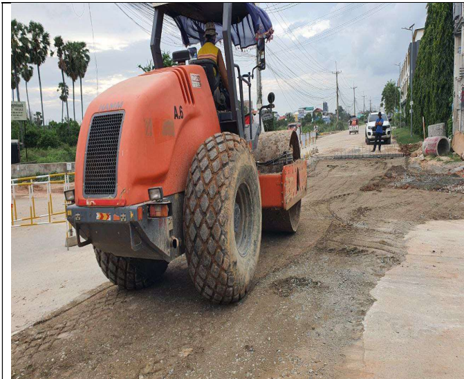
Base course backfilling and compaction
