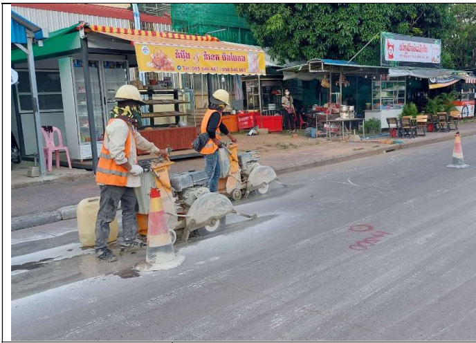
Photo: 07 Saw cutting of concrete road
