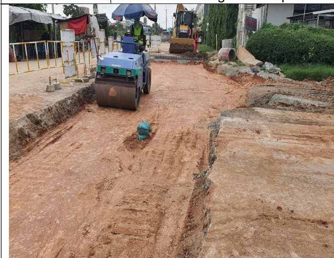
Photo: 05 Sand backfilling and compaction
