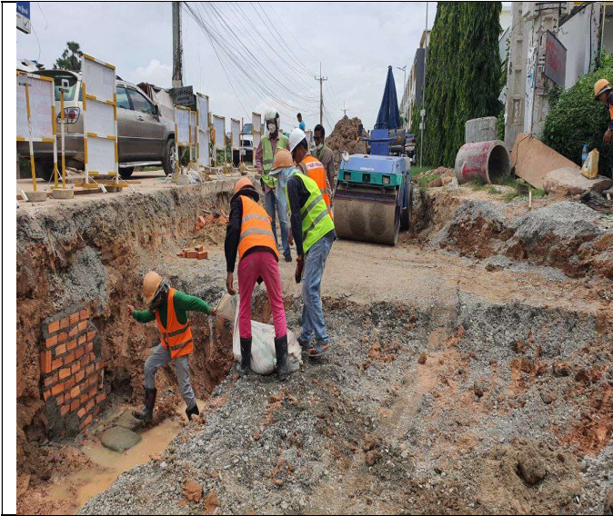
Photo: 01 Sand backfilling and compaction
