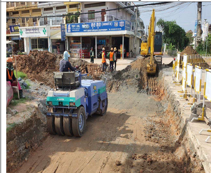
Photo: 03 Sand backfilling and compaction
