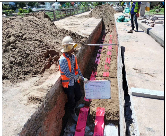
Photo: 12 Laying concrete protection slab and warning tap
