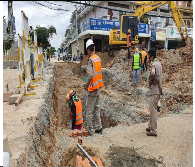
Photo: 02 Sand backfilling and compaction
