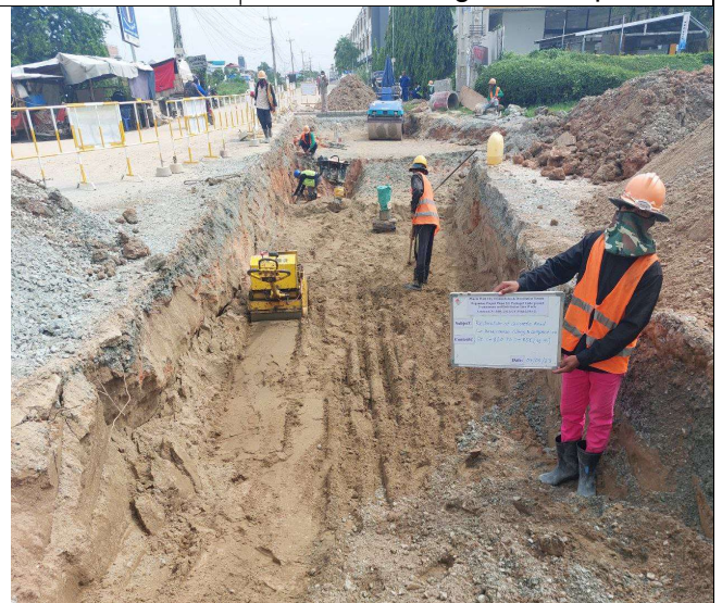
Photo: 04 Sand backfilling and compaction
