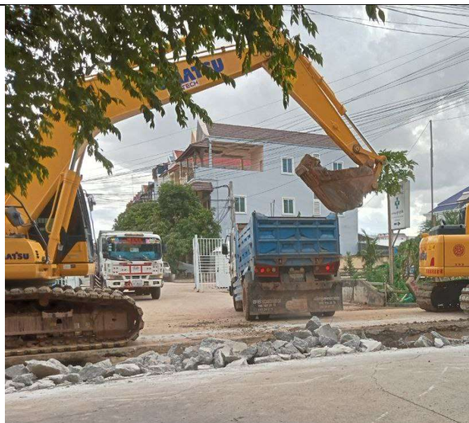
Photo: 06 Soil excavation and concrete road
