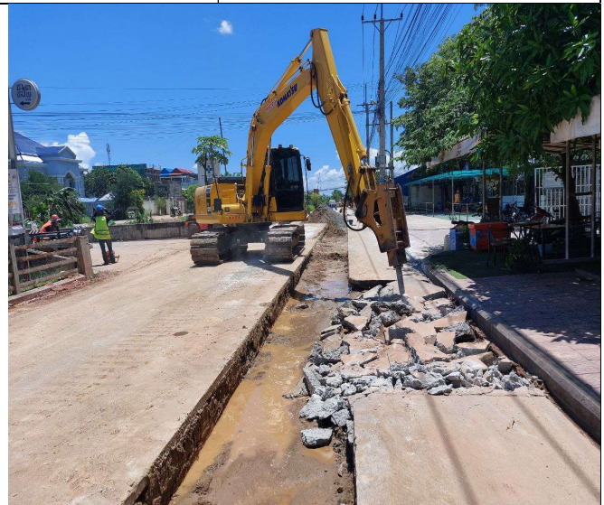
Demolition of concrete road
