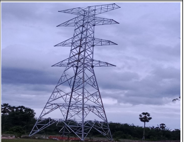
Tower erection TB24
