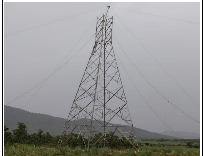
Tower erection TA176
