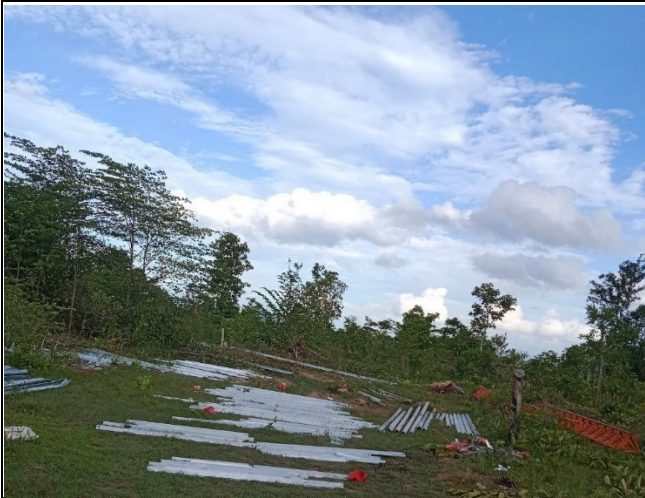
Tower erection TB25
