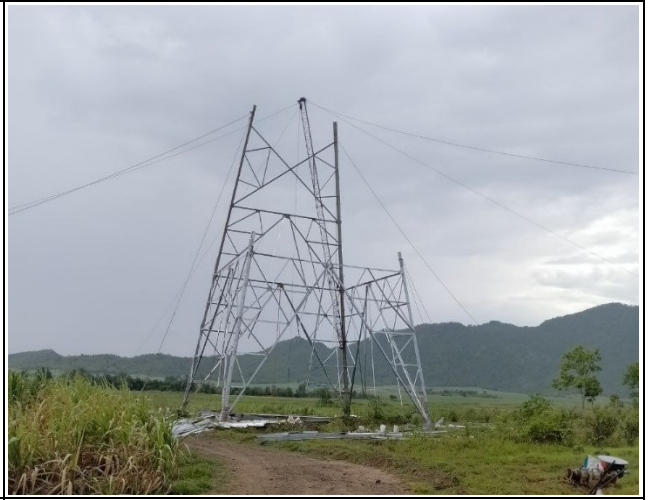
Tower erection TA147
