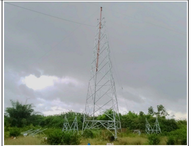
Tower erection TB17
