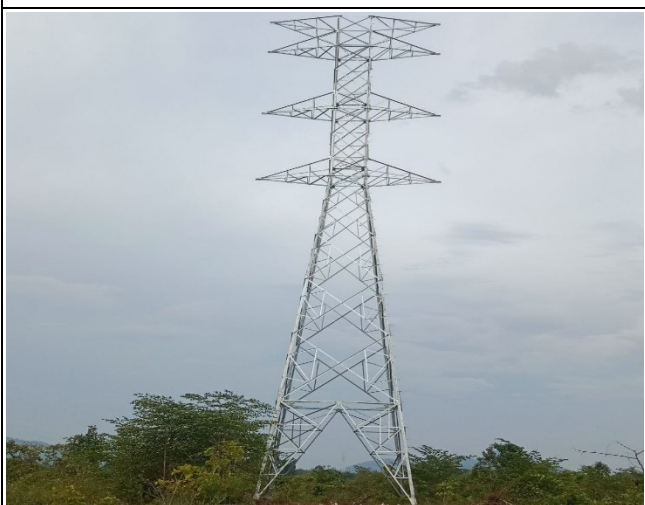
Tower erection TB25
