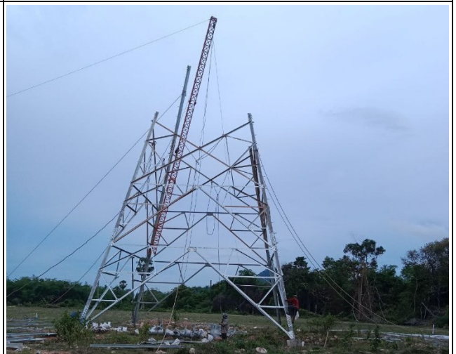
Tower erection TB37
