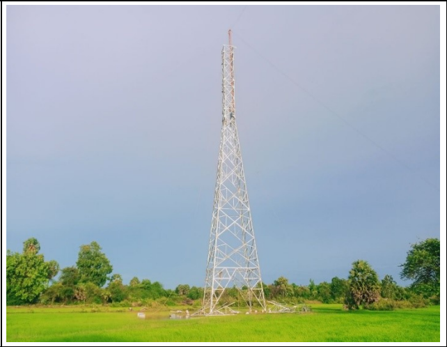
Tower erection TA50
