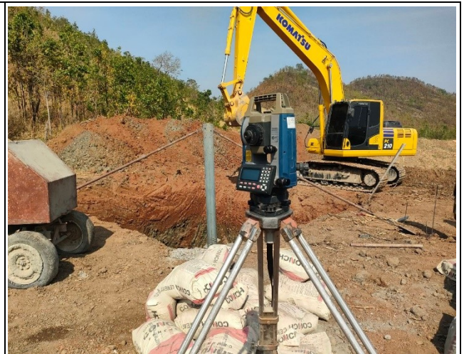
Stub setting of the leg A, B, C, D.
