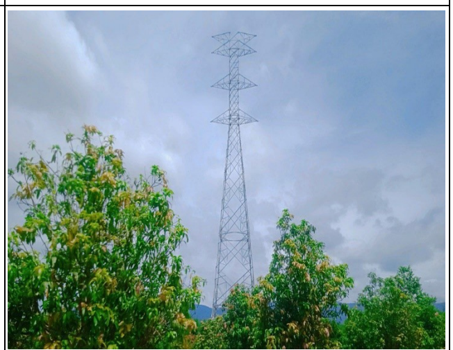
Tower erection TB20
