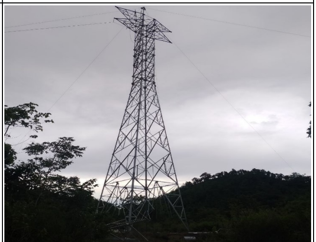
Tower erection TA144
