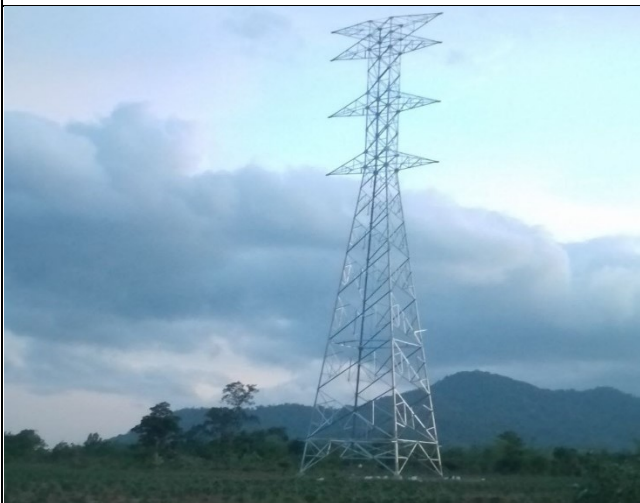
Tower erection TB22
