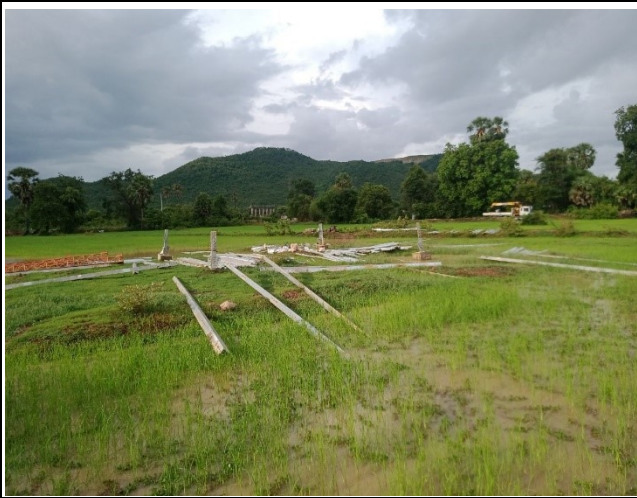
Tower erection TA50
