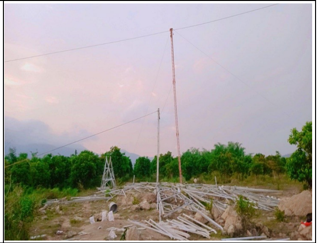
Tower erection TB20
