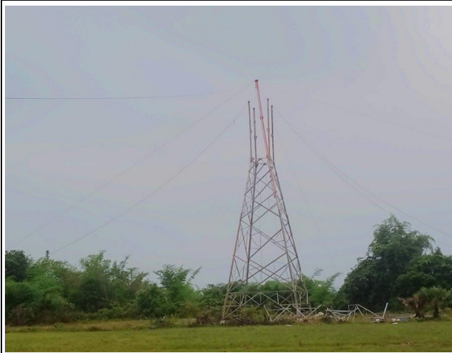
Tower erection TB16
