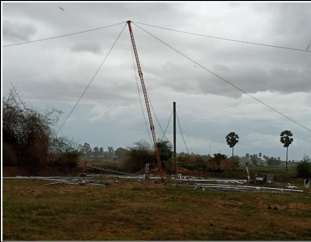
Tower erection TA33
