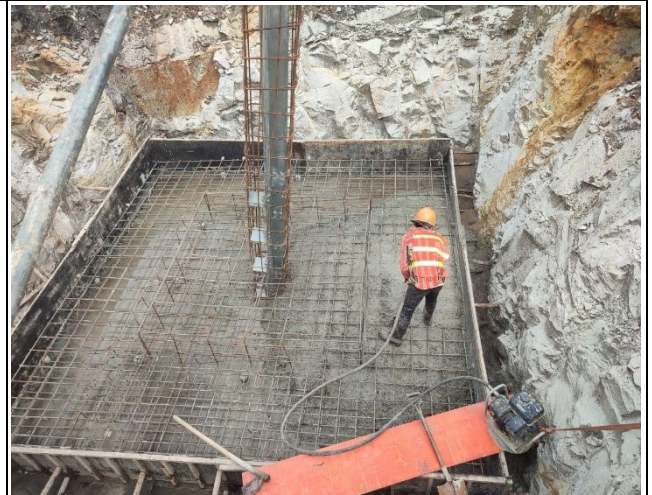
Casting base concrete of the leg A, B, C, D.
