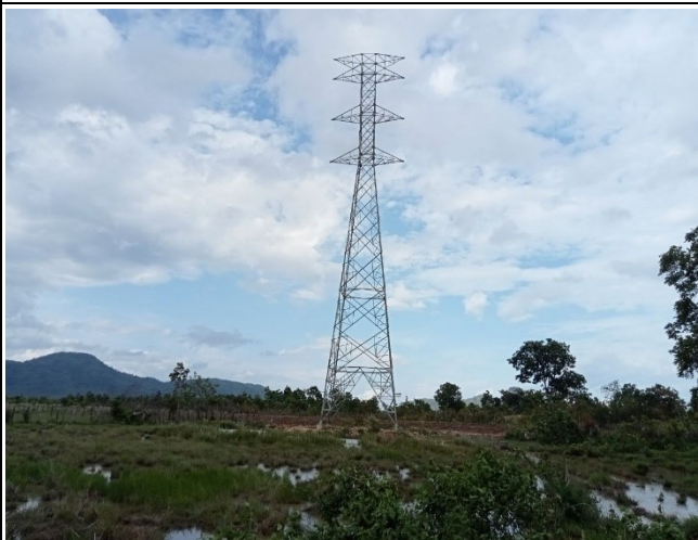
Tower erection TB18
