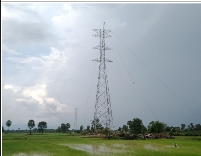
Tower erection TA52
