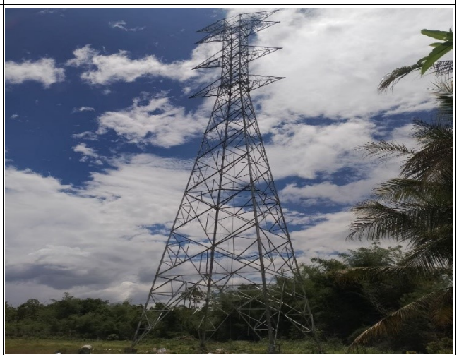
Tower erection TB37
