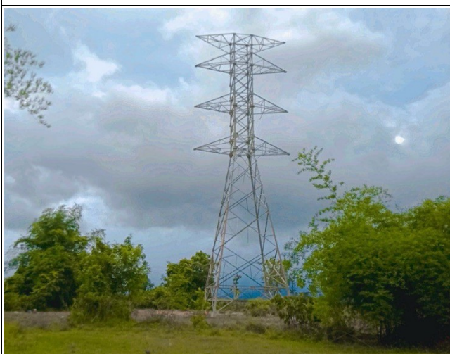
Tower erection TB16
