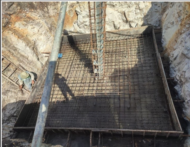
Base formwork installation of the leg A, B, C, D.
