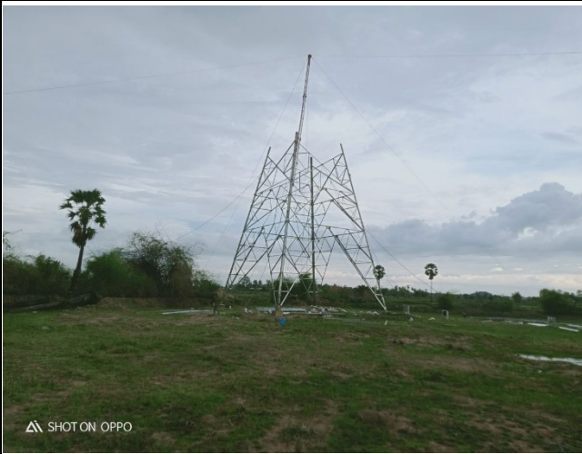
Tower erection TA33
