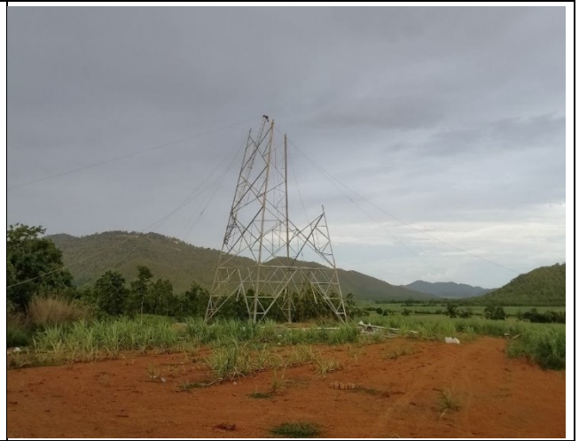
Tower erection TA176
