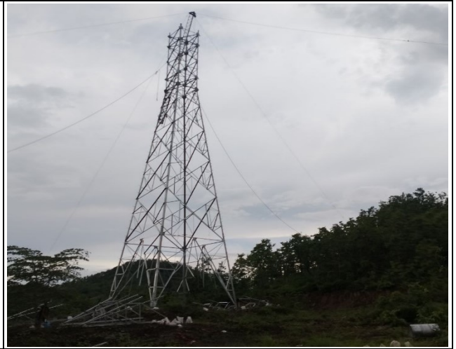
Tower erection TA146
