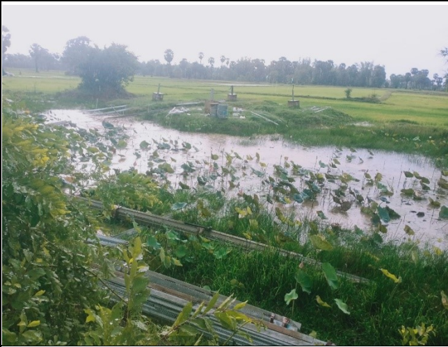
Tower erection TA51
