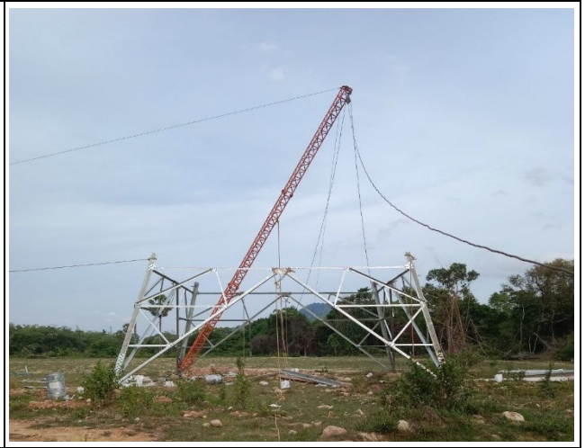
Tower erection TB37
