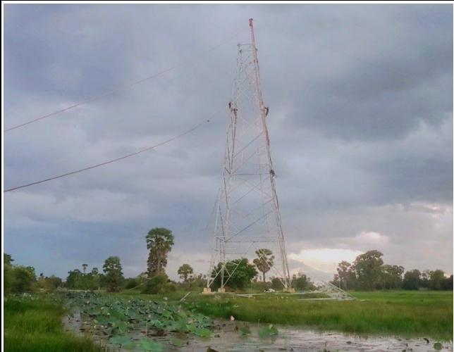
Tower erection TA51
