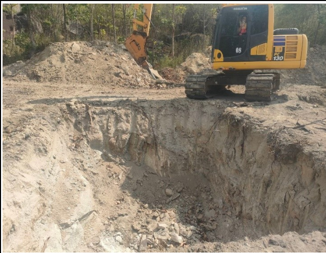
Soil excavation of the leg A, B, C, D.
