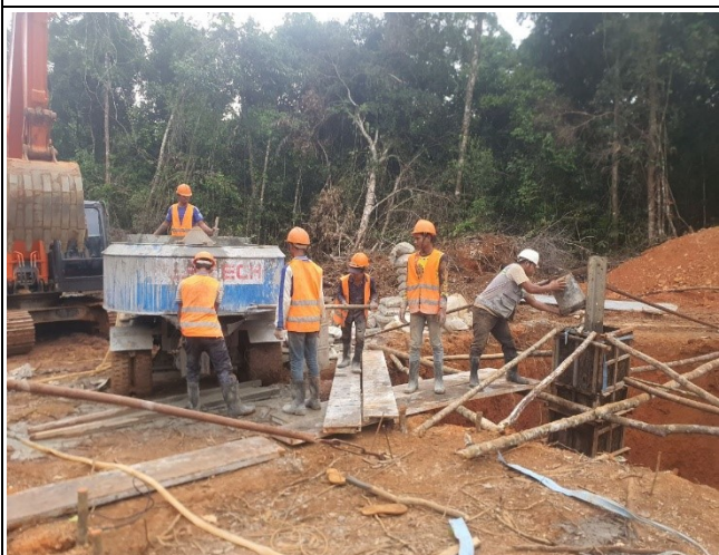
Casting chimney concrete of the leg A, B, C, D.
