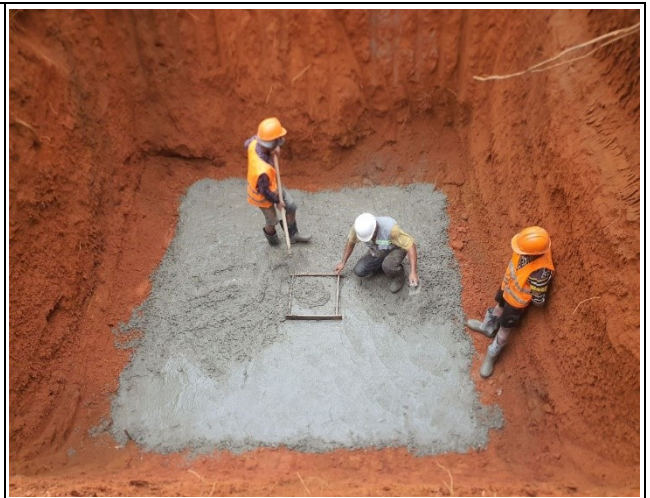
Lean concrete of the leg A, B, C, D.
