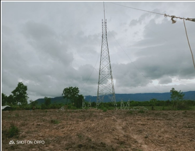
Tower erection TB18
