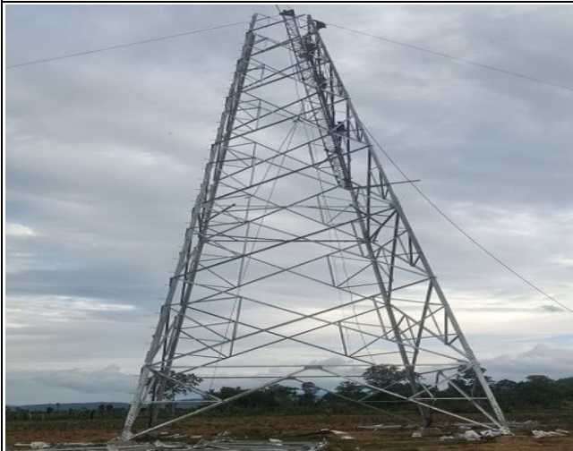
Tower erection TB22
