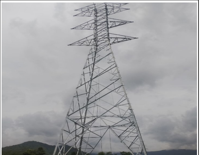
Tower erection TB24
