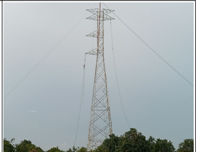
Tower erection TB20
