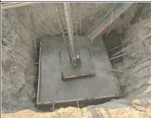
Casting base concrete of the leg A, B, C, D.
