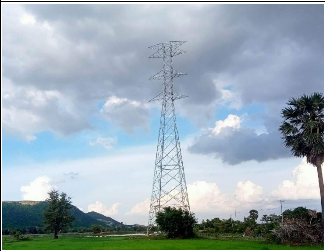
Tower erection TA51
