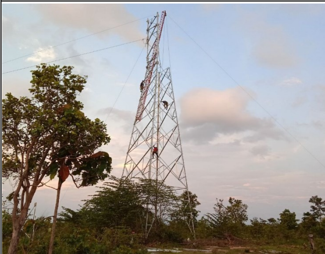
Tower erection TB25
