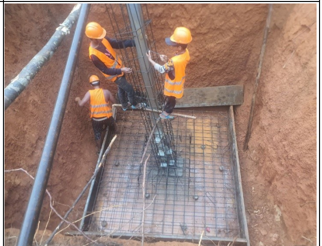
Rebar arrangement of the leg A, B, C, D.
