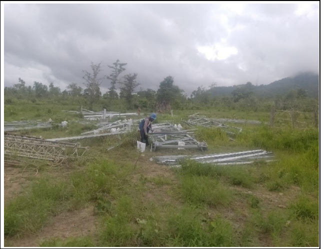
Tower erection TB24
