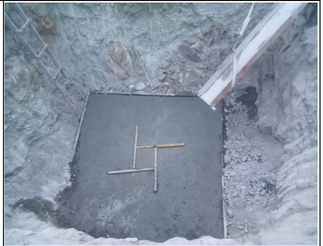
Casting lean concrete of the leg A, B, C, D.
