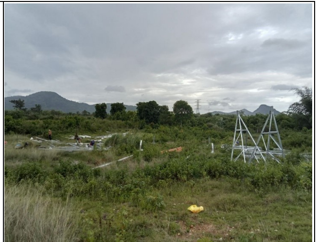
Tower erection TB17
