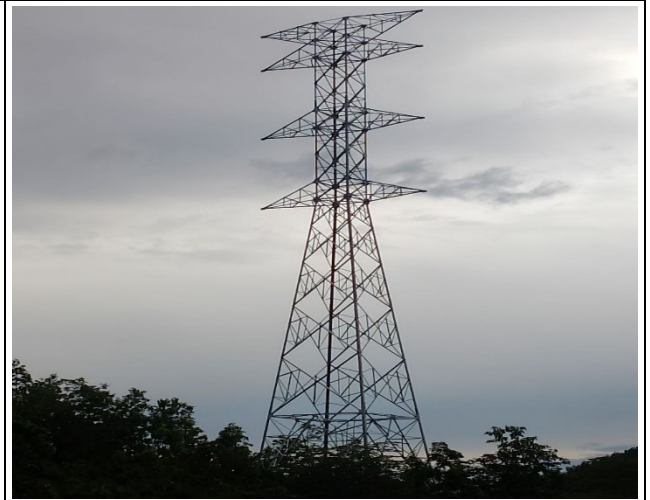
Tower erection TA146
