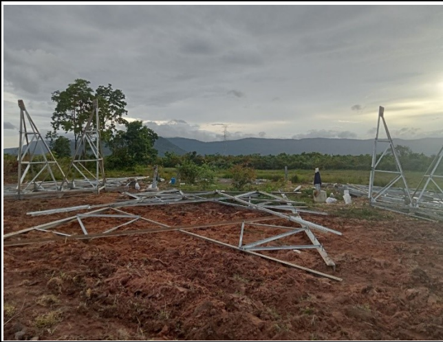
Tower erection TB18
