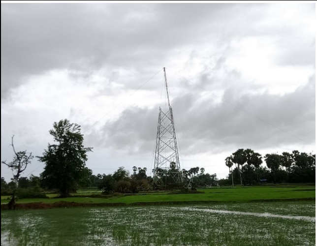
Tower erection TA52
