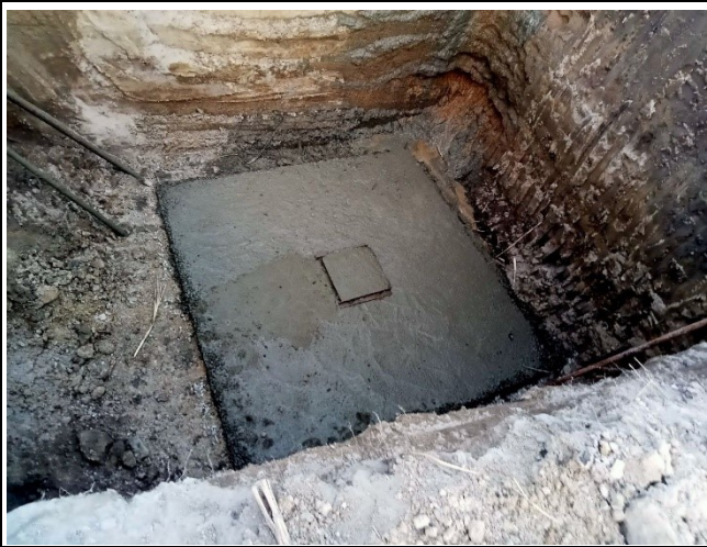
Casting lean concrete of the leg A, B, C, D.
