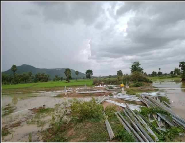
Tower erection TA52
