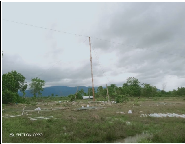
Tower erection TB16
