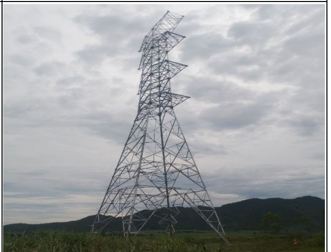
Tower erection TA147
