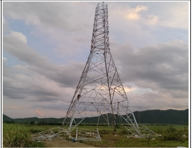
Tower erection TA147
