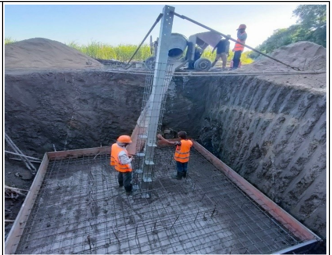
Base rebar installation of the leg A, B, C, D.
