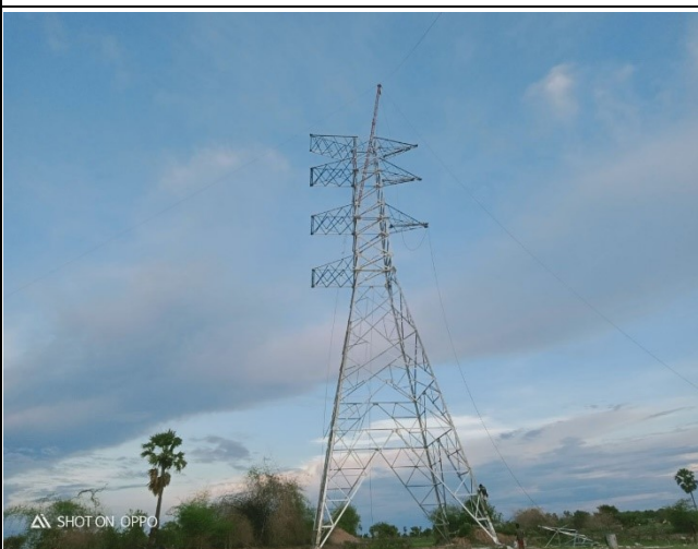
Tower erection TA33
