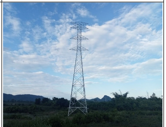
Tower erection TB17
