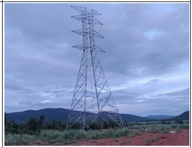
Tower erection TA176
