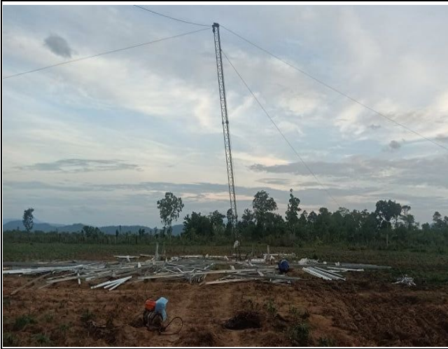
Tower erection TB22
